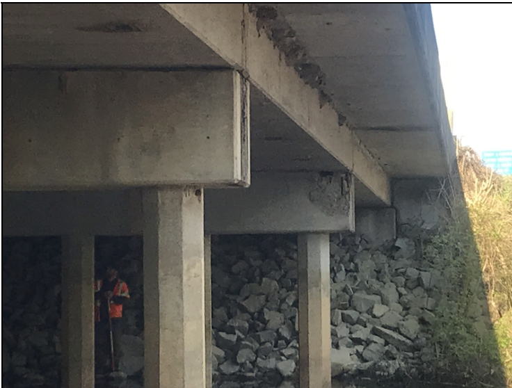
Bent 2 cap large spall with exposed rebar.
