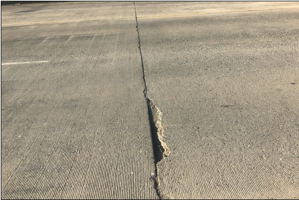
Span 3 Bent 4 spall
