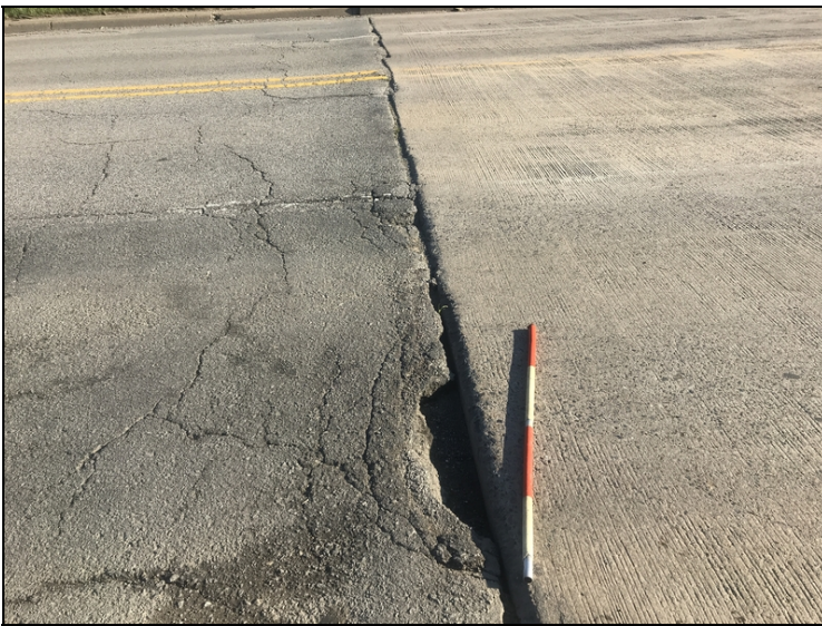
Pothole in asphalt approach at west end of the bridge.
