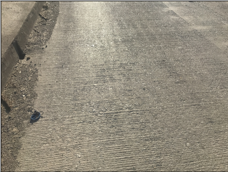
Span 2, longitudinal cracks in top up slab.
