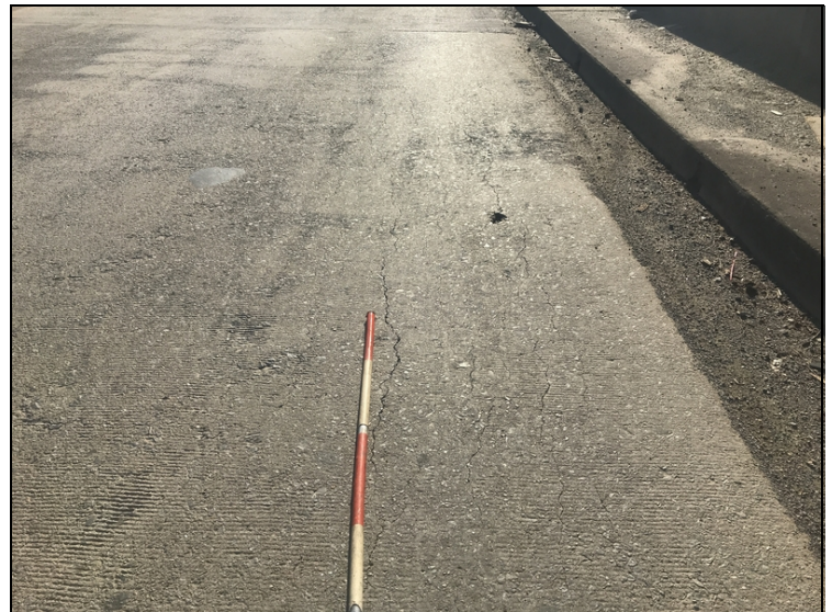
Span, longitudinal cracks in top of slab.
