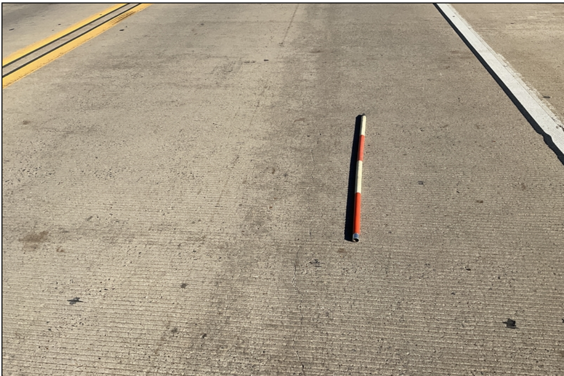
Span 6: multiple unsealed longitudinal cracks
