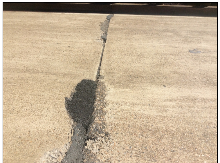
Joint at bent 1 is partially filled with asphalt.
