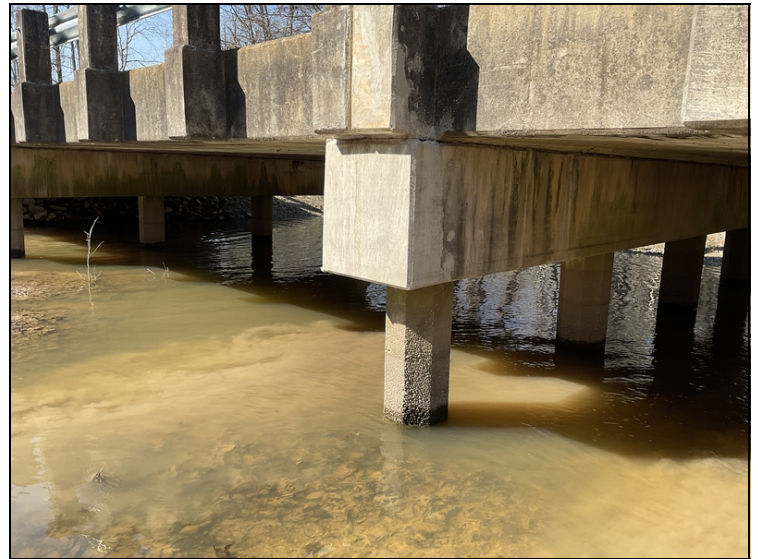
Bent 2: left end of cap has been repaired by contractor 2022.
