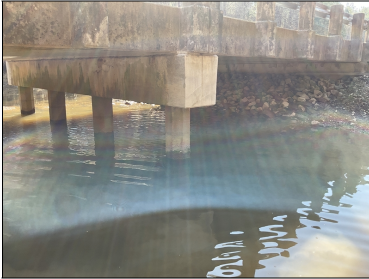
Bent 3: left side of cap has been repaired.
