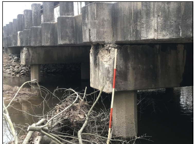
Bt. 2 & Bt. 3, left ends of caps have spalls with exposed rebar. Bt. 3 right end is similar.
