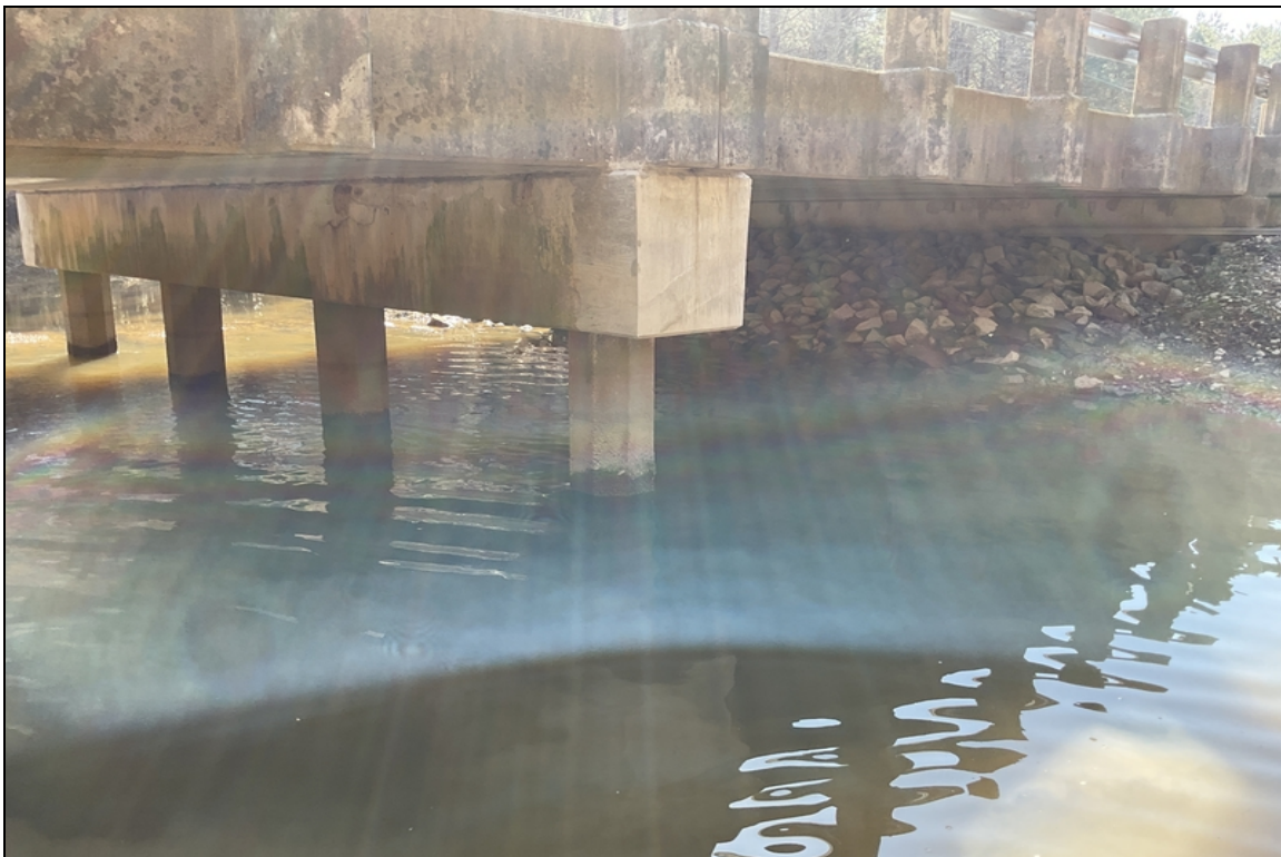
Bent 3: left side of cap has been repaired.
