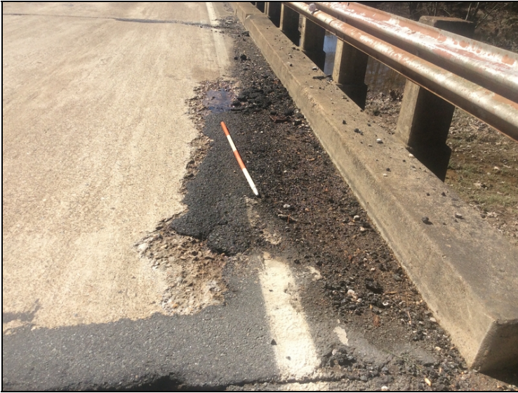
Span 1 right lane failed asphalt patch.
