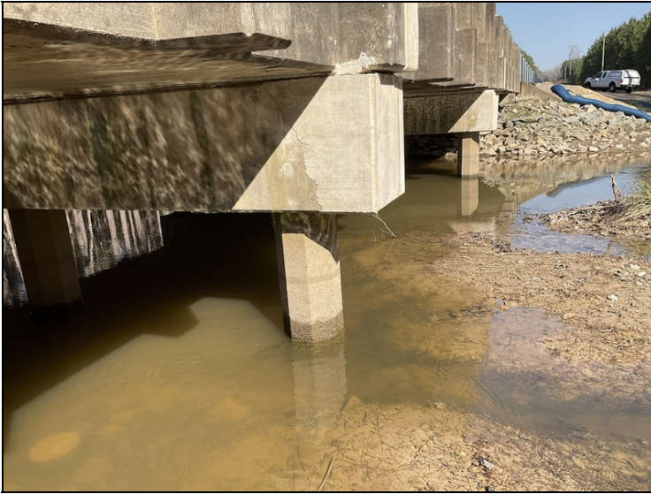
Bent 3: left end of cap has been repaired by contractor
