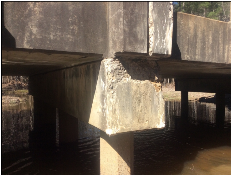
Bent 3 left side has spalls with efflorescence.
