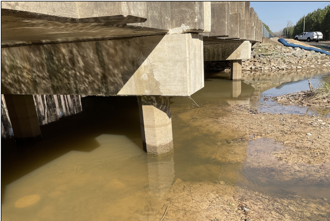
Bent 3: left end of cap has been repaired by contractor
