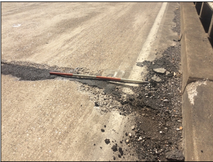
Span 1 failed asphalt patch at joint.
