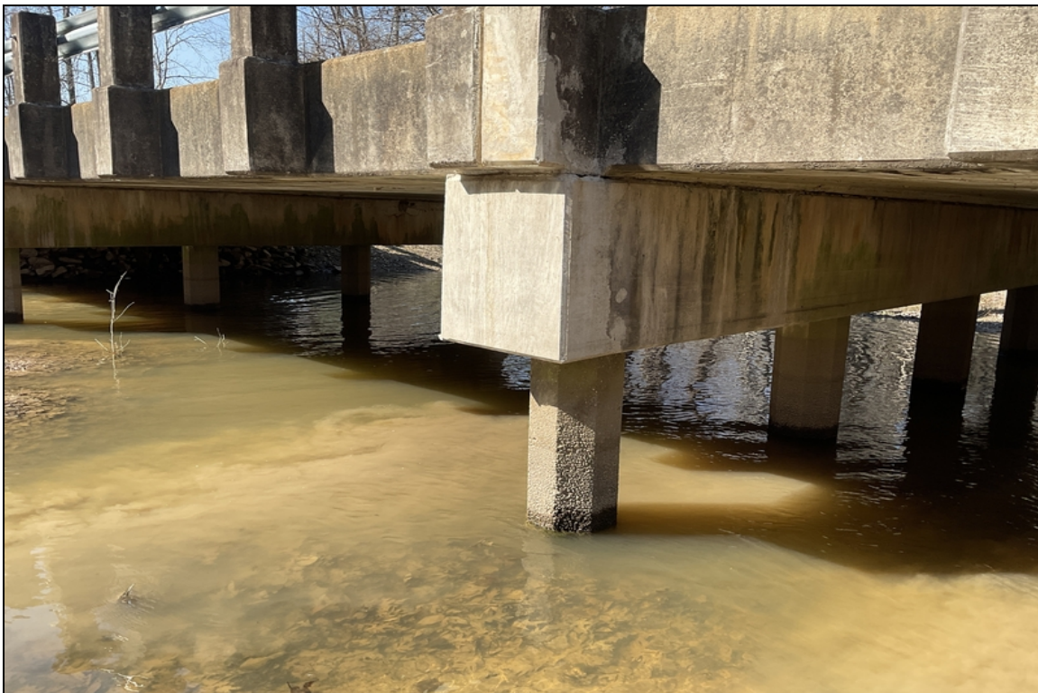
Bent 2: left end of cap has been repaired by contractor 2022.
