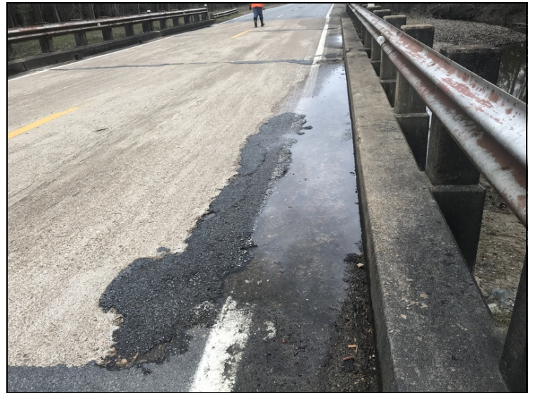
Spalls filled with asphalt, heavy scaling, joint seal missing.
