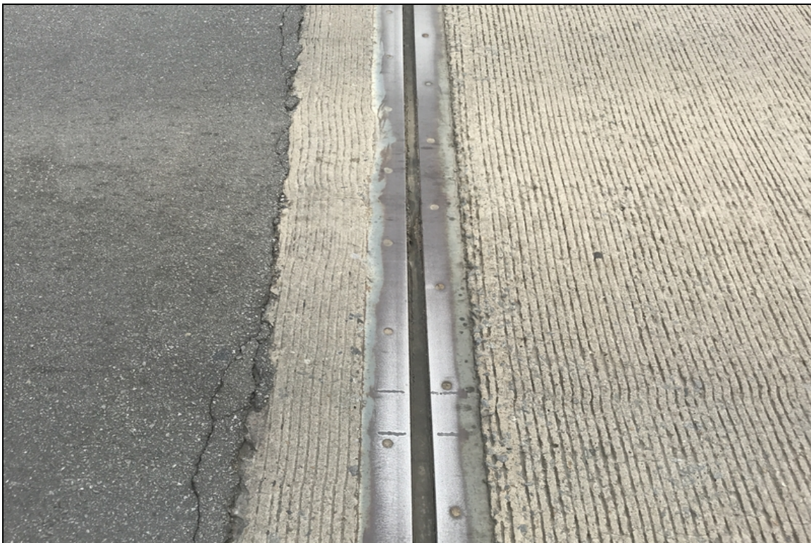
Bent 1: joint seal is losing bond allowing water to seep through.
