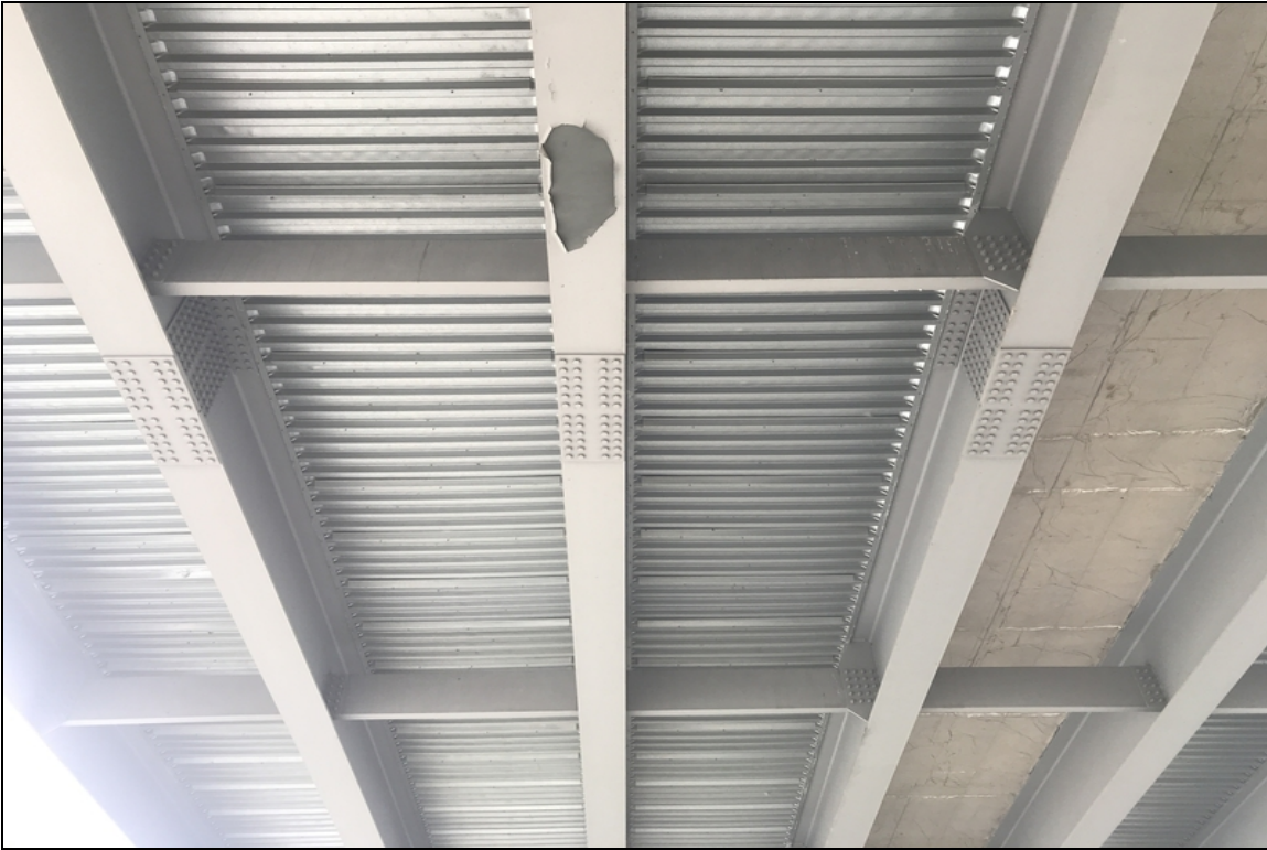
Span 3, girder 3: Area of paint is peeling.
