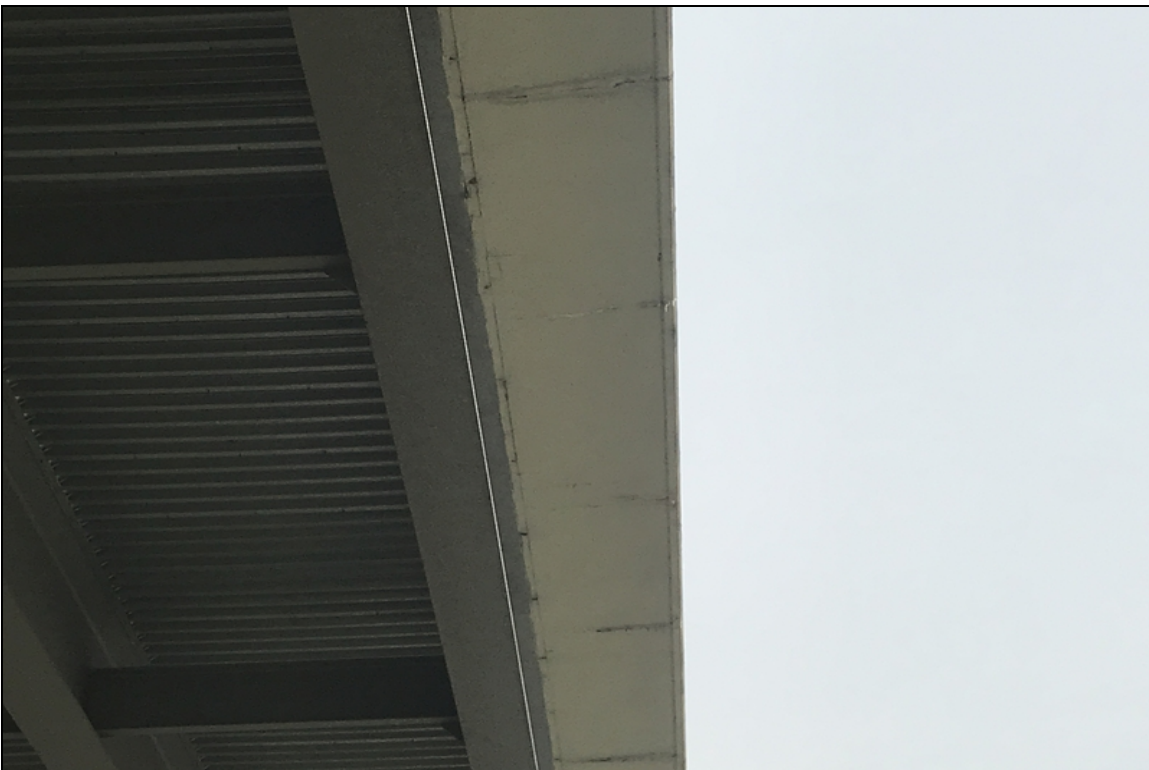
Overhang with numerous transverse cracks with efflorescence build up.
