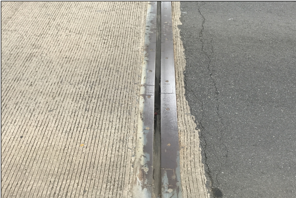
Bent 5: Joint seal has lost bond in numerous locations.
