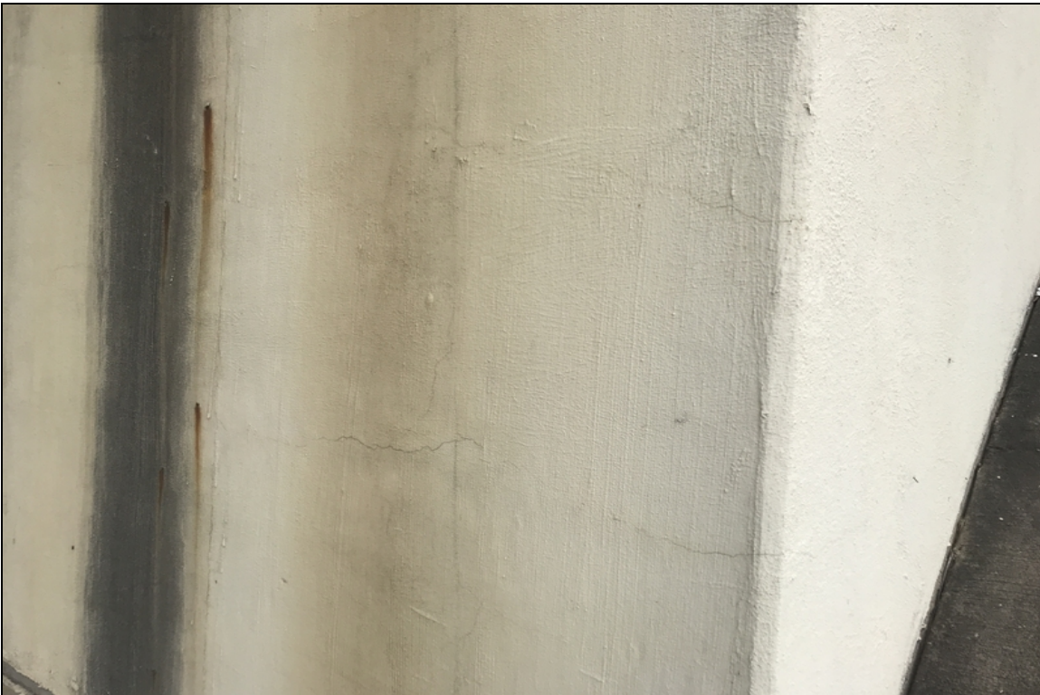
Bent 5 has horizontal cracking
