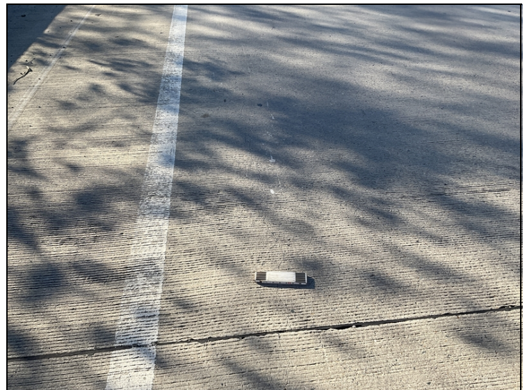
Span 2: Unsealed deck cracks up to 0.030 inch. Common to all spans
