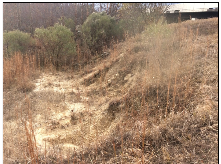
The emankment at the north end of the bridge on the right side has eroded, causing the side ditch to become partially blocked.
