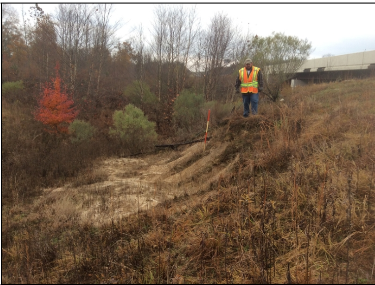
Looking south at the north end of the bridge on the right side. The embankment has eroded and caused the side ditch to become partially blocked.
