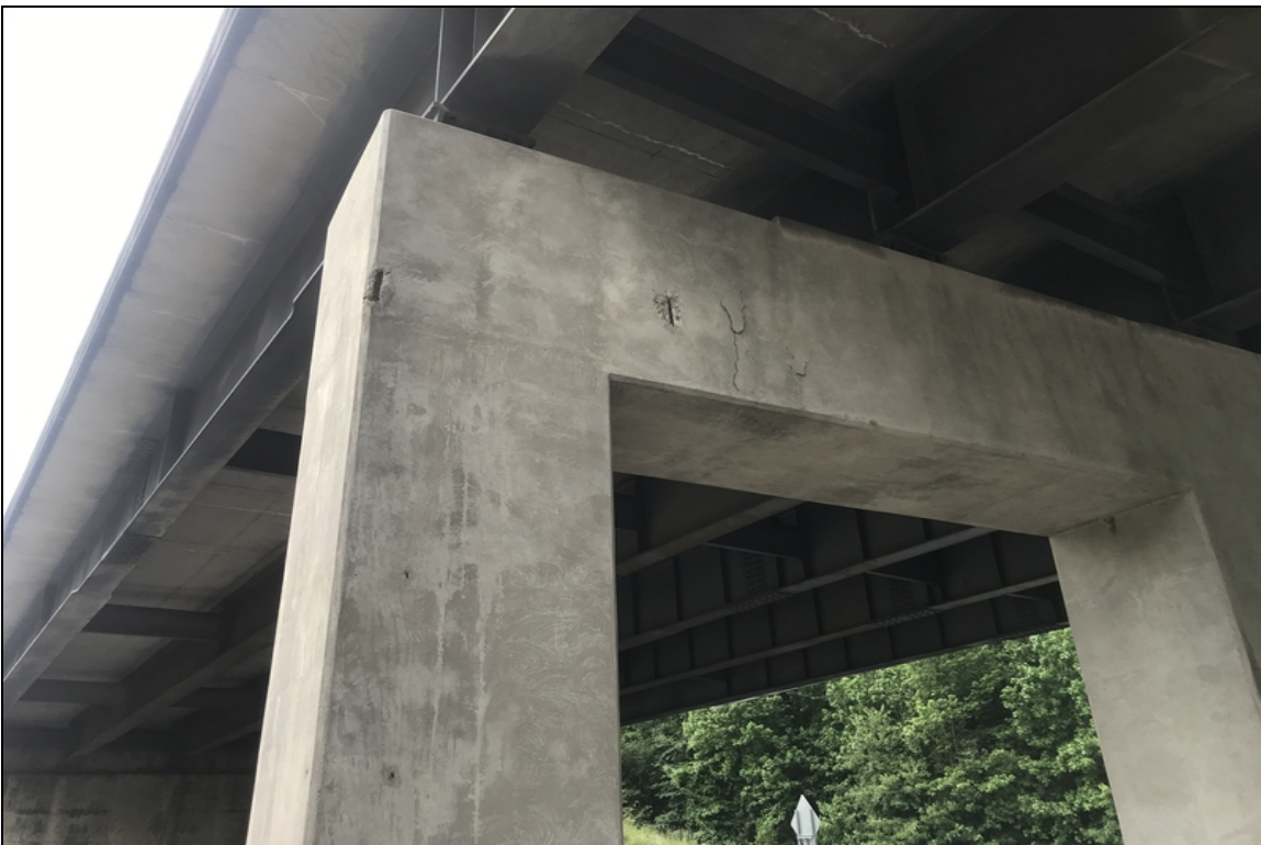
Ahead side of bent 2: a couple of spalls with exposed rebar
