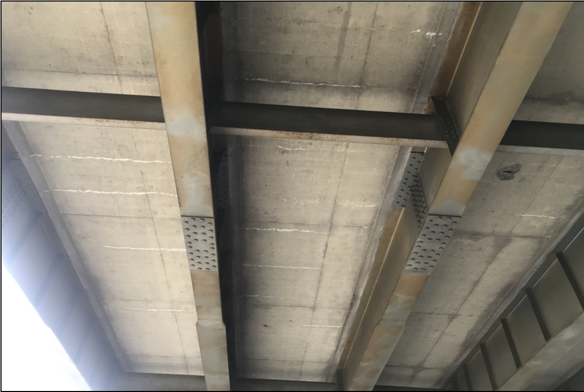
Span 1: scattered transverse cracks with efflorescence staining
