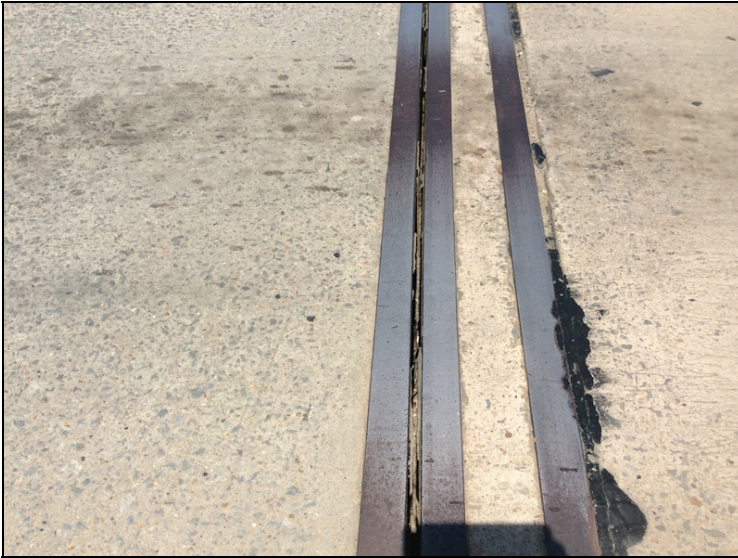
Joint material is missing at Bt. 1 & 3.
