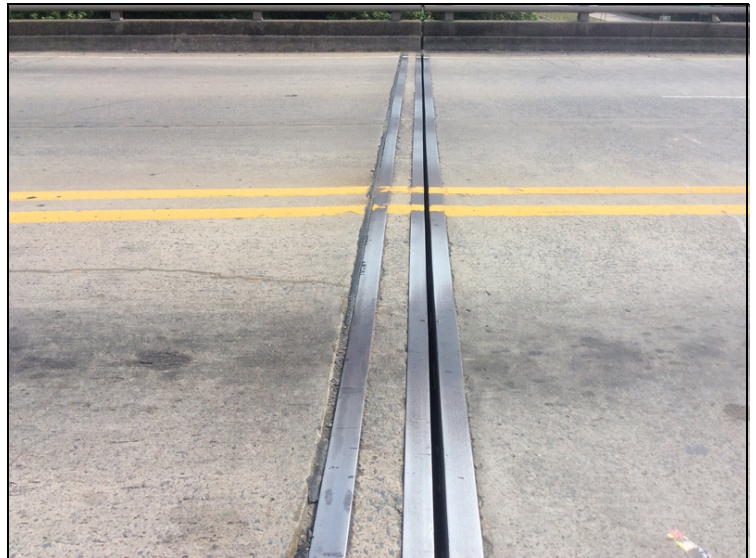
Bent 3 joint seal is missing.
