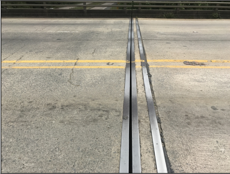
Bent 1: joint seal missing
