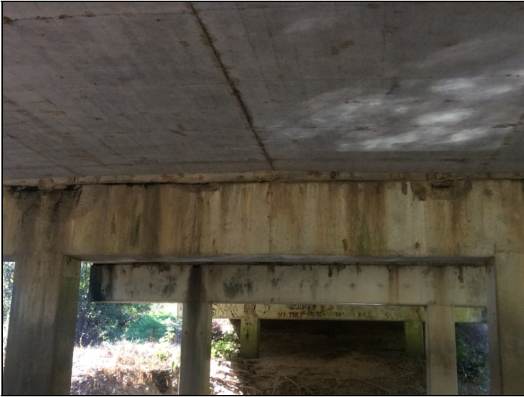
Bent 4 cap ahead spalls with exposed rebar.
