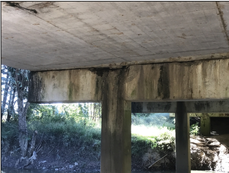
Ahead side of bent 4 with couple large spalls with exposed rebar.
