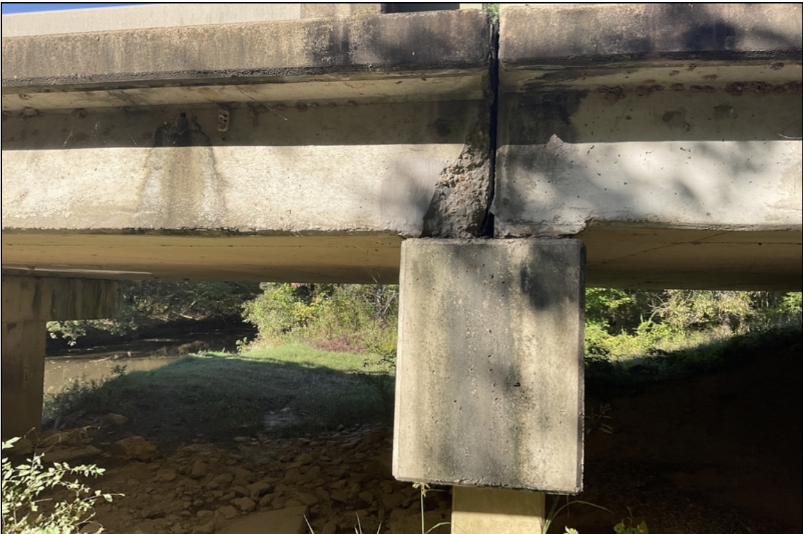
Spall on Right side of span 5 at bent 6
