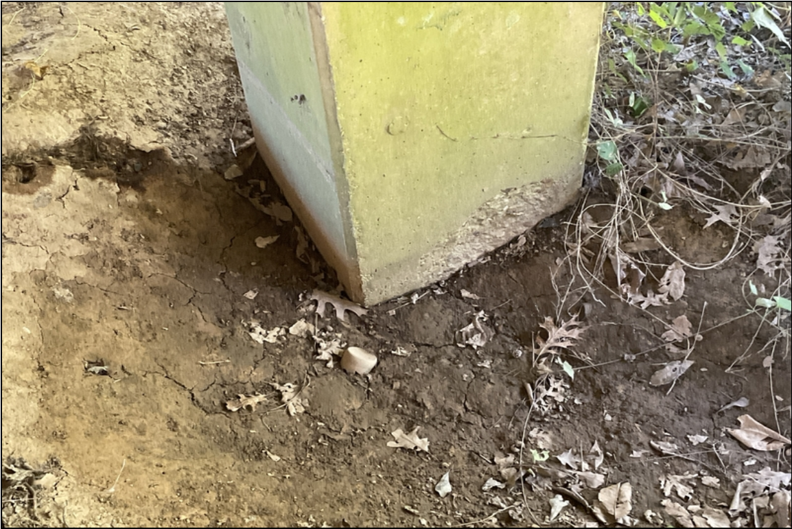
Bent 2 column 1 has a spall at ground line.
