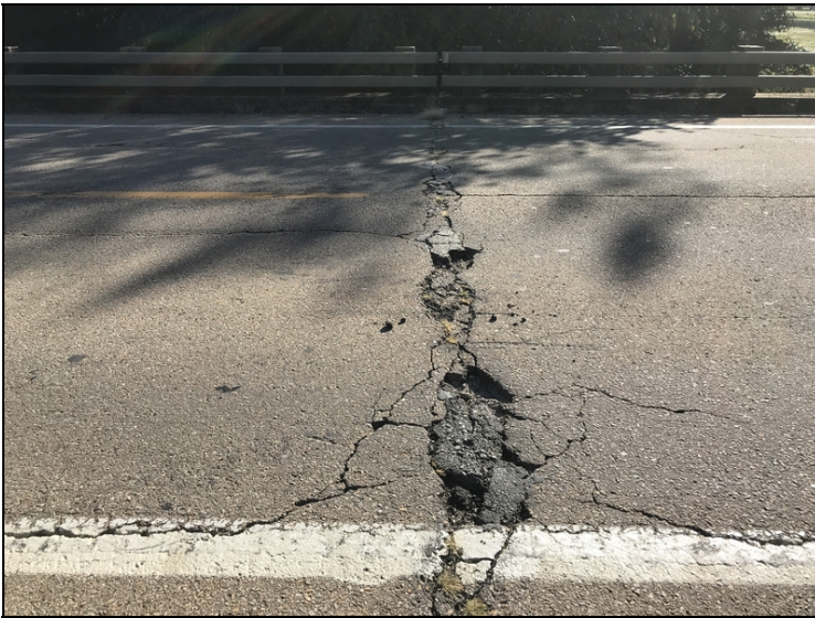
Bent 3: joint with open spalls in the asphalt overlay
