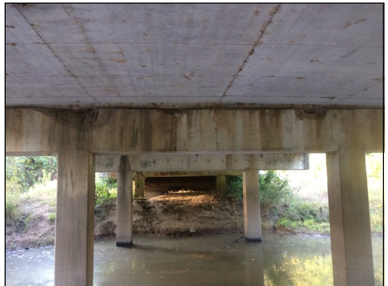
Bent 4 ahead side, looking back. Spalls and exposed rebar.
