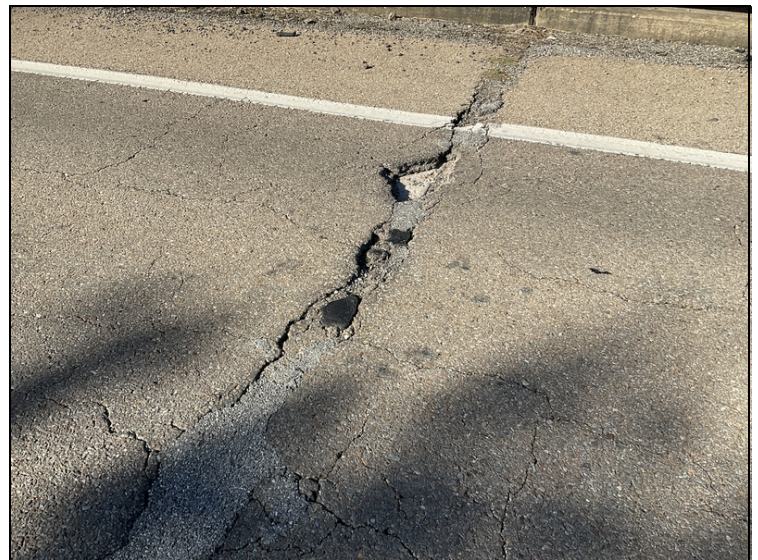
Bent 2 joint with open spalls in the asphalt overlay
