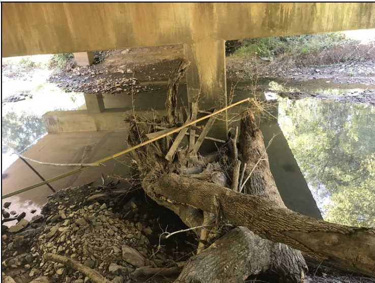
Bent 3: drift and debris build up around column 1
