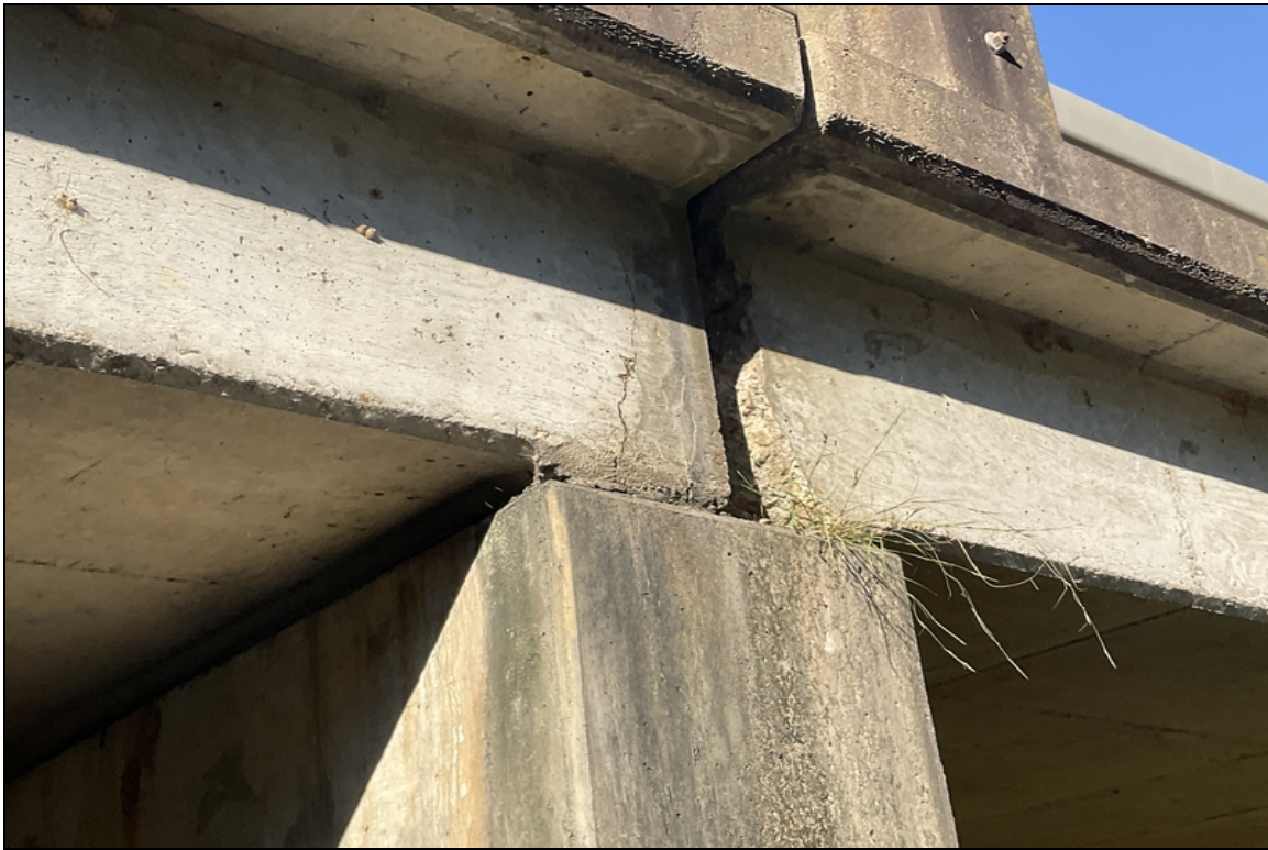
Spalls on the right side of spans 2&3 at bent 3.
