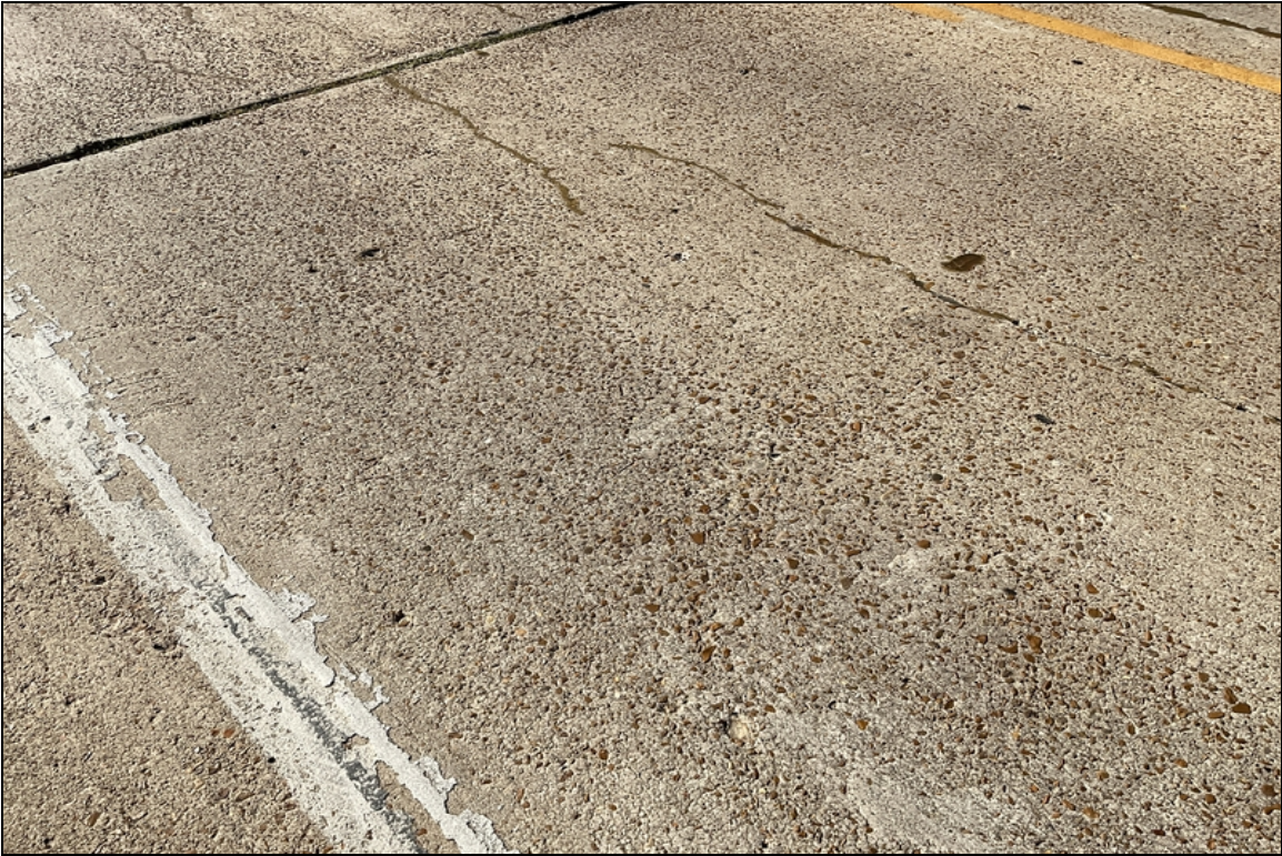
Span 3 abrasion
