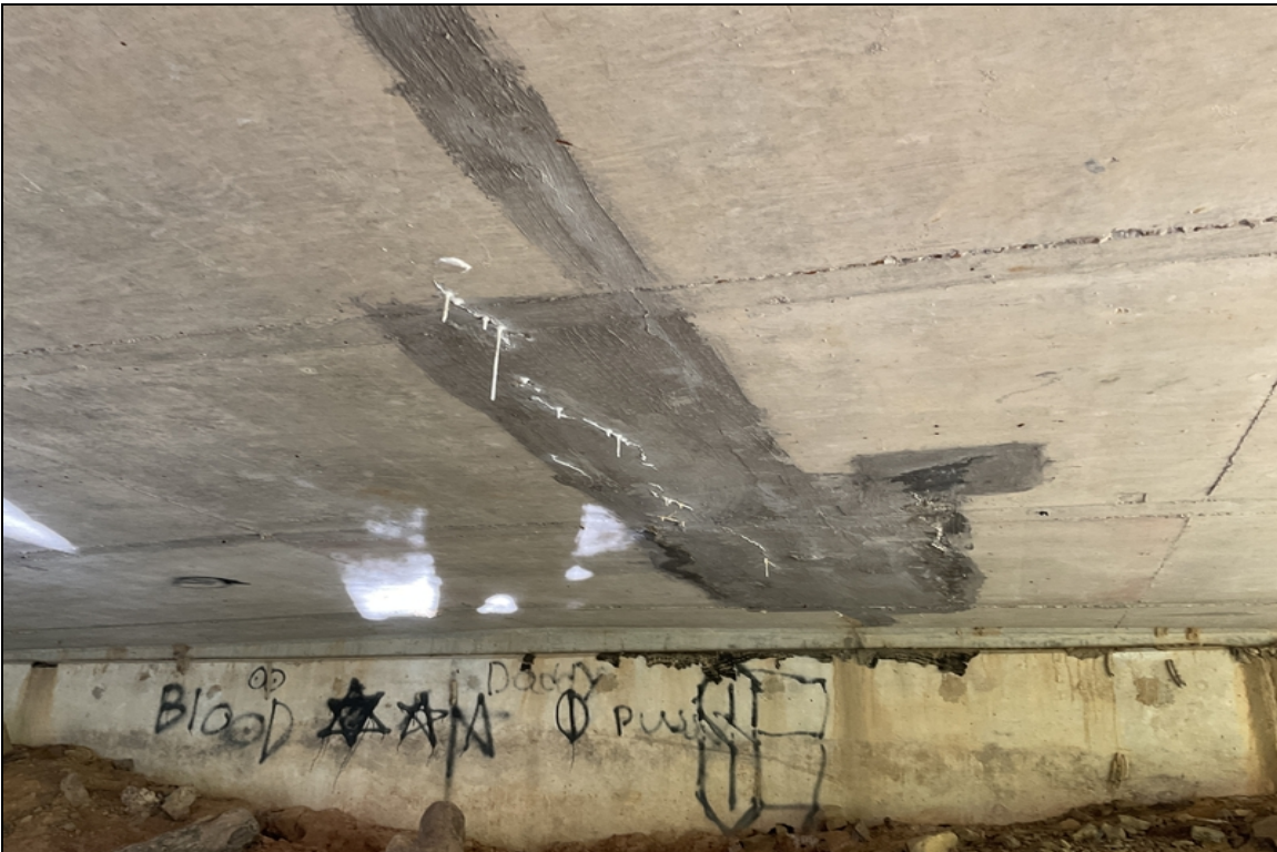
Span 3 efflorescence
