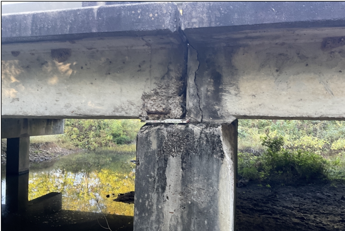
Right side of spans 2&3 over bent 3: spall and spall with exposed rebar
