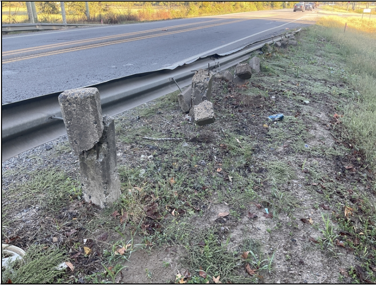
North side of the northbound lane: the approach rail is damaged and 7 of the posts are broken off allowing rebar to stick up.
