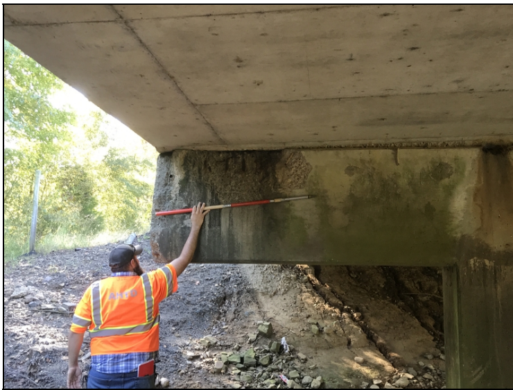
Ahead side of bent 2: large spall with exposed rebar
