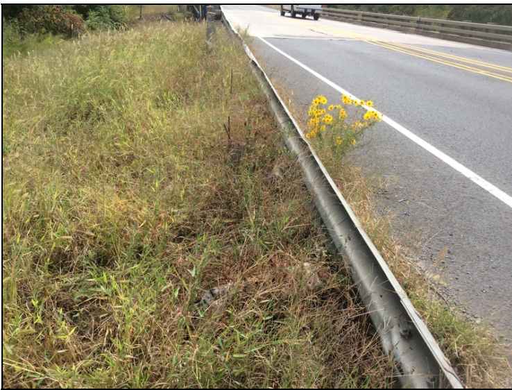
Looking southbound, the left approach rail has all of the posts and spacer block broken due to collision damage.
