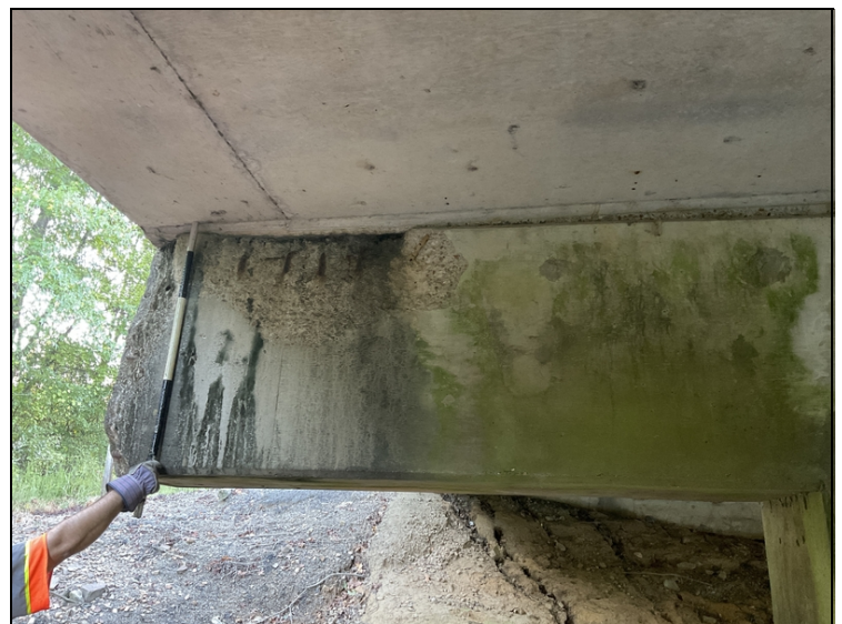
Bent 2 spall with exposed rebar on ahead face
