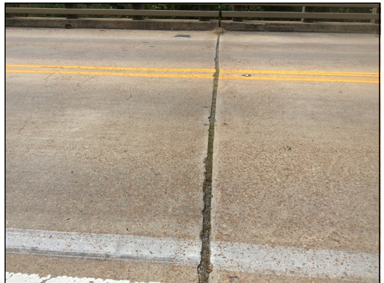
Bent 3 looking left. The joint seal is missing and the joint is 1 1/4" width and filled with debris.
