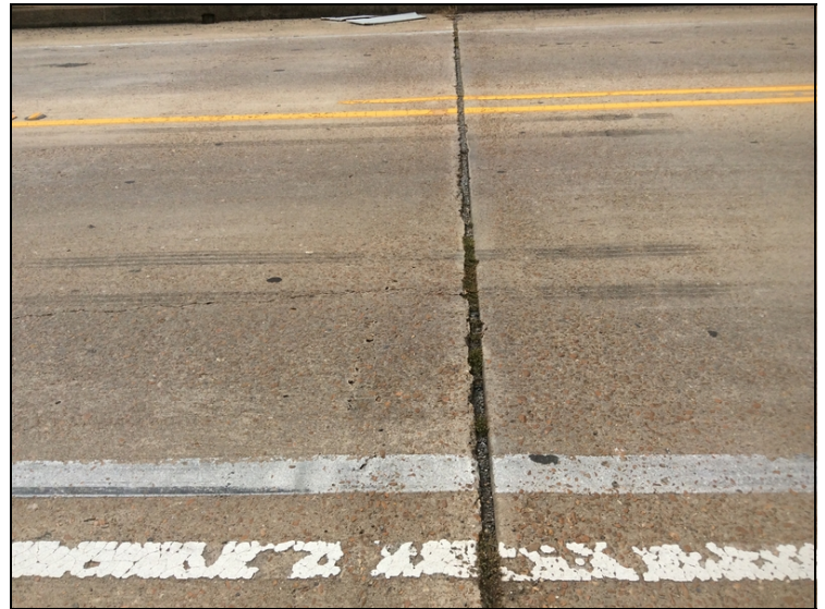
Bent 2, the joint seal is missing and impacted with debris. 1" width.
