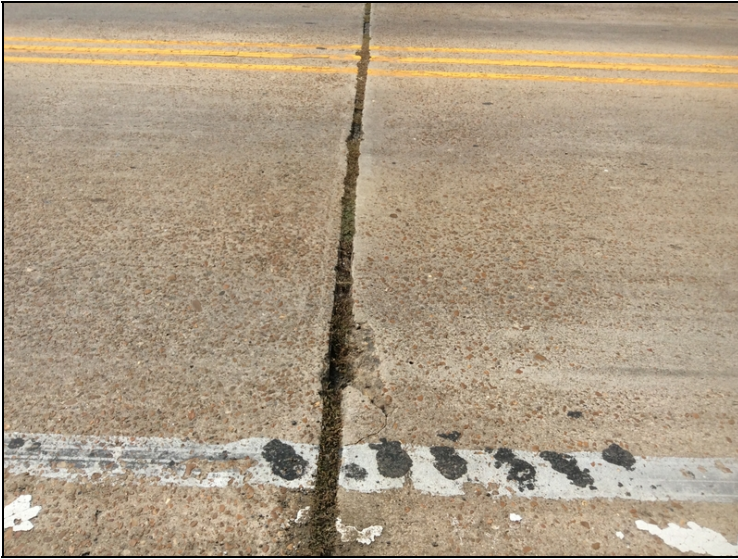
Joint at bent 4, looking left. 1 5/8 inch wide with no seal.
