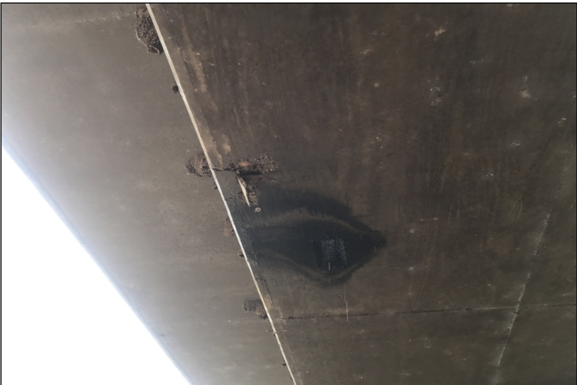
Spall with rebar in span 2
