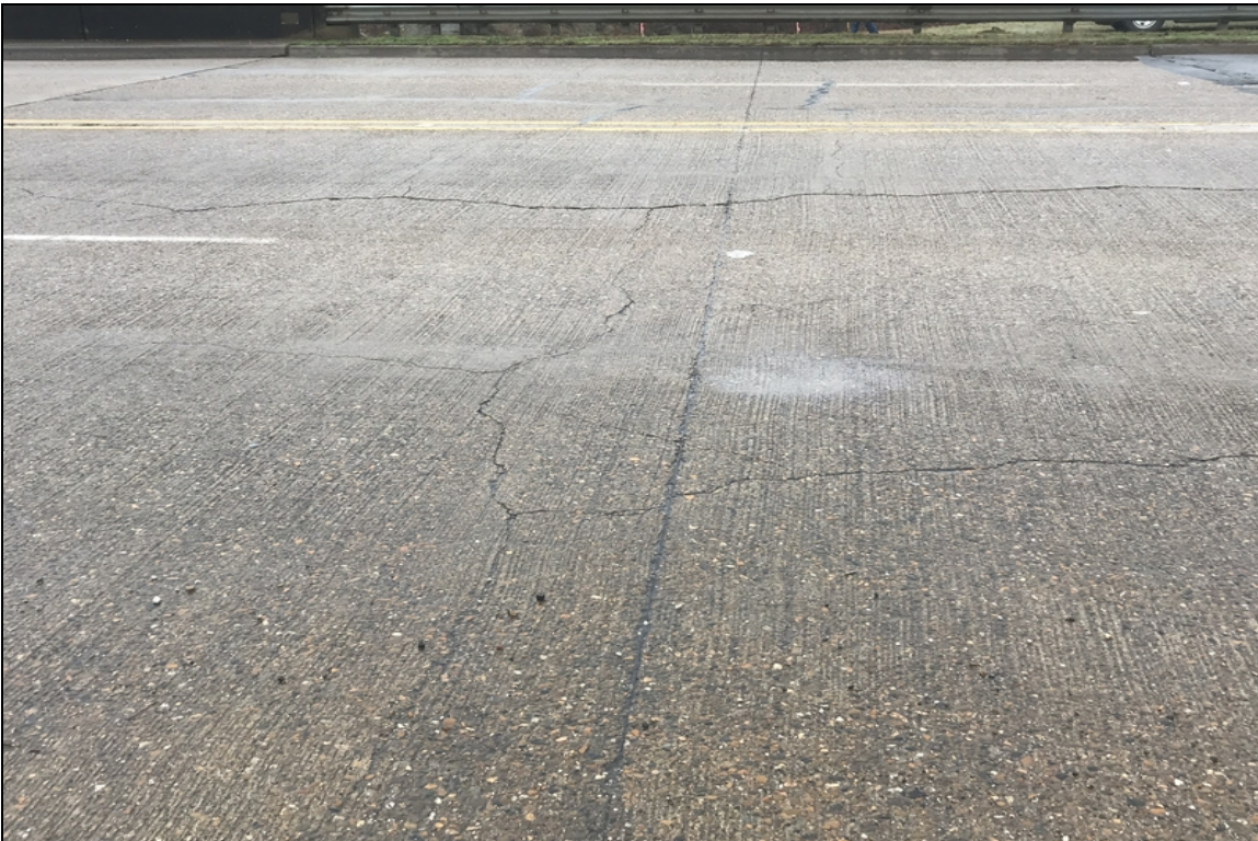
Diagonal cracks in both of the approach slabs
