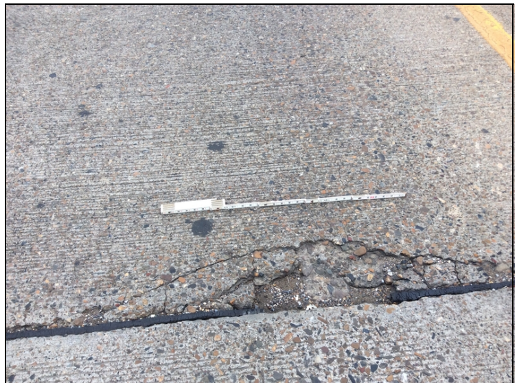
Span 3, above bent 3, spall near center line of slab.
