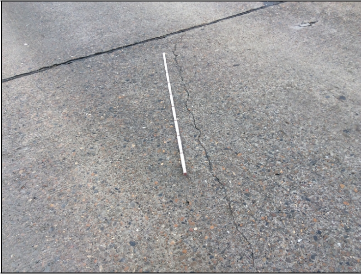
Span 1, diagonal crack up to 1/8" wide.
