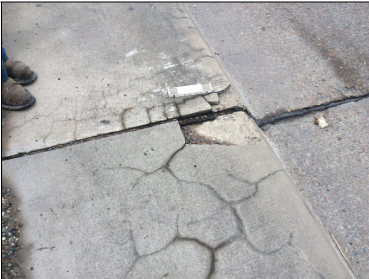
Left sidewalk, spall at bent 3
