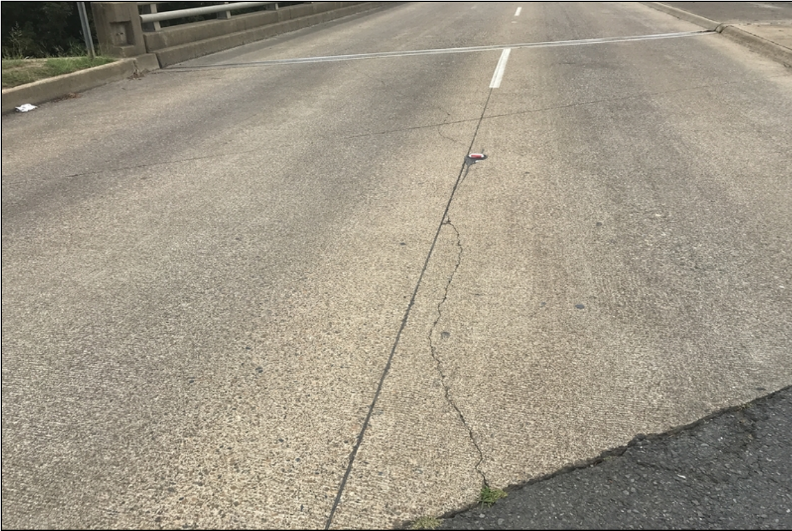
All approach slabs have large unsealed cracks
