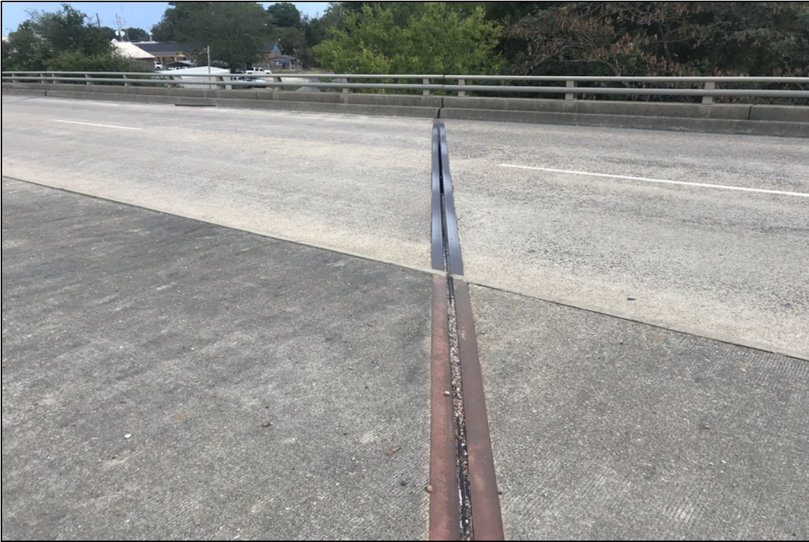
Joint seal has fallen out at bent 4
