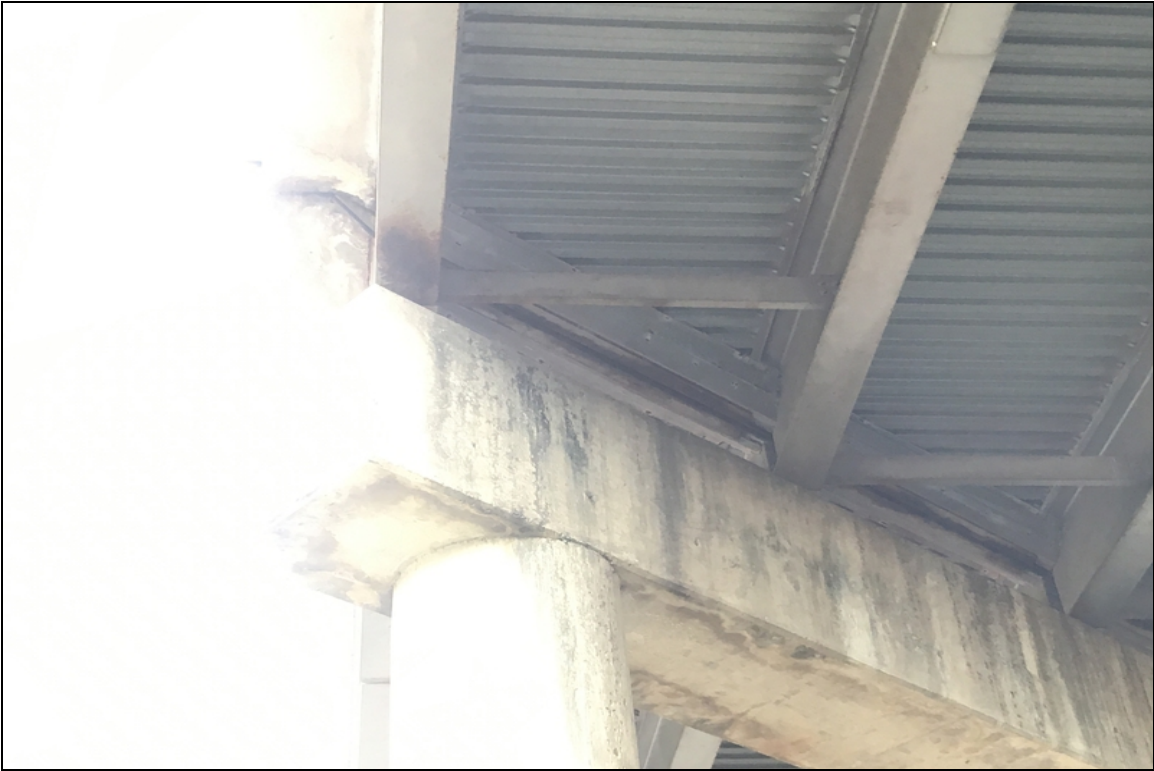
Corrosion on the beam ends at bent 2
