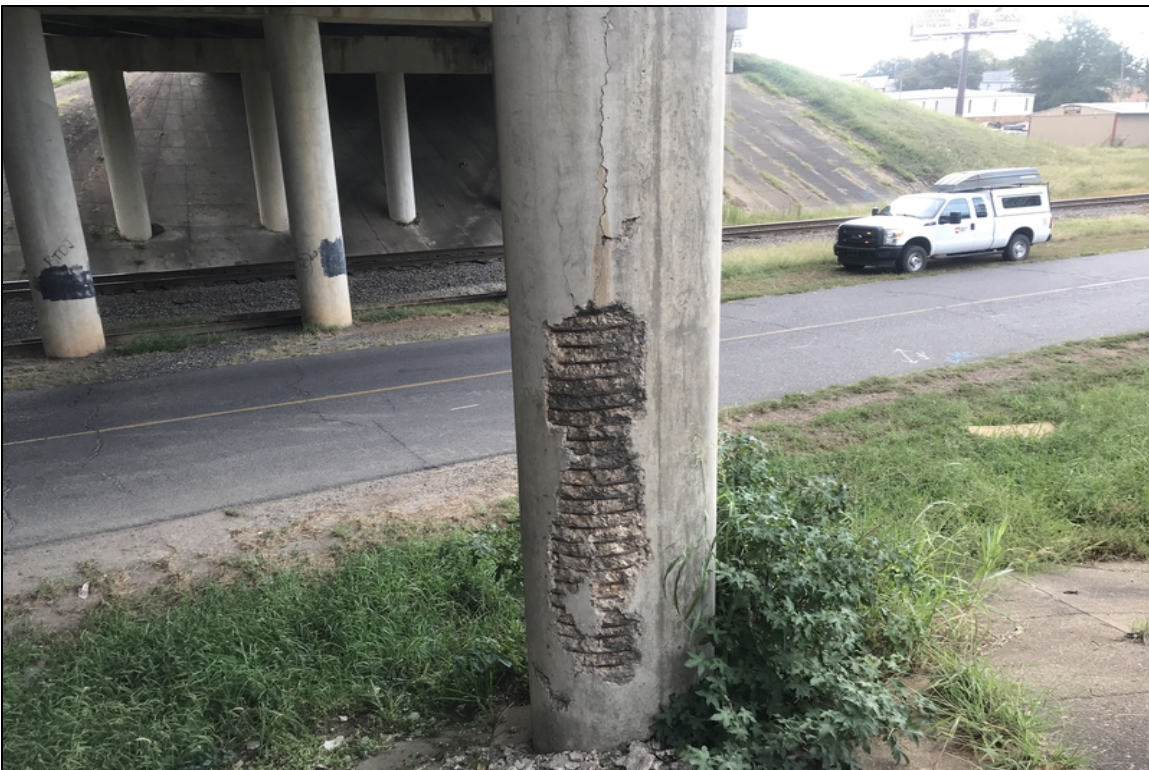
Column 7 at bent 2 has large spall with exposed rebar and large vertical cracks
