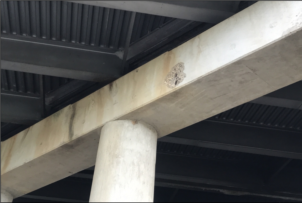
Spalls with rebar at bent 3
