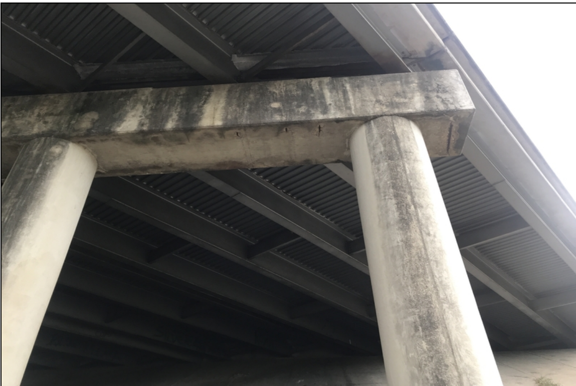
Spalls with rebar in the underside of the cap at bent 4
