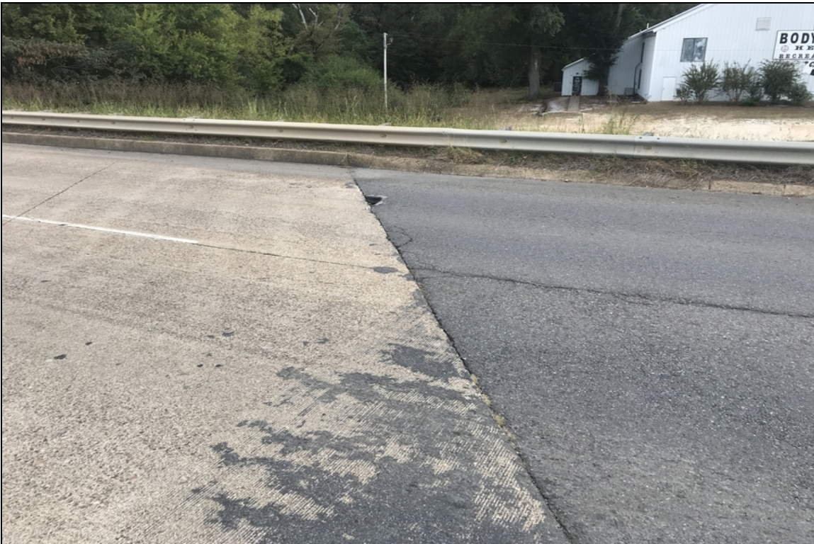
Potholes at south east end of the bridge
