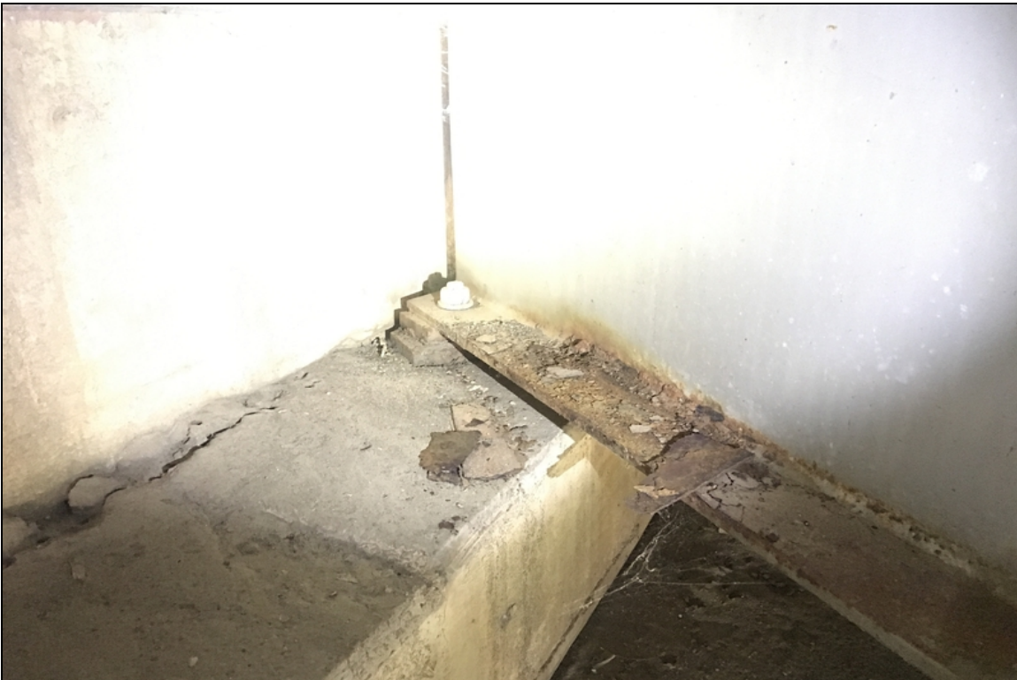
beam ends have light to moderate corrosion starting to form due to leaking joints.
