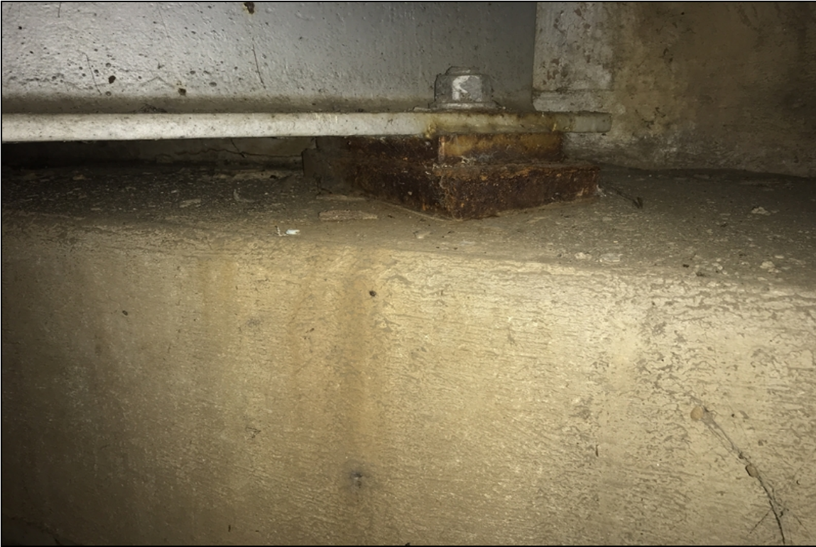
all Bearings have heavy corrosion and laminating rust
