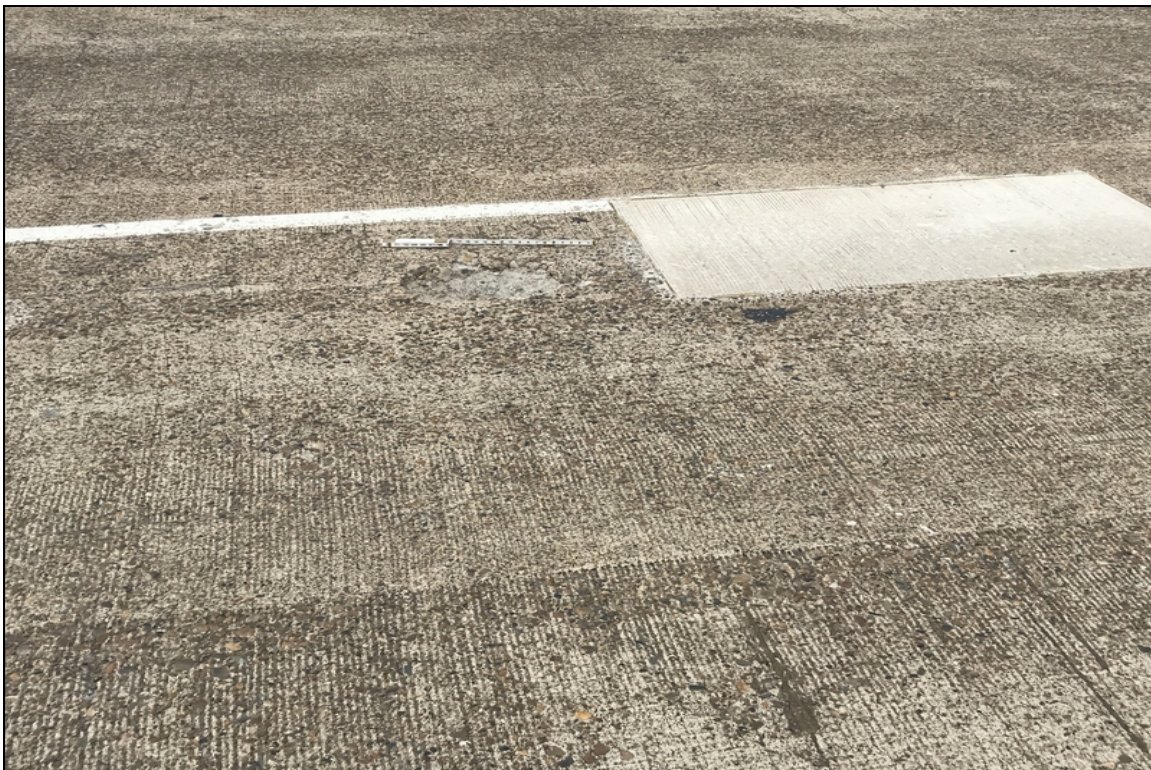
right side of span 2 has a large pothole with exposed rebar
