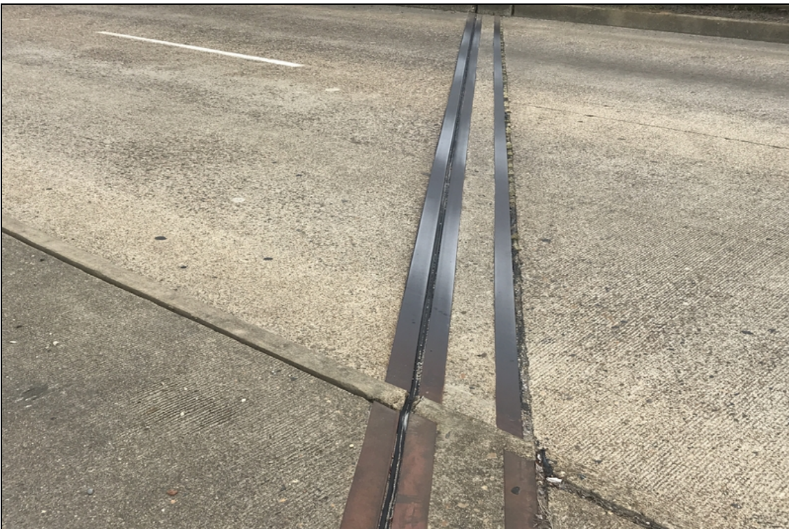
Joint seal at bent 5 is torn and leaking
