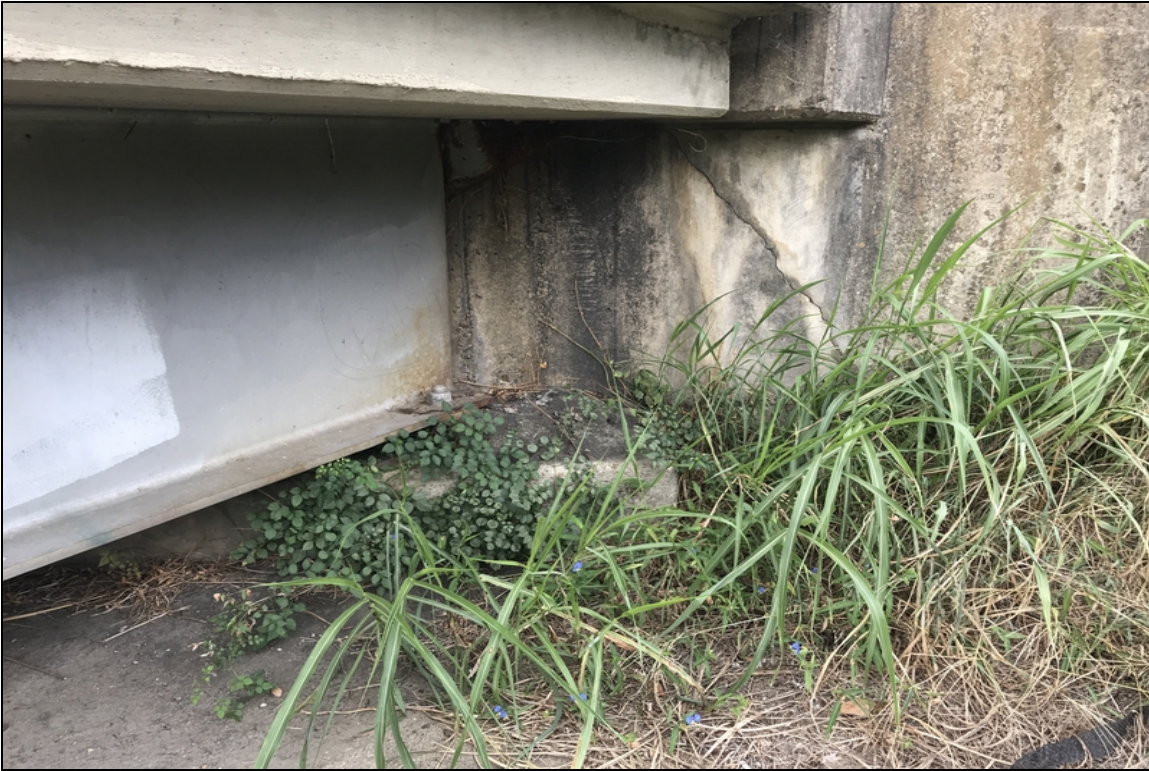
Cracks in back wall at bent 1 beam 1
