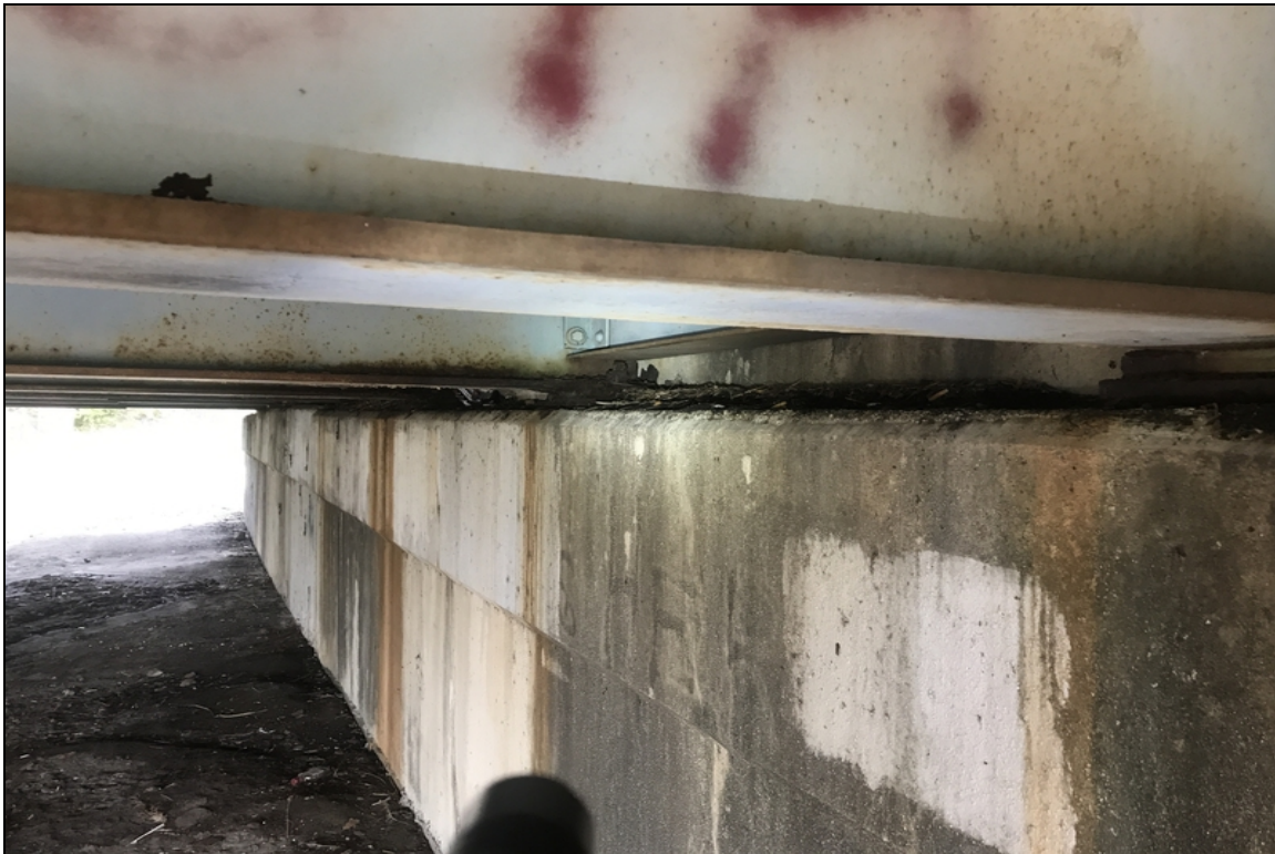
Dirt and debris build up around bearings on the cap at abutment 2
