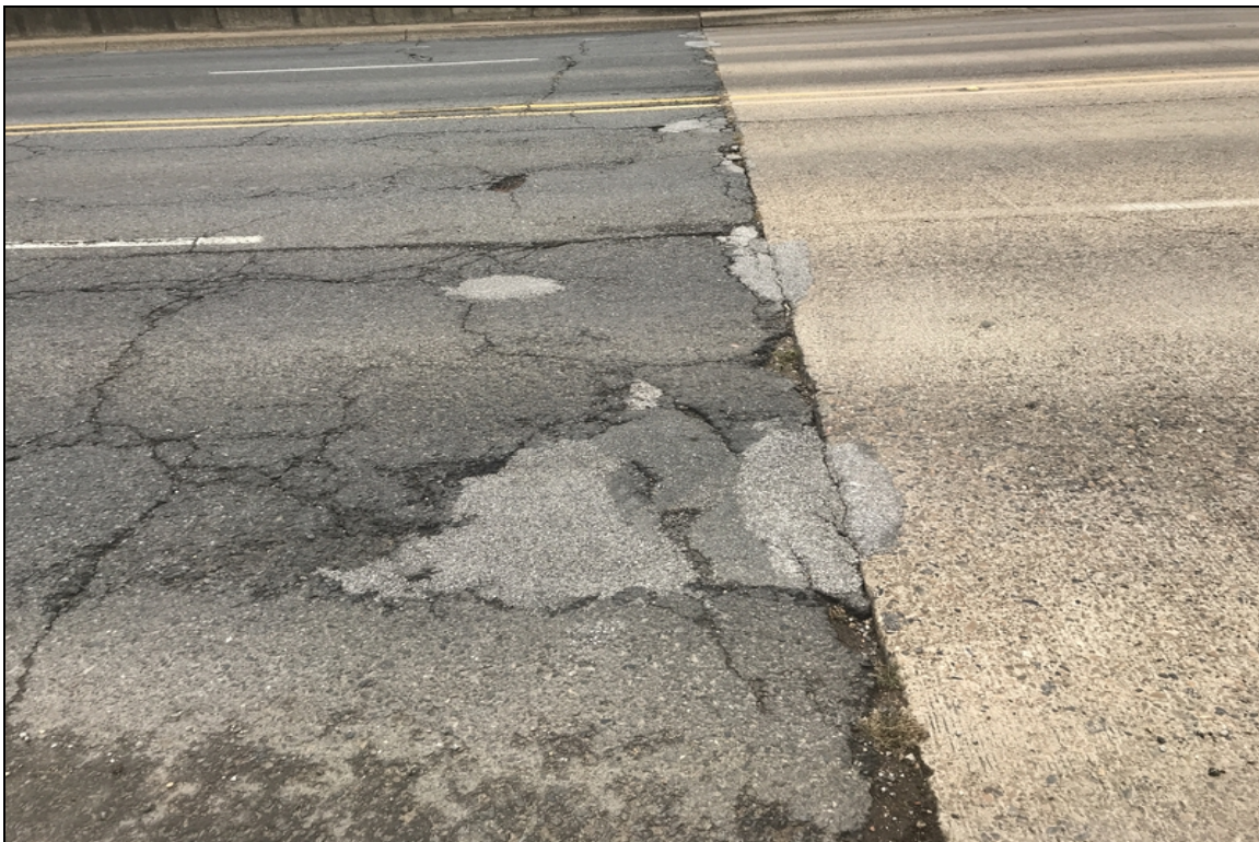
Potholes at the approach slabs at abutment 2
