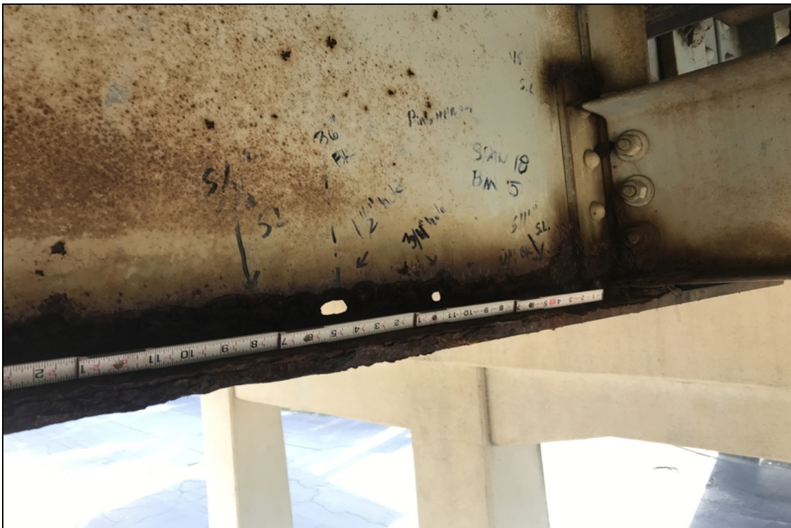
Span 18 beam 5 has 5/16 section loss to bottom flange and two holes, 1 1/2 inch; and 3/4 inch; that are 36 inch; back from beam end
