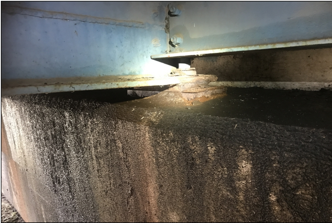
Bearing at abutment 1 beam 7 is corroded with laminating rust
