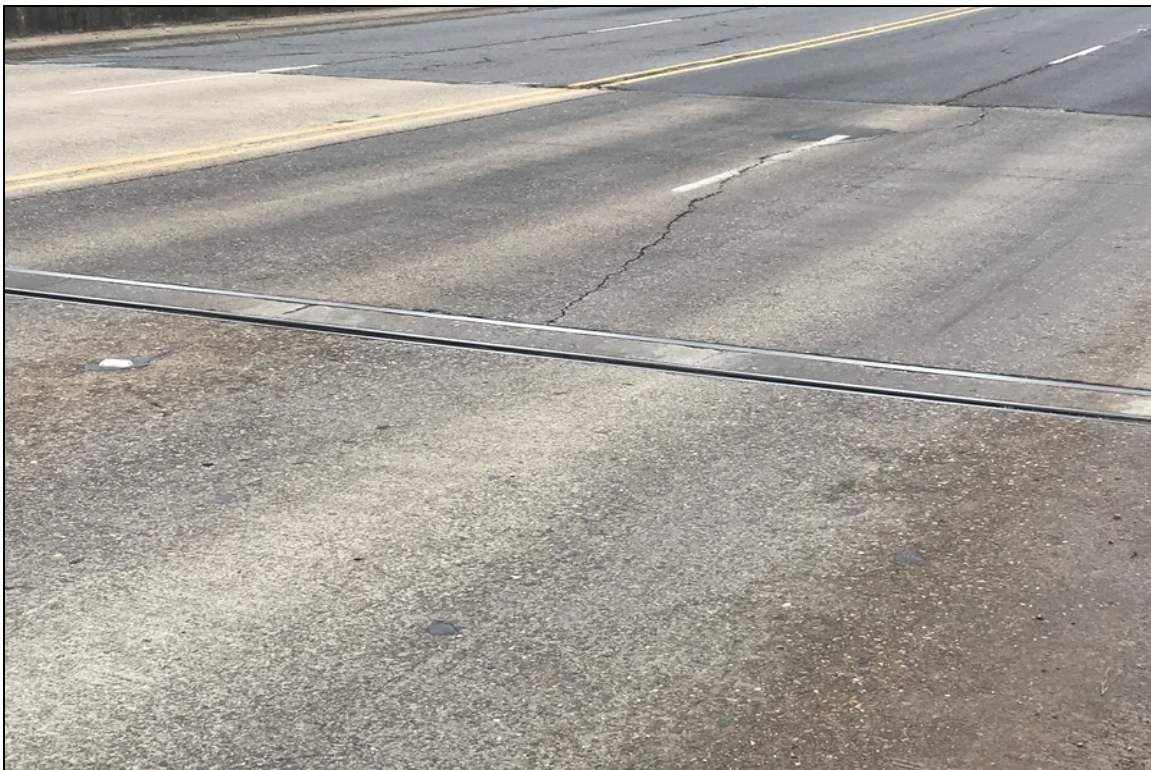
Large cracks in Approach slab at abutment 1
