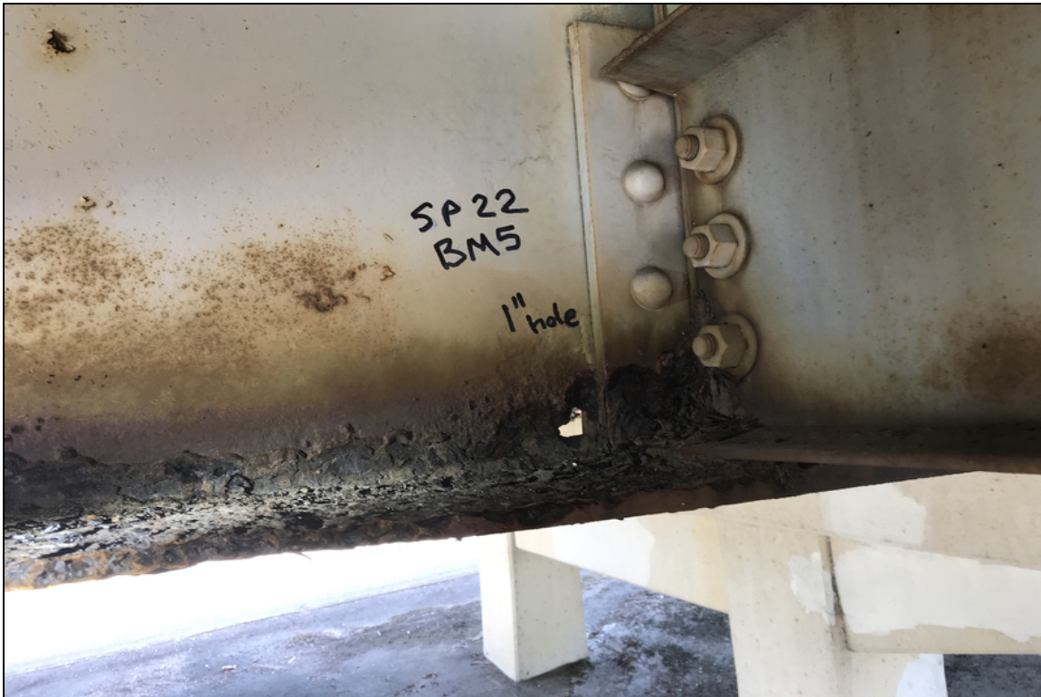
1 inch hole at beam end in span 22 beam 5
