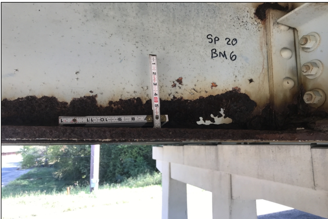
3.5 x2 hole at span 20 beam 6
