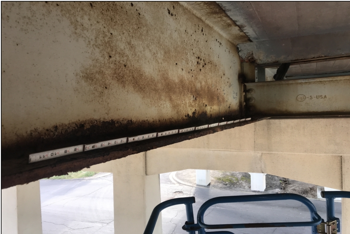
Span 18 girder 5 section loss at lower web and bottom flange
