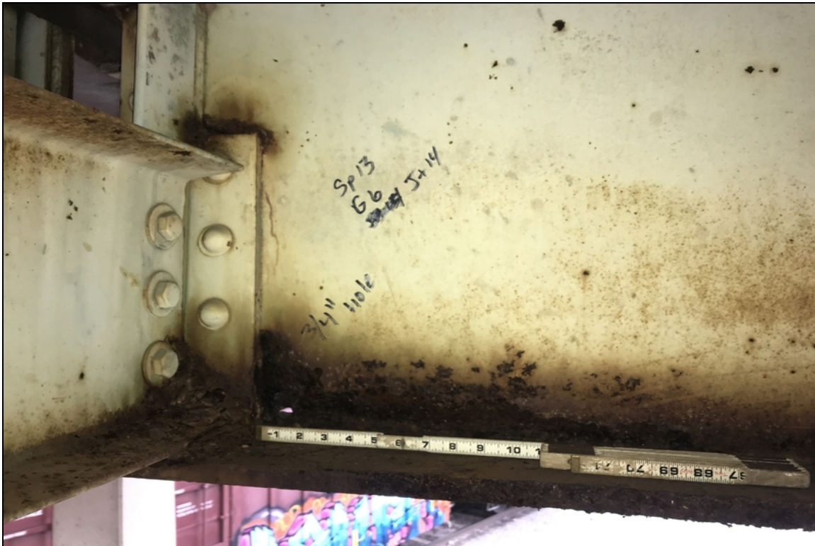
span 13 beam 6 joint 14 has a 3/4\"/>
