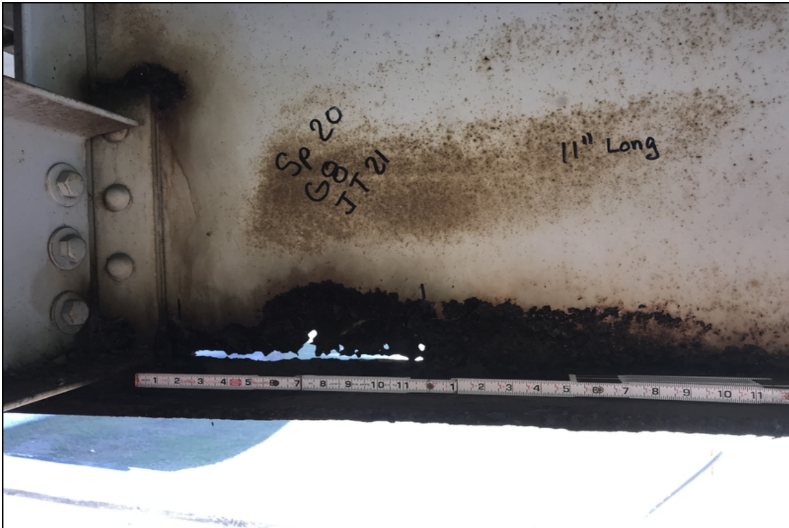
11" x 1.5 hole at span 20 beam 8 joint 21
