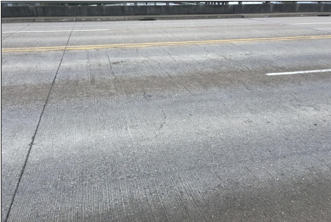
Transverse Deck cracks in span 4
