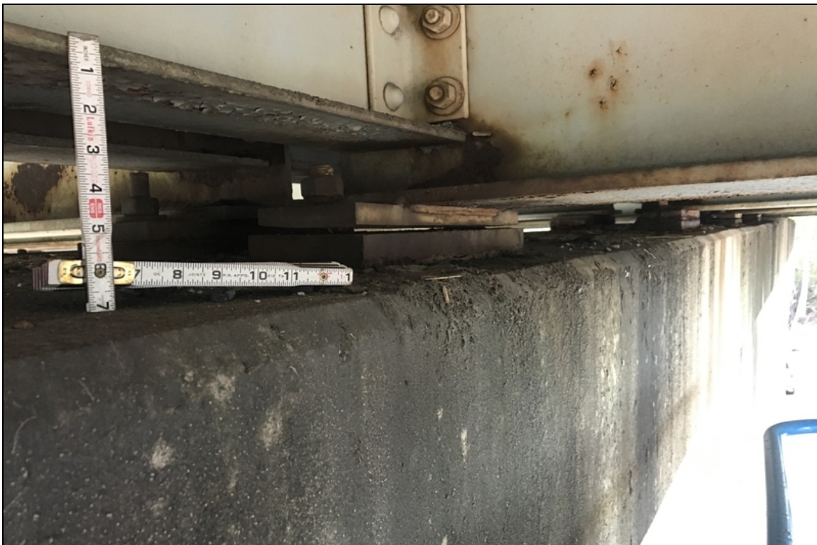
Bent 9 bearings 6 and 8 have an 1/8" gap
