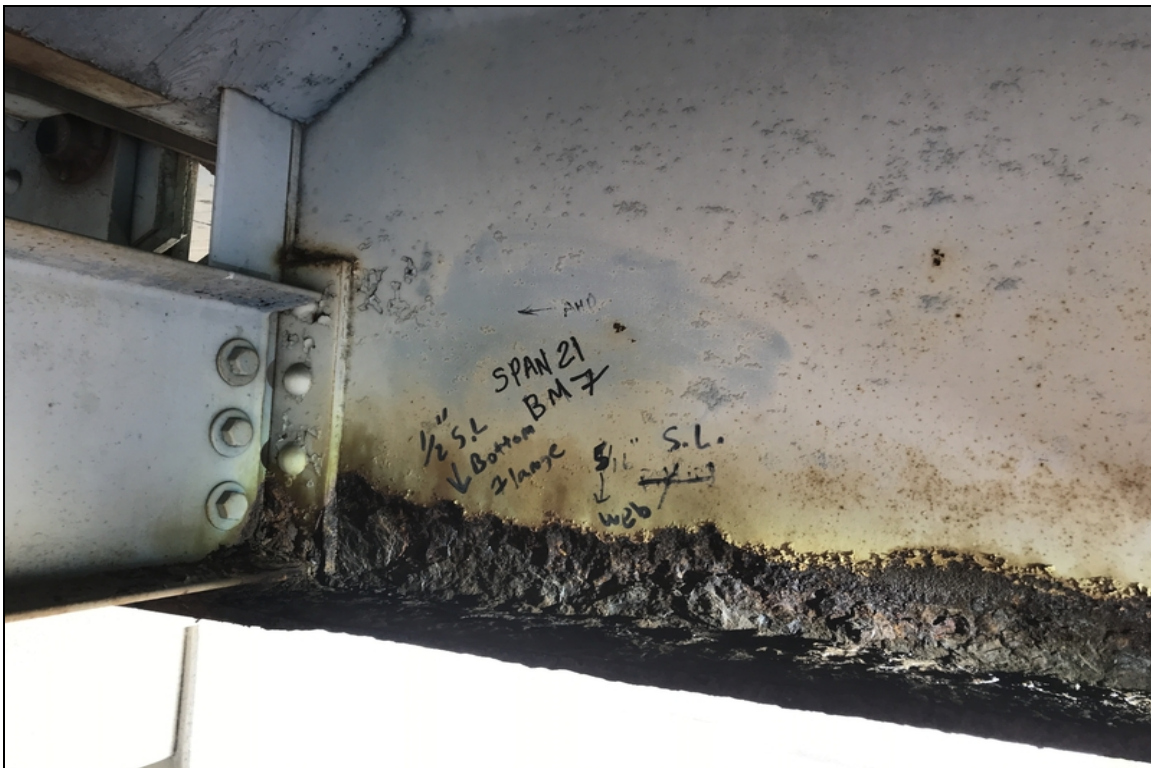
Span 21 beam 7 has 1/2" section loss to bottom flange and 5/16" section loss to lower web
