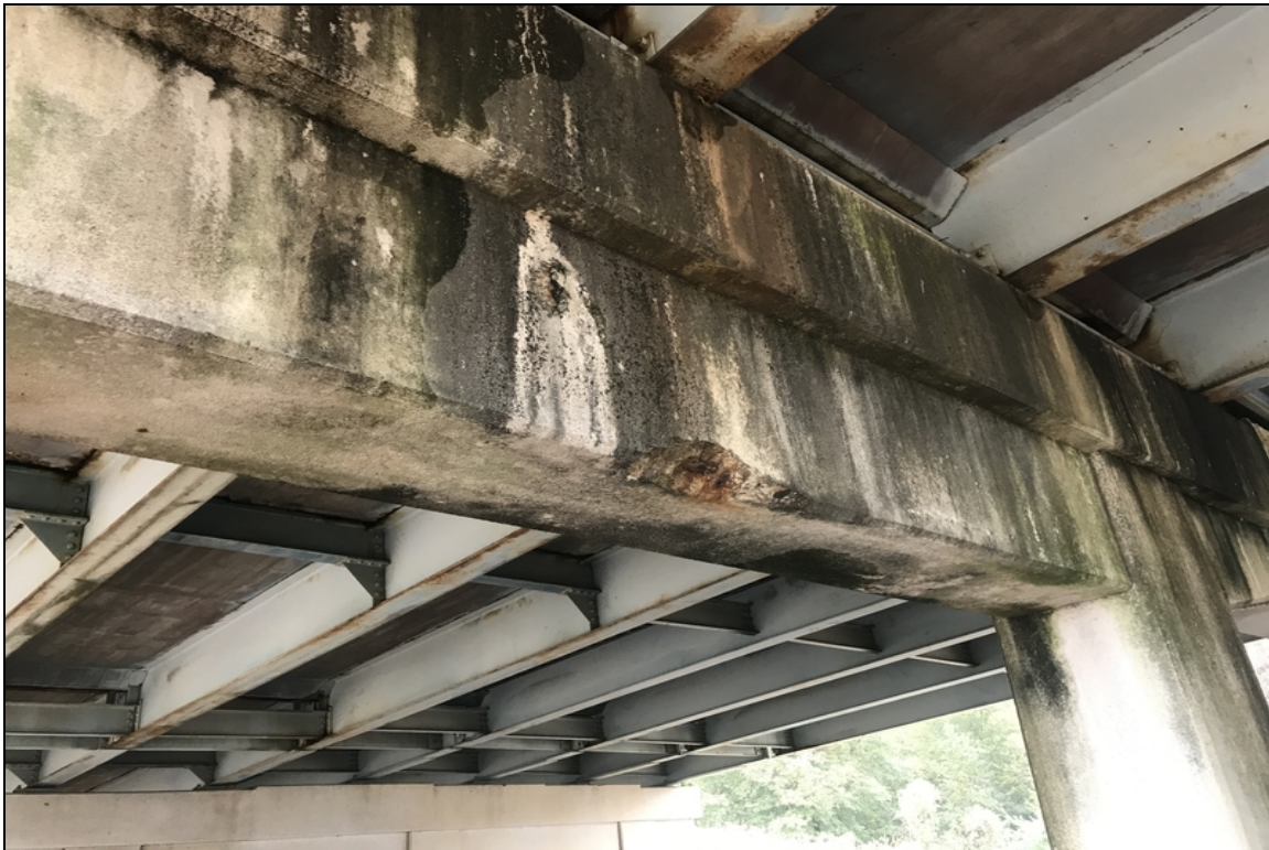
Bent 4 cap has a spall with exposed rebar
