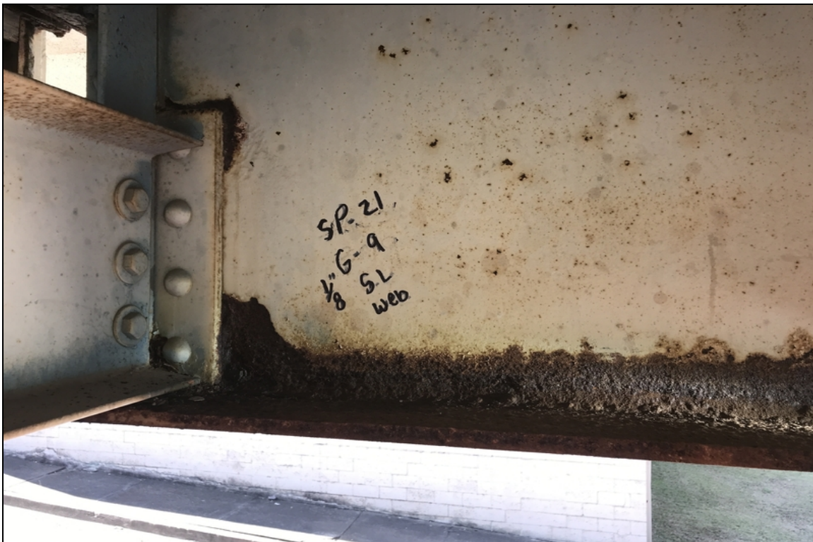
Span 21 beam 9 has 1/8 section loss to the lower web
