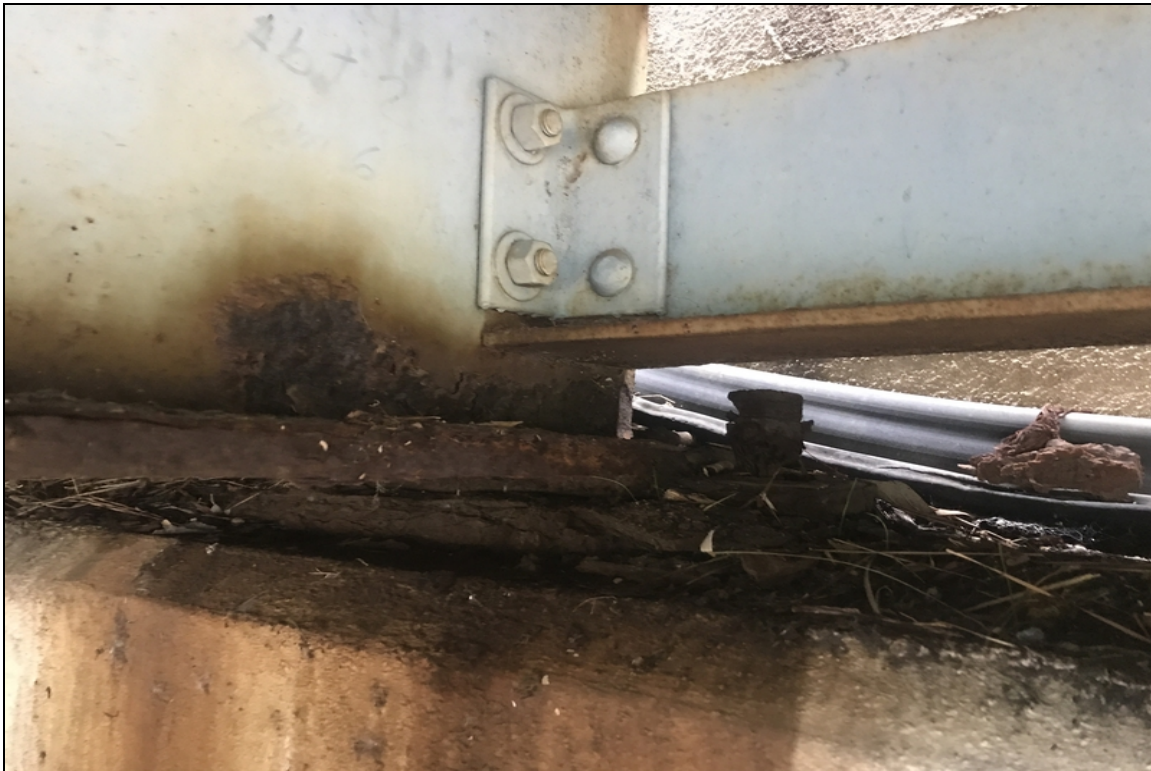
Bearings at Abutment 2 are heavily corroded with the bearing at beam 6 being the worst case
