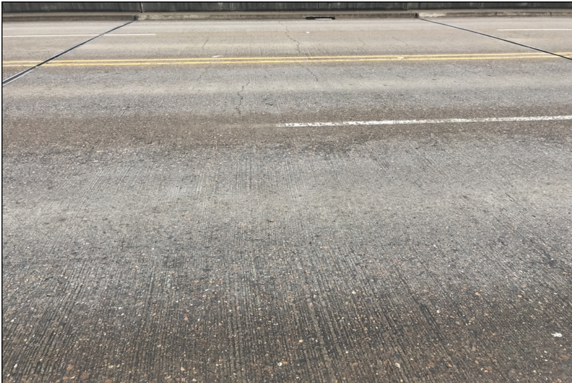
Deck cracks in span 13
