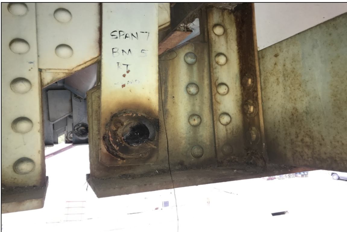
Span 7 beam 5 ahead hanger at lower pin has section loss up to 1/8" behind washer
