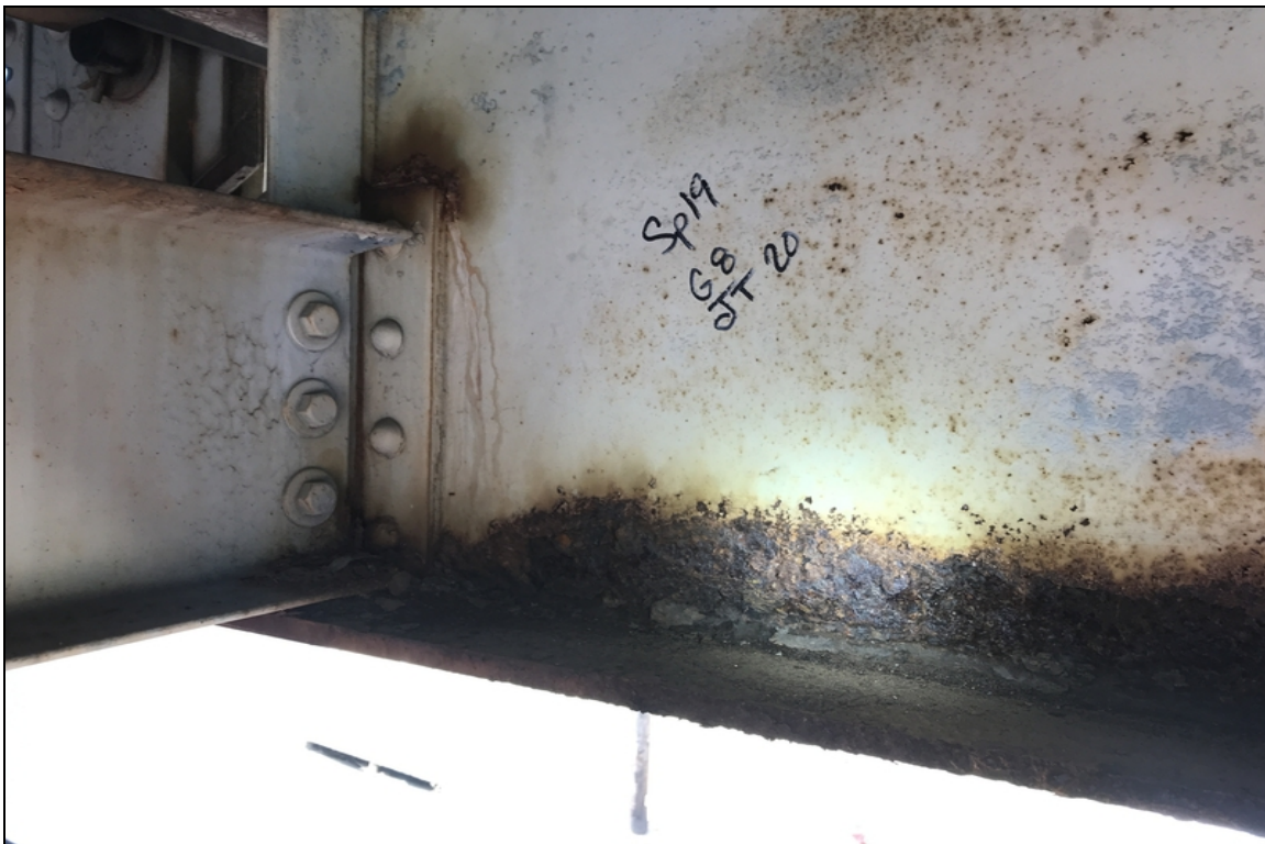
span 19 beam 8 joint 20 has 1/8" section loss
