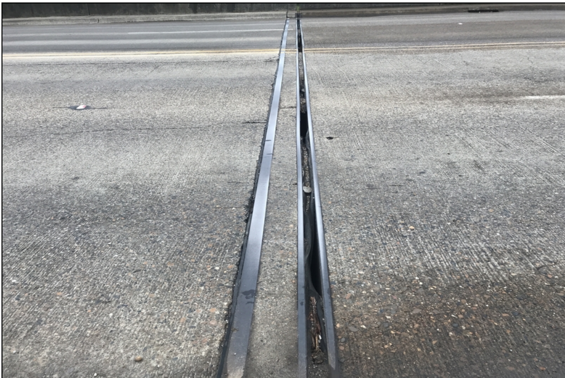
Joint seal at abutment 2 has lost bond and fallen out.
