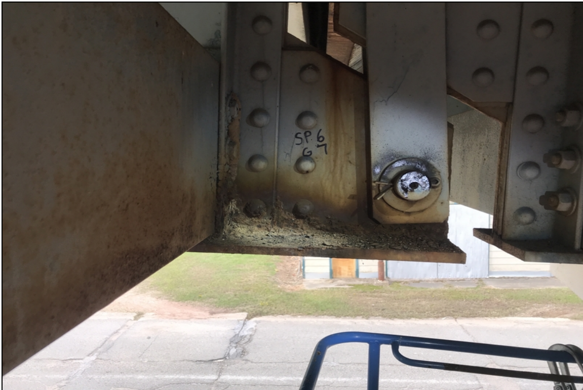
Span 6 beam 7 lower web and bottom flange section loss
