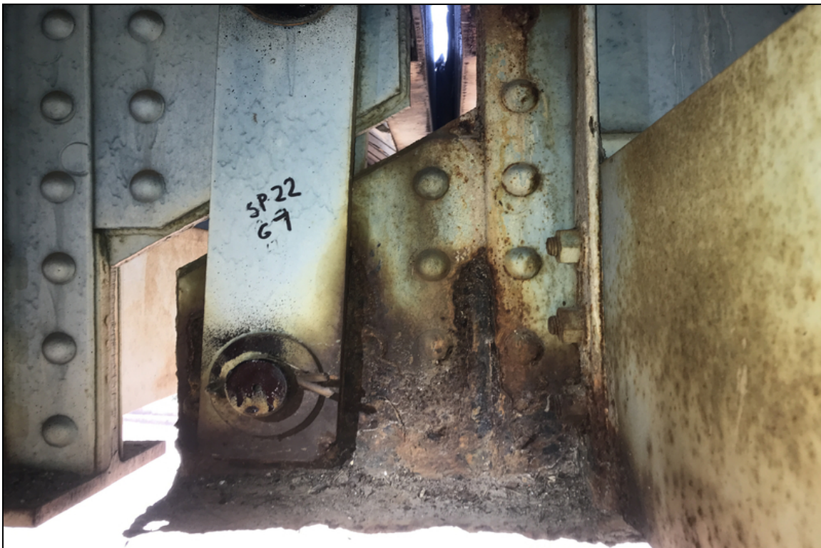
Beam end at Span 22, girder 7, is down to a knife edge in the flange with heavy pitting in the lower web
