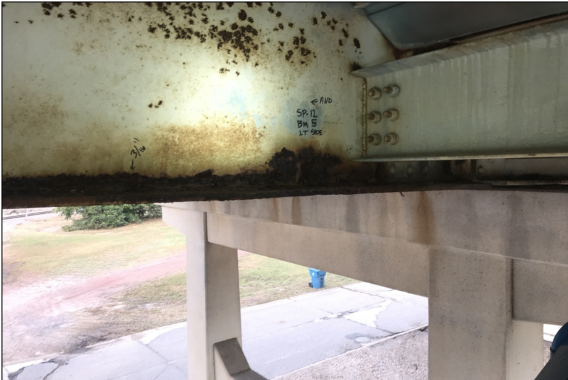
Span 12 Beam 5 lt side 3/16 section loss to lower web
