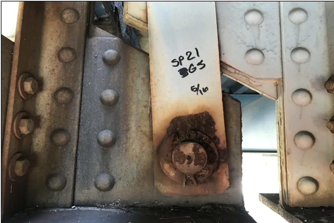
5/16 section loss to hanger at span 21 beam 5
