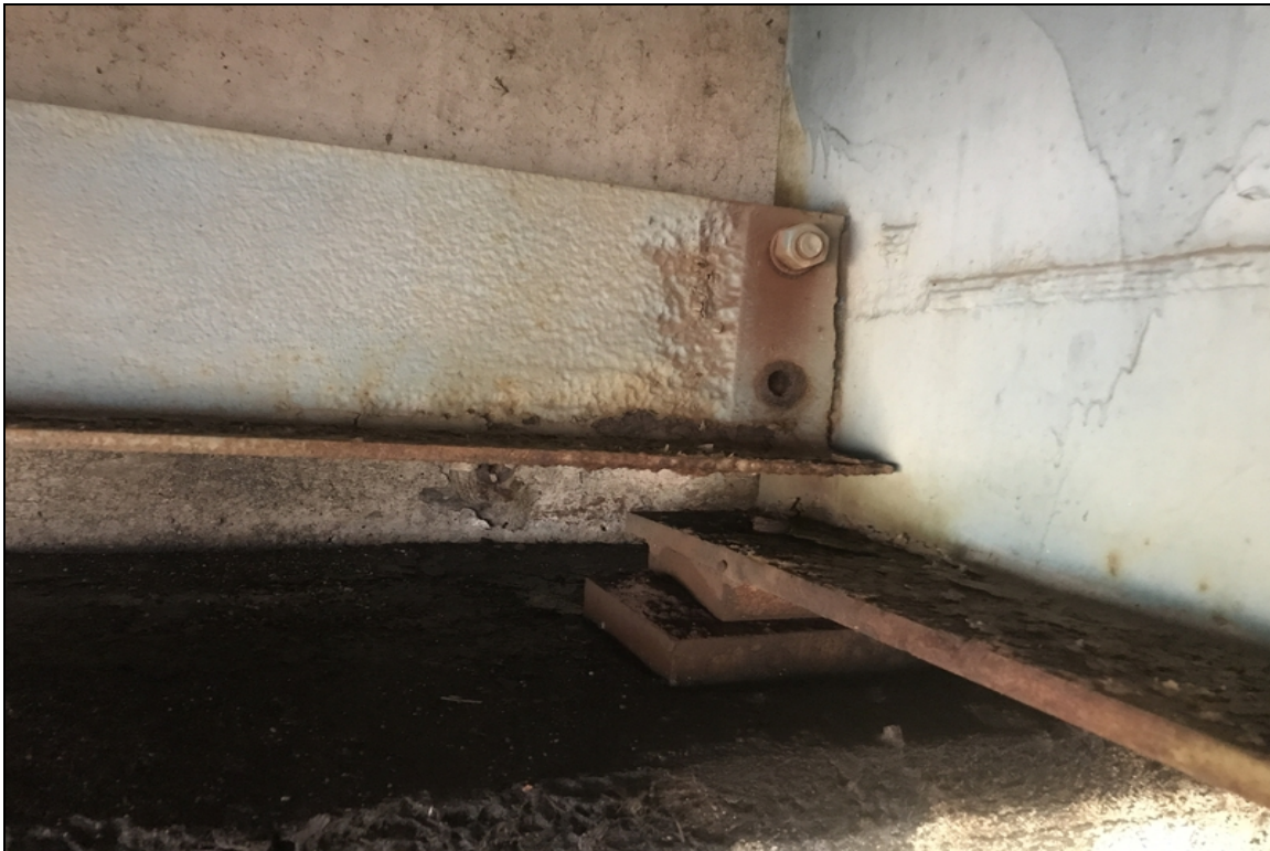
Abutment 1 beam 6 right side at the diaphragm has a missing bolt
