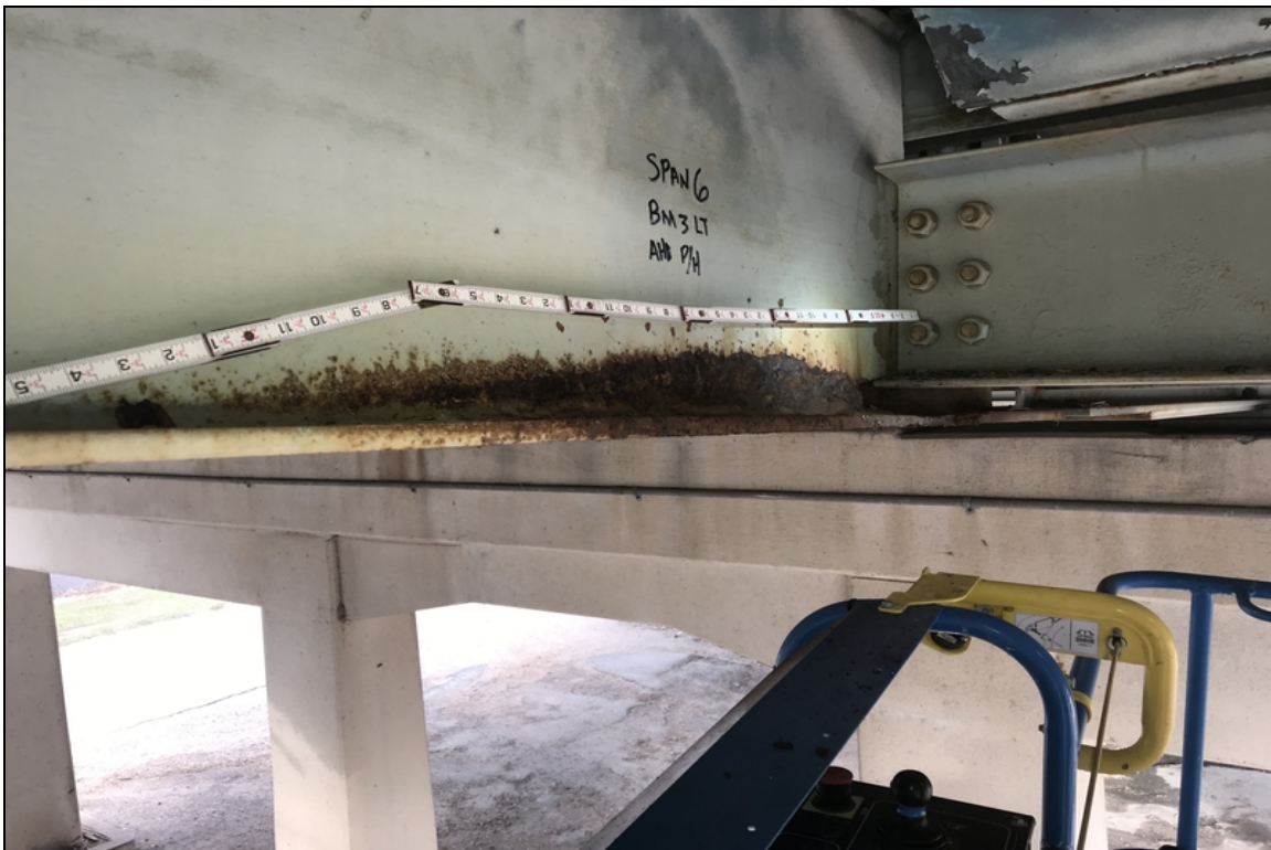
Span 6 beam 3 left side ahead of pin and hanger section loss to lower web and bottom flange
