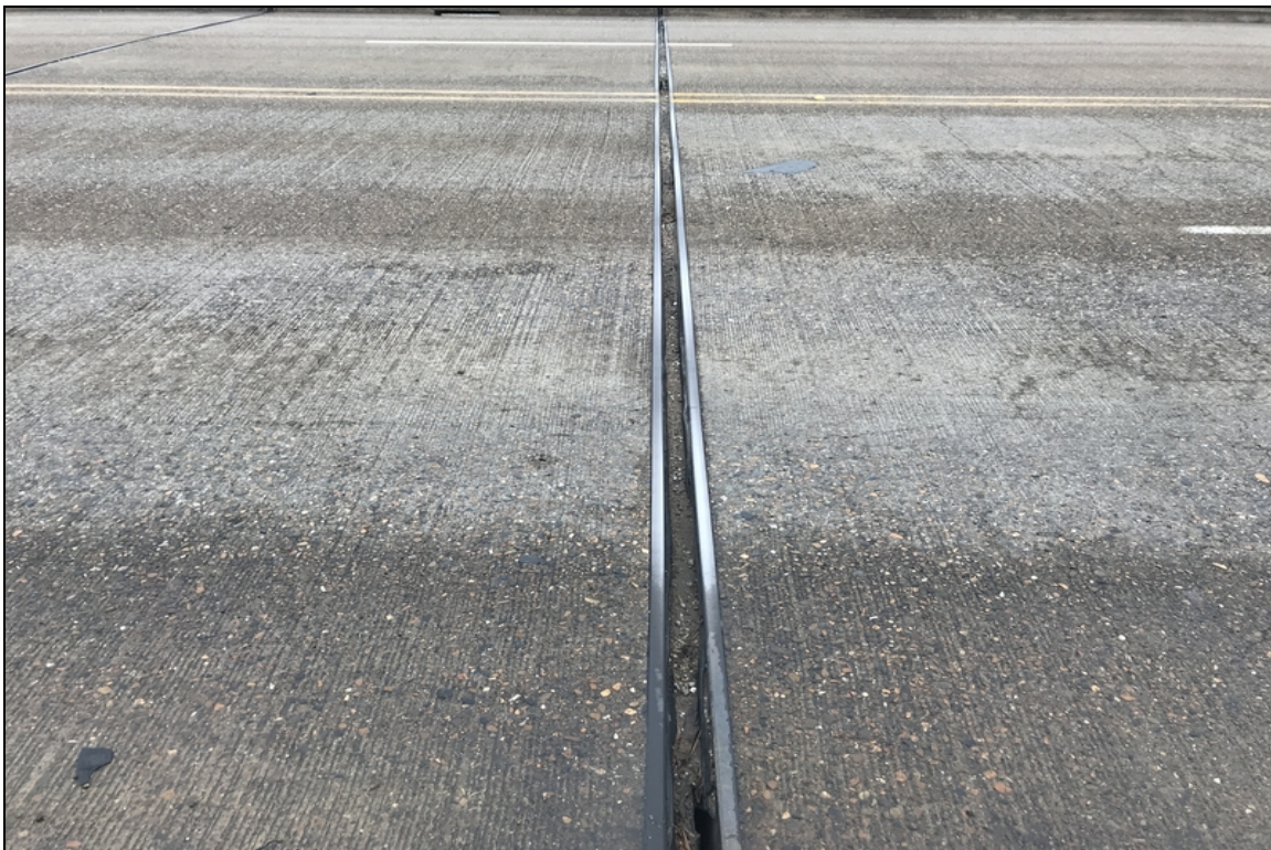
Joint seal at bent 14 is full of debris has lost bond and is leaking
