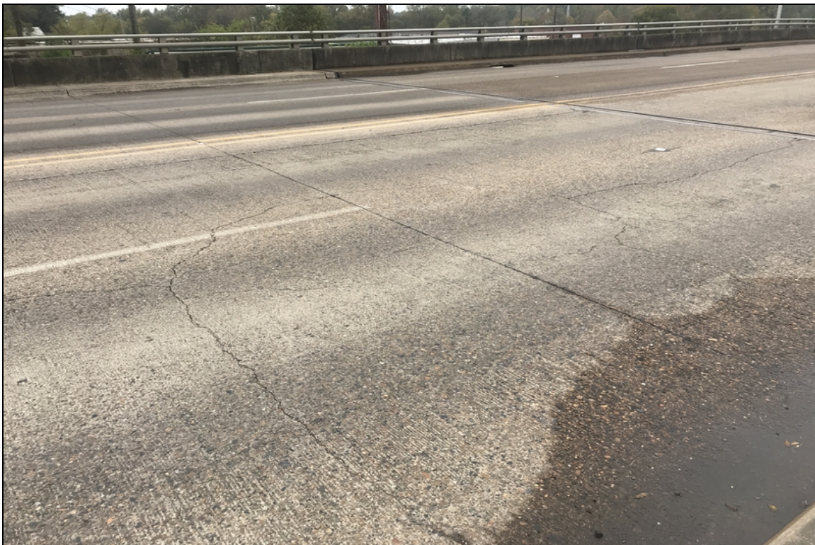
Approach slabs at abutment 2 have large Transverse and longitudinal cracks
