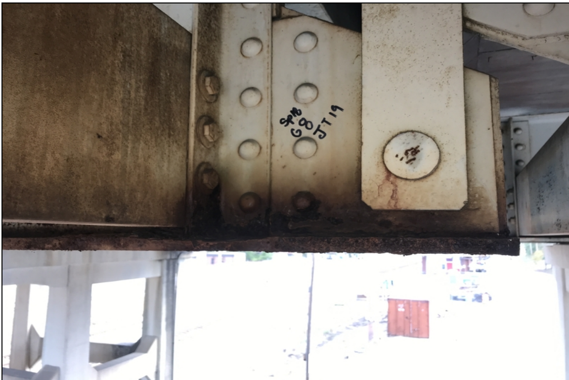
Span 18 beam 8 has 1/4" section loss at the bottom flange
