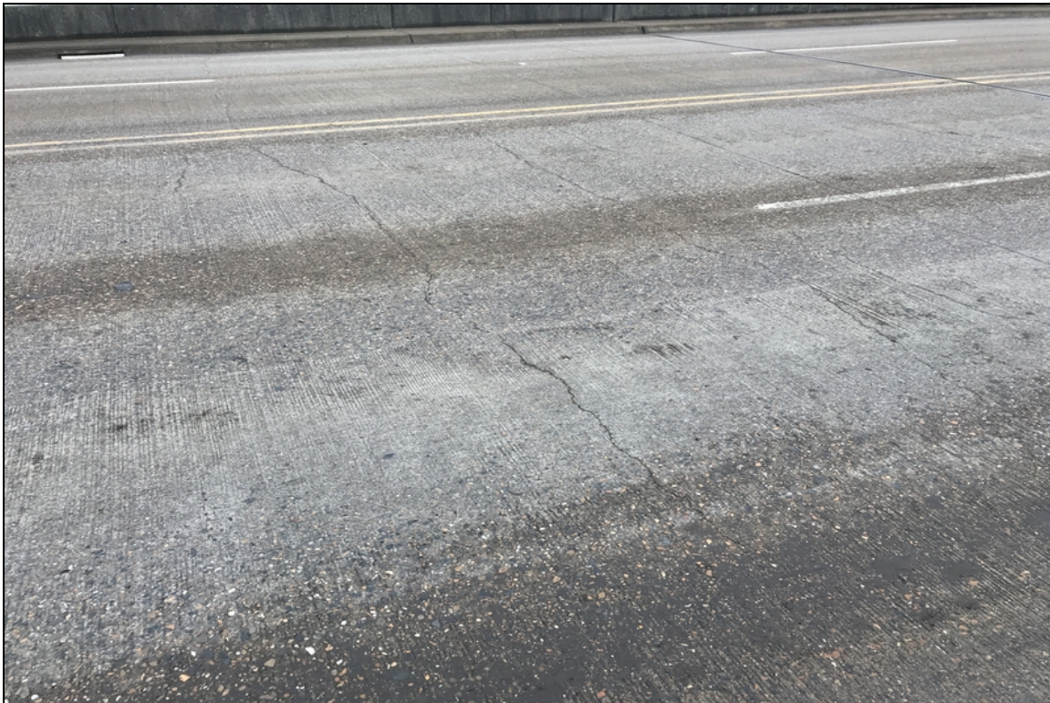
transverse Deck cracks in span 23
