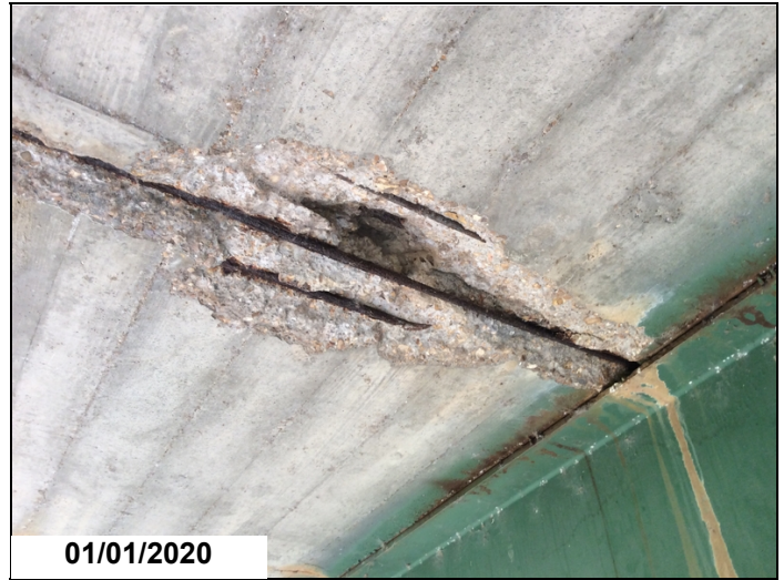
Deep Spall with exposed rebar at Span 18 between Girders 3 & 4.
