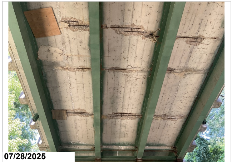
Typical undersurface with exposed rebar and efflorescence.
