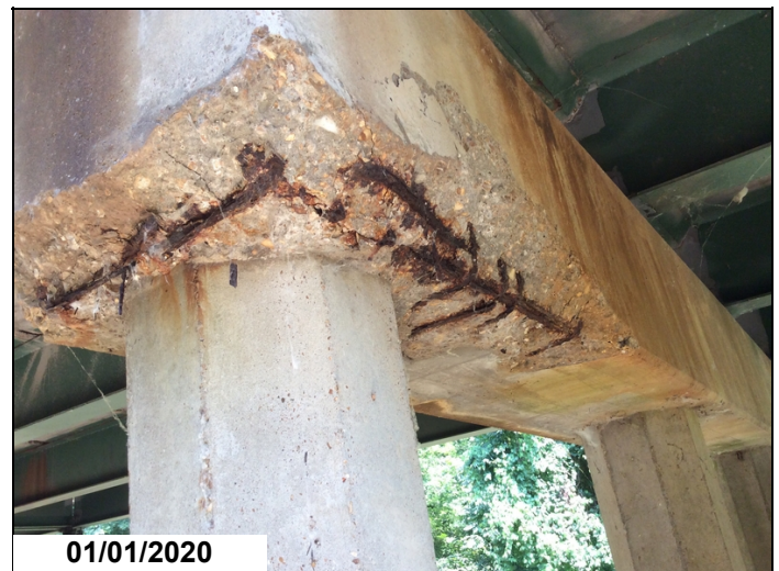
Cap at Bent 22, spalls with exposed rebar at Pile 4.
