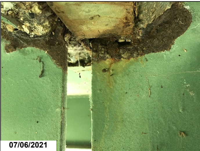
Severe section loss to Girders 2 & 3 with holes in web below haunch @ Bent 17 & 19. Bent 19, girder 2, 3, & 4. - 2021
