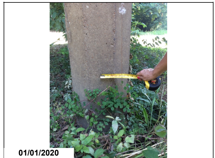
Bent 2 out of plumb.
