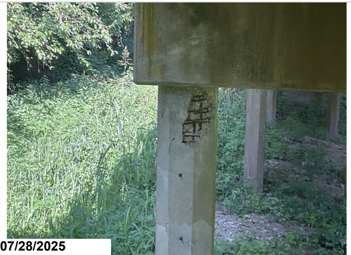
Bent 9, Pile 4 has spalling with exposed rebar and heavy deterioration at the cap connection. 1EA CS3
