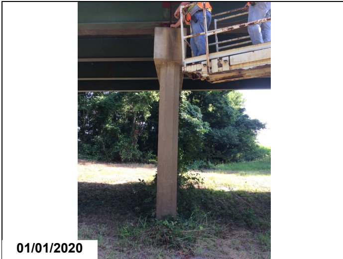
Bent 2 out of plumb.
