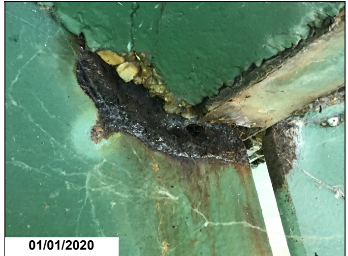
Small hole @ end of Girder 3 @ haunch area @ Bent 19. - 2020
