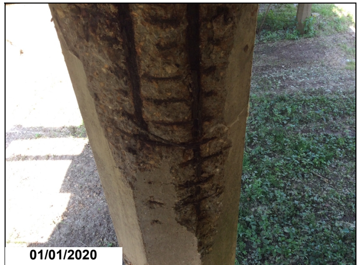
Pile 3 at Bent 15, spalls with exposed rebar with 100% section loss.
