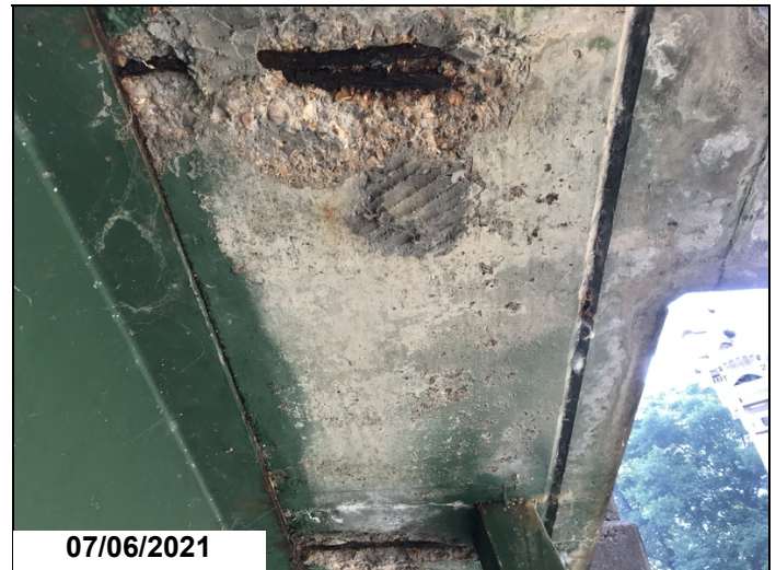
07/06/2021 Spalls with rebar exposed to deck below & to left & right overhang at all spans. Typical to Lt & Rt overhangs. Span 2, Rt side.
