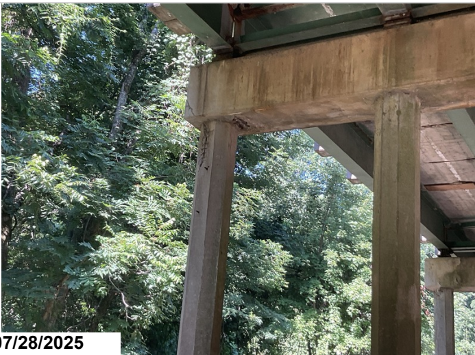
Bent 21, pile 4: has spalling with exposed rebar. 1EA CS3
