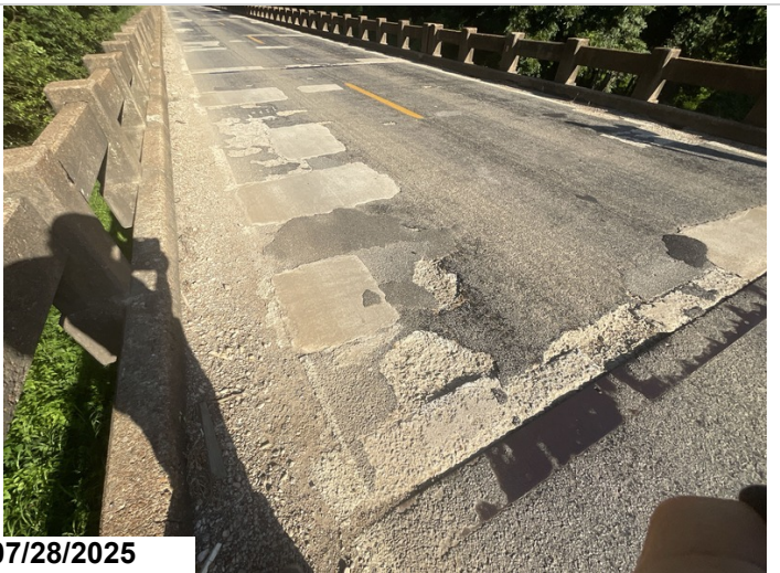
Span 10: has widespread patches and scattered spalls. 81SF CS2 | 27SF CS3
