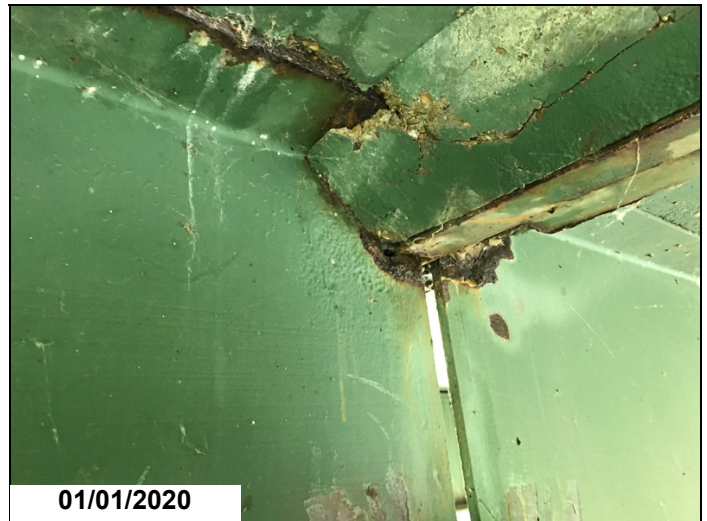
Small hole @ end of Girder 2 @ haunch area @ Bent 19. - 2020
