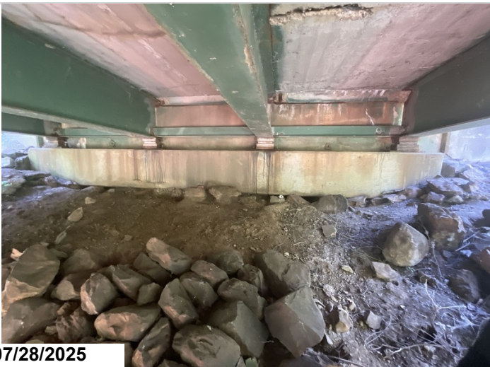
Abutment 2: has diagonal efflorescent map cracks with leaching buildup on the ends. 10LF CS3
