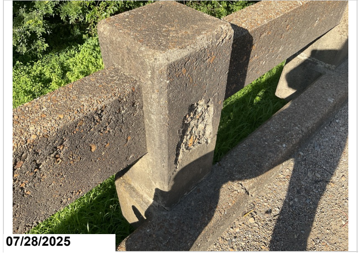
Typical spalling and deterioration of the railing.
