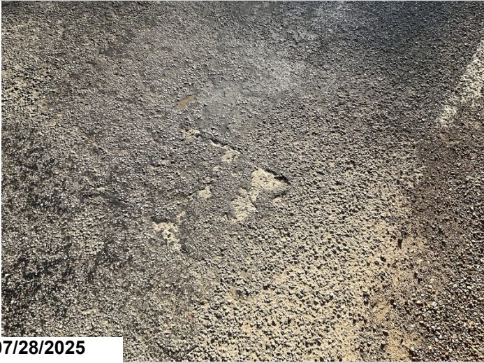
Typical spall on wearing surface
