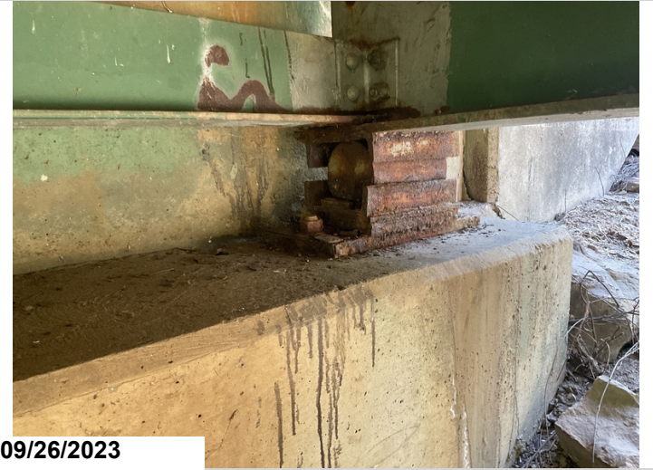
Bent 26, bearing 4: typical flaking rust. CS3.
