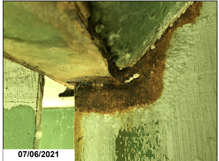
Severe section loss to Girder 3 & 4 with hole in web below haunch @ Bent 21. Girder 3. - 2021
