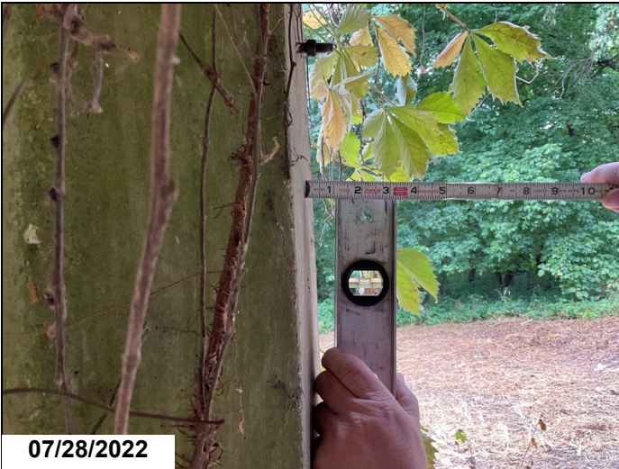
Bent 1, pile 1 is out of plumb
