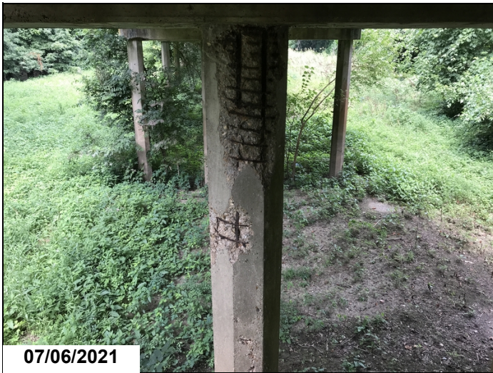
Cracks, delaminated areas & spalls with rebar exposed to Piles at Bents 1, 2, 6 - 12, 14, 15, 17, 19 - 21, 23. Bent 15, pile 3 ahead side.
