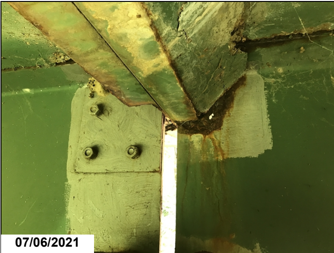
Severe section loss to Girder 3 & 4 with hole in web below haunch @ Bent 21. Girder 4. - 2021
