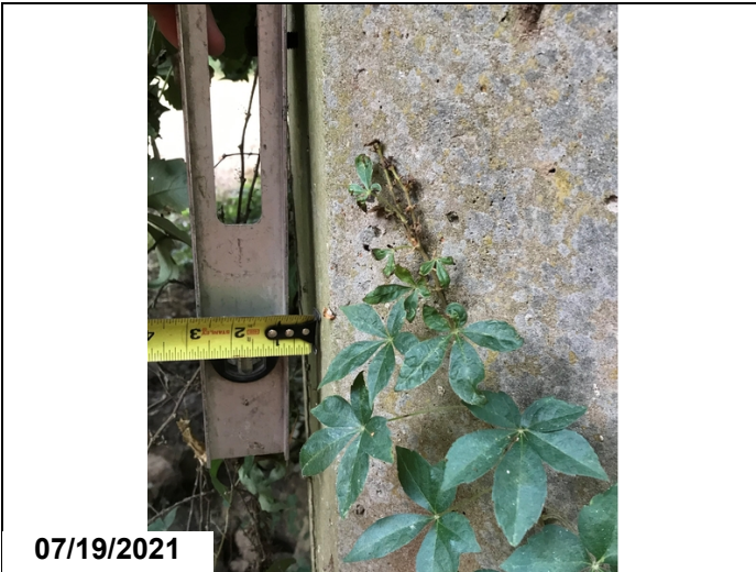
Bent 1, pile 1 is out of plumb
