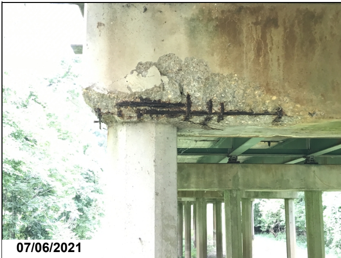
Cracks, delaminated areas & spalls with rebar exposed to caps at Bents 3, 12, 14, 15, 16 - 24. Ahead side of bent 22 @ pile 4.
