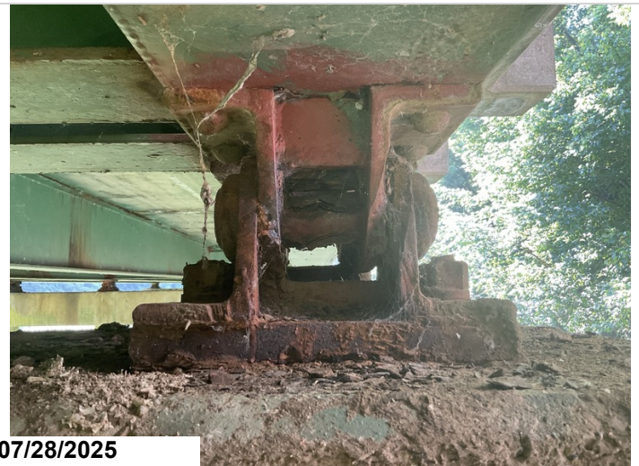
Bent 6, back, bearing 5: typical condition of the bearings. CS3
