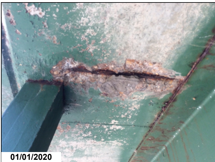
01/01/2020 Typical spall with exposed rebar to overhangs.
