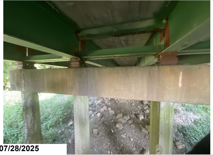
Typical replaced bearings are in better condition than the originals but still have flaking and pack rust between the plates. CS3
