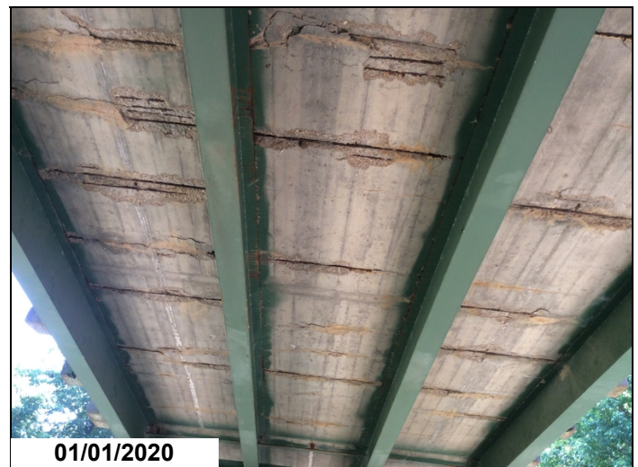
01/01/2020 Span 22. Soffit has 85' of exposed rebar.
