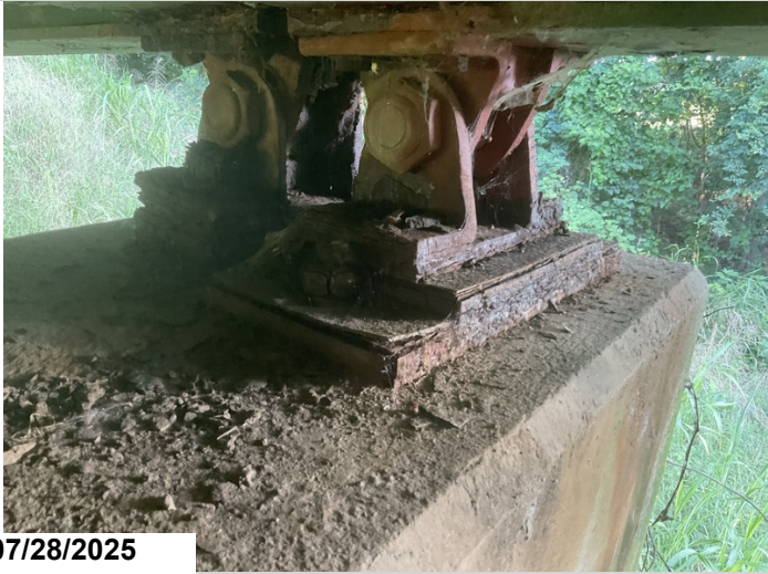
Typical original bearing. CS3
