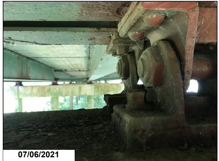
Bent 6 - Girder 3 & 4 has anchor bolt & nuts missing @ ahd. side. Girder 3.
