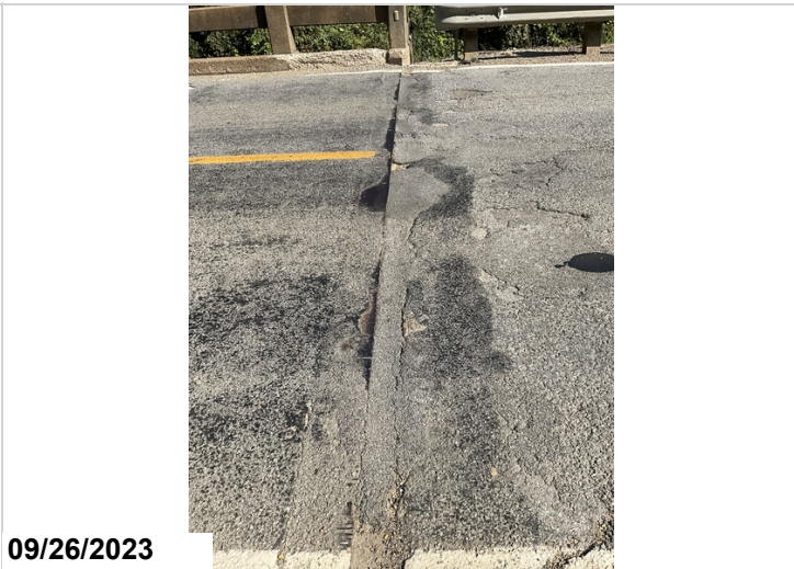
Joint over Bent 26, debris impact due to asphalt overlay, typical.
