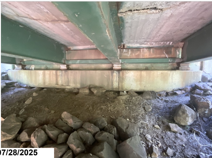
Abutment 2: typical bearings. CS3
