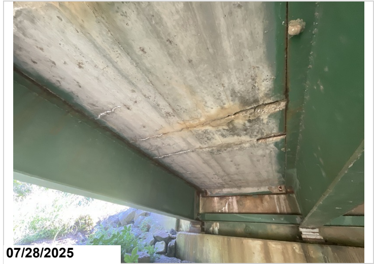
Span 26, bay 1: has typical, widespread efflorescence and rust-stained cracks. 65SF CS3
