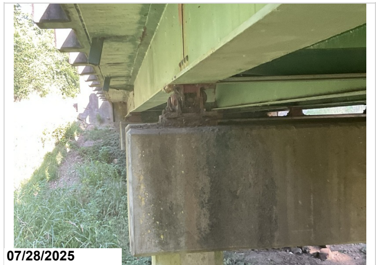
Bent 2, ahead, bearing 4. typical condition of the bearings throughout. CS3
