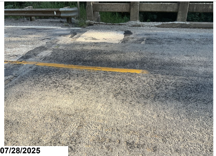
Typical patched areas of the driving surface.
