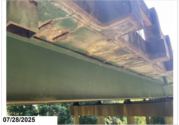
Spans 21-23, girders 1 and 5: have pack rust at the top flange for their full length raising the deck. 64LF CS3
