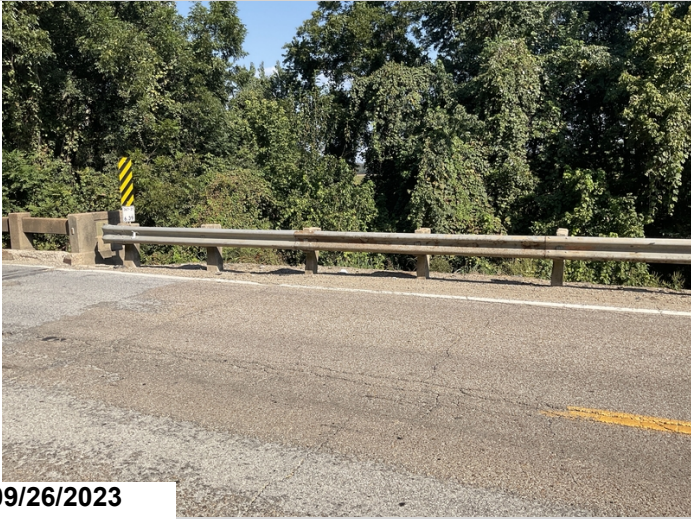
The transitions do not connect to the bridge.
