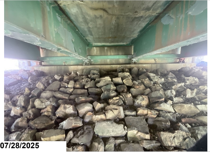
Abutment 1: has diagonal efflorescent map cracks with leaching buildup on the ends and similar vertical cracks in the center. 16LF CS3
