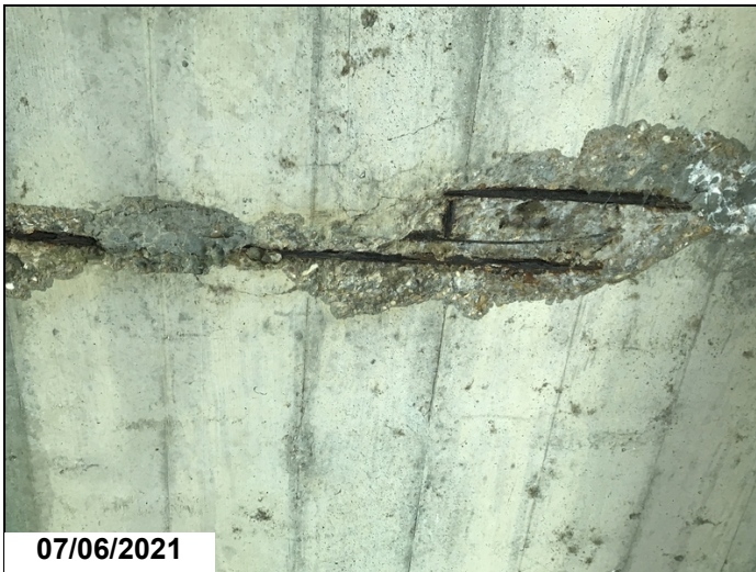
07/06/2021 Spalls with rebar exposed to deck below & to left & right overhang at all spans. Span 5, between girders 3 & 4.
