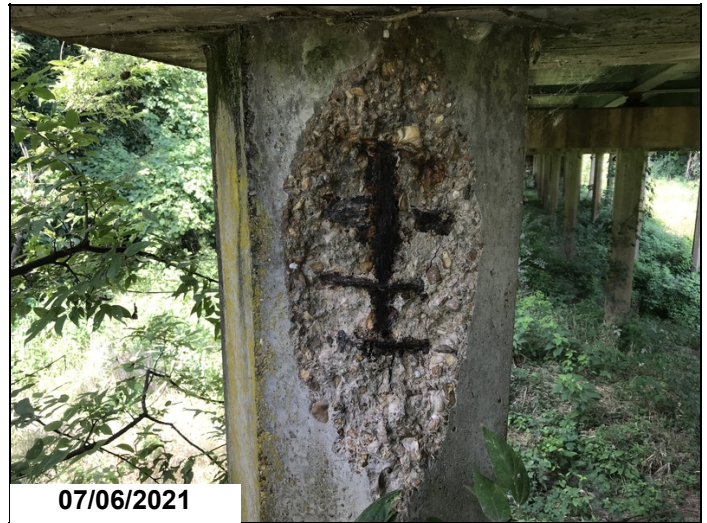
Cracks, delaminated areas & spalls with rebar exposed to Piles at Bents 1, 2, 6 - 12, 14, 15, 17, 19 - 21, 23. Bent 8, pile 4 @ ahead side.
