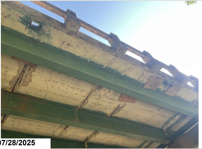
Typical overhangs with efflorescence and exposed rebar.
