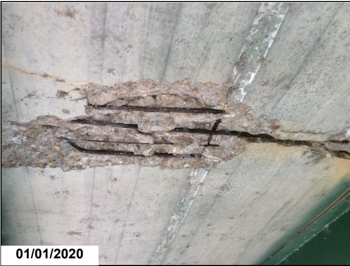
Deep Spall with exposed rebar at Span 19 between Girders 3 & 4.
