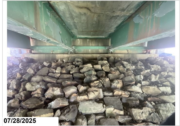
Abutment 1: typical bearings. CS3
