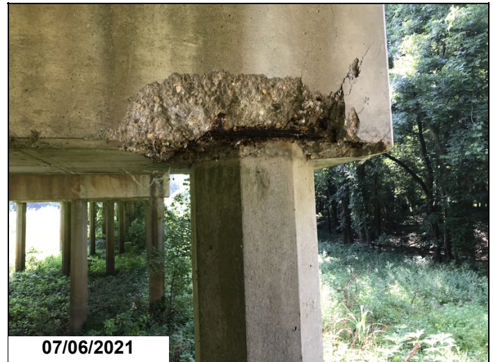
Cracks, delaminated areas & spalls with rebar exposed to caps at Bents 3, 12, 14, 15, 16 - 24. Bent 3 @ pile 4.
