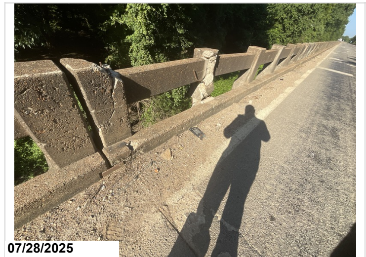
Span 15, right: has a large area of impact damage. 5LF CS3
