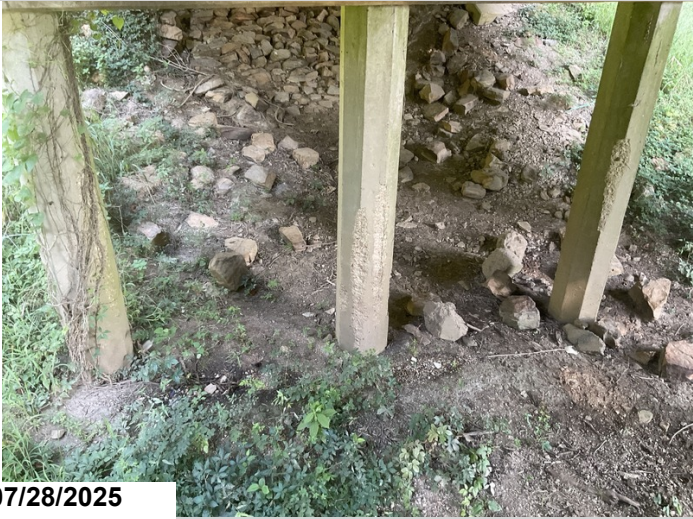
Bent 1, ahead, piles 2-4: have large, shallow, spalls near the ground line. 3EA CS3
