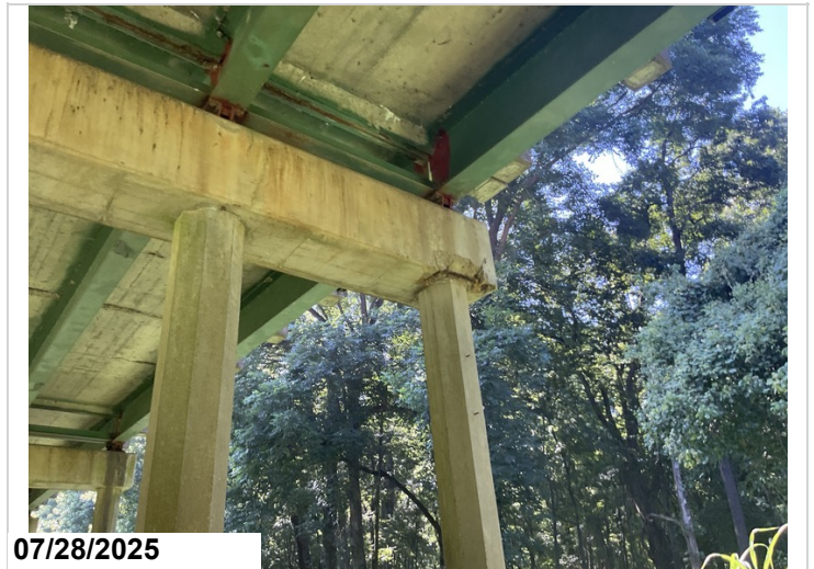
Bent 3 back, right, underside: has spalling with exposed rebar. 2LF CS3
