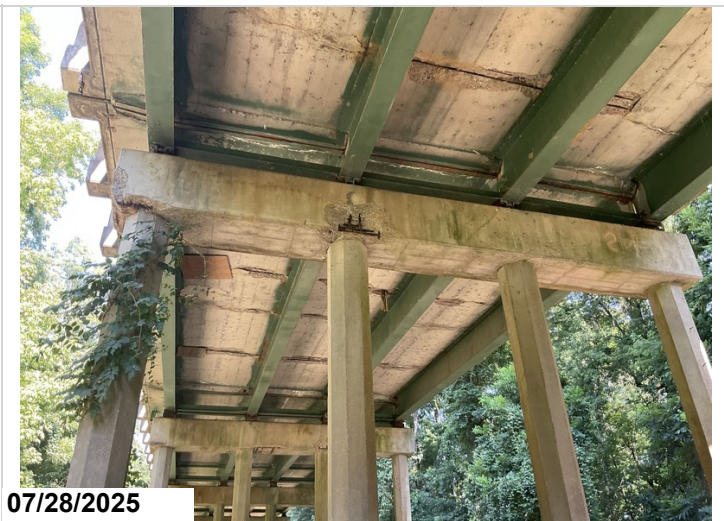
Bent 24 ahead, adjacent to pile 3: has a spall with exposed rebar that has lost adhesion. 2LF CS4
