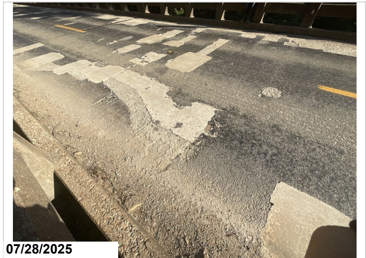
Span 7: has widespread patches and scattered spalls. 102SF CS2 | 24SF CS3
