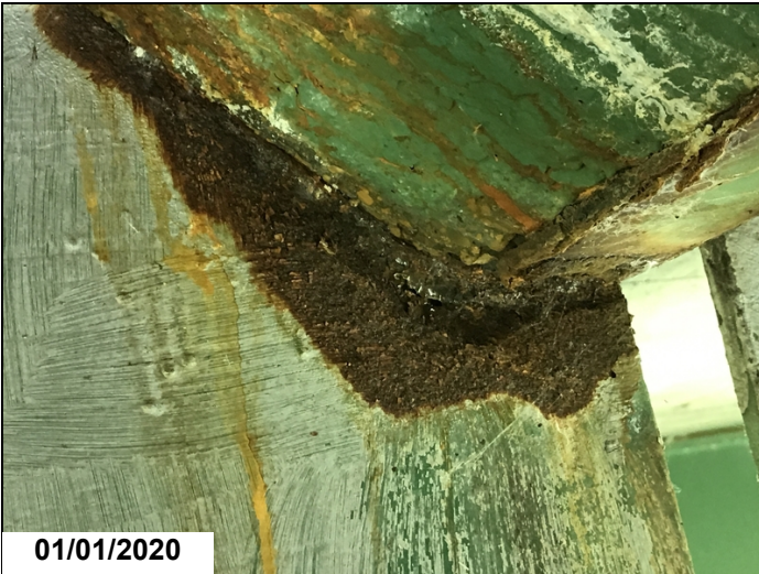
Severe section loss to end of Girder 3 with hole in web below haunch @ Bent 21. - 2020
