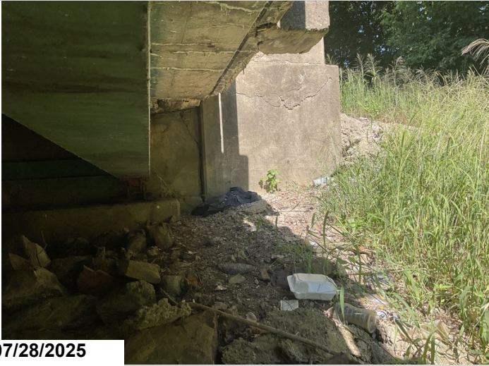
Abutment 1: the left wing has heavy vertical cracks at the abutment connection. 2LF CS3
