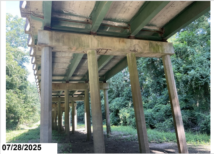
Bent 23 has scattered spalls with exposed rebar. 5LF CS3
