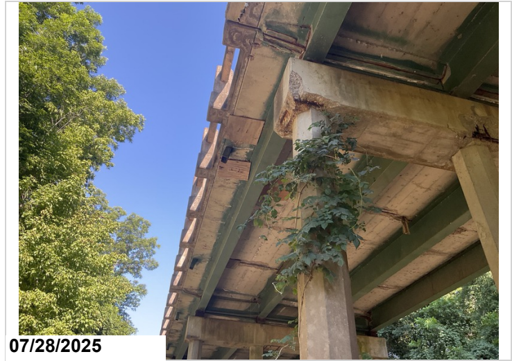
Bent 24 ahead has spalling with exposed rebar. 2LF CS3
