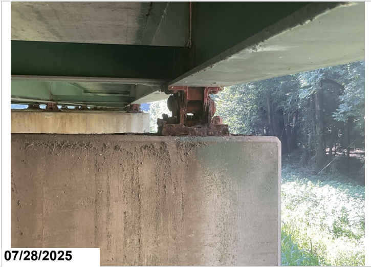
Typical condition of the bearings. CS3
