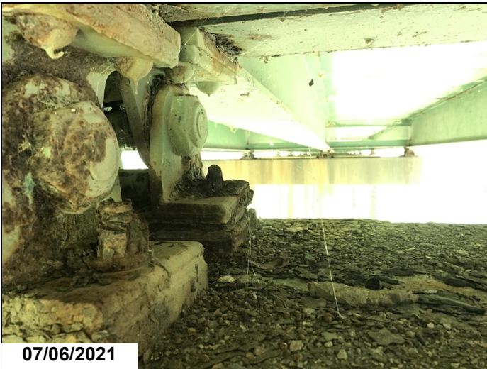
Bent 19 - Girder 3 & 4 has 1 anchor bolt nut missing on ahd. side.
