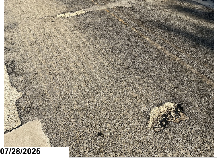
Span 2: has widespread patches and scattered spalls. 118SF CS2 | 10CS3
