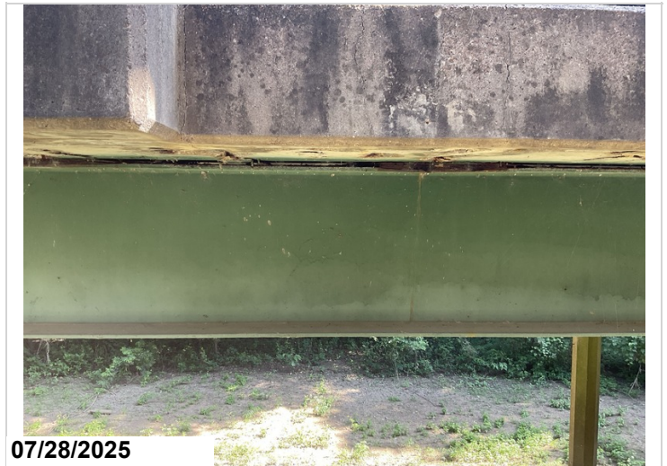
Span 18: all girders have pack rust pushing up on the deck with areas floating. 136LF CS3
