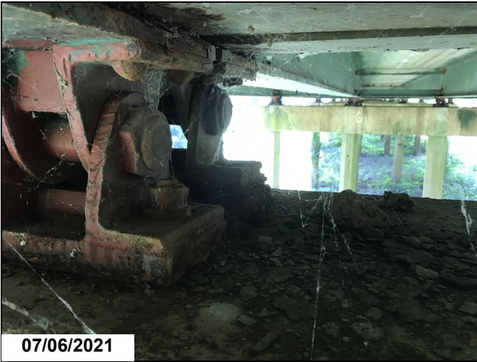
Bearing assem. have heavy rust and section loss & are missing anchor bolts &/or nuts at:
