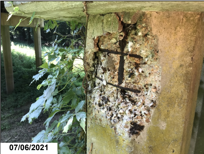
Cracks, delaminated areas & spalls with rebar exposed to Piles at Bents 1, 2, 6 - 12, 14, 15, 17, 19 - 21, 23. Pile 1 @ bent 2.
