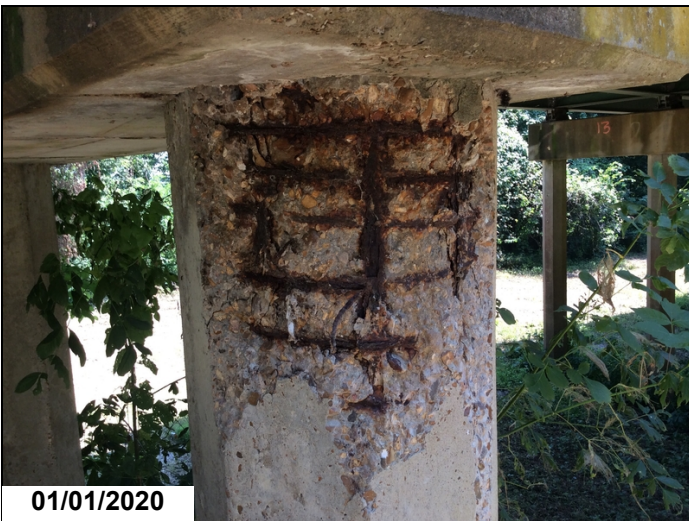
Pile 4 at Bent 12 spalled at top with 6' of exposed rebar with 100% section loss.
