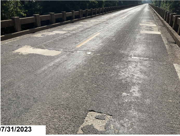
The deck is heavily deteriorated and in need of repair.
