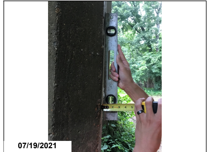
Bent 25, pile 3 is out of plumb.
