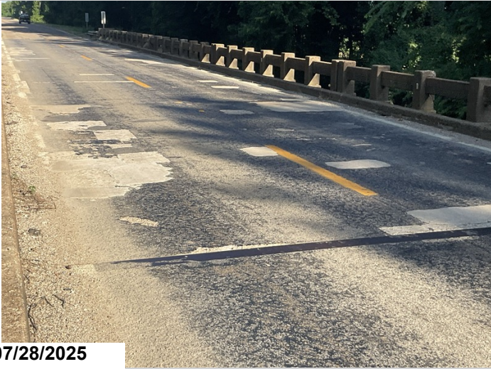
Span 5: has widespread patches and scattered spalls. 139SF CS2 | 17SF CS3
