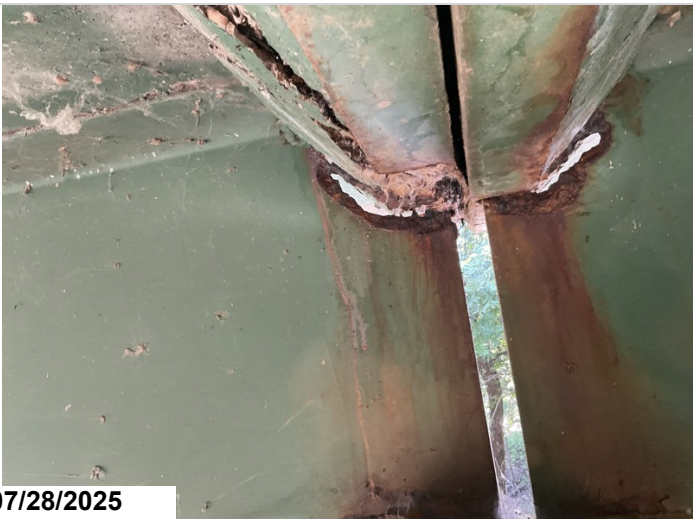
Span 20, bent 19, girder 4: has section loss at the haunch with a 3/4" x 7" hole in the web. 1LF CS4
