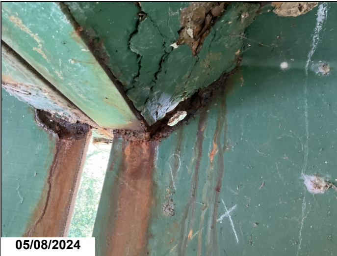
Span 2, Bent 2, Girder 4: 0.5" X 1" Hole in the Web in the Haunch area.
