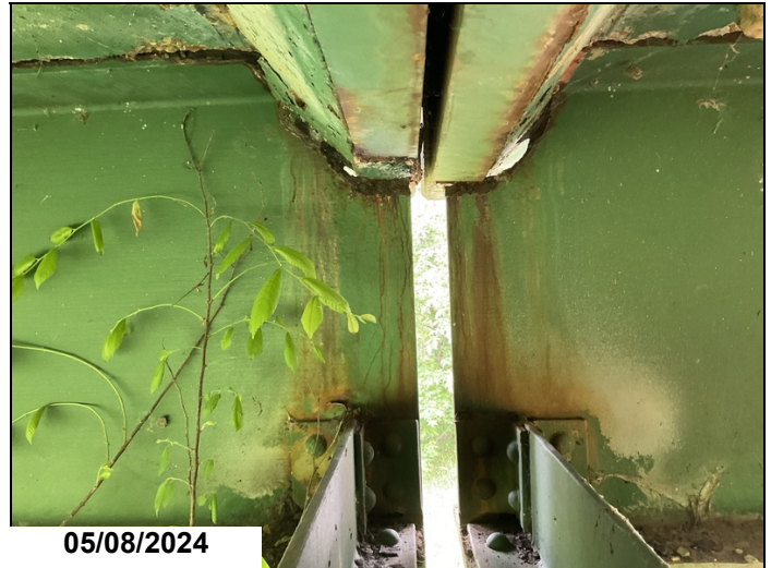
Span 11, Bent 11, Girder 4: 1" X 6" Hole in the Web in the Haunch area.
