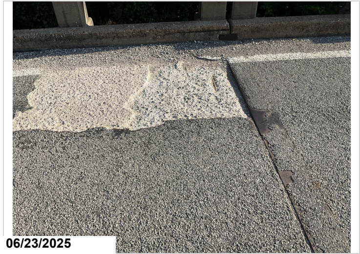
Span 1: Spalls with corroded rebar exposed. 2SF CS3
