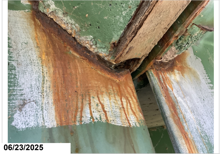
Span 8: EOS: Girder 4: Heavy section loss with 3/4" x 1 1/2" hole in web below haunch. 1LF CS4
