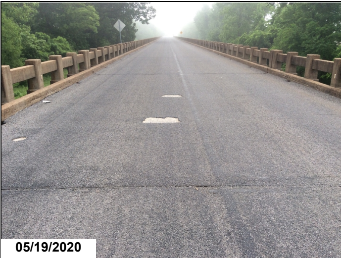
Typical spalls to wearing surface at Spans 4, 5, 8, 16, 20, & 30.
