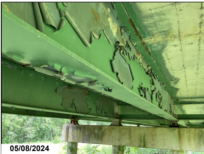
Span 26, Girders: Peeling paint.
