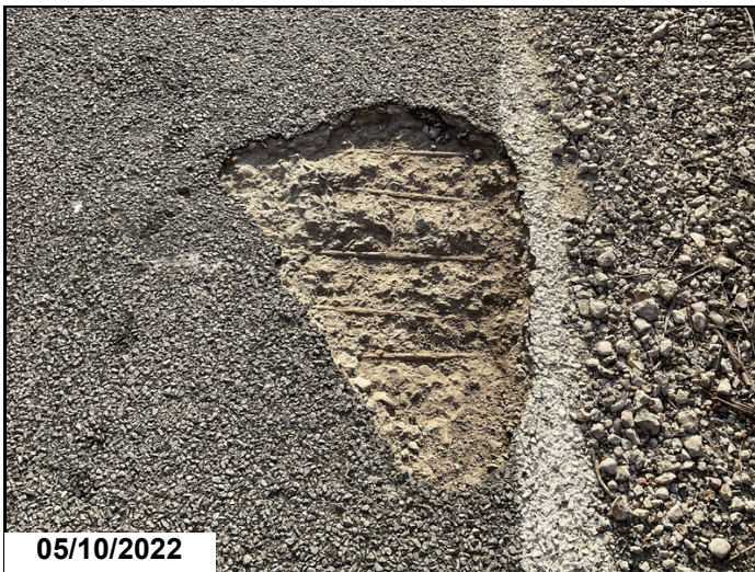
Spall with 3' of rebar exposed to deck @ span 26.
