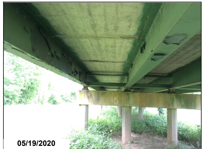
Girders 3 & 4 @ Span 19. Paint peeling.
