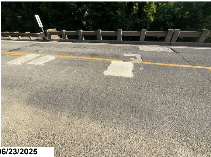
Span 1: Spalls/unsound patches. 33SF CS3
