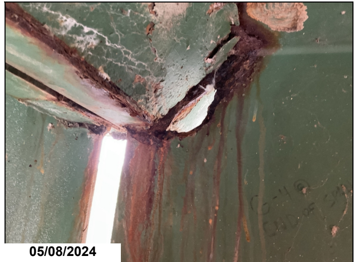
Span 5, Bent 5, Girder 4: 2" X 4" Hole in the Web in the Haunch area.
