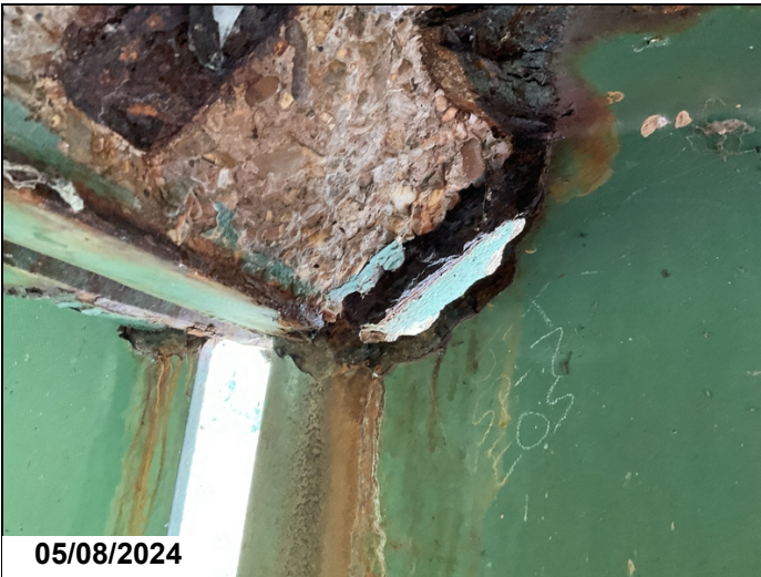
Span 7, Bent 7, Girder 4: 1.25" X 5" Hole in the Web in the Haunch area.
