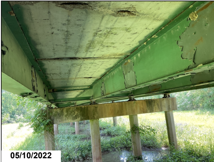
Paint peeling to girders 1-4 @ span 24.
