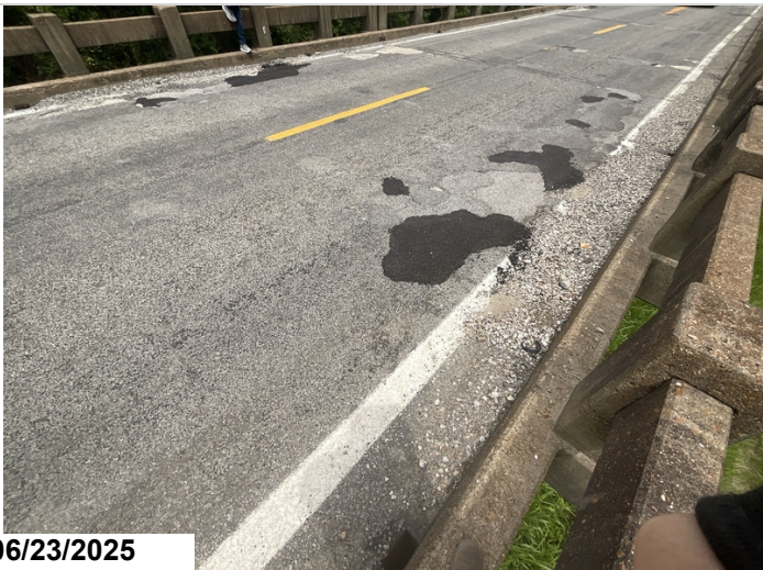
The gutters have widespread debris
