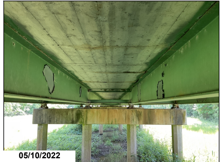
Spans 19 - 24, and 26 - 30 Paint peeling at girders 1 - 4 with surface rust in exposed areas. Girders 2, 3, & 4, span 21.
