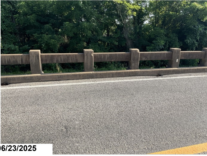
Typical post spalling.
