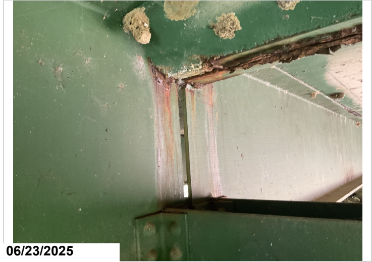
Typical area of minor section loss at the haunches.
