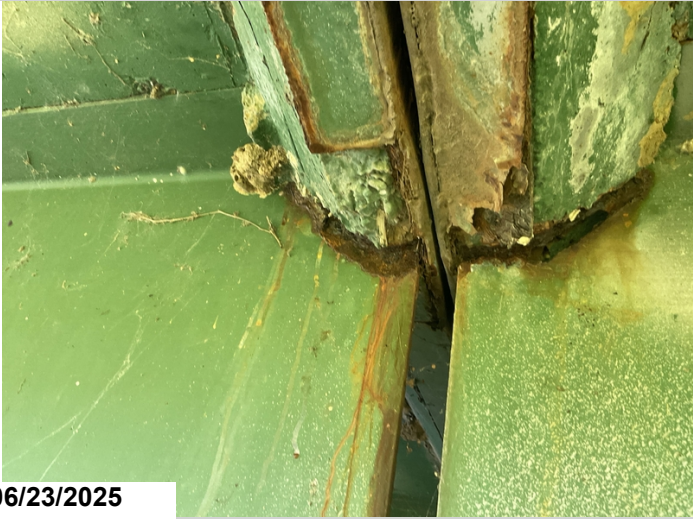
Span 2: EOS: Girder 1: Heavy section loss with 1/2" x 3/4" hole in web below haunch. 1LF CS4
