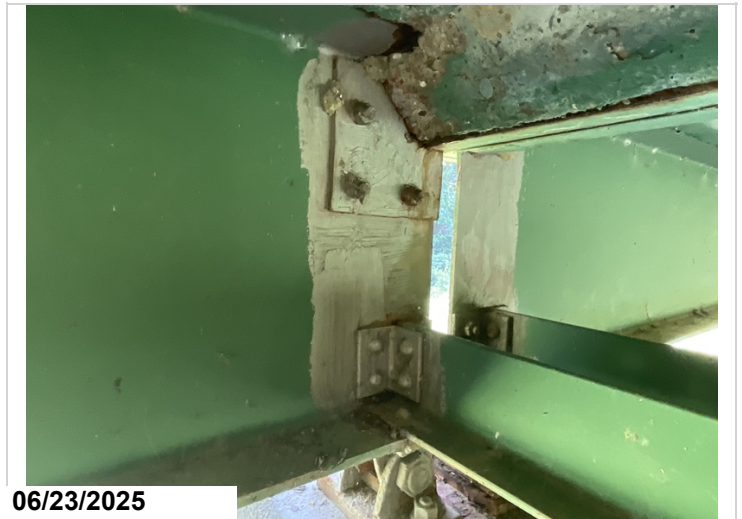
Span 12, bent 12, girder 1: repair
