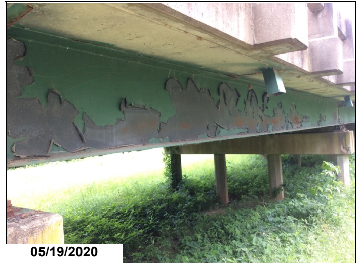
Girder 4 @ Span 19. Paint peeling with rust.
