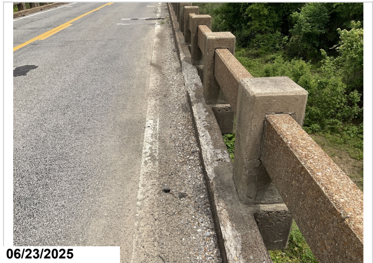
Span 1, right curb: deterioration.
