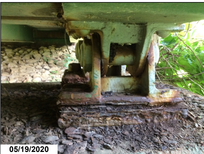
Bearing 1 Bent 1 ahead has bolt missing.
