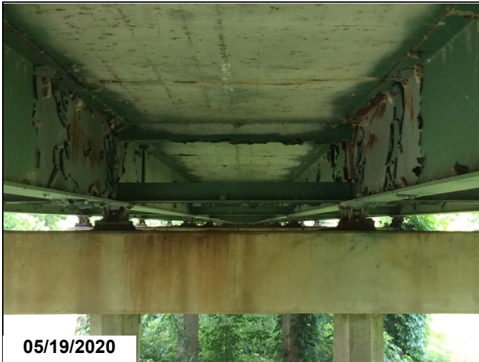
Paint peeling with rust to Girders 2 & 3 @ Span 29.
