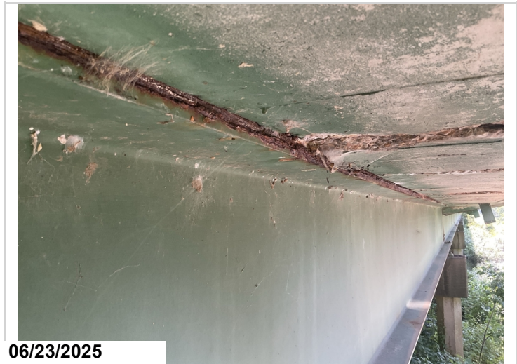
Typical pack rust lifting the deck over the girders.
