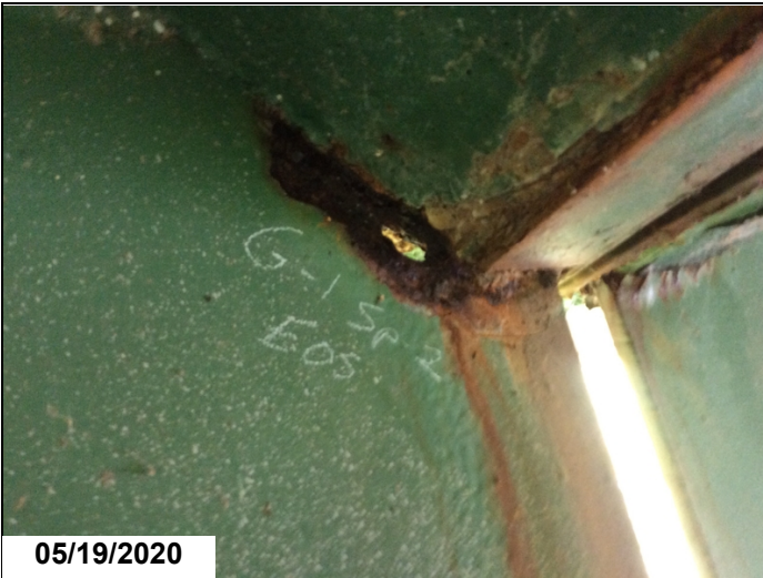
Hole in web @ paving haunch @ Girder 1 end of Span 2.
