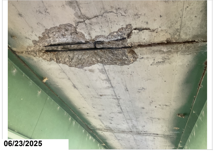
Span 9, bay 2: typical rebar
