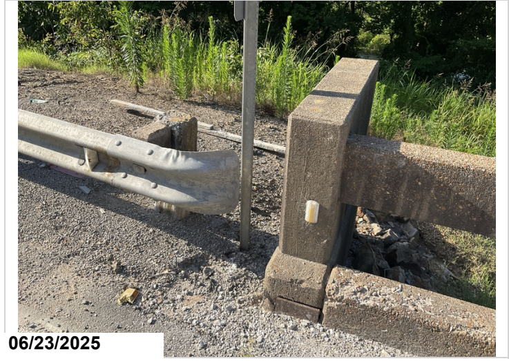
The transitions are not attached to the bridge.
