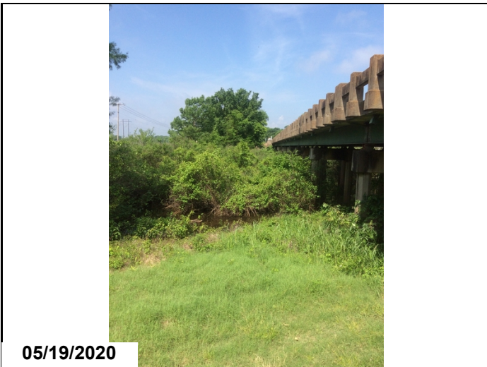
Spans 3 - 8 has heavy vegetation and trees growing along Left & Right sides of bridge. (Looking back)
