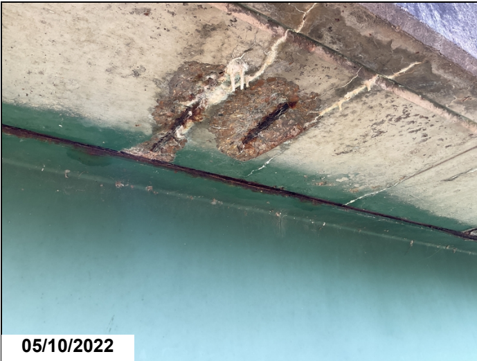
Soffit: Spalls with rebar exposed to soffit and Lt and Rt overhangs at all spans. Span 2, Rt overhang
