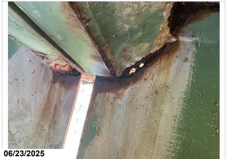
Span 4: EOS: Girder 4: Heavy section loss with 1/2" x 2" hole in web below haunch. 1LF CS4
