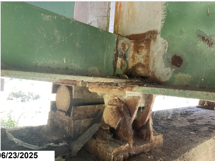
Typical diaphragm connections over the bents.
