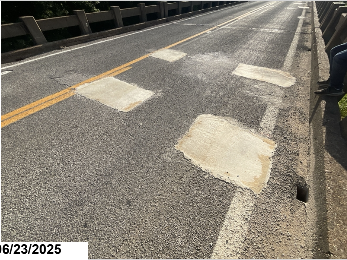
Typical deck patching.
