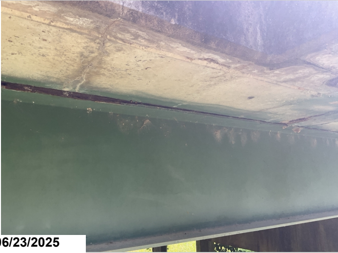
Span 23, girder 4, midspan: has pack rust between the top flange and the deck creating a 1/2" gap. 15LF CS3
