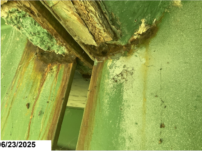
Span 11: EOS: Girder 4: Heavy section loss with 1" x 7 1/2" hole in web below haunch. 1LF CS4
