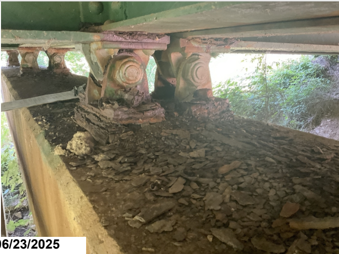
Bent 1: bearings
