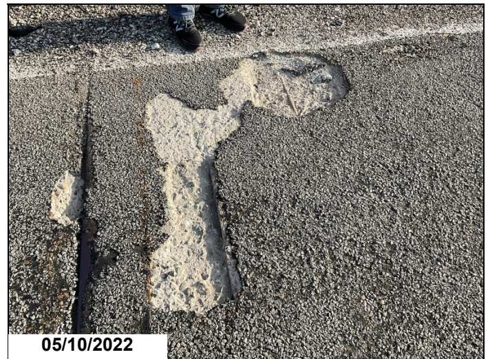
Deep spall with rebar exposed to deck @ span 12.
