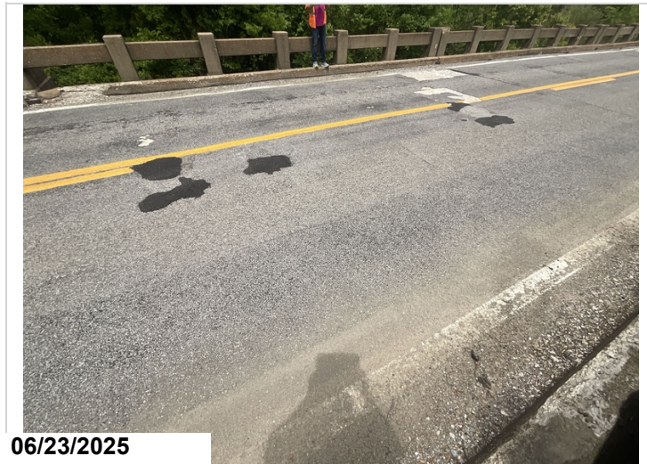
Span 1: typical patches and spalls
