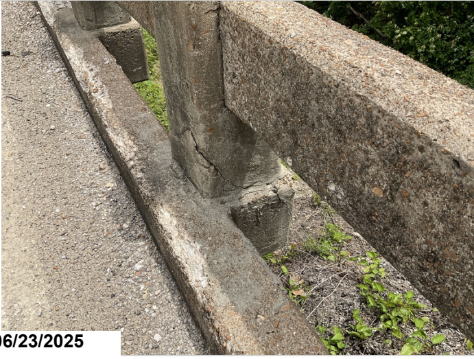
Span 1, right: typical cracking
