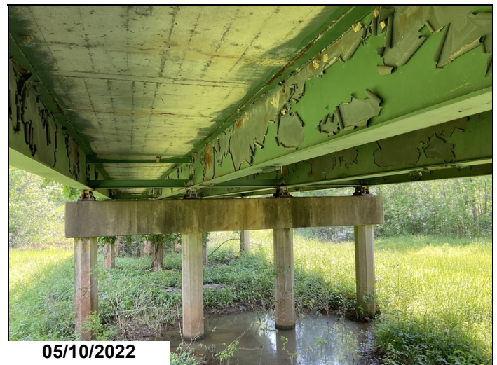
Typical Paint peeling to girders 1-4 @ span 26.
