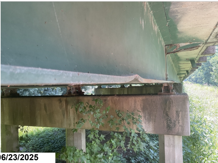
Span 13: Midspan: Girder 4: Bent bottom flange. 1LF CS3
