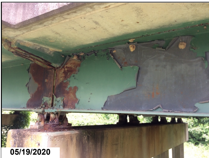
Paint peeling with rust to Girder 4 over Bent 28
