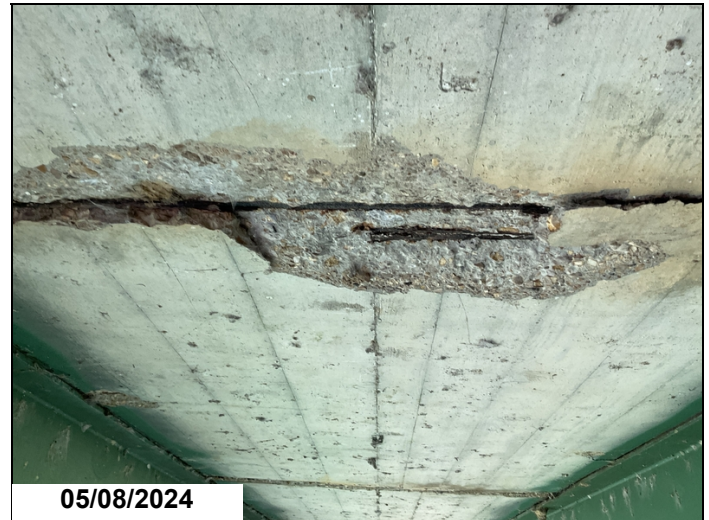
Span 13, Undersurface: Spalling with 40' of exposed reinforcing steel with section loss.
