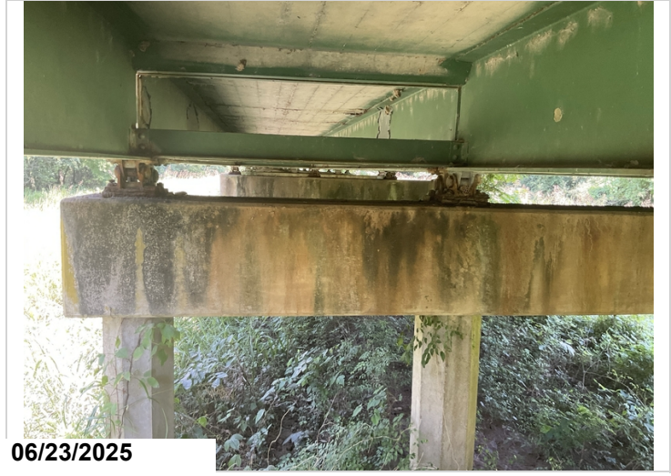
Typical bearings with heavy corrosion.
