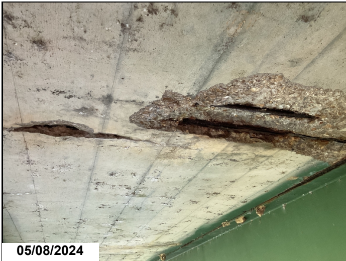
Span 2, Bays 1 - 3: Spalling with 31' of exposed reinforcing steel with section loss.
