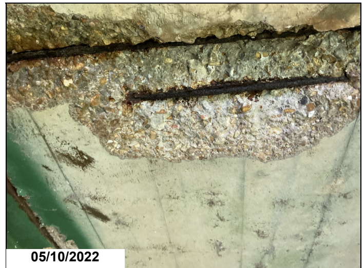
Soffit: Spalls with rebar exposed to soffit and Lt and Rt overhangs at all spans. Soffit @ Span 2.
