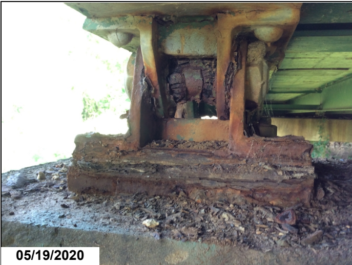
Bearing 4 ahead @ BOS 3 has heavy pack rust with both bolts missing.
