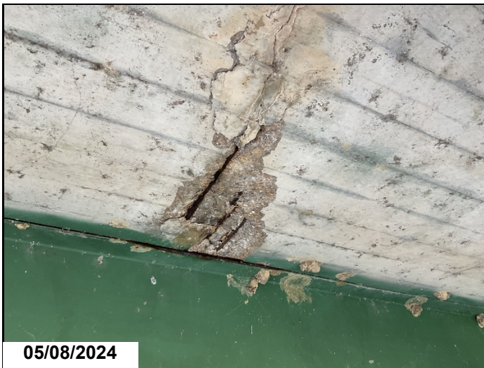
Span 4, undersurface: Spalling with 28' of exposed reinforcing steel with section loss.
