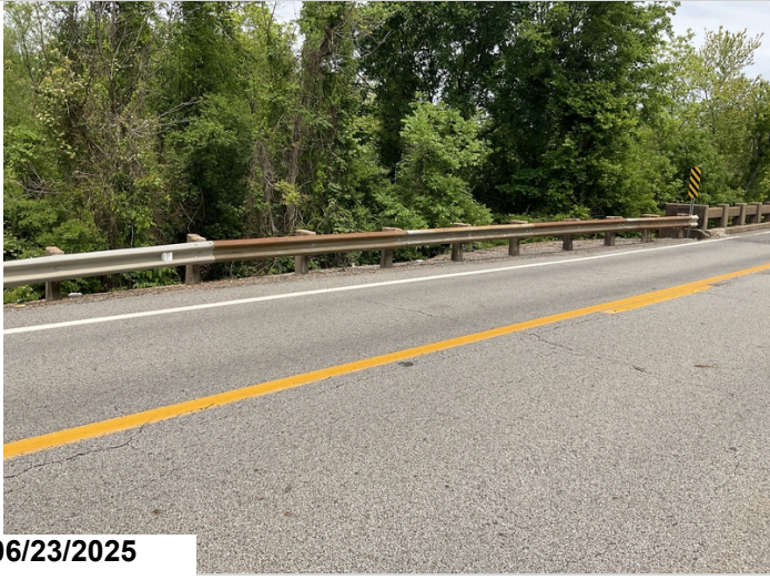
The transitions are not attached to the bridge.
