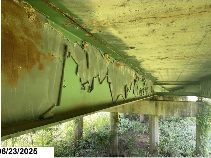
Span 26 paint condition.
