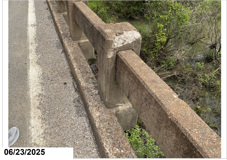
Span 8, right: post 2: spalling
