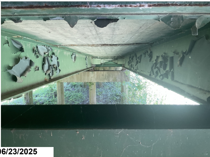
Span 19, girders 3 and 4: have peeling paint throughout.
