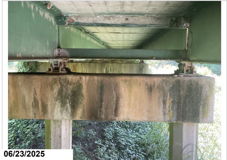
Typical with rust and pack rust
