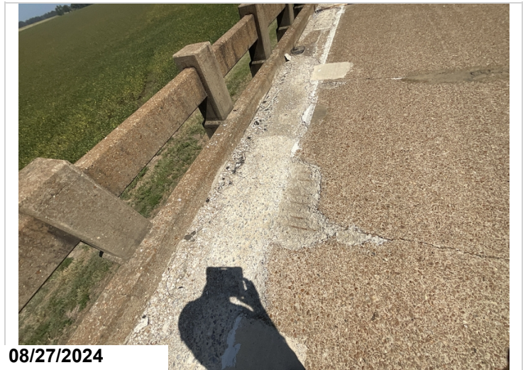
Span 6, left, driving surface: has a spall with exposed rebar. 3SF CS3
