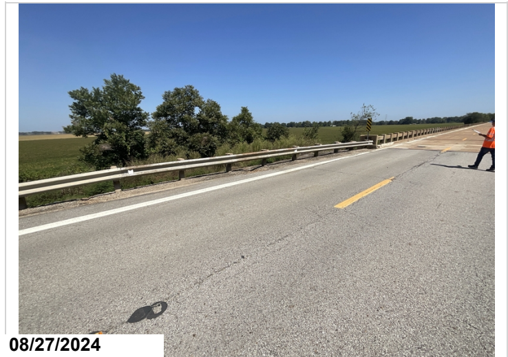
The railing transitions are in good condition with minor surface corrosion throughout.
