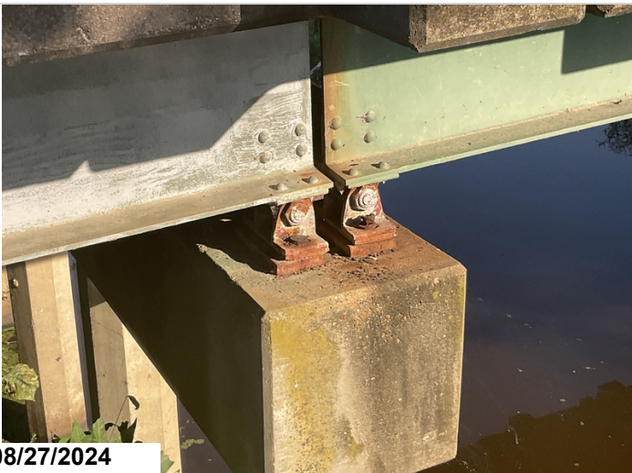
Bent 1, back, bearing 4: the masonry plate is beginning to slide out. Bearings 3 and 4 on the ahead side are similar. 3EA CS3
