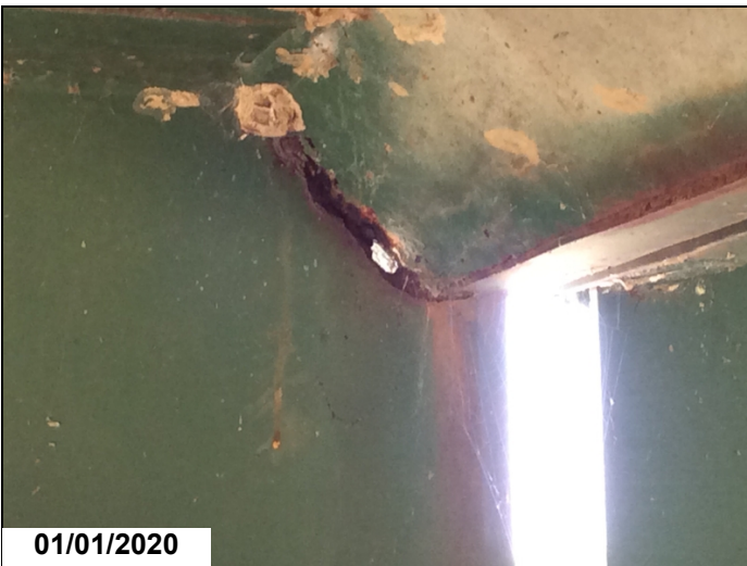
Hole in web below paving haunch @ Girder 1 EOS 16.
