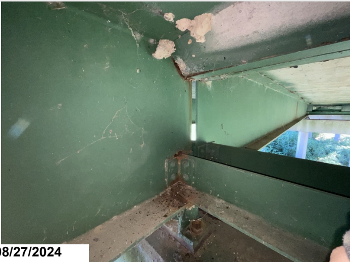
Bent 8, back, girder 2: has a 1"x2" hole at the haunch. 1LF CS3
