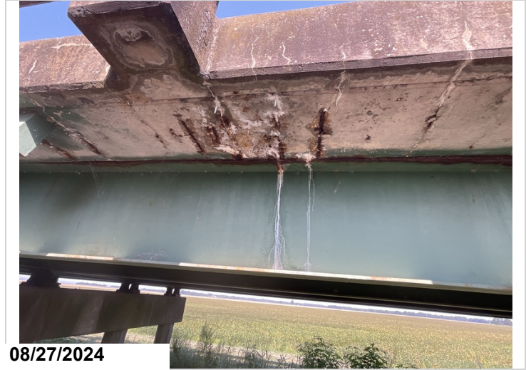
Span 8, right: heavy deterioration typical to curbs and overhangs.
