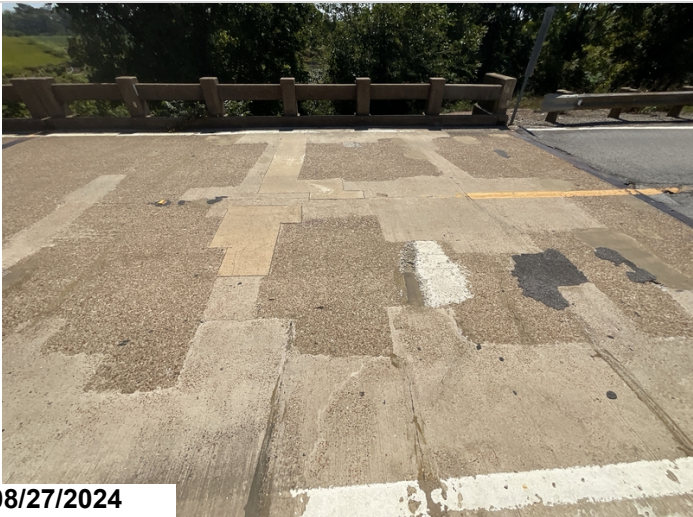
Span 1: has extensive patched areas covering 40% of the driving surface.
