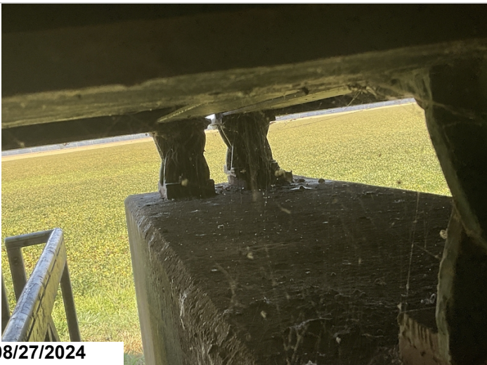
Bent 6, ahead, bearings 1-4: have missing anchor bolts/nuts. Bearing 1 is moving off of the masonry plate. 1EA CS3
