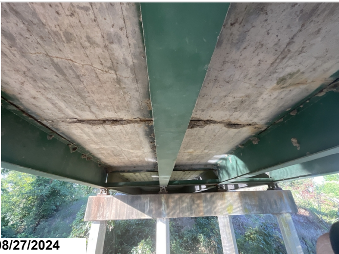
Span 2, bays 1-3: have full-width exposed rebar. 28SF CS3
