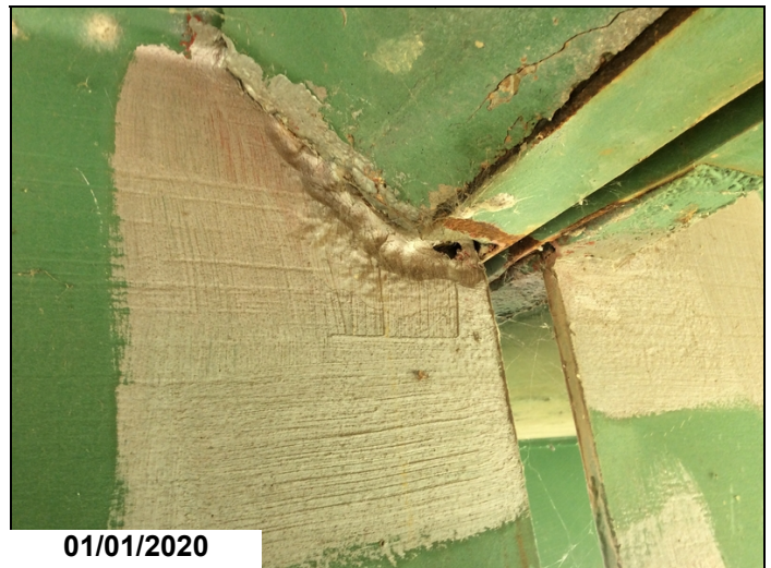
Hole in web below paving haunch of Girder 3 @ EOS 22.
