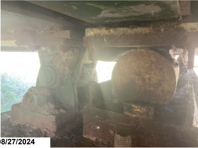
Bent 4, ahead, bearings: have been replaced. Bearings 2 and 3 are non bearing. 2EA CS2 corrosion, 2EA CS3 connection.
