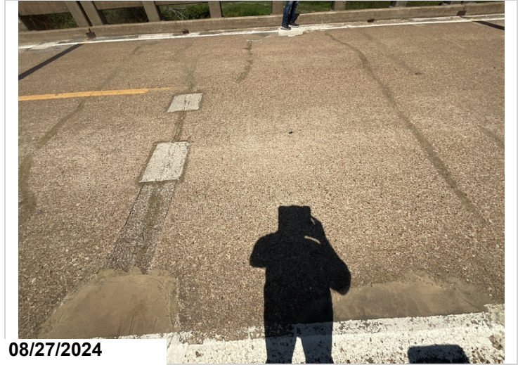
Typical driving surface with patched areas and cracks throughout.
