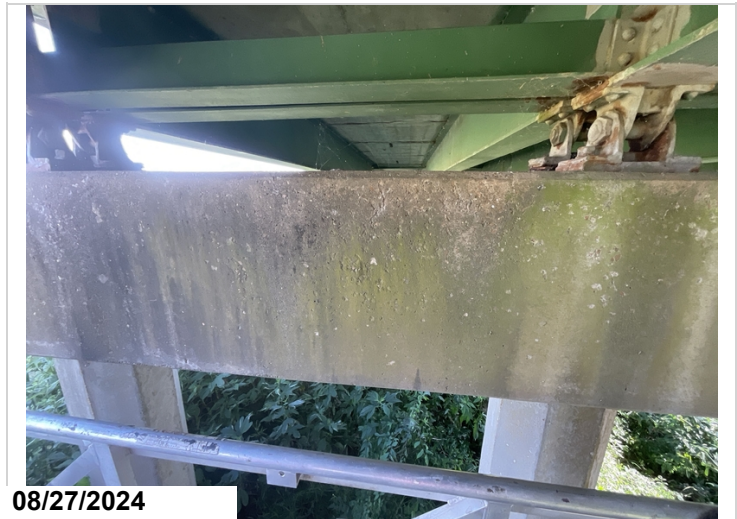
Typical minor cracking to caps.
