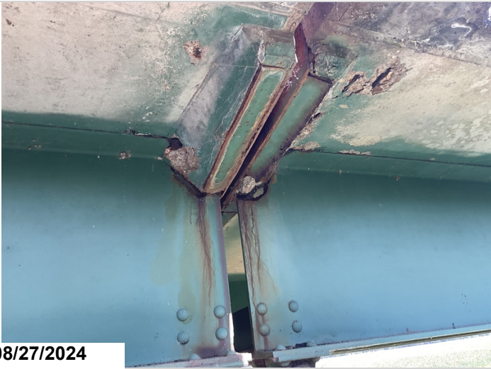
Bent 18, ahead, girder 4: has corrosion with a hole in the haunch area at the beam end measuring 1"x2". 1LF CS3
