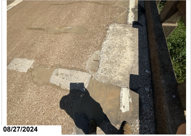
Span 9, right, driving surface: has exposed rebar 2'. 2SF CS3
