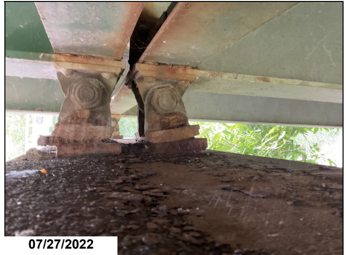
Moveable Bearings at Bents 1 through 7 are all rotated. Bent 1.
