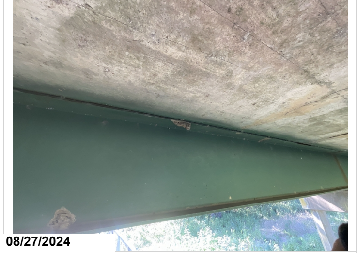
Span 9, midspan, girders 1-3: Typical separation of the deck due to pack rust and corrosion in the top flanges. 60LF CS3
