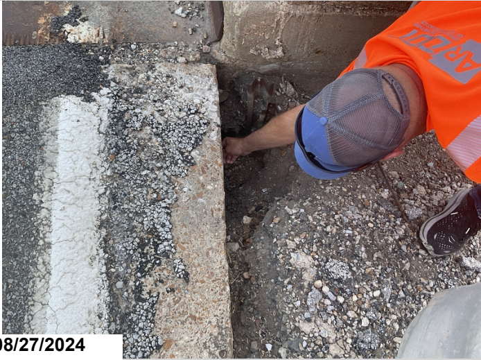
Abutment 1, right: 6' folding rule inserted all the way. Left side similar. Void presumed to go all the way across.
