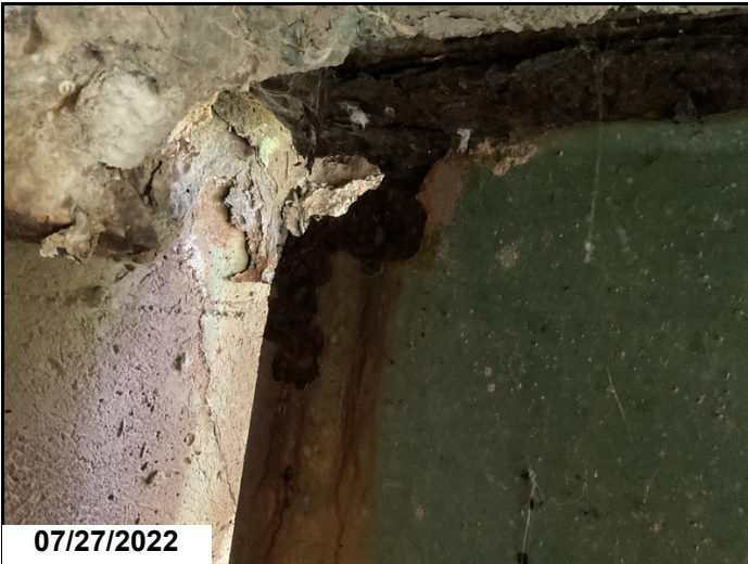
Abutment 2, girder 4 has heavy deterioration and holes at the top flange and web at end of span. Knife edge to the remaining web at the end of girder and to the top flange 1.5' back.
