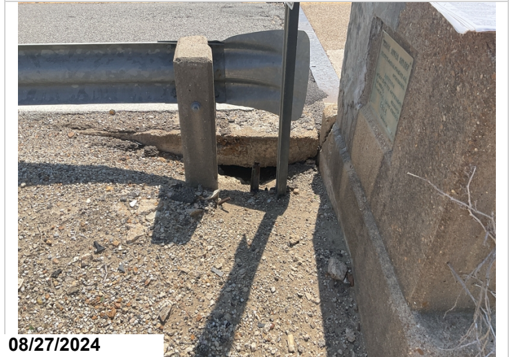
Abutment 2 left: Void under slab. Probing did not produce an end to the void on this side. On the right side, the void was 4' back under the approach slab.
