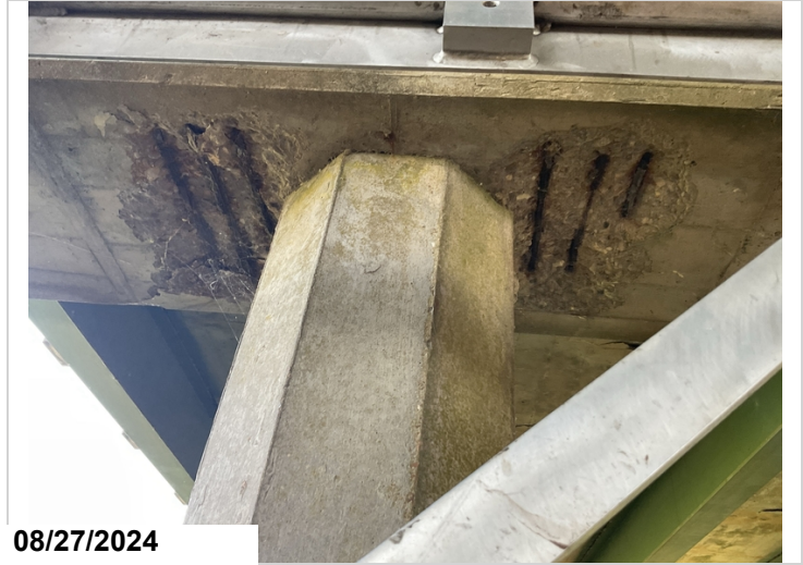
Bent 14, cap, adjacent to pile 2: has a large spall with exposed rebar in the underside. The rebar has completely corroded in two at this location. 6LF CS3
