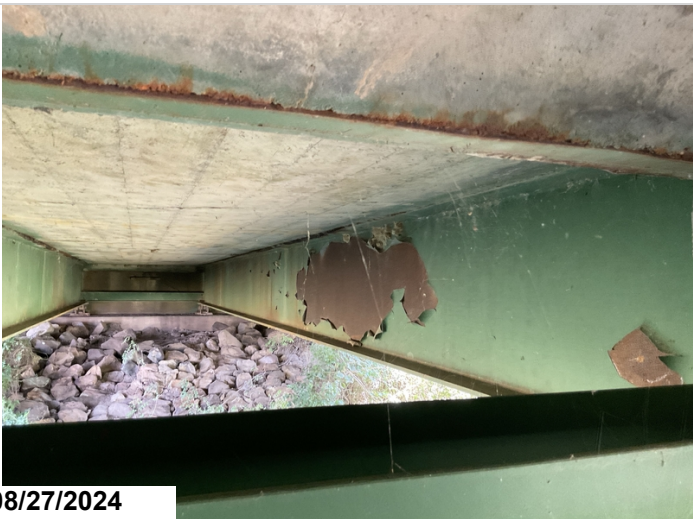
Span 31, girder 3: has a large area of peeled paint at midspan. 36SF CS4
