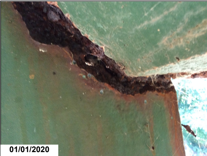
Hole in web below paving haunch @ Girder 4 @ BOS 19.
