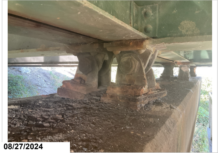
Bent 1, back: all bearings are rotated ahead. 4EA CS3 alignment
