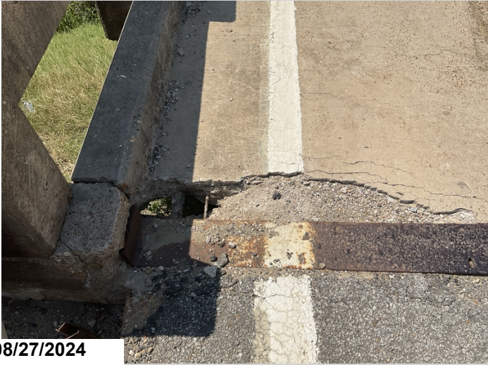
Abutment 2, right: 1'x2' hole in the deck at the shoulder
