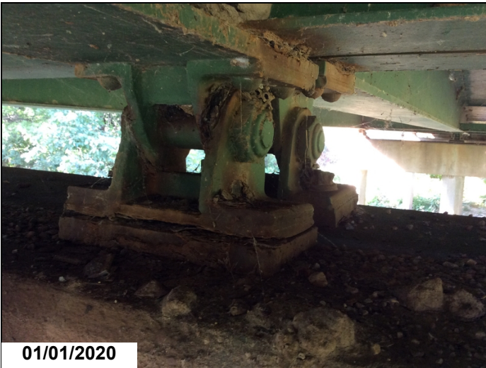
Anchor bolt & nut missing @ Bearing 3 @ Bent 3.
