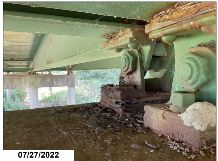
Several Bearing assemblies thru-out are missing Anchor Bolts and/or Nuts. Bent 18 bearings 2 - 4.
