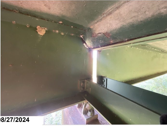
Bent 10, back, girder 1: has a 4" x1.5" hole at the haunch. 1LF CS3
