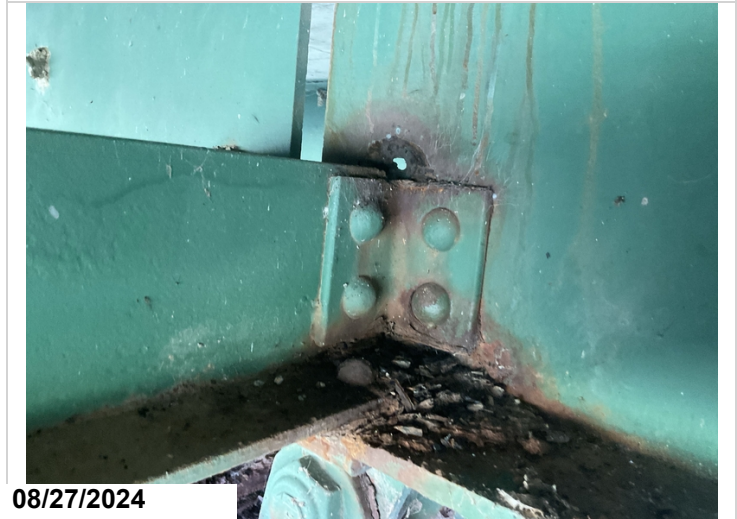
Bent 6, back, girder 3: has a 1" hole in the web above the diaphragm connection. 1LF CS3
