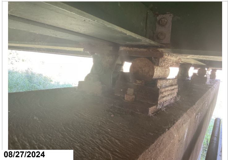
Bent 4, ahead, bearings: have been replaced. Bearings 2 and 3 are non bearing. 2EA CS2 corrosion, 2EA CS3 connection.
