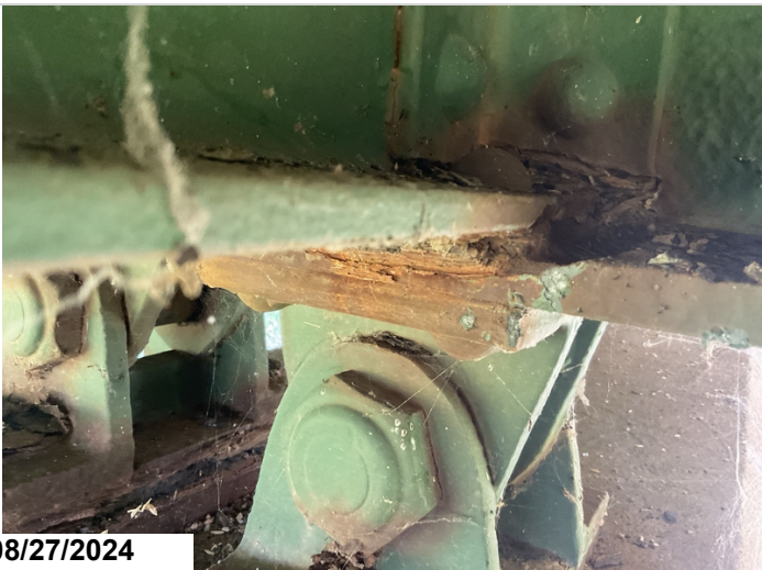
Bent 13, back, girder 3: typical section loss to the bottom flange. 1LF CS3
