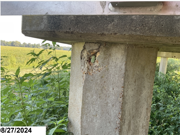
Bent 11, pile 1 spall. Move to pile photos.
