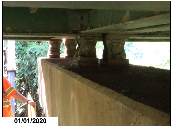
Moveable bearings @ Bent 2 are rotated ahead.
