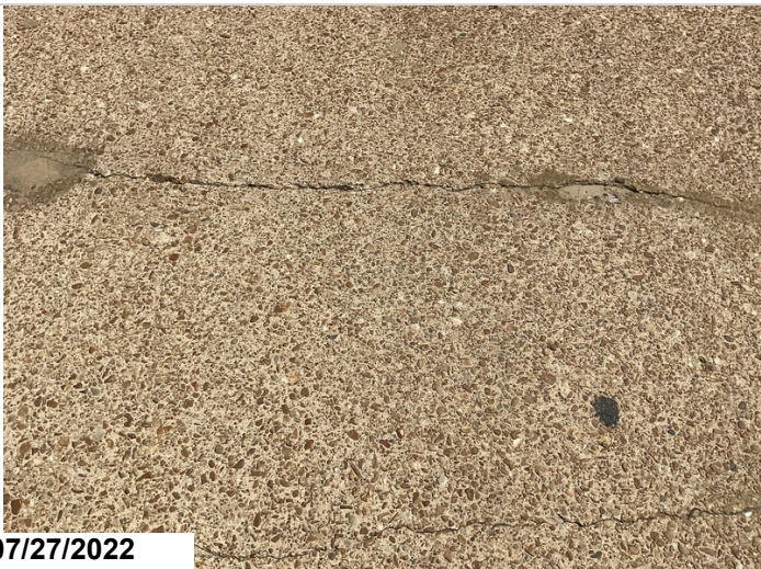
All spans have unsealed cracks.
