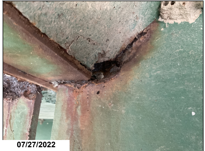
Holes rusted in the webs of Girder Ends under concrete haunch at End of Span at: Girder 2 @ bent 3.
