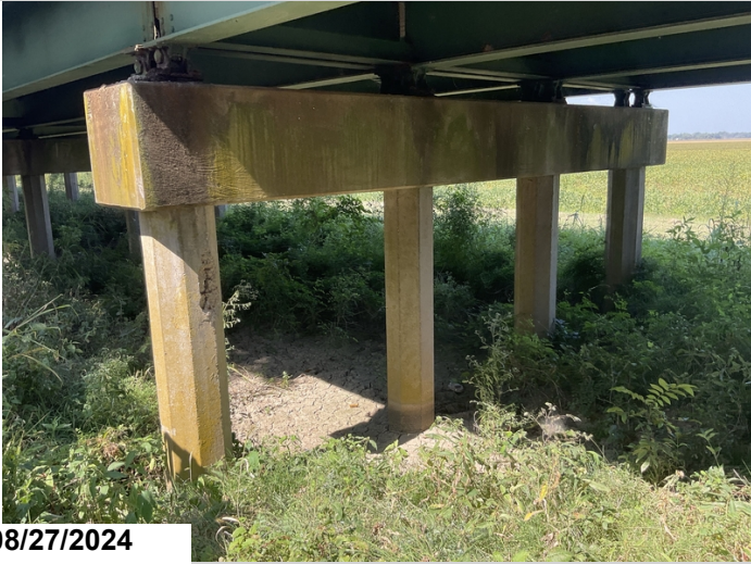
Bent 18, pile 4: has a spall with exposed rebar. 1EA CS3
