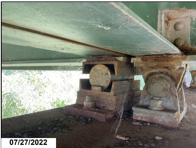
Moveable Bearing 3 @ Bent 29 is non-bearing.
