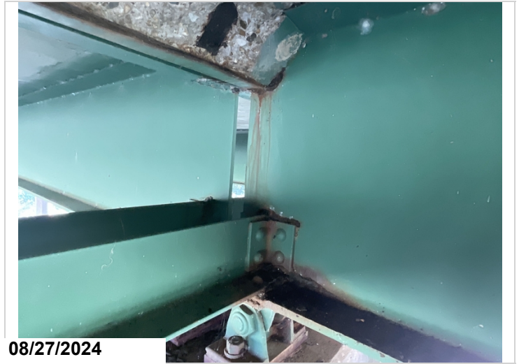
Bent 17, back, girders: have corrosion with section loss in the beam ends. Girder 3 has a 1" diameter hole in the same area and 1/8" section loss at the web to bottom flange connection. 4LF CS3
