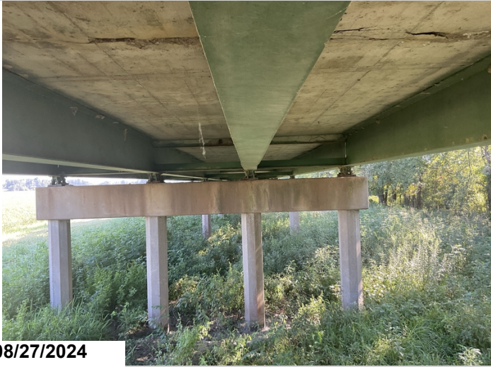
Span 5, girder 3: is bowed halfway between midspan and bent 5. 2LF CS3
