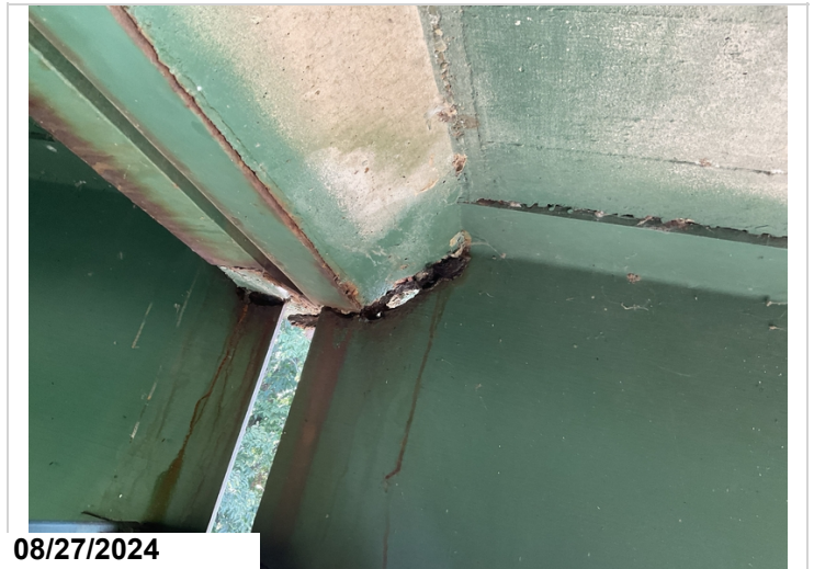
Bent 13, back, girder 4 has a 4"x1" hole in the haunch area. 1LF CS3
