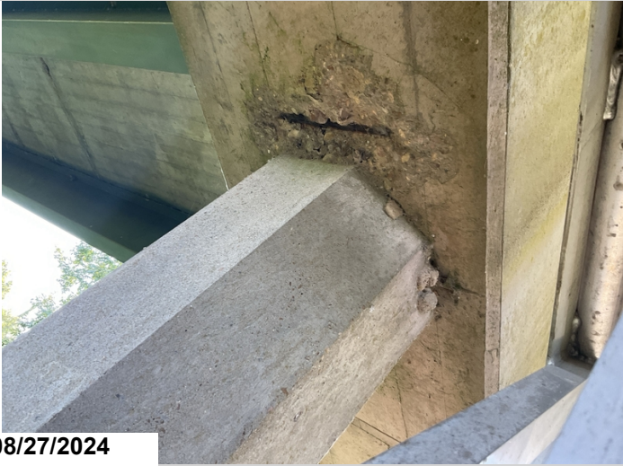
Bent 9, adjacent to pile 3, cap: has a spall with exposed rebar in the underside. 1LF CS3
