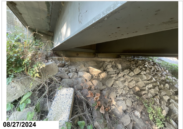
Abutment 1: efflorescent cracks are widespread. 13LF CS3
