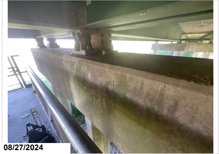
Bent 14, ahead, bearings 1-3 have been replaced and have only minor surface corrosion. 3EA CS2
