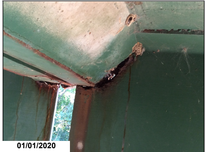
Holes in web below paving haunch @ Girder 4 EOS 13.
