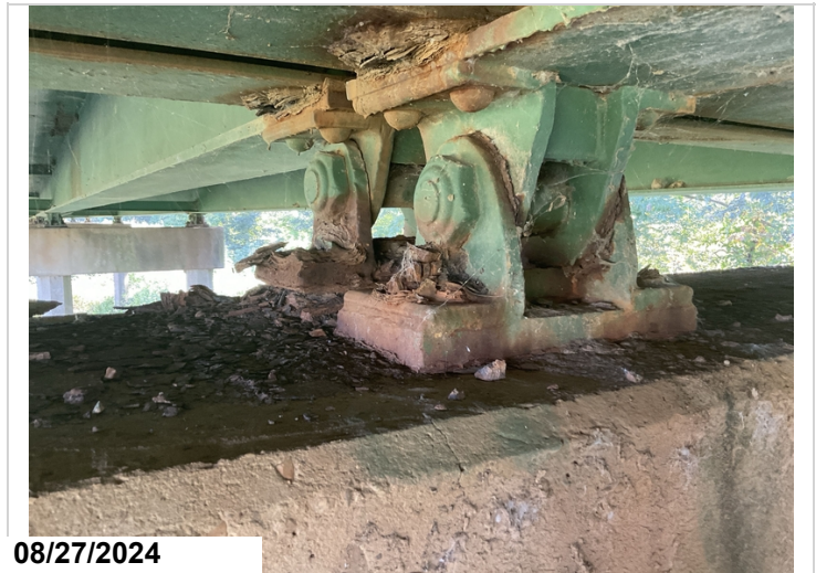
Typical bearings have heavy corrosion
