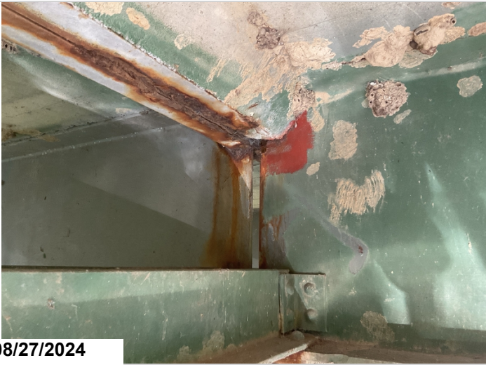
Bent 1, girders: have corrosion with section loss at the haunches. 8LF CS3
