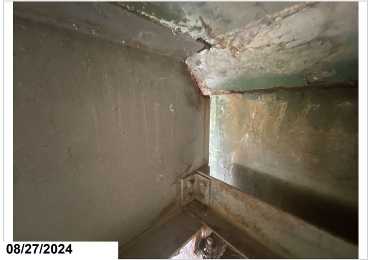
Abutment 1, girder 4: has 3/16" section loss at the haunch. 1LF CS3
