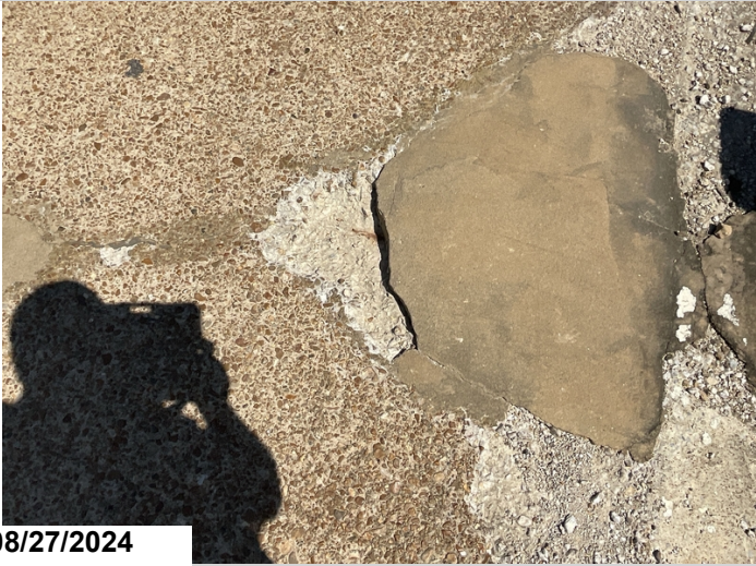
Span 6, left and right lanes, driving surface: have spalls with exposed rebar. 4SF CS3
