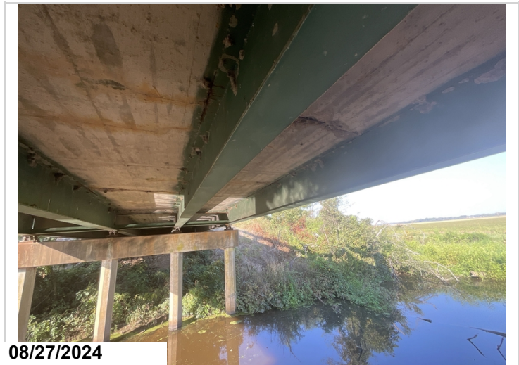
Span 2, midspan, girders 1-4: have corrosion in the top flange at the deck connection. 40LF CS3
