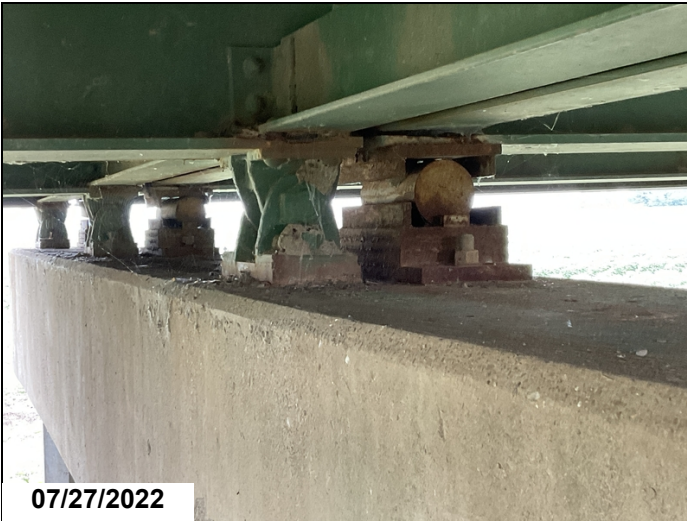
Moveable Bearings 2 & 3 @ Bent 4 are non-bearing.
