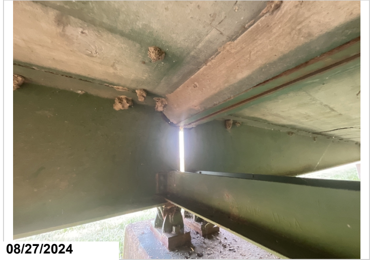
Bent 3, back, girder 1: has a 1/4" diameter haunch hole. 1LF CS3
