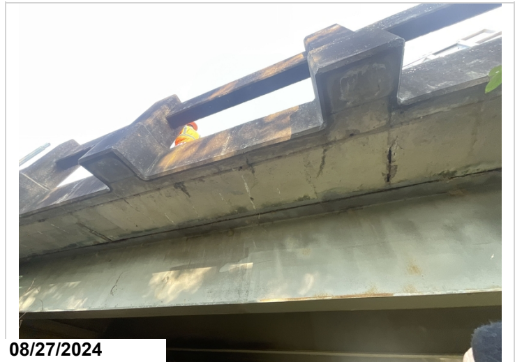
Span 1, right: Typical exposed rebar and efflorescent cracks to overhangs.
