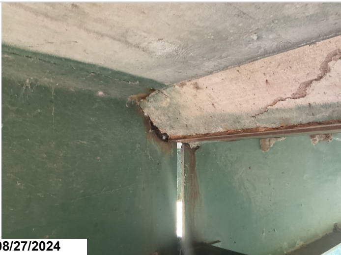
Bent 3, back, girder 2: has a 1/2" hole at the haunch. 1LF CS3
