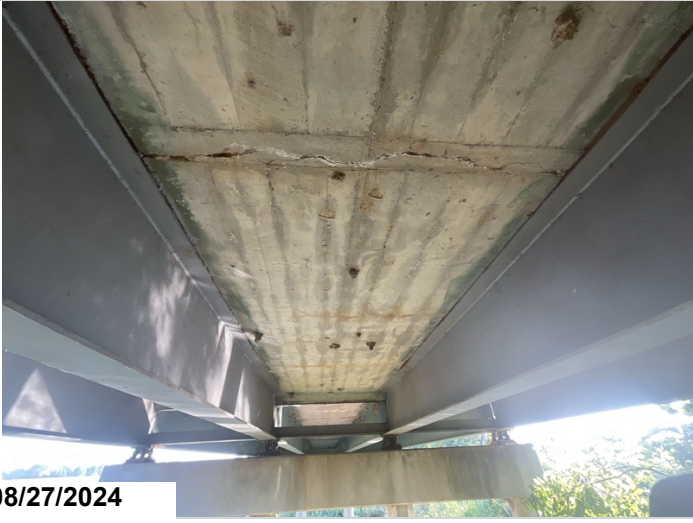
Transverse efflorescent cracks are widespread .
