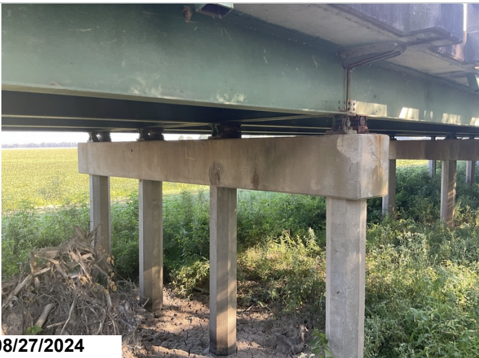
Bent 4, back, over pile 3: has a spall with exposed rebar. 1LF CS3
