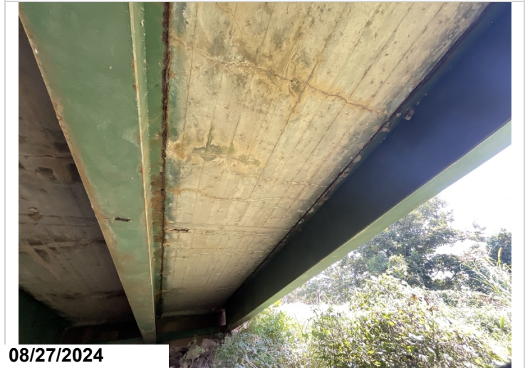
Span 31, girder 4: has a 4"x3" haunch hole. 1LF CS3
