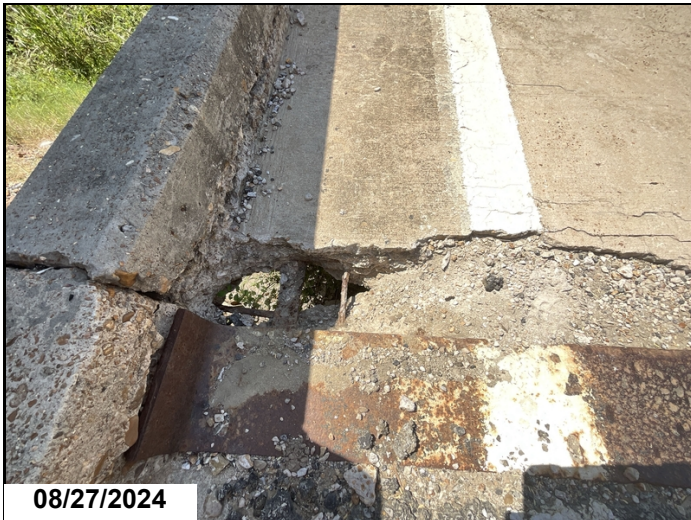
1x2' hole in the right shoulder span 31
