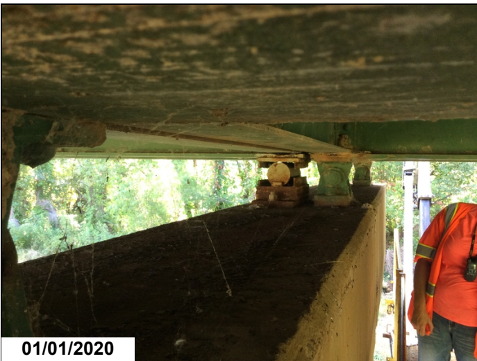
Moveable bearings @ Bent 4 are non bearing.
