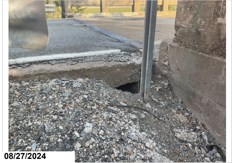
Abutment 1, right: voids under approach slab.
