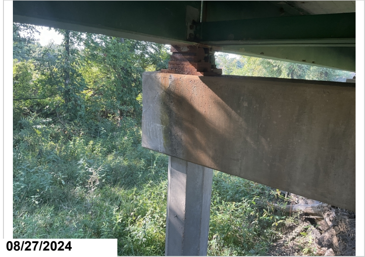
Bent 4, ahead, under bearing 4: there is a moderate diagonal crack. 1LF CS3
