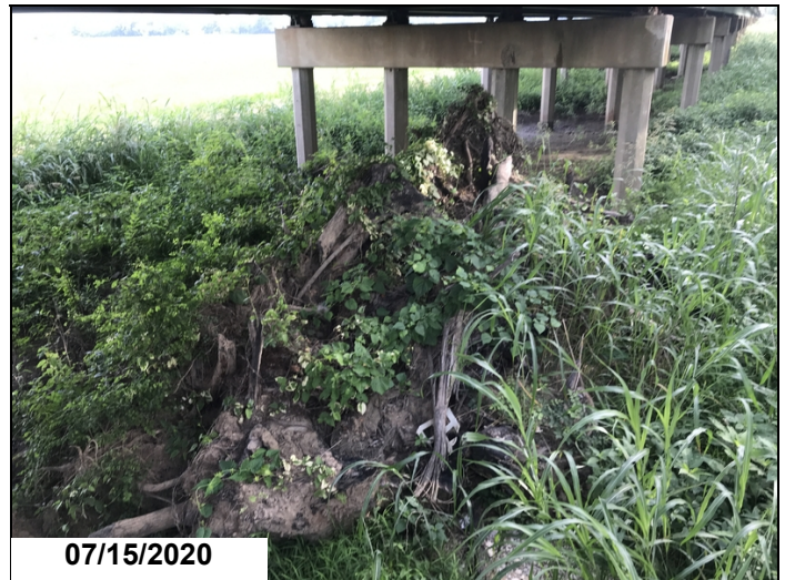
Span 4: Large pile of debris (brush) pushed up in pile under bridge.
