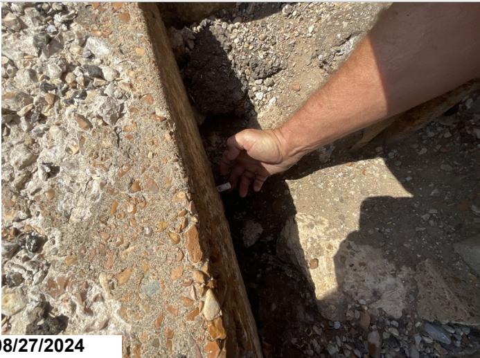
Abutment 2 left: Void under slab. Probing did not produce an end to the void on this side. On the right side, the void was 4' back under the approach slab.
