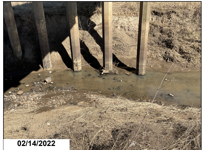
Scour to Piles 1 - 5 @ Bent 3.
