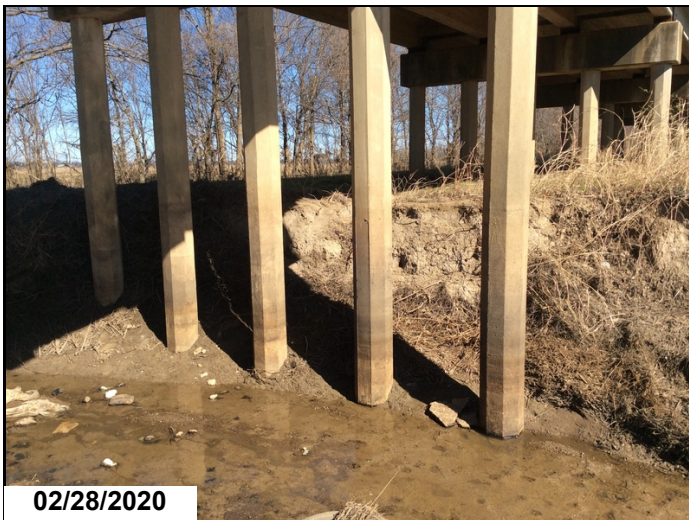
Scour to Piles 1 - 5 @ Bent 3.
