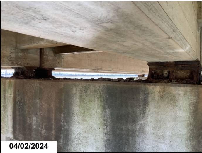
Span 4, Bent 3, Bearings 2 & 3: active corrosion with pack rust.
