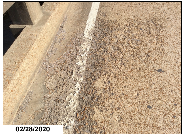
Heavy scaling and spalls to Left Gutter line @ Span 1.
