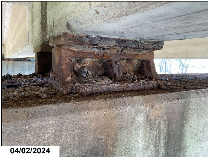
Span 3, Bent 2, Bearings 2 & 3: anchor nuts rusted off.
