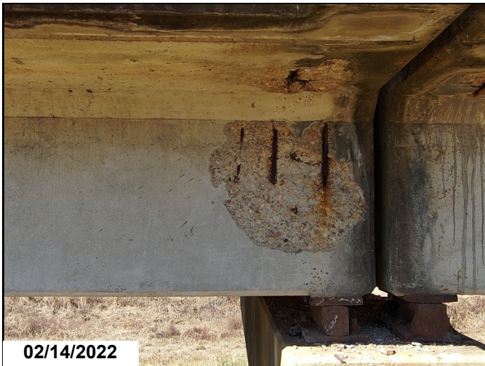
Girders at Spans 1, 2, 4, 7, 8, 9, 10, 11, 12, 13 & 15 Spalls with rebar exposed to girders. Span 7, Girder 4.
