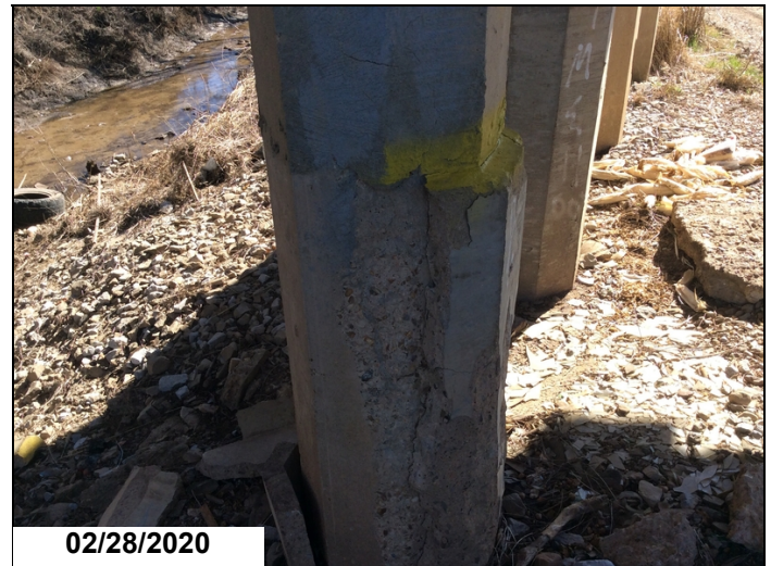
Concrete casing @ Pile 2 Bent 2.
