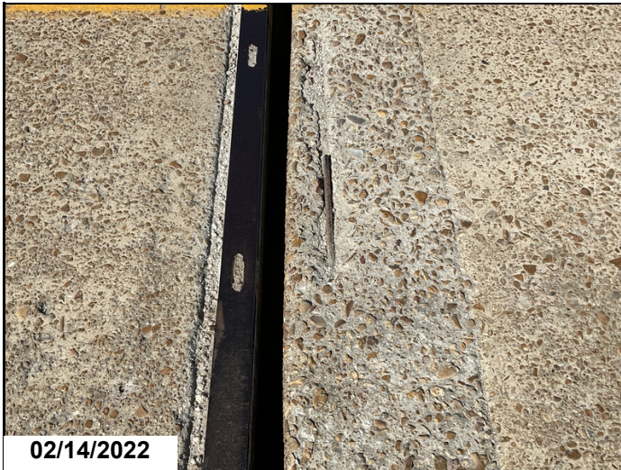
Spall with rebar exposed in Right lane @ beginning of Span 11, end of span 13 & beginning of Span 15. Span 11.
