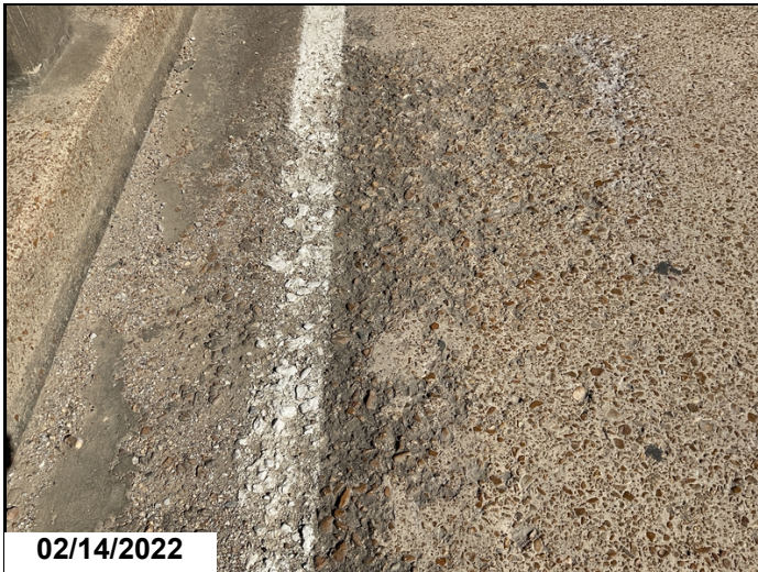
Deck Spans 1, 3, 4, 11, 13, 15, 17 & 18. Areas of Heavy Scaling to Left &/or Right Gutter Lines.
