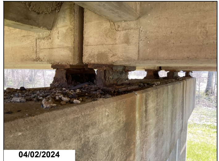
Span 6, Bent 6, Bearings 2 & 3: missing anchor bolts. CS3.
