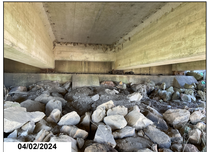
Span 1, Abutment 1, Bearings: active corrosion with pack rust.
