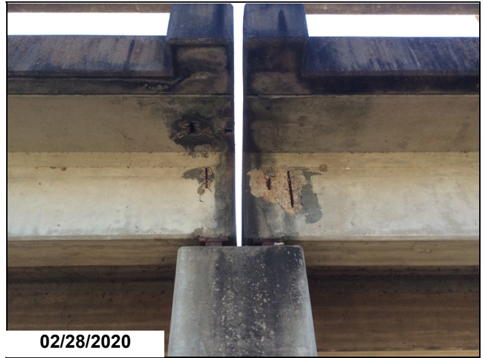
Girder 1 @ end of Span 12 & beginning of Span 13. Spalls with rebar exposed.
