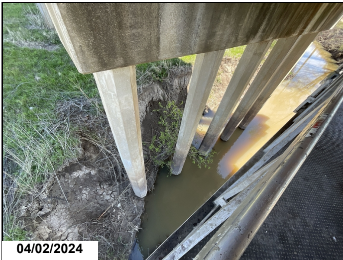
Bent 3, Piles 1 - 5: embankment erosion around all piles causing scour.
