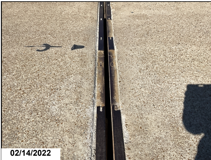
Broken road iron in Right & Left lanes @ Bents 2 & 4. Bent 2.
