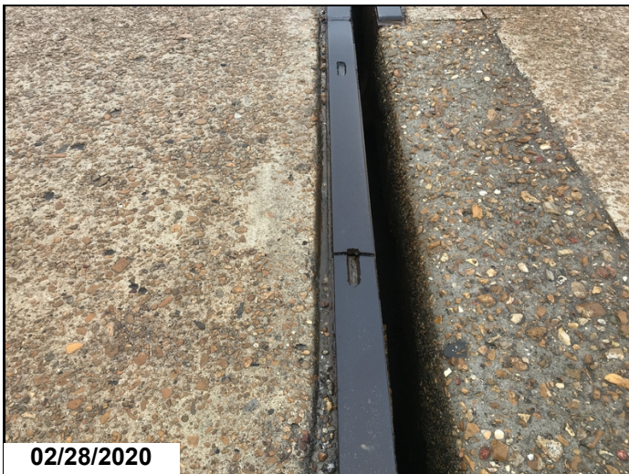
Broken road iron in Right lane @ Bent 4.
