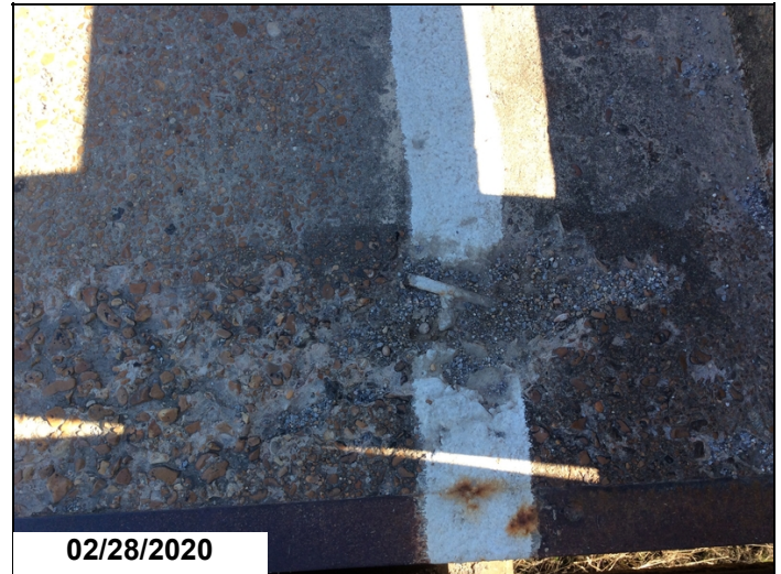
Spall with rebar exposed to Right Gutter line @ beginning of Span 15.
