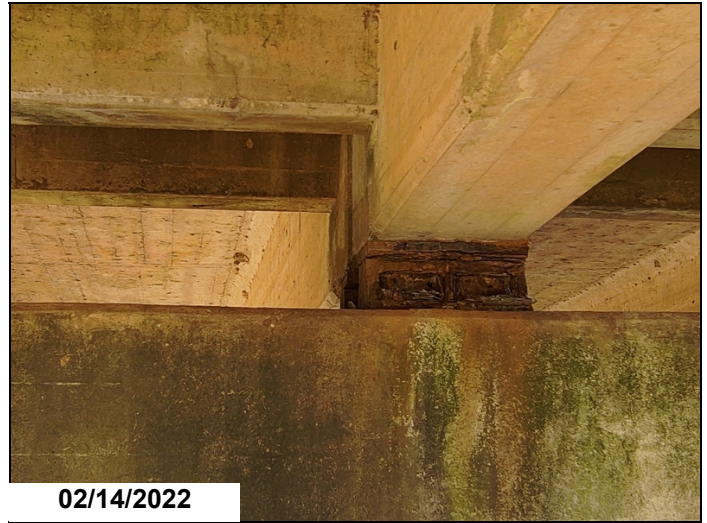
Moveable Bearing Assemblies Corrosion with moderate to severe section loss Typical.
