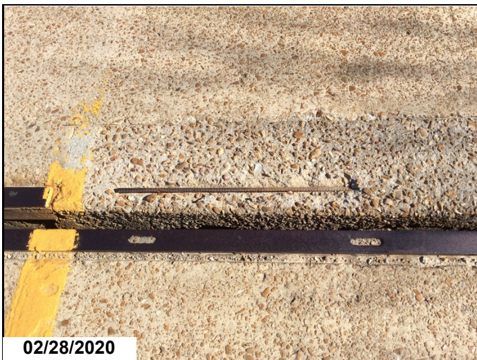
Spall with rebar exposed in Right lane @ Beginning of Span 11.
