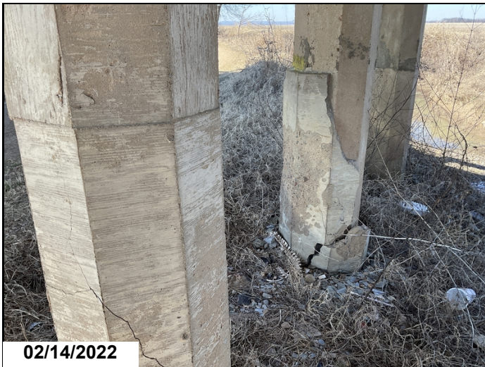
Concrete Pile casing is cracked and spalling @ Piles 2 & 3 @ Bent 2.
