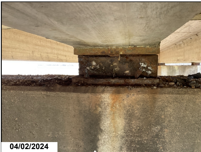
Span 2, Bent 2, Bearings 2 & 3: anchor nuts rusted off. Span 3, Bent 3, Bearings 1 - 3: anchor nuts rusted off.
