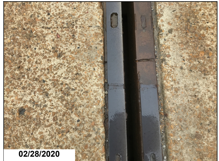
Broken road iron near centerline @ Bent 2.
