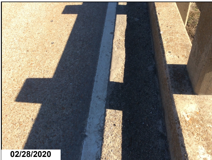
Heavy scaling and Spalls to Right Gutter line @ Span 3.
