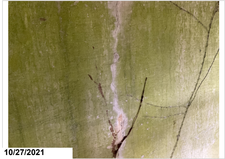
Full height vertical efflor crack @ abutment 2.
