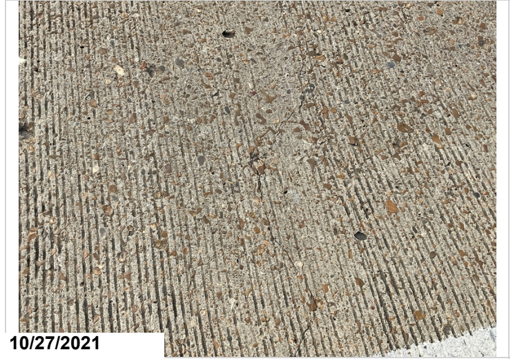
Typical cracks to deck @ all spans.
