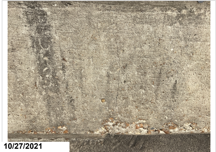
Typical cracks to Lt & Rt parapet wall.
