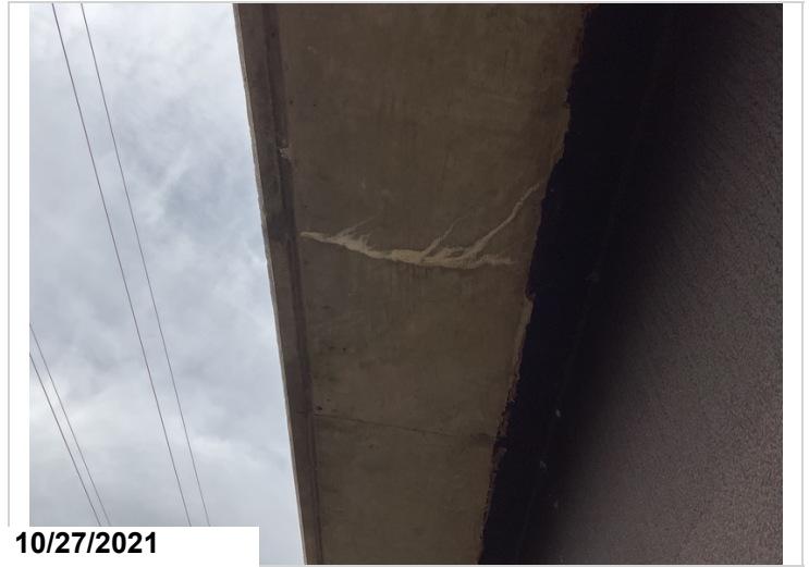
Typical efflor cracks to Lt & Rt overhangs.
