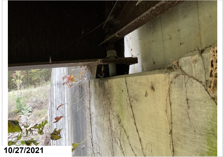
Elastomeric bearings 1-5 @ Abutment 2 are misaligned. Bearing 1.
