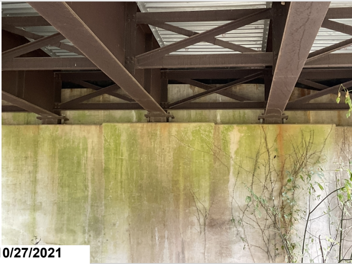
Typical efflor cracks to back wall @ abutment 1.
