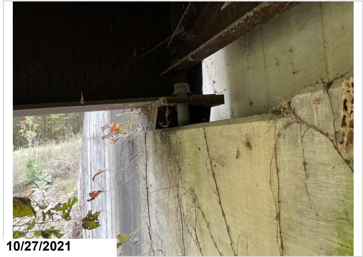
Elastomeric bearings 1-5 @ Abutment 2 are misaligned. Bearing 1.
