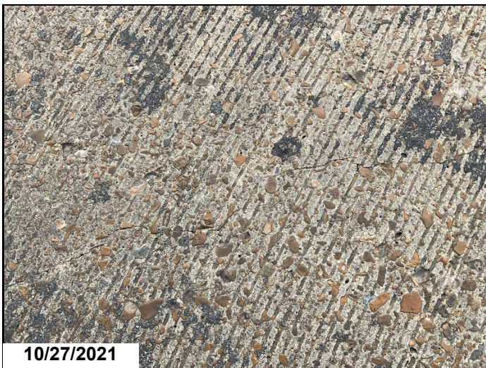
Unsealed transverse cracks to deck @ all Spans.
