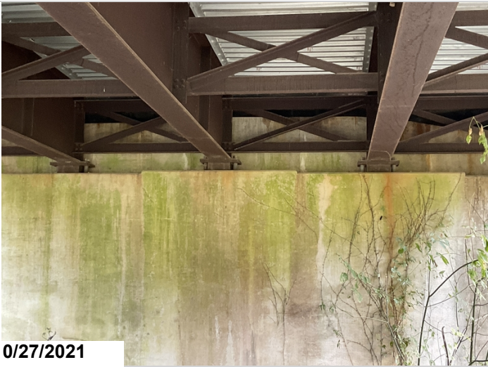
Typical efflor cracks to back wall @ abutment 1.
