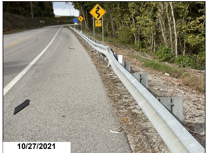
Approach guardrail has minor collision damage at Abutment 2 Left and Right. Lt approach guard rail.
