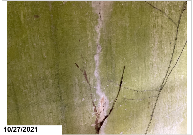
Full height vertical efflor crack @ abutment 2.
