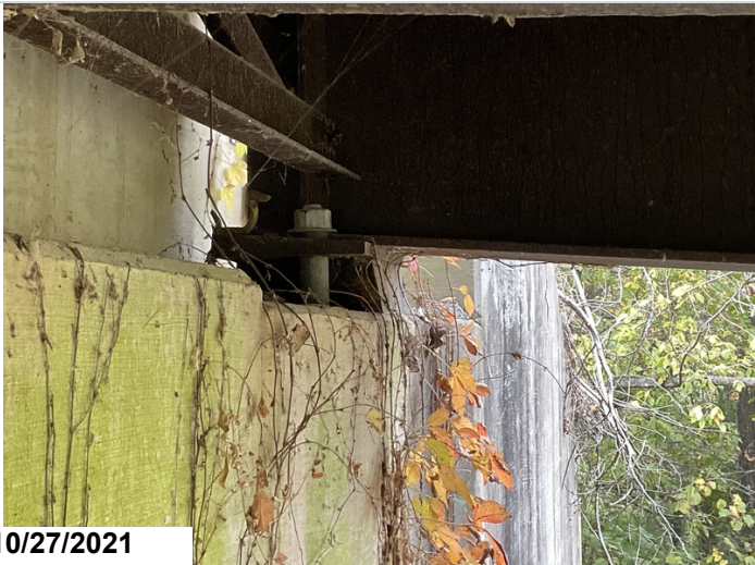
Elastomeric bearings 1-5 @ Abutment 2 are misaligned. Bearing 5.
