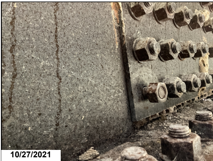
Span 3 - Girder 1 has 1 loose bolt at first splice plate in web.
