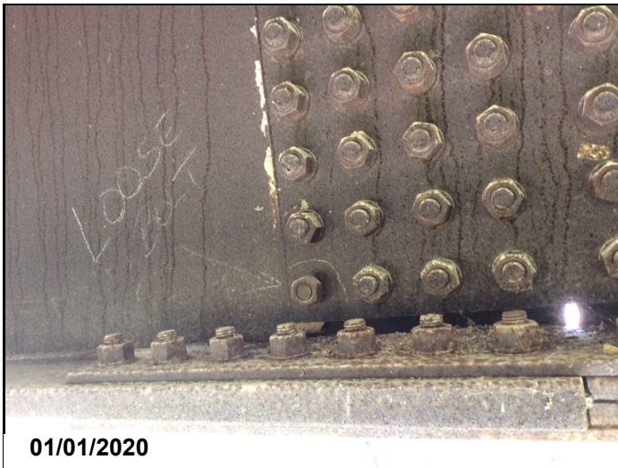
Span 3 has 1 loose bolt at first splice plate in web of Girder 1.
