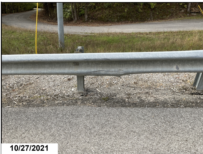
Approach guardrail has minor collision damage at Abutment 2 Left and Right.
