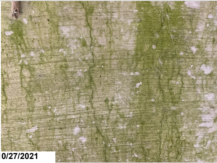
Typical vertical cracks to all caps.
