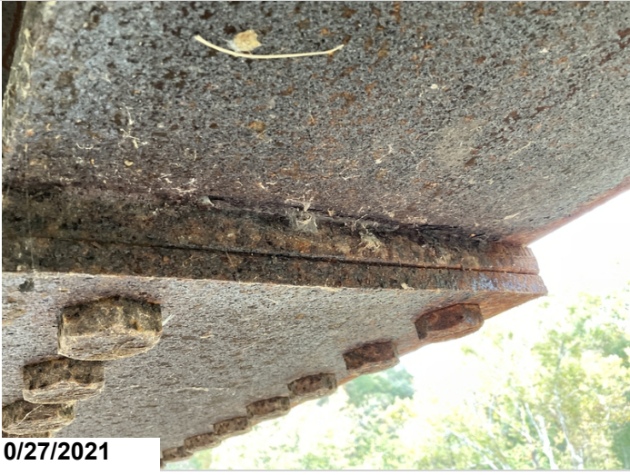
Span 2, girders 1 & 5 has pack rust to first splice plate.
