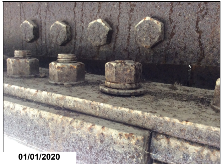
Span 3 has 1 loose bolt at first splice plate in bottom flange of Girder 4
