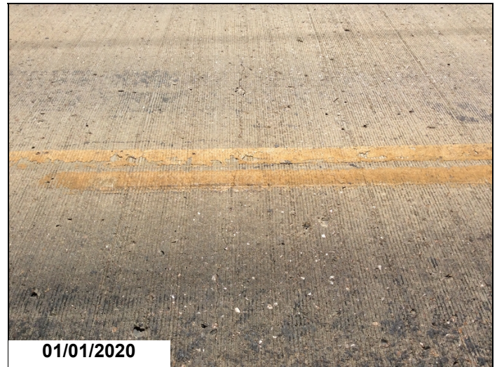
Span 1 Deck cracks.
