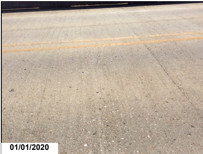
Span 2 Deck cracks.
