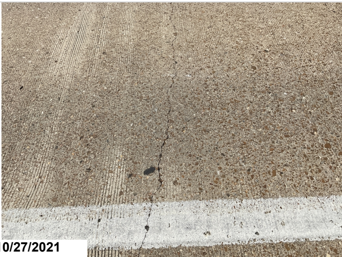
Typical cracks to deck @ all spans.
