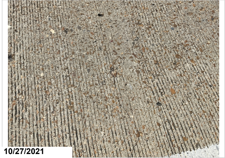
Typical cracks to deck @ all spans.
