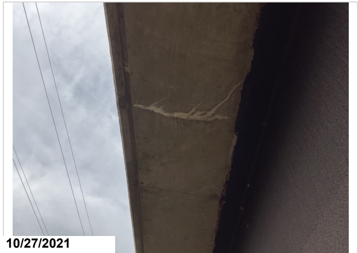
Typical efflor cracks to Lt & Rt overhangs.
