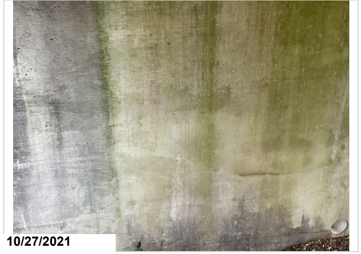
Full height vertical crack @ abutment 1.
