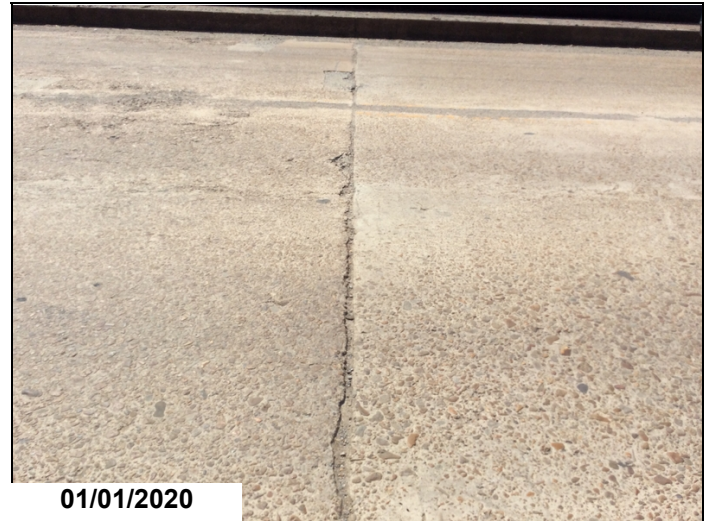
Typical poured joint.
