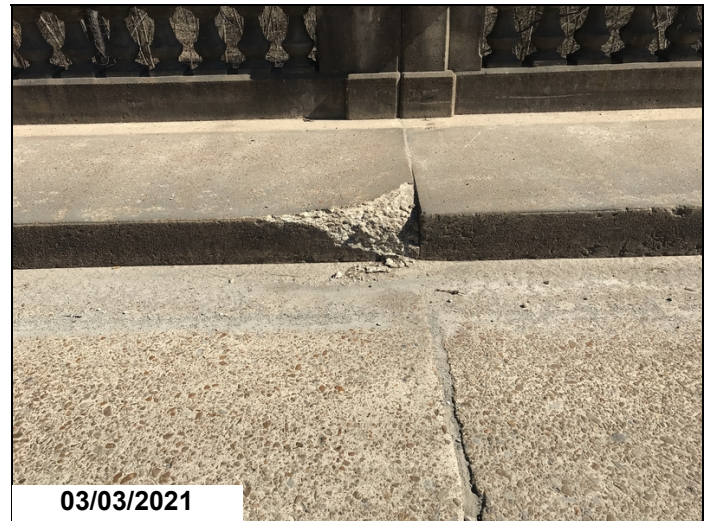
Spalls and deterioration to curbs / sidewalks.
