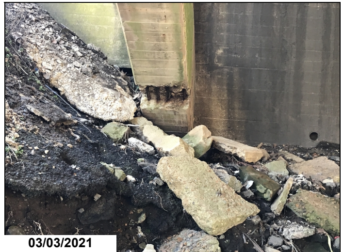
Span 5 - Arch rib 1 has large spall with 5' of rebar exposed at end of span.
