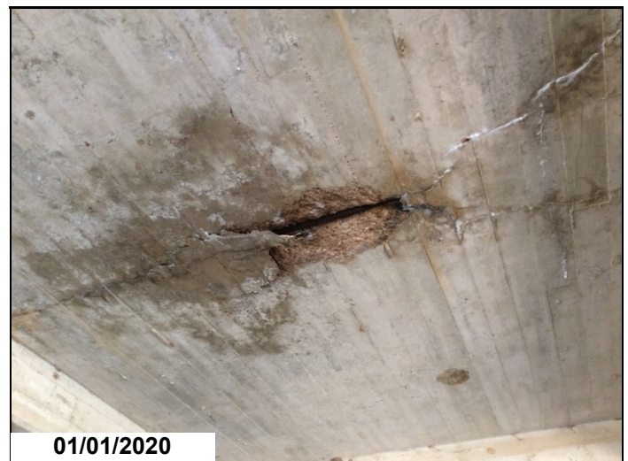
Spall with exposed rebar to soffit between Arch Rib 2 & 3 near end of Span 5.
