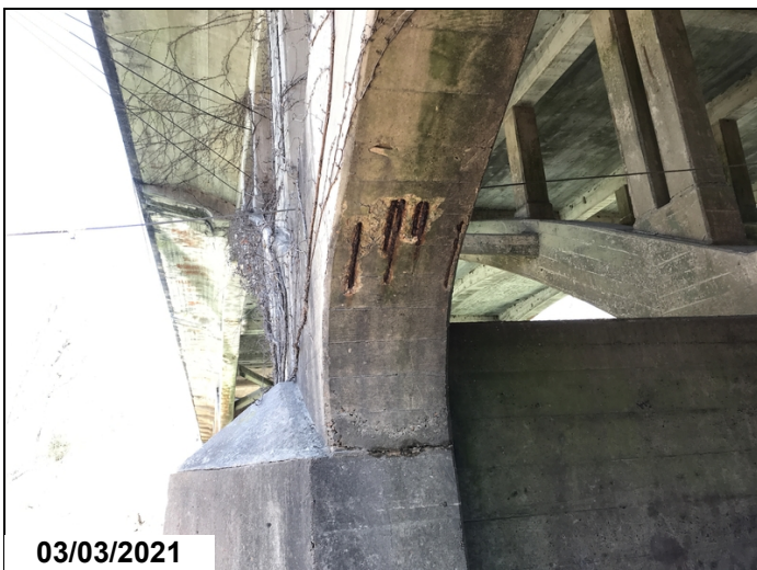
Span 5 - Arch Rib 4 has spall with 4' of rebar exposed at beginning of span.
