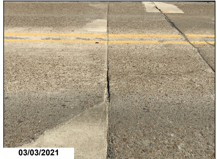
Poured joint seals are deteriorated, filled with debris and drain openings are plugged.
