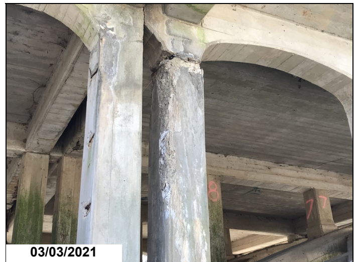
Cracked and delaminated areas, and spalls with rebar exposed to spandrel columns at all spans.
