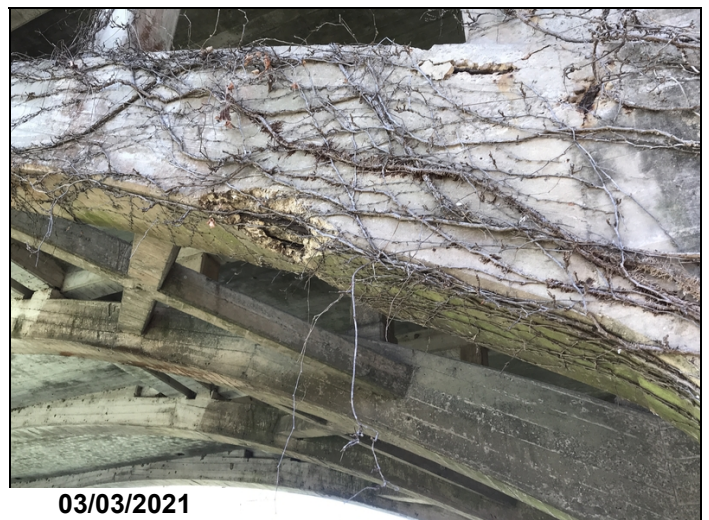
Span 4 - Arch rib 4 has spall with 5' of rebar exposed at end of span.
