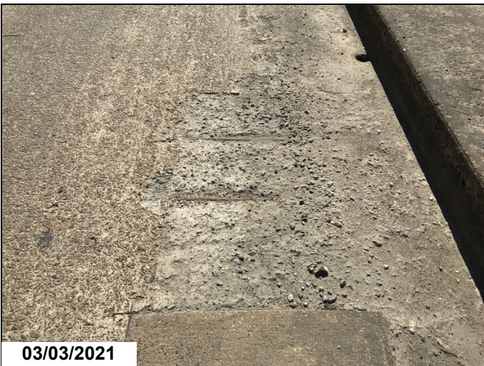
Spalls with rebar exposed to deck at Span 3 & 4 Span 3.
