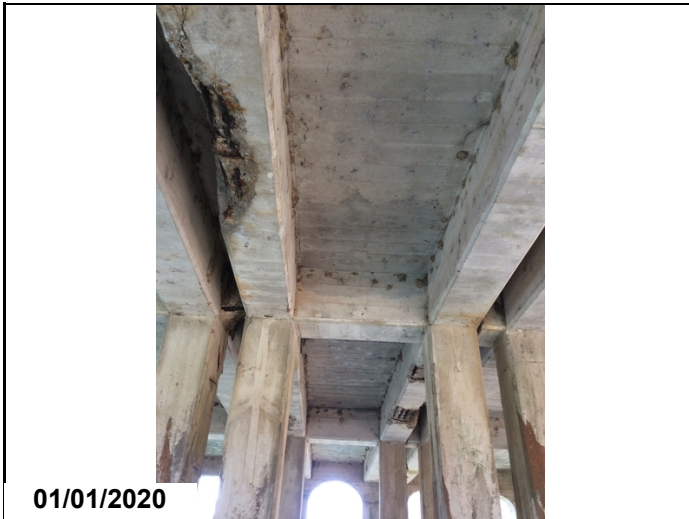
Concrete Diaphragms at Bent 3
