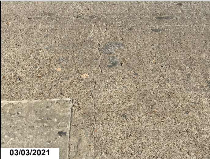
Unsealed cracks, areas of scaling, and spalls to deck at all spans.
