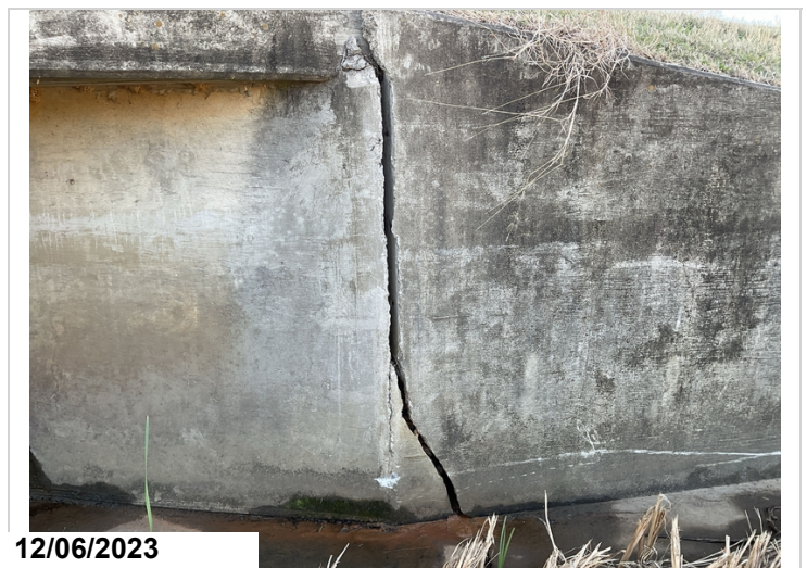
Crack & minor rotation to Left wing @ Abutment 1
