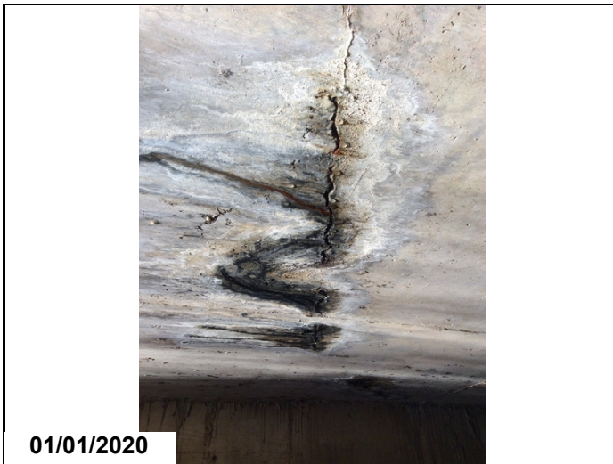
01/01/2020 Barrel 3 a has 1/4" wide Rust Stained longitudinal crack to Deck below near Outlet end.
