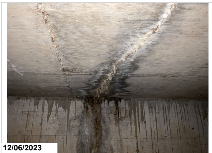
Typical #3 efflor cracks to soffit @ all barrels.
