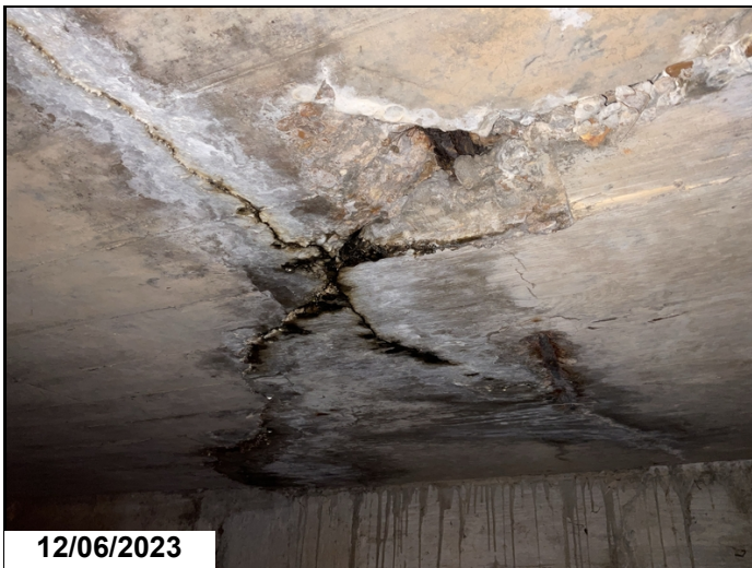
01/01/2020 Barrel 3 a has 1/4" wide Rust Stained longitudinal crack to Deck below near Outlet end.
