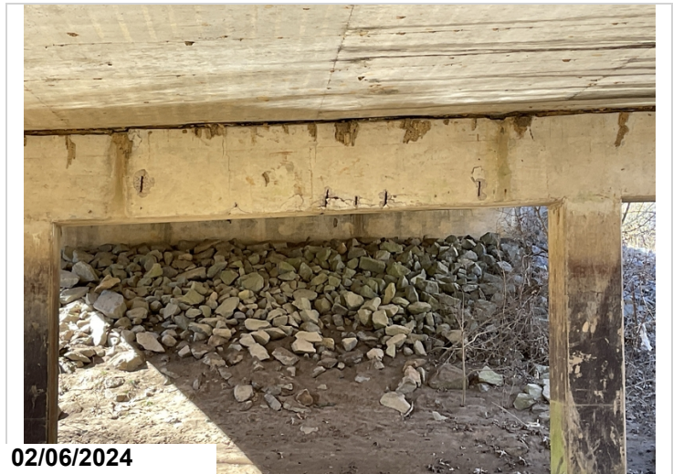
Spalls with rebar exposed with section loss to backside of cap @ Bent 2.
