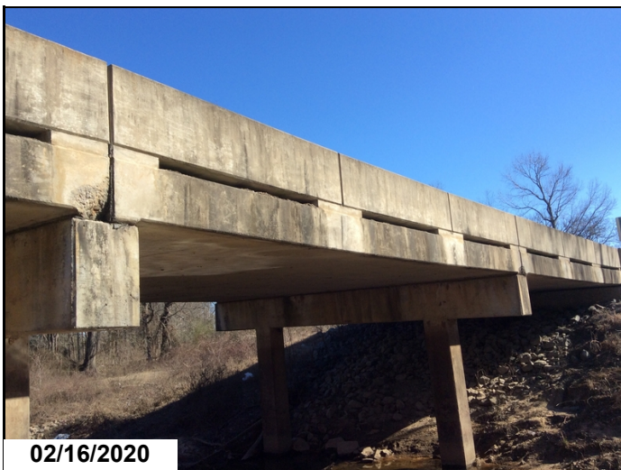
Typical spall to outside edge of deck @ Bent 1 & 2.
