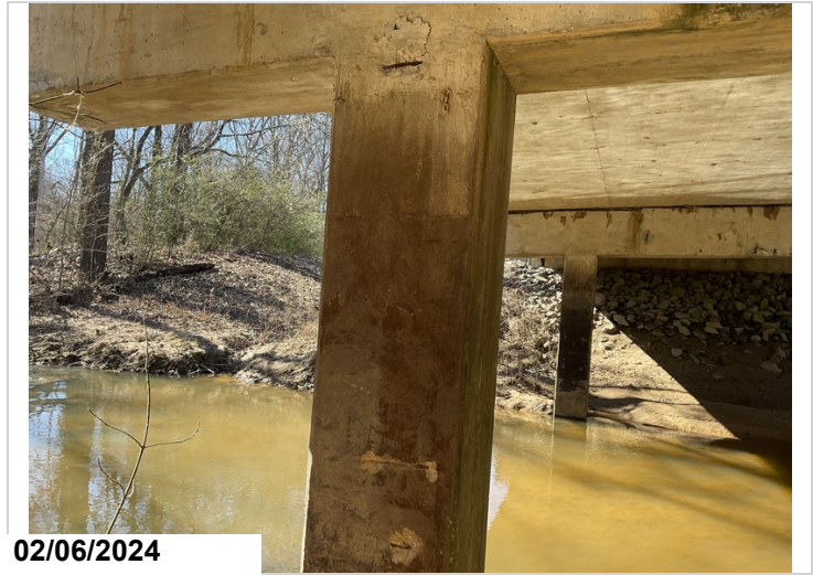
Spalls with rebar exposed to column 1 @ bent 1.
