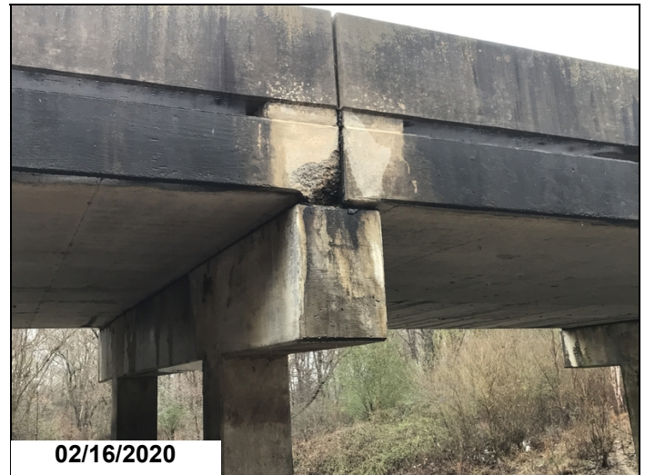
Cracks & spalls to left & right outside edge of deck over Bent 1 & to right edge over Bent 2
