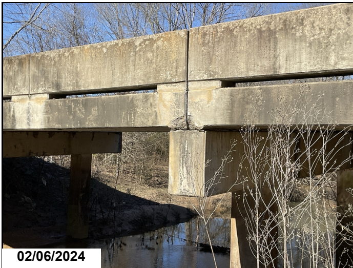
Cracks & spalls to left & right outside edge of deck over Bent 1 & to right edge over Bent 2 Lt side of bent 1.
