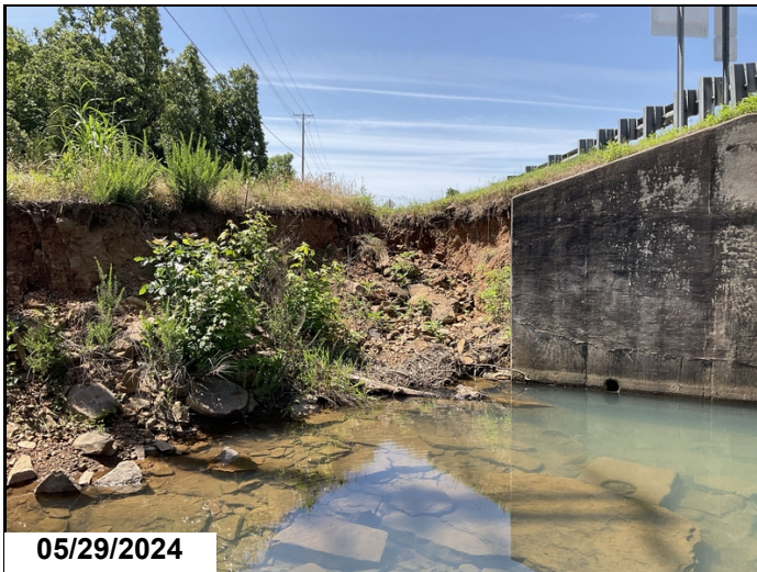
Erosion to embankment & behind Right wing at Abutment 1. Scour along footing and Right end of Abutment 1.
