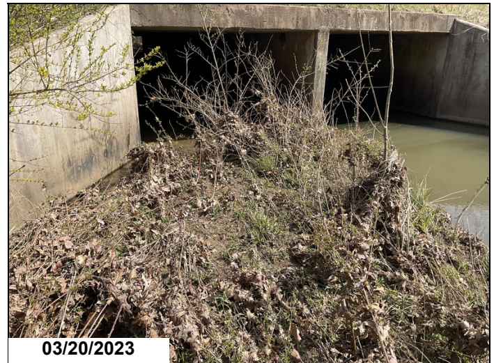
Sediment buildup & vegetation is restricting flow in channel at inlet and outlet ends of Barrel 1
