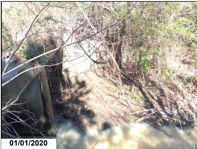
Sediment @ trees restricting flow @ outlet end of Barrel 1.
