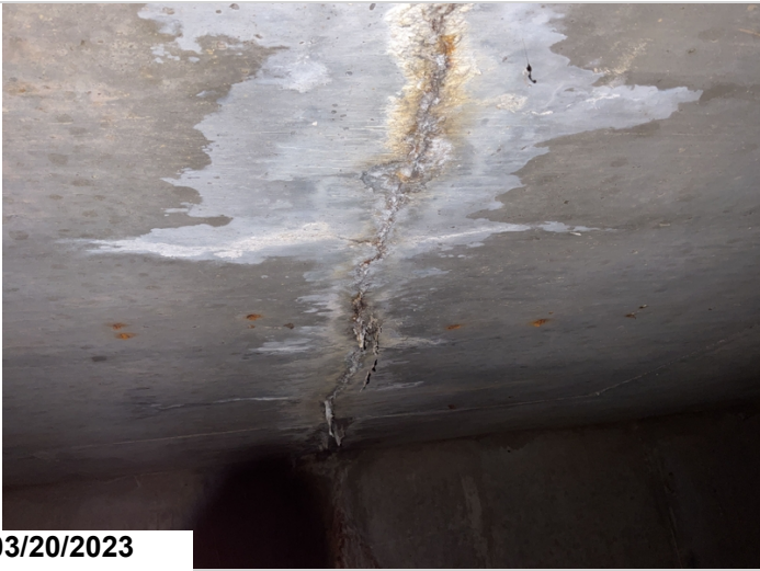
Efflor cracks with rust stain @ barrel 1.
