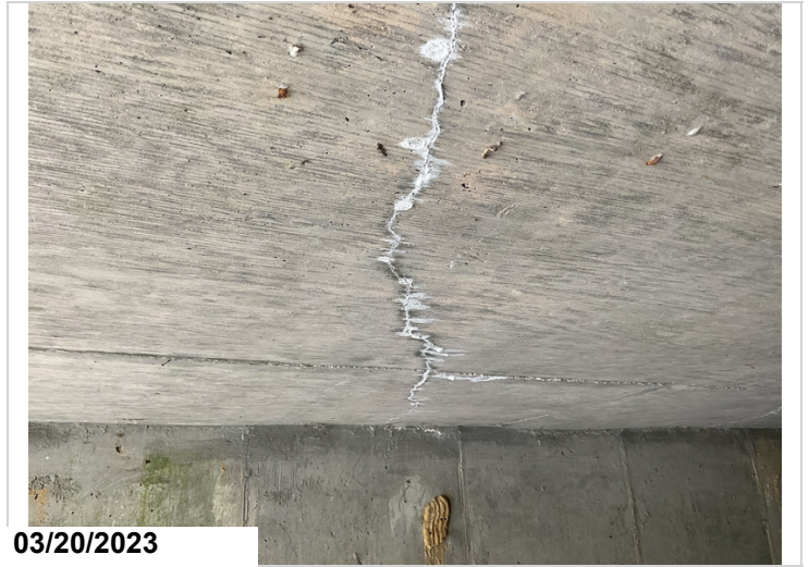
Typical efflor cracks to barrels 1 & 2.
