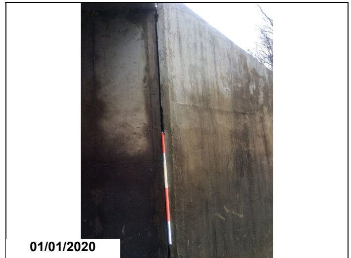
Right & left wings at Abutments #1 & #2 have separated
