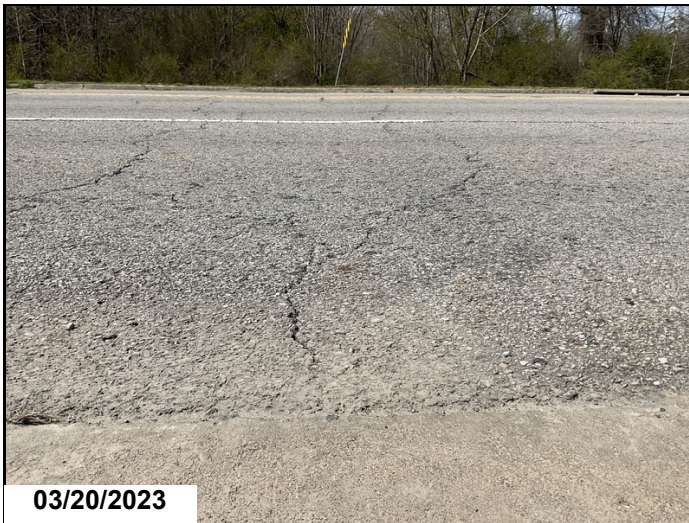
Visible settlement to approach roadways Abutment 2.
