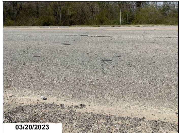
Visible settlement to approach roadways Abutment 1.
