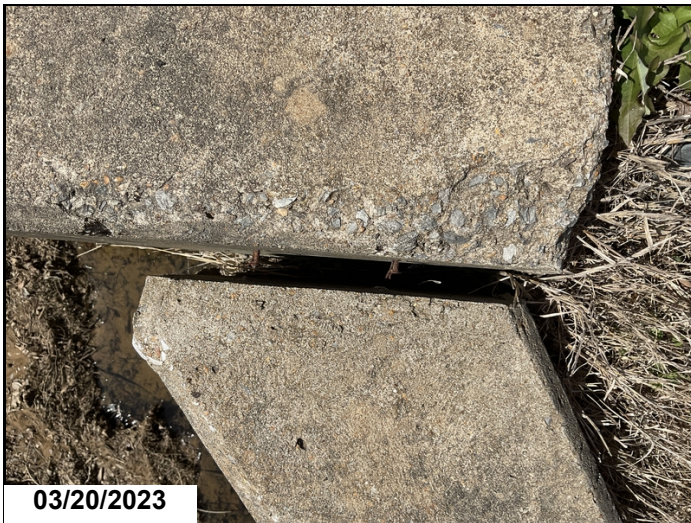
Left & Right wings at Abutments 1 & 2 have separated.
