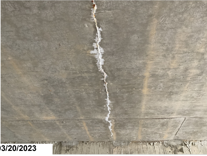
Typical efflor cracks to @ barrels. Barrel 3.
