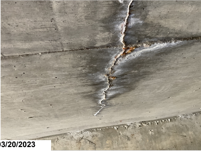
Few efflor cracks with rust to all barrels. Barrel 3.
