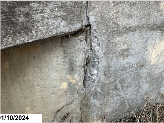
Spall with rebar exposed to Lt side of abutment 1.
