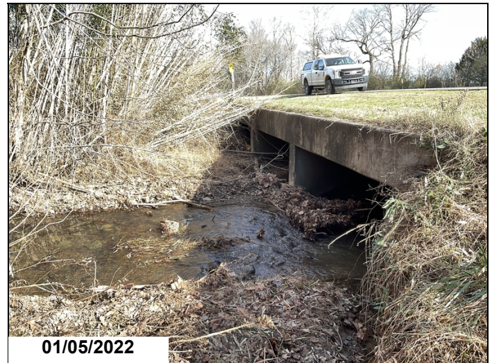
Sediment & vegetation buildup on Right side.
