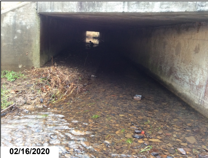
Minor sediment in Barrel 3.
