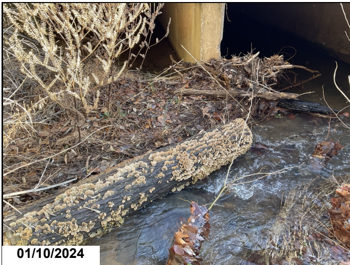
Drift buildup @ barrels 1-3.
