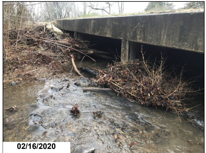
Heavy drift buildup @ barrels 1-3.
