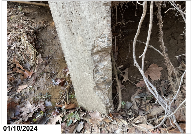
Spalls to Left end of Walls 1 & 2.(#3)(Wall 1)
