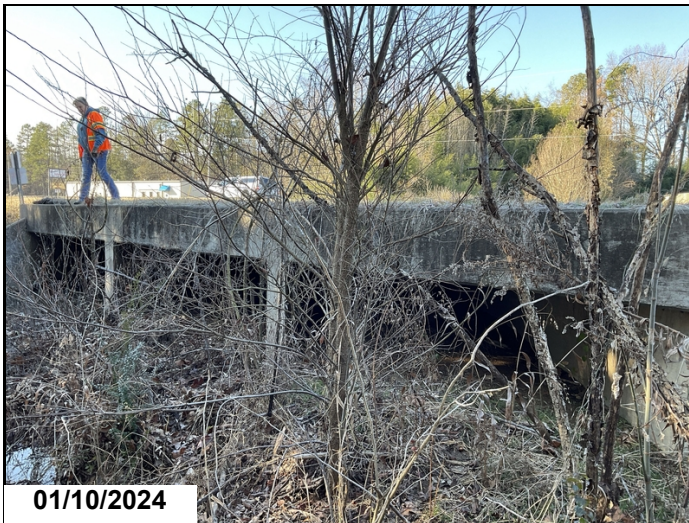
Sediment & vegetation buildup to Right & Left side.
