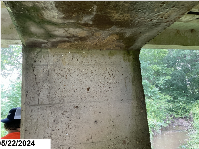
Vertical crack to Lt side of column 2 @ bent 2.
