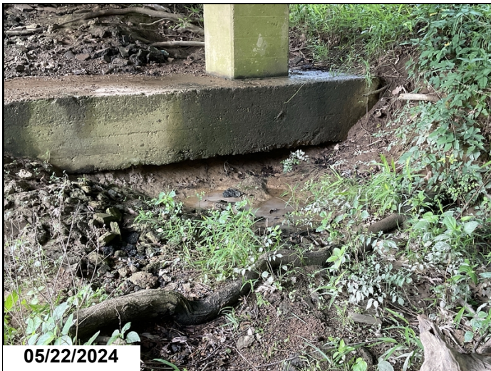
Scoured below bottom and back under footings @ Bents 1, 4 & 5. Bent 5
