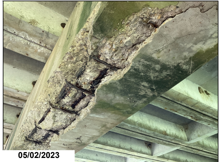
Bent 4 - Areas of delamination & spalls with 13.5' rebar exposed.
