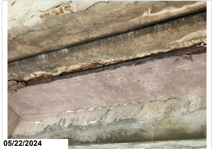
Spall with rebar exposed with 2' of rebar not adhered to unit 4, span 3.
