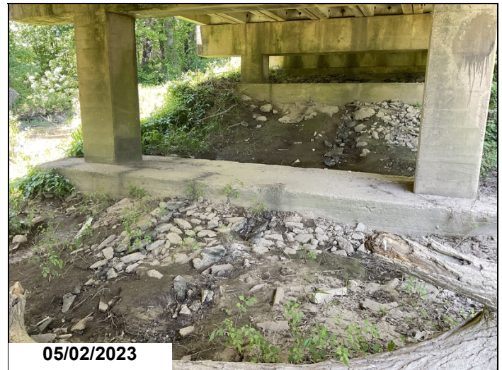
Scour with Footings exposed at Bents 2, 3, & 6. Bent 2.
