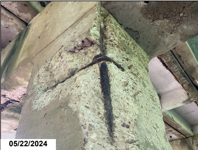
Bent 4 - Column 2 has large deep spalls with 6' of rebar exposed.
