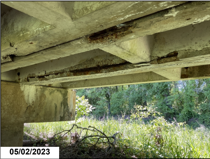
Longitudinal cracking with rebar exposed to Girders at all SpansUnit 6, span 6.
