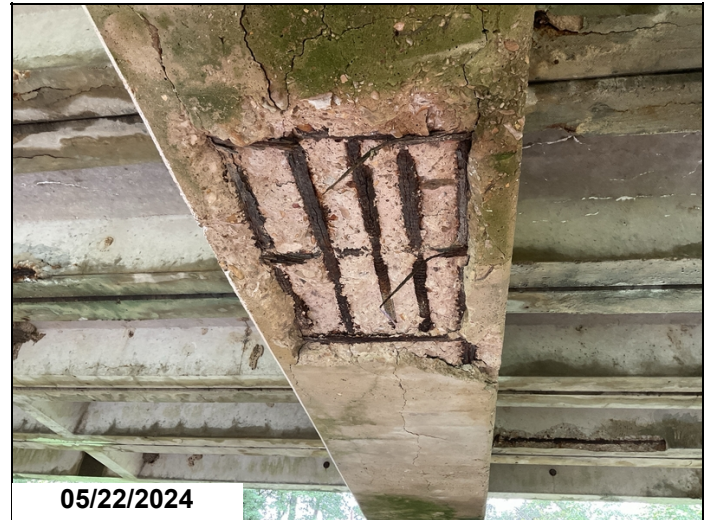
05/22/2024 Bent 3 - Heavy cracking, areas of delaminating & spalls with 8' rebar exposed.
