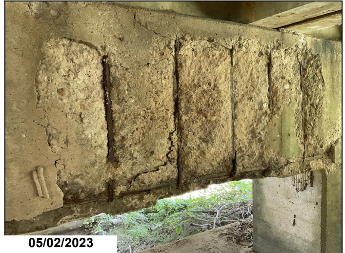
Bent 1 - Horizontal cracks & spalls with 10' rebar exposed.
