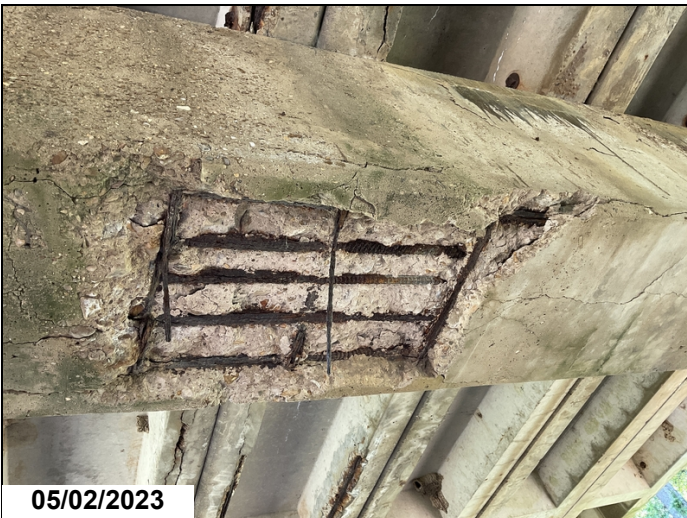
Bent 3 - Heavy cracking, areas of delaminating & spalls with 10' rebar exposed.
