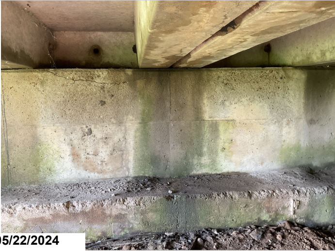
15' of horizontal crack to Abutment 2.
