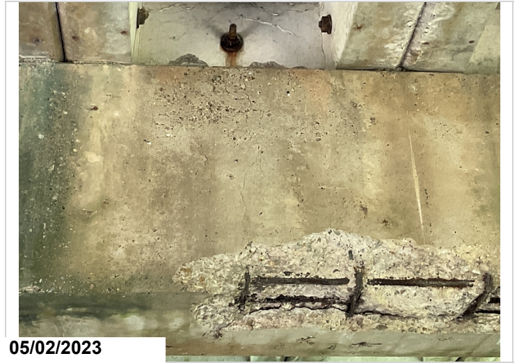
Vertical crack to backside of cap near centerline @ bent 4.
