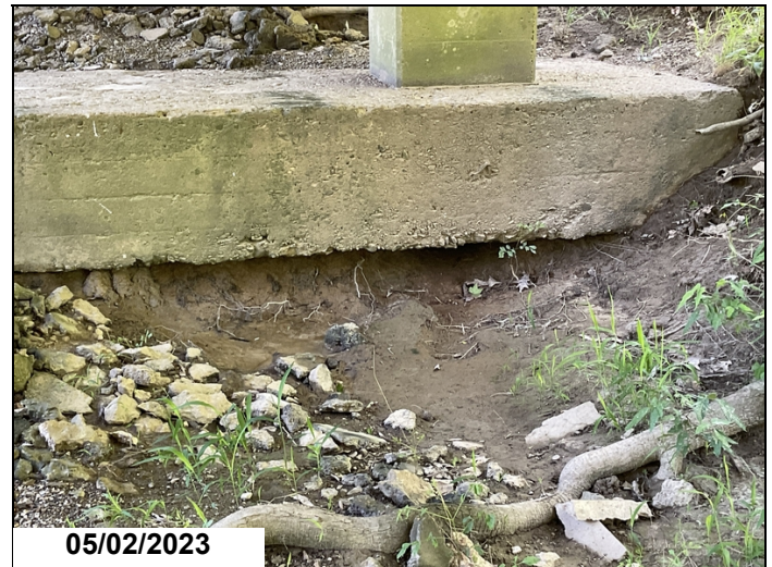
Scoured below bottom and back under footings @ Bents 1, 4 & 5. Rt side of bent 5.
