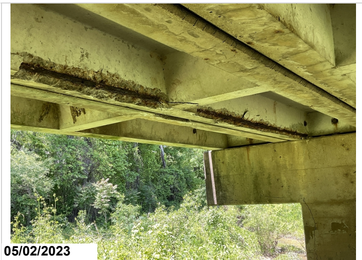
Typical spalls with rebar exposed to girders @ all spans.
