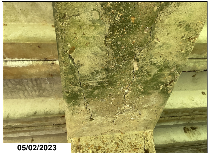
Horizontal cracks to rt side of cap near large spall.
