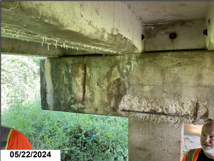
Bent 5 - Large areas of delamination & spalls to ahead side of cap with 5' of rebar exposed.
