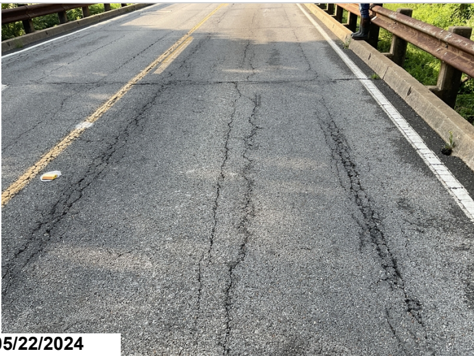
Typical cracks to wearing surface
