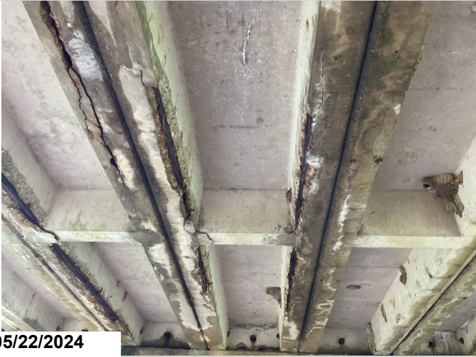
Typical spalls with rebar exposed to units @ all spans
