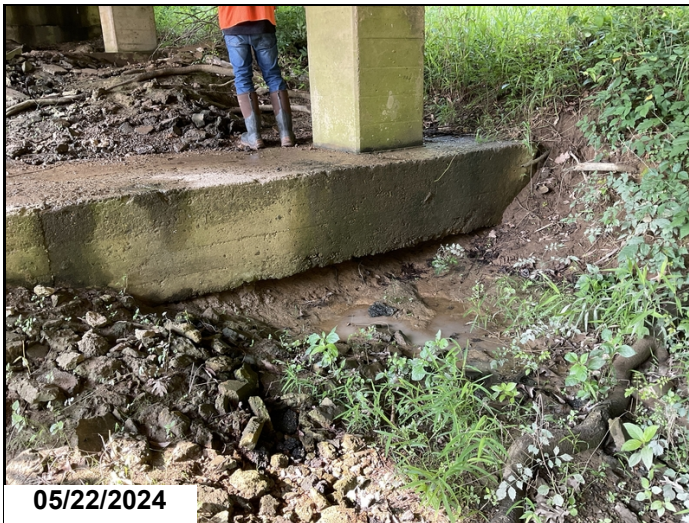
Scour with Footings exposed at Bents 1 - 6 Bent 5
