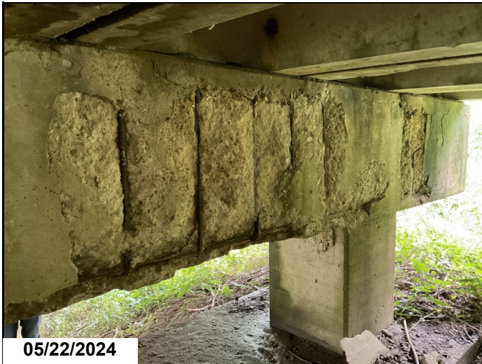
05/22/2024 Bent 1 - Horizontal cracks & spalls with 10' rebar exposed.
