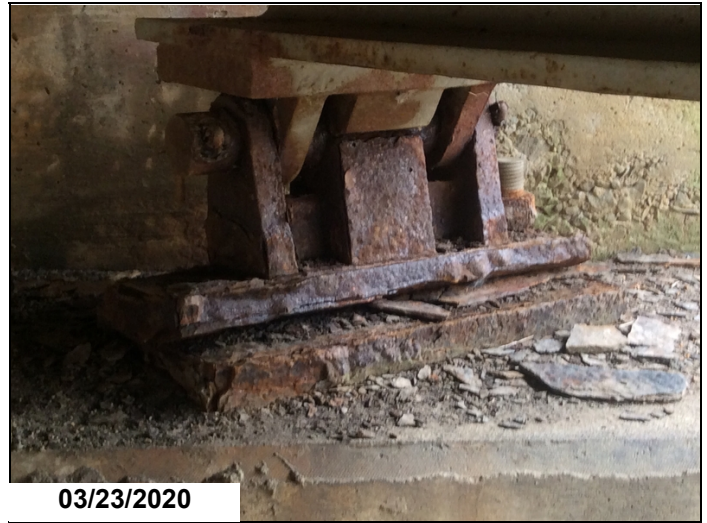
Rust, corrosion & flaking to moveable bearings at Abutments 1 & 2.
