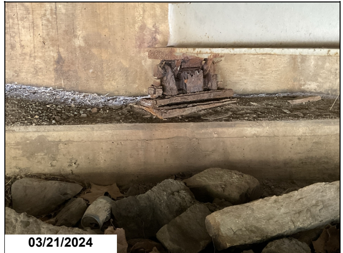
Rust, corrosion & flaking to moveable bearings at Abutments 1 & 2. Abutment 1, bearing 2.
