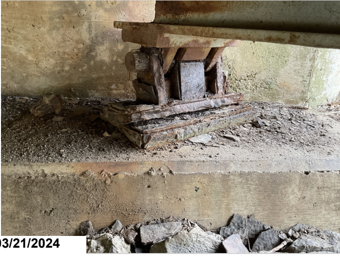
Typical (#3) rust & pack rust to Moveable Bearings. Girder 1, Abutment 1.
