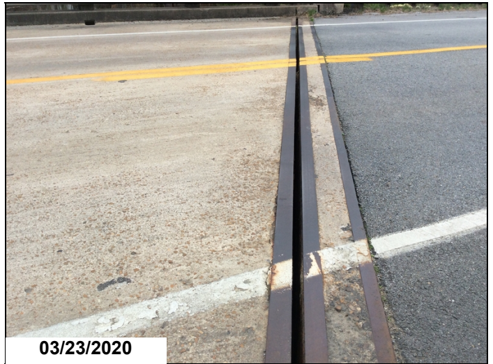
44' of compression joint seal has lost adhesion & is missing @ Abutment 2.
