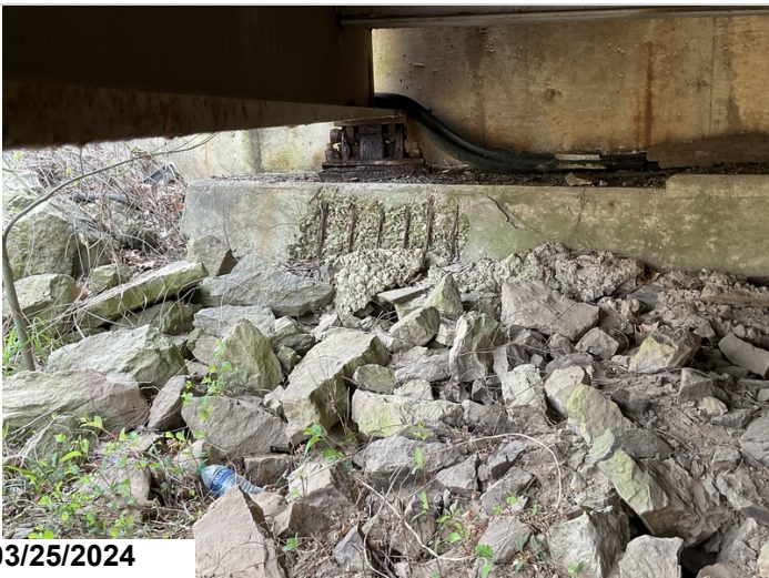
3' Spall with 6' of (#3) rebar exposed to Abutment 2 on Left end.(#3)
