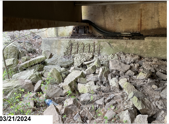
3' Spall with 6' of (#3) rebar exposed to Abutment 2 on Left end.(#3)
