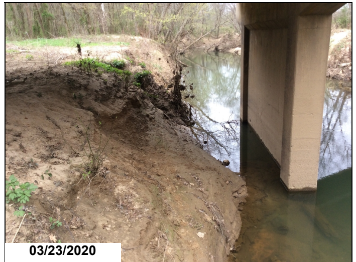
Moderate scour @ Bent 2 & to embankment @ Span 3.
