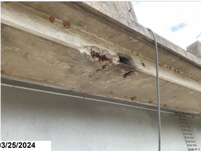
Span 2 - Spall to soffit with 2' rebar exposed near 1st drain on Right.
