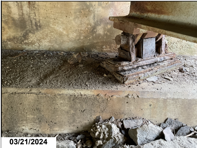
Anchor bolt missing to Bearing Assembly 1 at Abutment 1.
