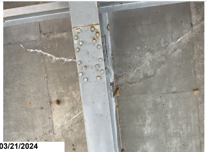
Typical efflorescence cracks to undersurface @ span 2.
