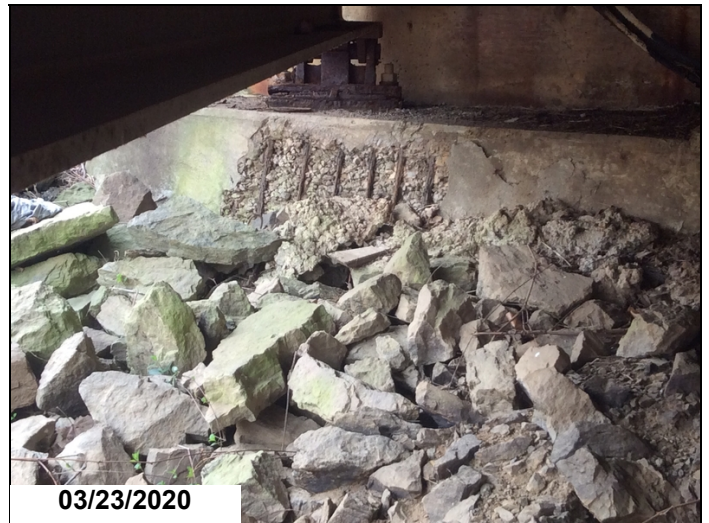
Spall with 6' rebar exposed to left end of Abutment 2.
