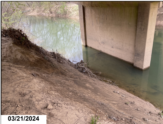
Moderate scour @ Bent 2 & to embankment @ Span 3.
