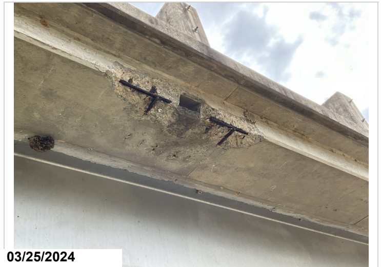
Span 1 has spall with 2' rebar exposed to soffit @ 2nd drain opening on Right.
