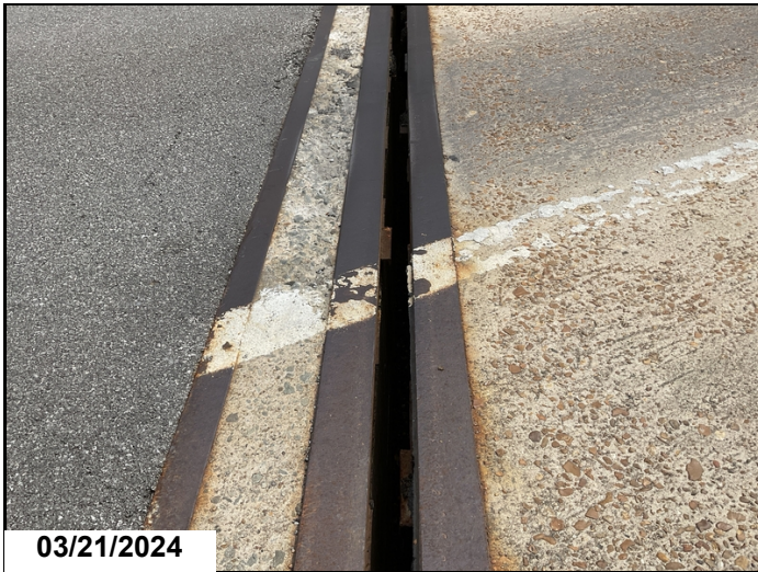
31' of compression joint seal has lost adhesion & is missing @ Abutment 1.
