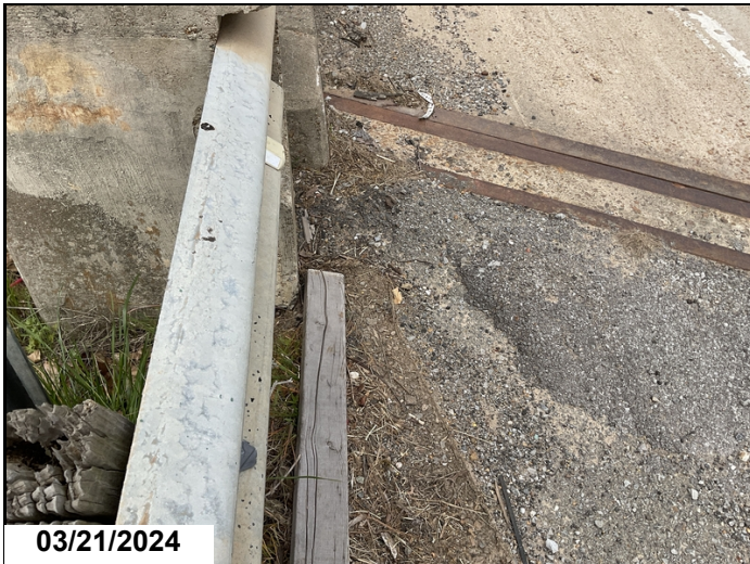
Eroded area 1' deep @ roadway & ±4' long under Right approach at Abutment 2. Repaired
