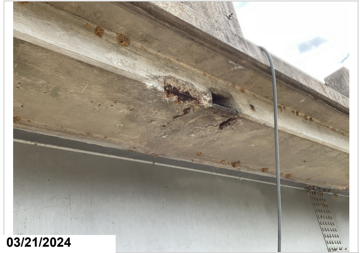
Span 2 - Spall to soffit with 2' rebar exposed near 1st drain on Right.
