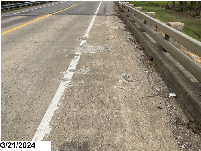
Spalls to deck @ span 1.
