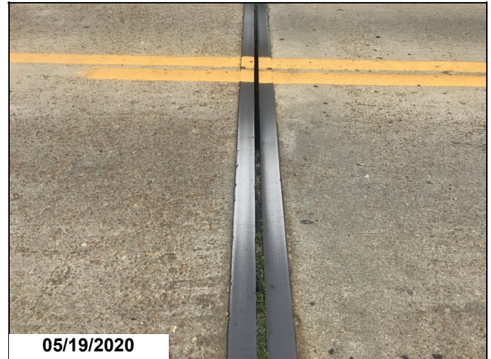
All Compression Joint Seals cracked, deteriorated & leak. Bent 1 - 6' Joint seal has failed. Bent 4 - 8' Joint seal has failed.
