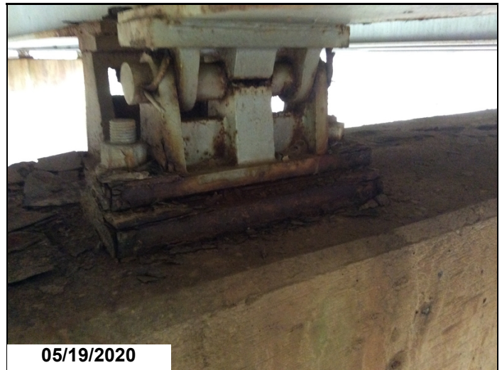
Rust/pack rust & section loss to moveable Bearing Assembly at all Spans.
