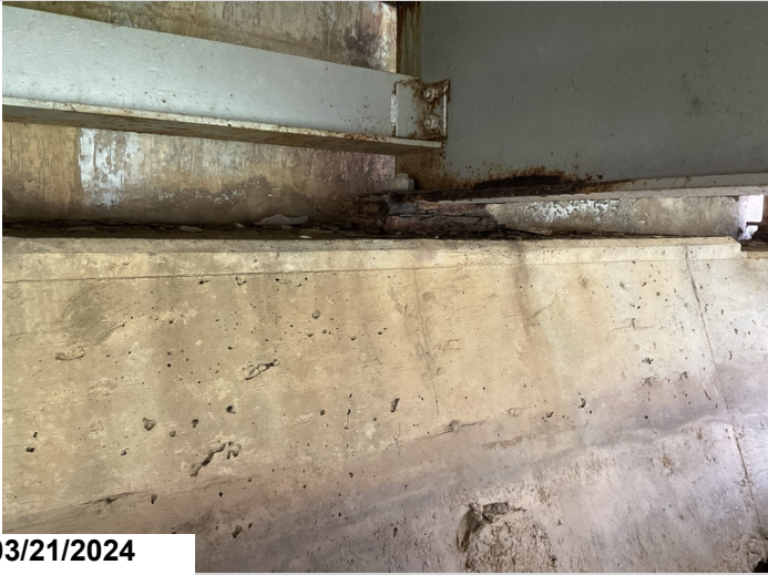
Typical (#3) corrosion to bearings 1 - 5 @ abutment 1.
