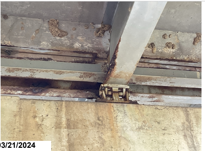
Typical corrosion to girders @ end of spans. Girder 5, end of span 2.
