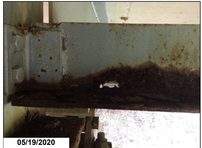
Holes in Diaphragm at Beginning of Span 2 between Girders 2 - 4. Beginning of Span 3 between Girders 2 & 3.
