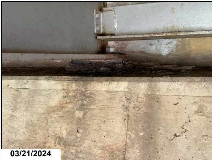
Rust/pack rust & section loss to moveable Bearing Assemblies at all Spans. Typical rust to bearings 1 - 5 @ abutment 1.
