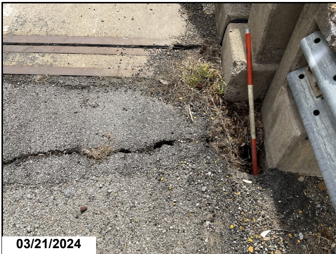
1'x1'x2' down Erosion to edge of roadway to Rt end of abutment 1.
