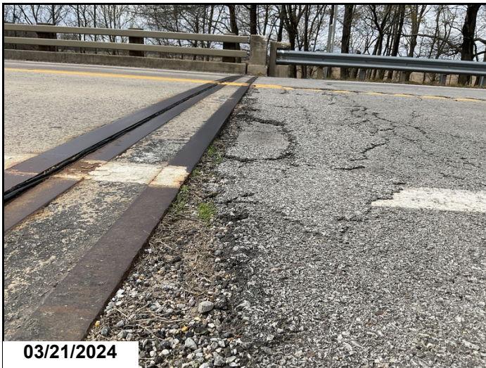
Visible settlement to Roadway at Abutment 1 & 2.
