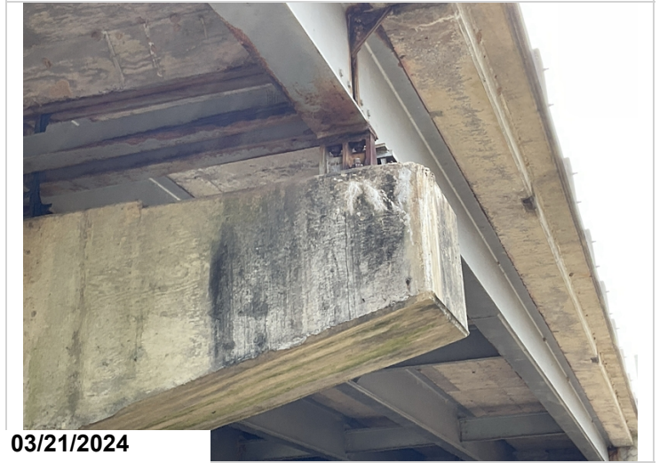
Efflor cracks to Rt ahead side of cap @ bent 1.
