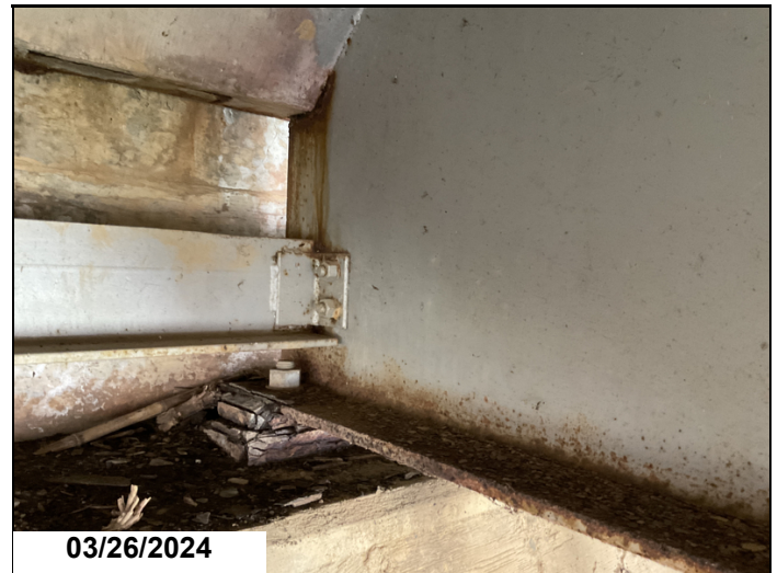
03/26/2024 Rust with s/l to web below haunch @ Girder 3 @ Abutment 1.(#3,
