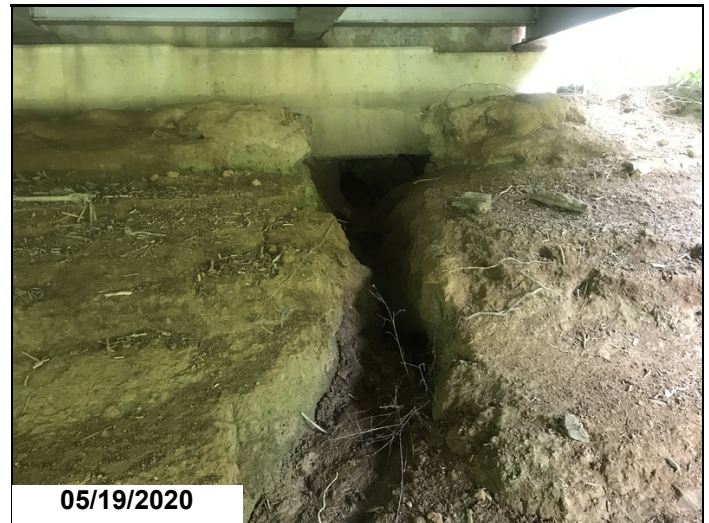
Erosion to slope at Abutment 1.
