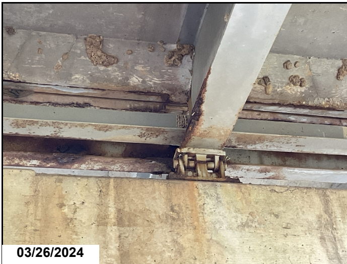
03/26/2024 Typical corrosion to girders @ end of spans. Girder 5, end of span 2.
