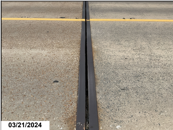
Bent 1 - 22' Joint seal has failed.
