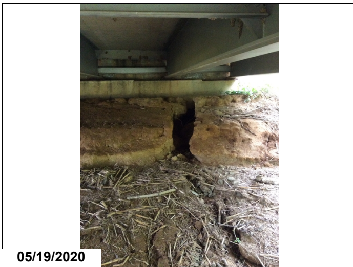
Erosion to slope at Abutment 1.
