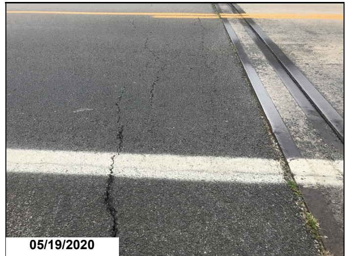
Visible settlement to Roadway at Abutment 1 & 2.
