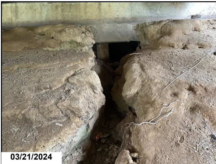
Erosion to slope at Abutment 1.
