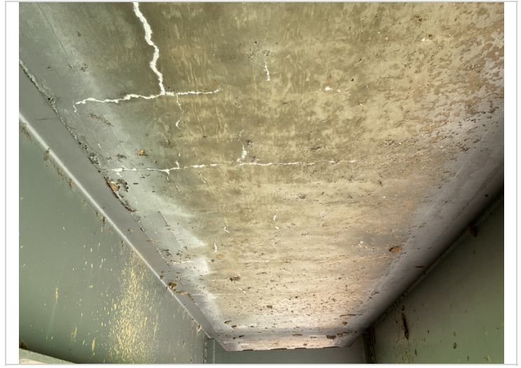
Efflorescent cracking to soffit @ Span 1.(#2 typical)
