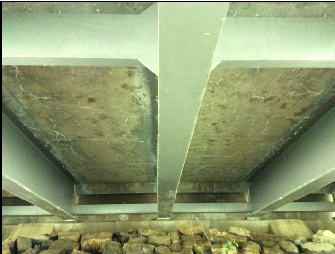
Efflorescent cracking to deck below.
