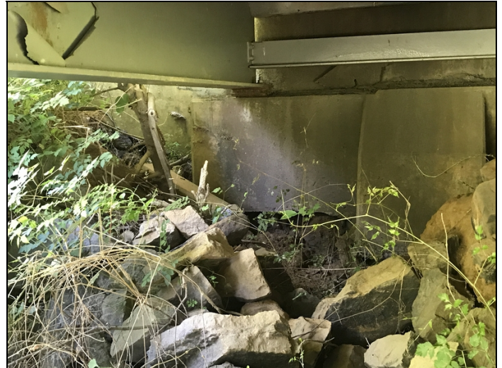
Embankment has settled to left end of Abutment 2.
