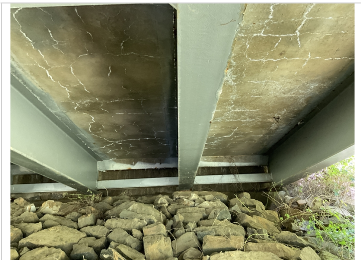
Efflorescent map cracking to soffit @ Span 3.(#3)
