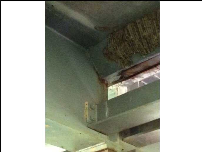
Existing pitting & section loss to webs of girders at all spans.
