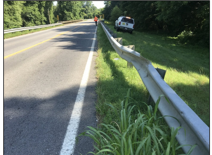
Approach guard rail damage on Right at Abutment 1.
