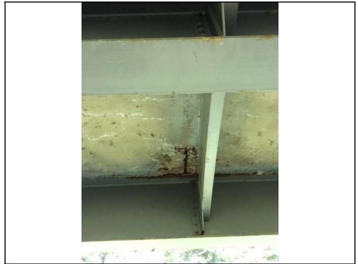
Spall with 1.5' of rebar exposed to deck below between Girders 4 & 5 at Span 3.
