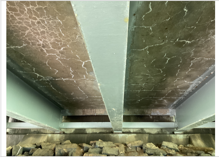
Efflorescent map cracking to soffit @ Span 1.(#3)
