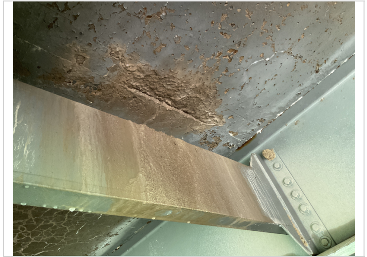
Spall to soffit between Girders 3 & 4 @ Span 1.(#3)
