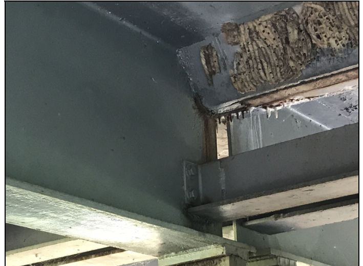
Existing pitting & section loss to webs of girders below paving haunch at all spans.
