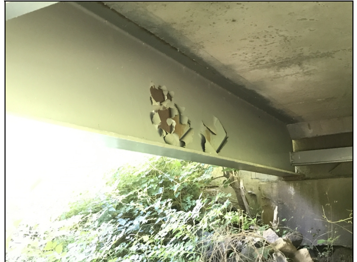
Areas of peeling paint to Girders 1 & 2 at Span 3.
