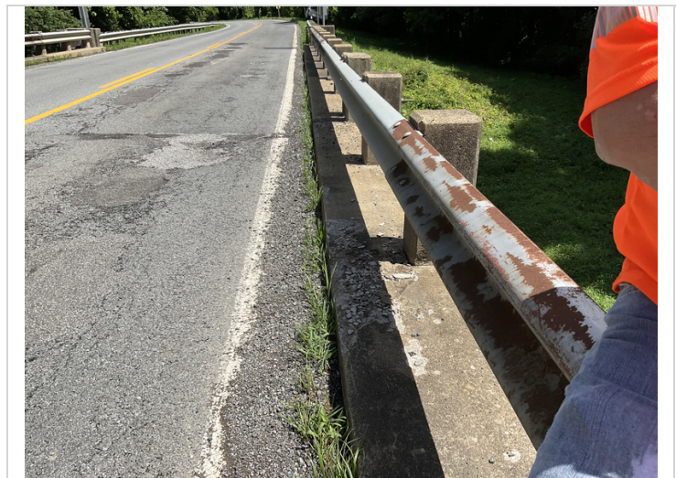
Deterioration & spalling to Right curb Spans 2 & 3.
