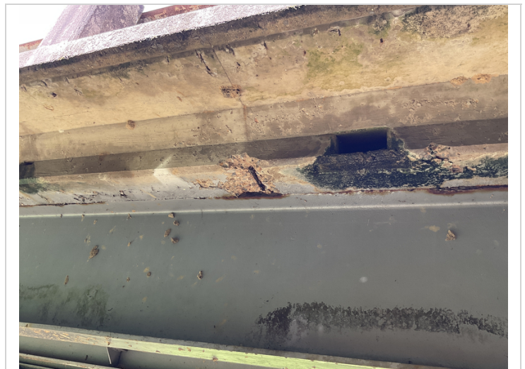
Spall with rebar exposed with s/l to Right overhang @ Span 1.
