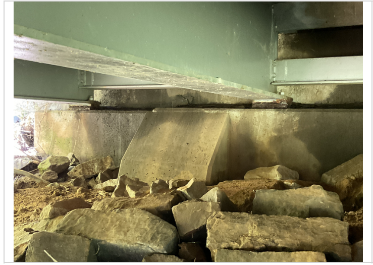
Rust with pack rust to Fixed Bearings @ Abutment 1.(#3)
