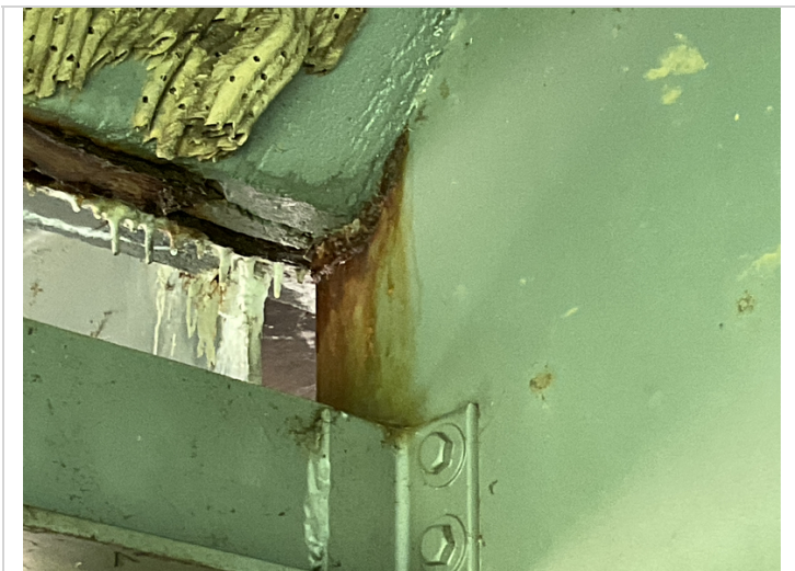
Rust with s/l to web below haunch @ Girder 2 @ end of Span 1.(#3 typical)
