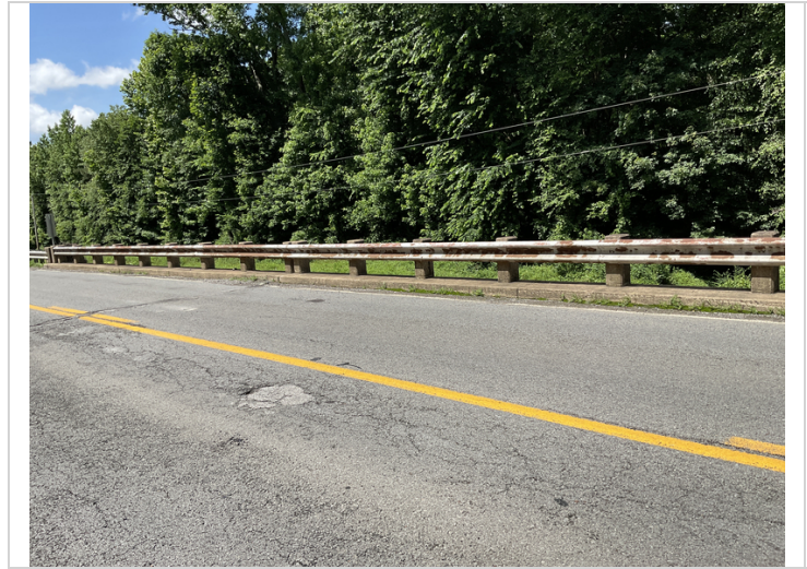
Typical rust to rails.
