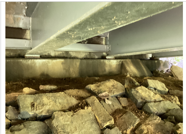
Rust to Fixed Bearings @ Abutment 1.(#2)
