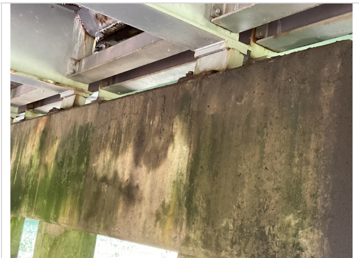
Horizontal cracking to ahead side of cap @ Bent 1.
