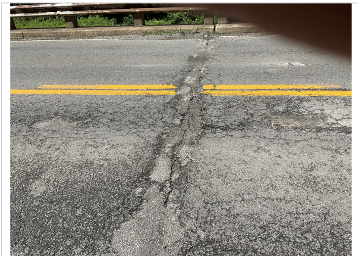
Debris impactation to joints.(#3)
