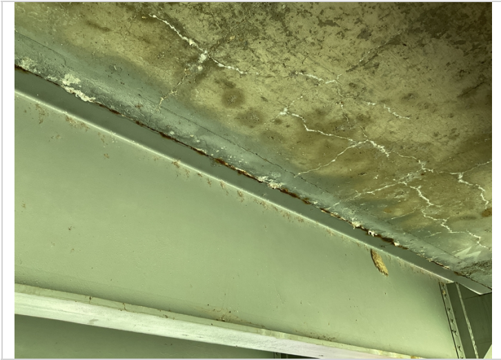
Typical rust to top flange @ all spans.(#2)
