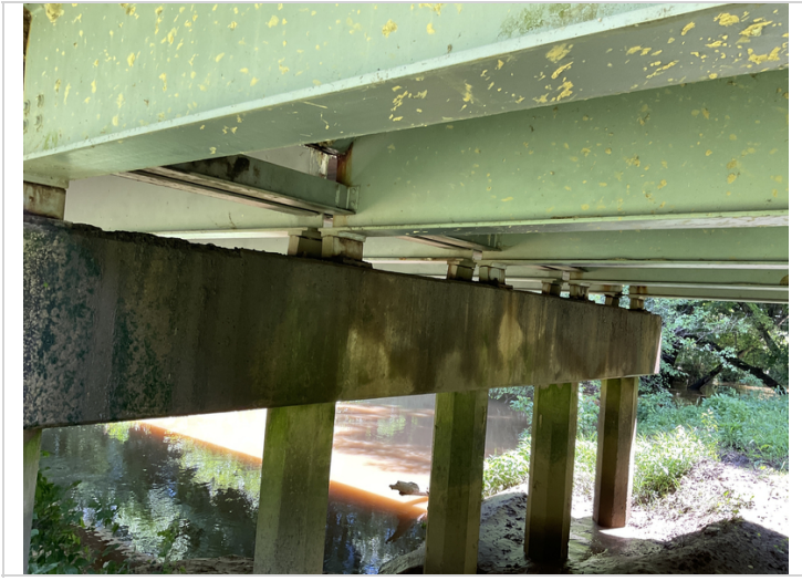
Moveable Bearings @ beginning of Span 2 are rotated back.
