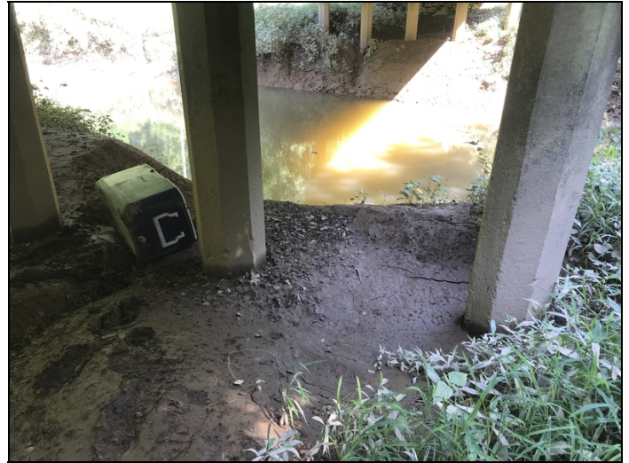
Erosion/scour to slope around Bents 1 & 2.
