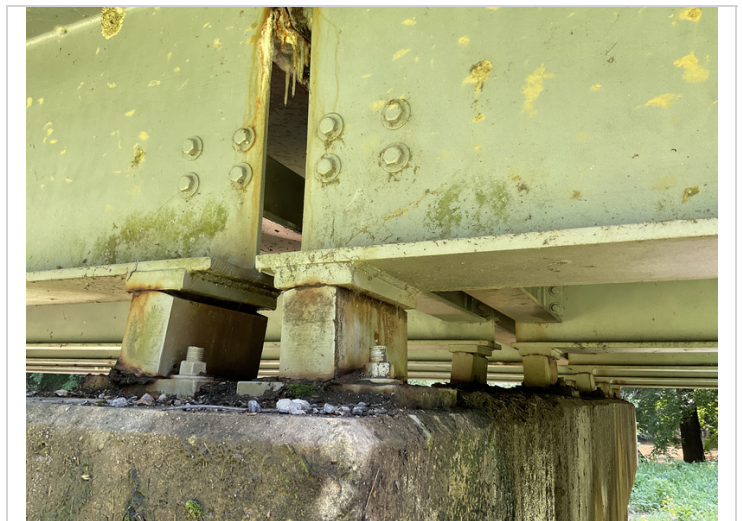
Rust @ pack rust to Moveable Bearings @ Bent 1.(#3 typical)
