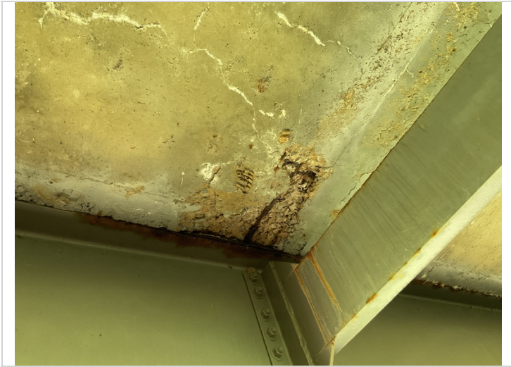
Spall with rebar exposed with s/l to soffit @ Span 3.(#3)
