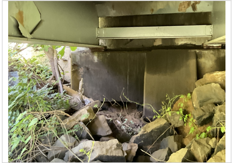
Scour 1' below & back under Left end of Abutment 2.(#3)
