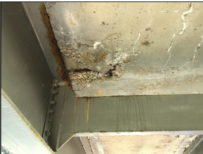
Spall with 1.5' of rebar exposed to deck below between Girders 4 & 5 at Span 3 Efflorescent Cracking to deck below at all spans.
