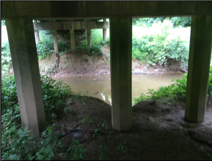
Erosion/scour to slope around Bents 1 & 2.
