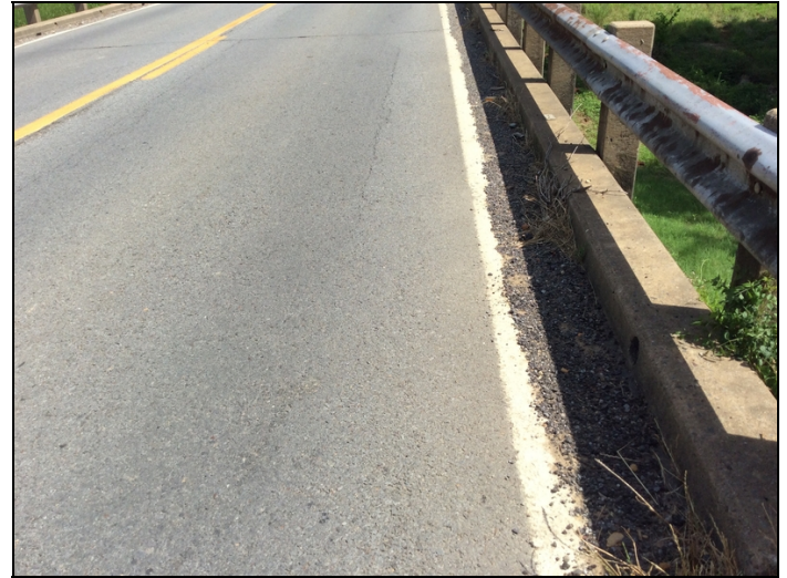
Debris in Right gutterline.
