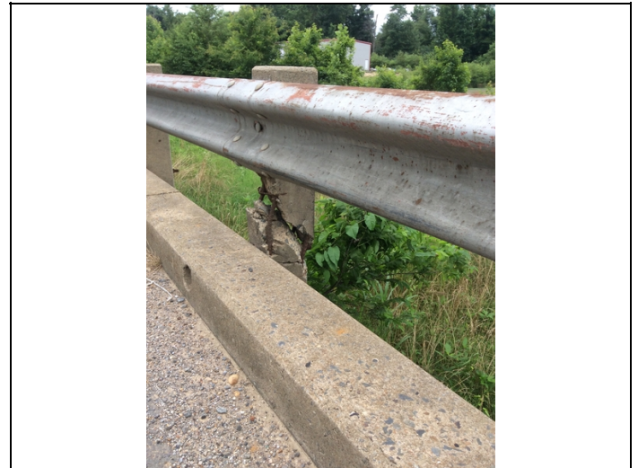
Collision damage to right rail and 5th post at Span 4.
