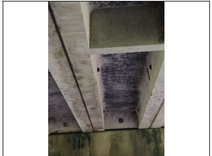
Spalls to Units 1 & 3 at Span 4. No rebar exposed.
