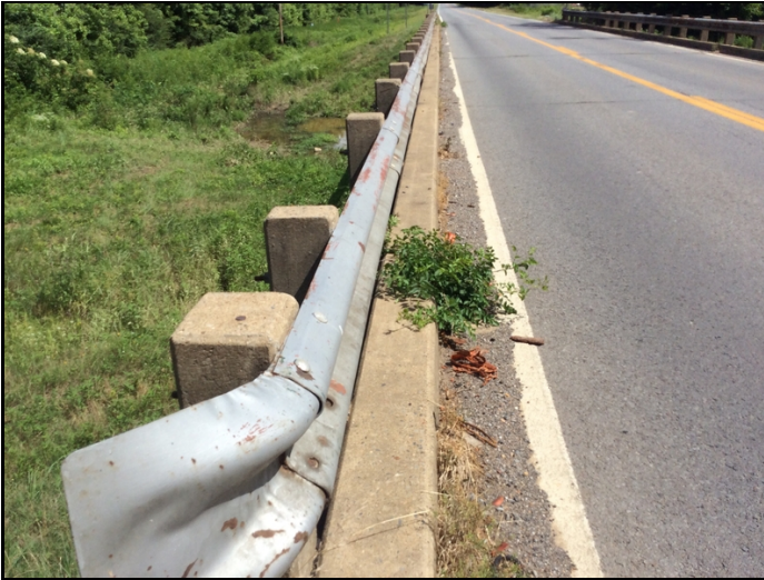
Debris in Left gutterline.
