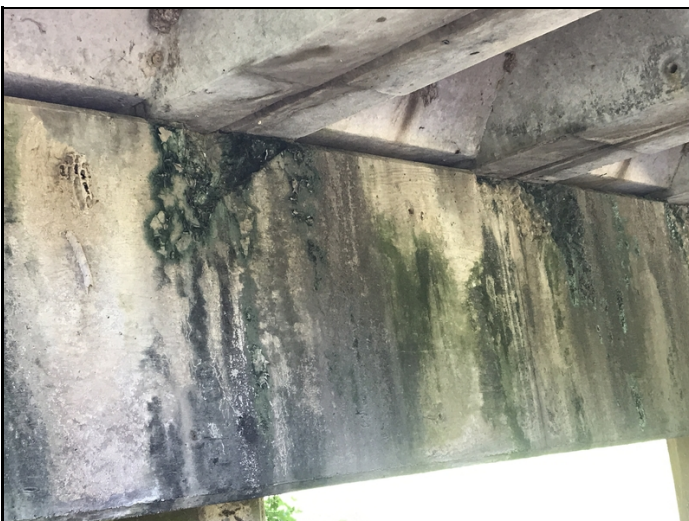
Spalls to cap at Bents 2 & 4.
