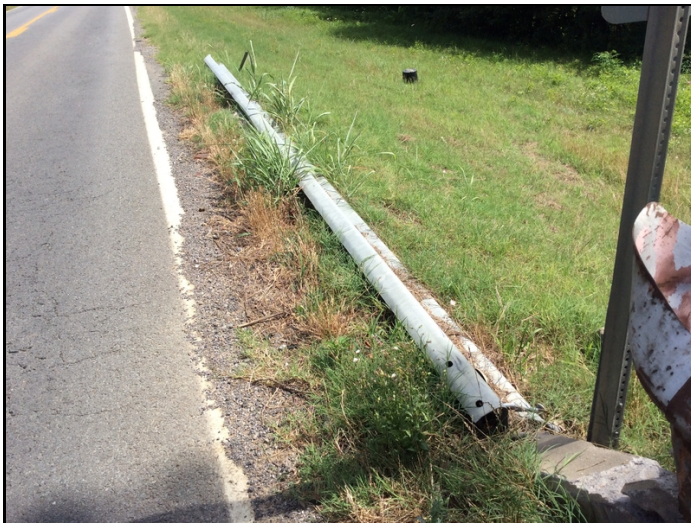
Right Approach Rail @ Abutment 2 has severe collision damage & is not functioning.
