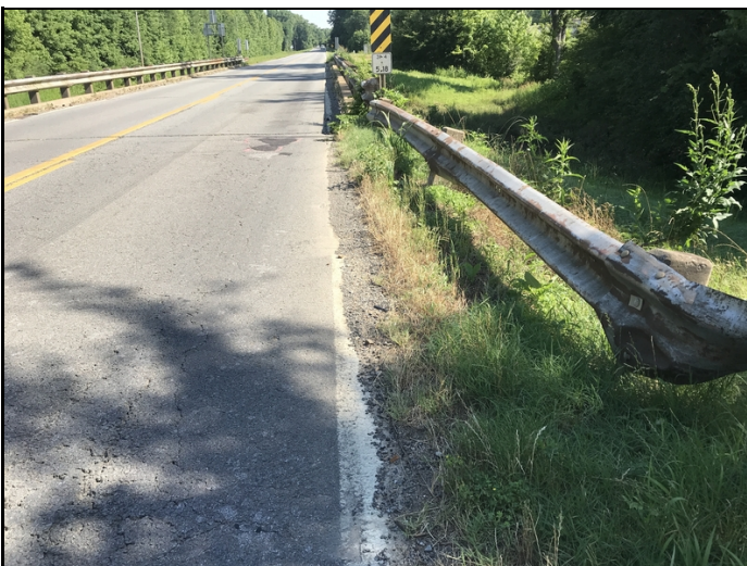
Collision damage to right rail & post at Abutment 1
