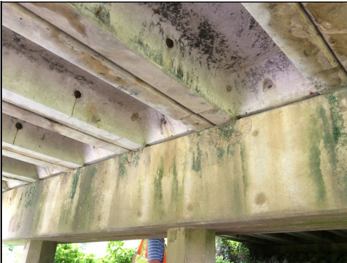
Spalls to cap at Bents 2 & 4.
