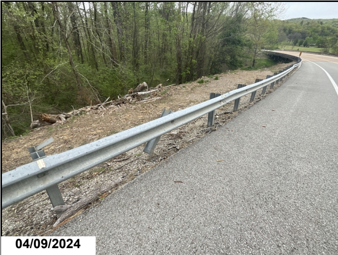
Abutment 1, Left Approach Railing, 5th post from beginning of railing: broken.
