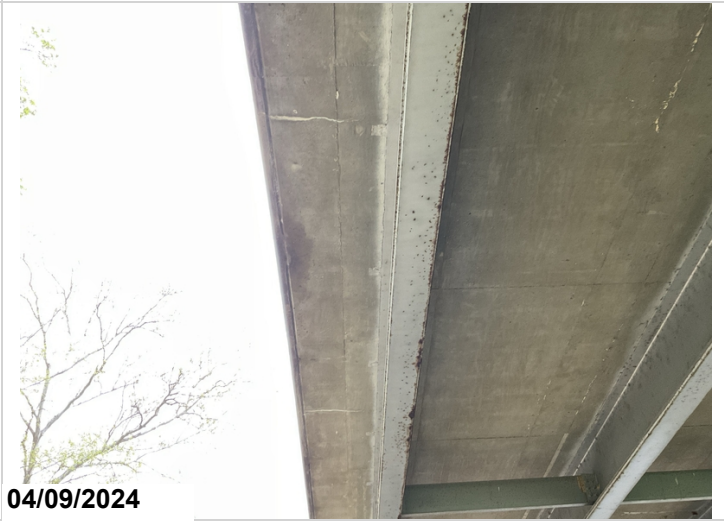
Span 2, Left overhang: cracking with efflorescence. CS2.
