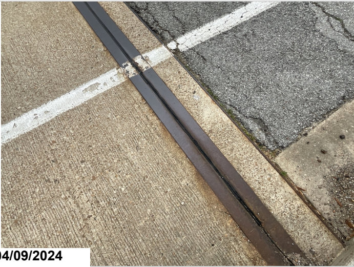
Joint at Abutment 1: seal cracking.
