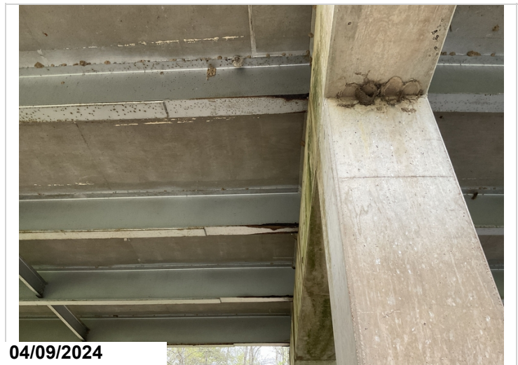
Span 2, Girders 2 - 4, Bent 2: active corrosion with flaking rust. CS3.
