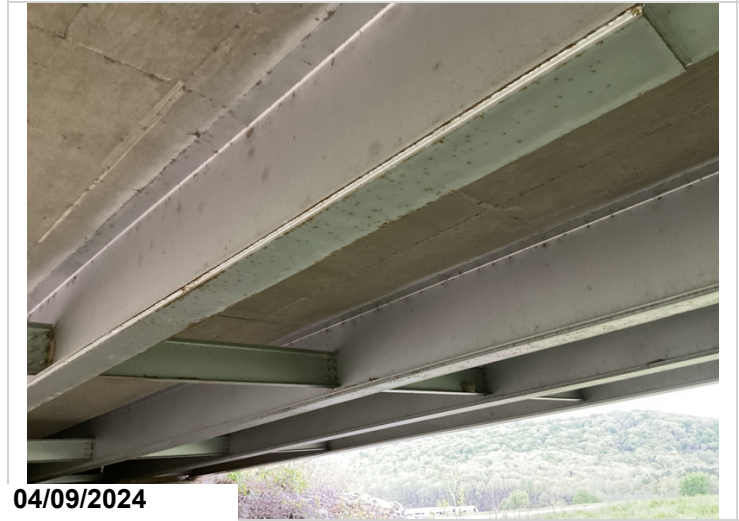
Spans 1 - 5, Girders: scattered areas of surface corrosion. CS2.
