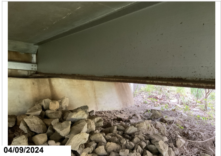
Span 1, Girder 2: surface corrosion. CS2.
