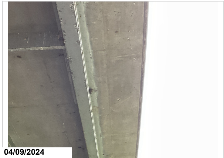
Span 3, Right overhang: cracking with efflorescence. CS2.
