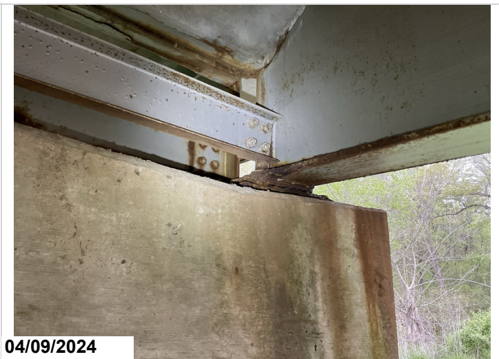
Span 5, Bent 4, Girders 1 & 2: active corrosion with flaking rust. CS3.
