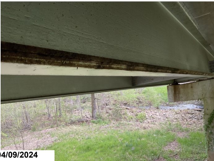
Span 1, Girder 2: active corrosion with flaking rust. CS3. 10'.
