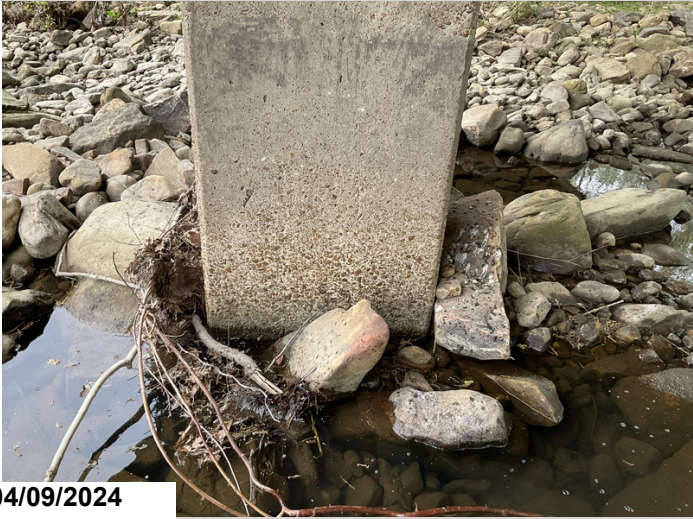
Bent 2, Columns 1 & 2: minor abrasion. CS2.
