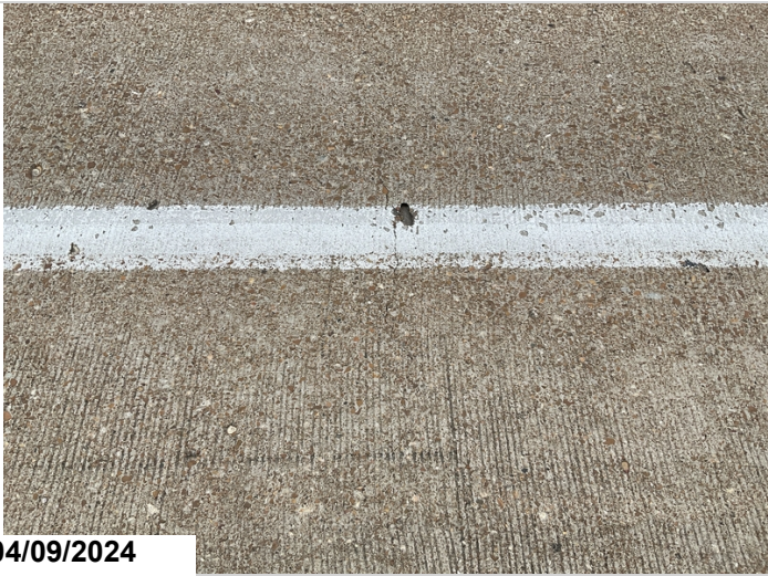
Span 4: transverse cracking. CS3.
