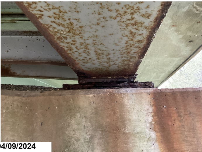
Span 5, Bent 4, Bearings 1 - 4: active corrosion with pack rust. CS3.
