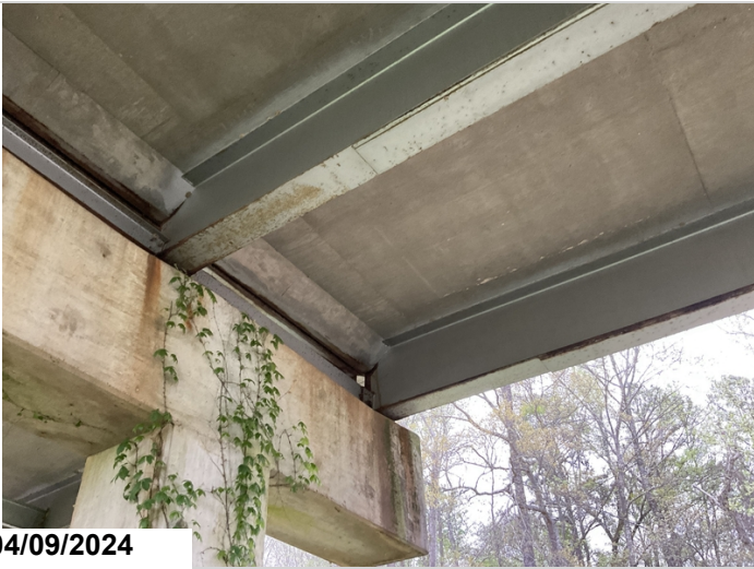
Span 2, Girders 1 - 4, Bent 1: active corrosion with flaking rust near girder ends. Girder 1: flaking rust along bottom flange to first diaphragm. CS3
