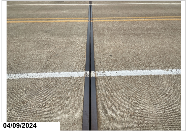
Joint at Bent 2: adhesion failure. CS3. Joint at Bent 4: adhesion failure. CS2.
