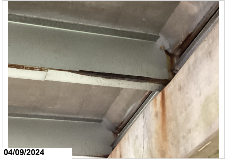
Span 1, Girder 2, Bent 1: active corrosion with flaking rust. CS3.
