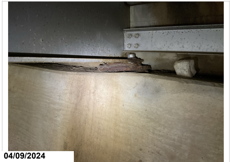
Span 1, Abutment 1, Bearing 3: active corrosion with pack rust. CS3.
