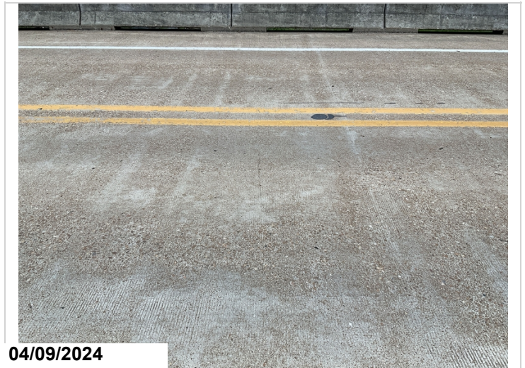
Span 4: transverse cracking. CS3.
