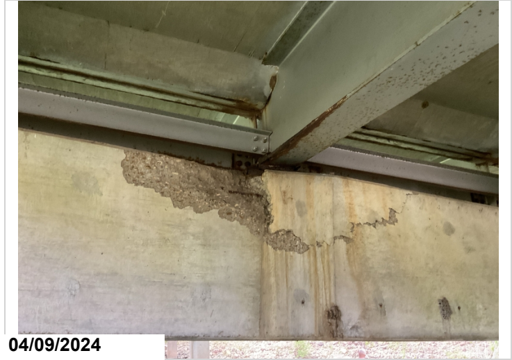
Bent 4, Ahead, adjacent to Girder 3: spalling with exposed reinforcing steel with no section loss and delaminated.
