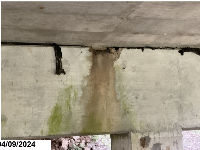
Bent 3, Back, Right Keyway: spalling. CS3.
