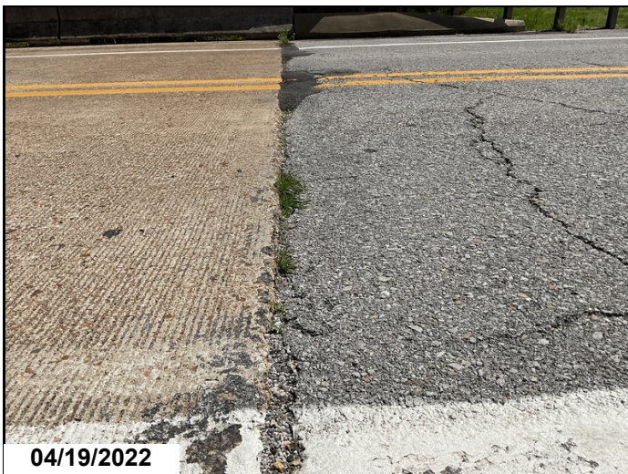
Approach roadwaysApproaches have settled at Abutments 1 and 2.Abutment 2.
