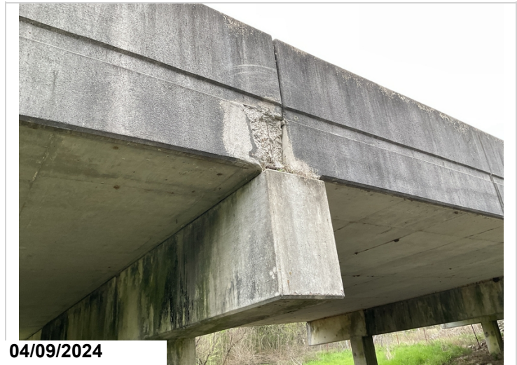
Span 1, Bent 1, Right edge of slab: large spall with exposed reinforcing steel with no section loss. CS3.
