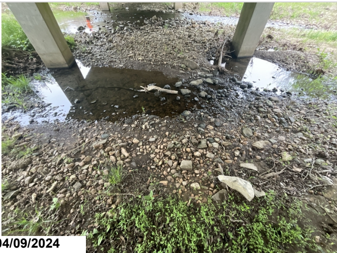
Bent 2, Columns 1 & 2: minor localized scour. CS2.
