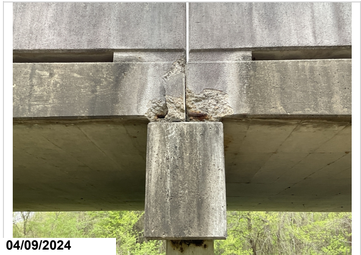
Spans 2 & 3, Bent 2, Left edge of slab: spalling with exposed reinforcing steel with section loss. CS3.
