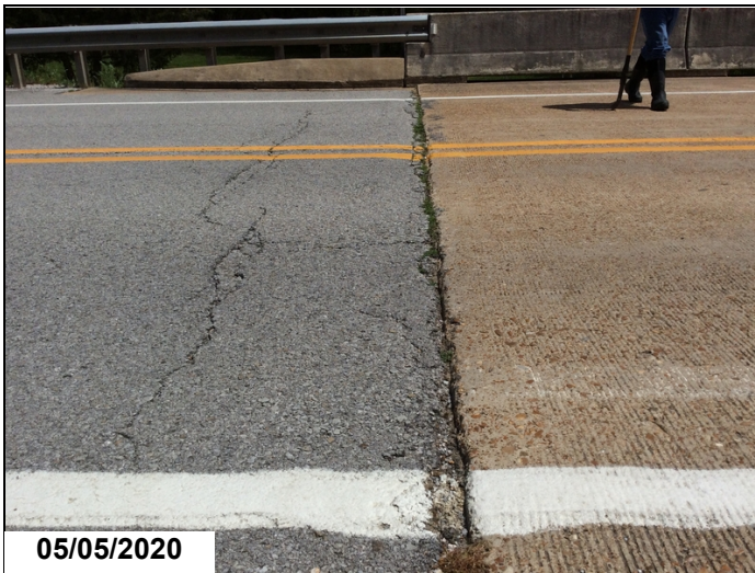
Approach roadway settlement @ Abutment 1.
