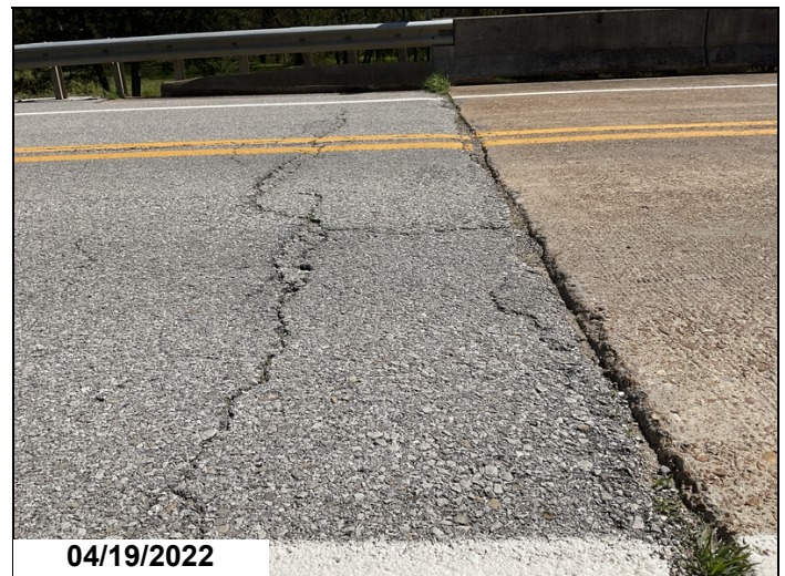
Approach roadwaysApproaches have settled at Abutments 1 and 2.Abutment 1.
