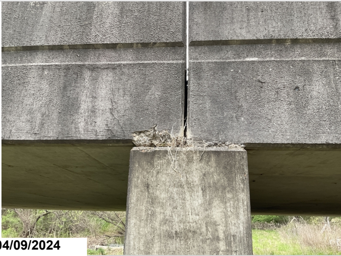
Span 3, Bent 3, Right edge of slab: spalling. CS3.
