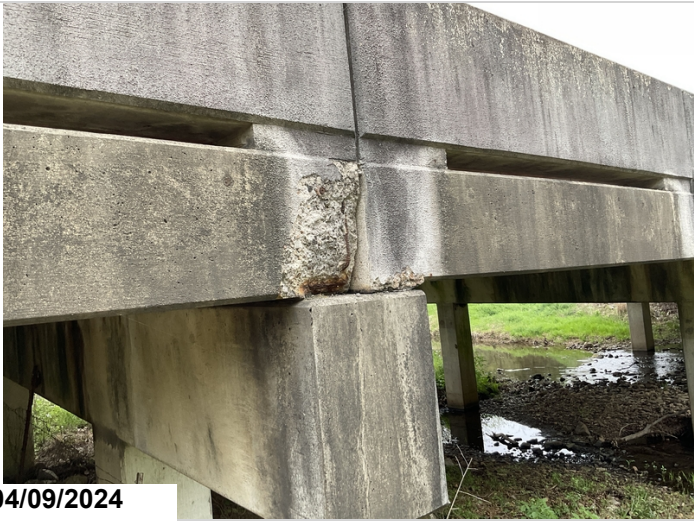
Span 4, Bent 3, Left edge of slab: spalling with exposed reinforcing steel with section loss. CS3.
