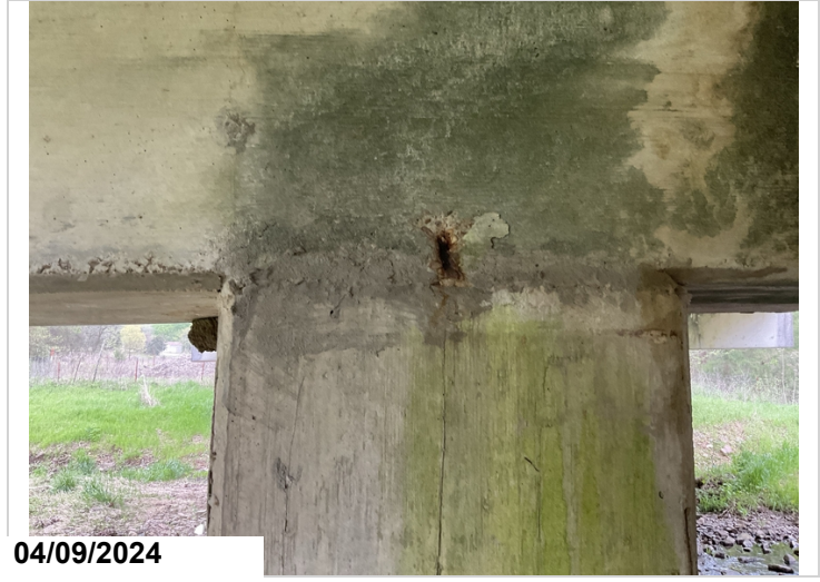
Bent 1, Back, adjacent to Column 1: exposed reinforcing steel with section loss. CS3.
