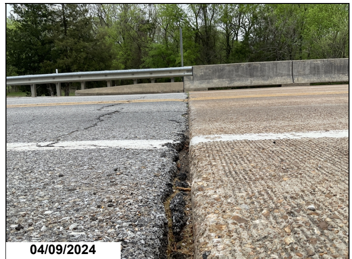
Abutment 1, Approach roadway: settlement.
