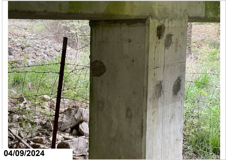
Bent 3, Column 2: spall. CS3.
