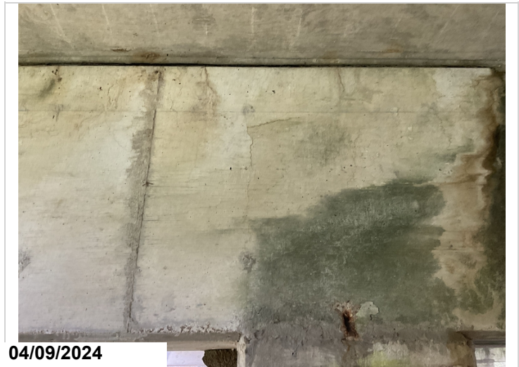
Bent 1, Back, adjacent to Column 1: vertical cracking. CS2.
