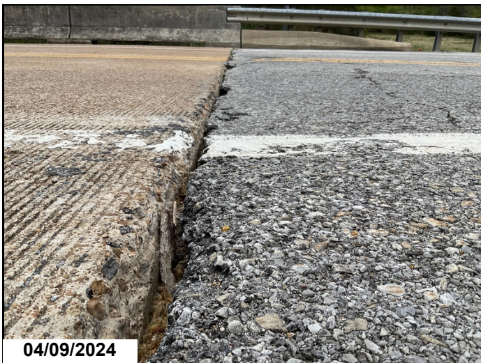
Abutment 2, Approach roadway: settlement.
