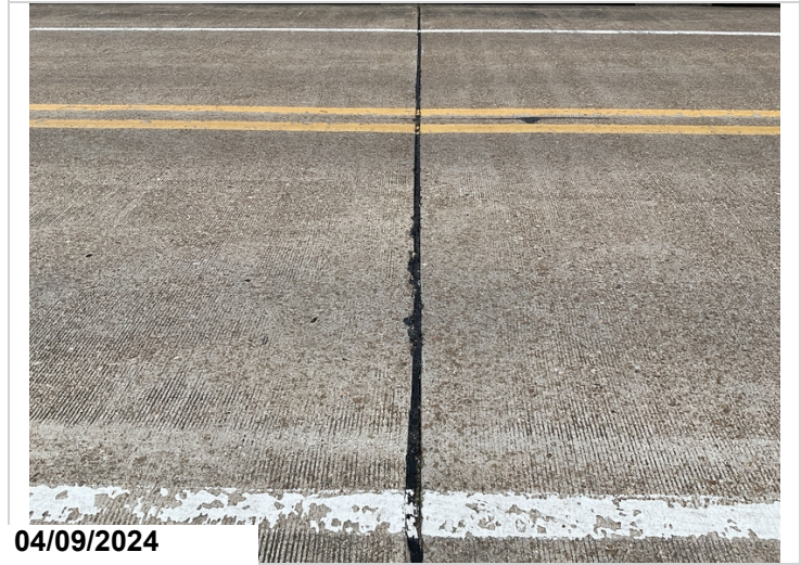
Joint at Bent 2: typical seal adhesion failure. CS3.
