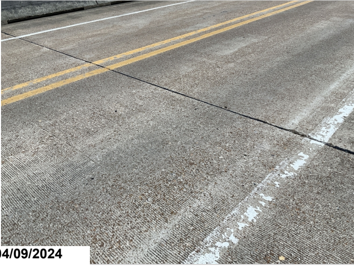
Spans 1 - 4: minor abrasion throughout structure. CS2.
