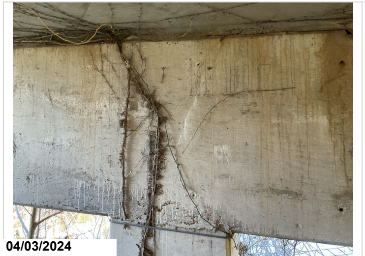
Bent 3, Ahead, adjacent to Column 3: Cracking with efflorescence to cap. CS2.
