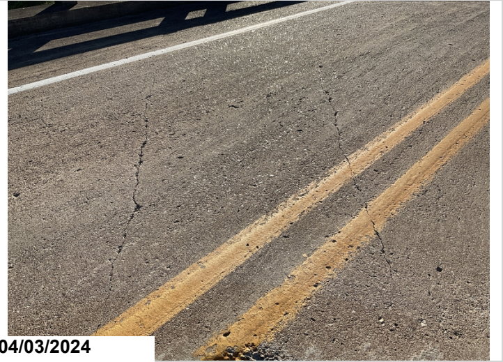
Span 3: Diagonal cracking to deck. CS3.
