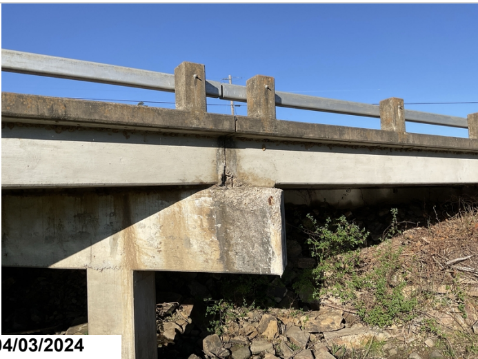
Spans 1 & 2, Right, Bent 1: Spalling with exposed reinforcing steel to outside edge of deck. CS3.
