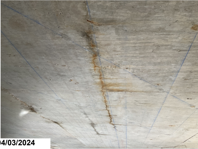
Span 1, Centerline: Cracking with rust staining to underside of deck. CS3.
