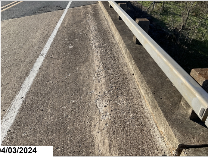
Span 4, Right gutter line: 30' of moderate abrasion to deck. CS3.
