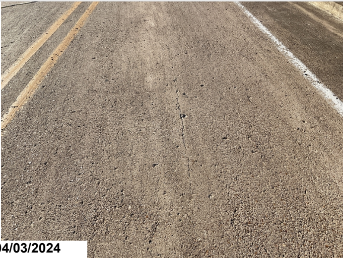
Span 2: Longitudinal cracking to deck. CS3.
