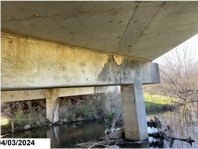
Bent 2, Back, Keyways: Delaminated areas to cap.
