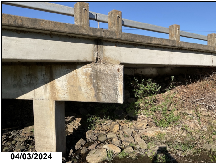
Bent 1, Left, Ahead: spalling with exposed reinforcing steel. CS3.
