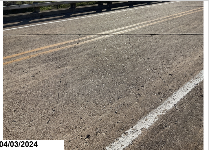
Spans 1 & 2: Diagonal cracking to deck. CS3.
