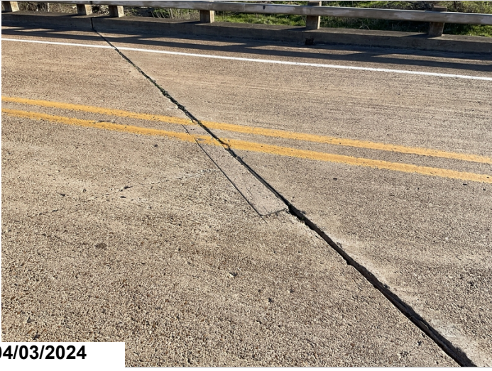
Span 1, Bent 1: 6' Patched area to deck.
