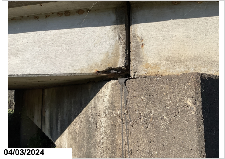
Span 4, Bent 3, Left: Spalling with exposed reinforcing steel to outside edge of deck. CS3.
