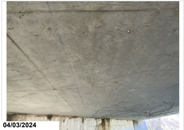
Span 3: Longitudinal cracking with efflorescence to underside of deck CS2.
