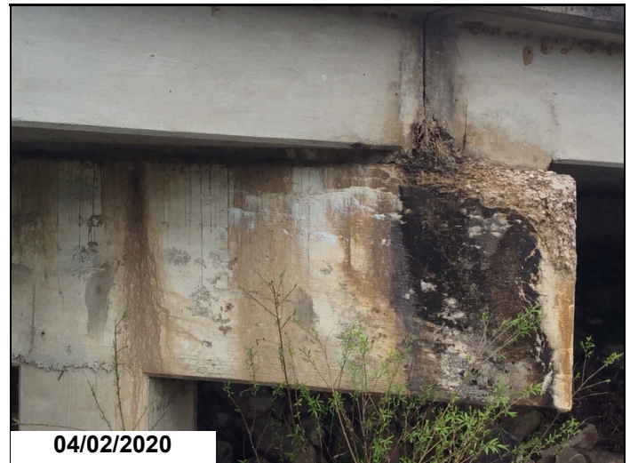
Efflorescent cracking & spalls to Left end of cap @ Bent 1.
