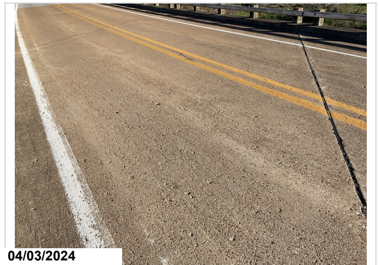
Spans 1 - 4: Abrasion to deck. CS2.
