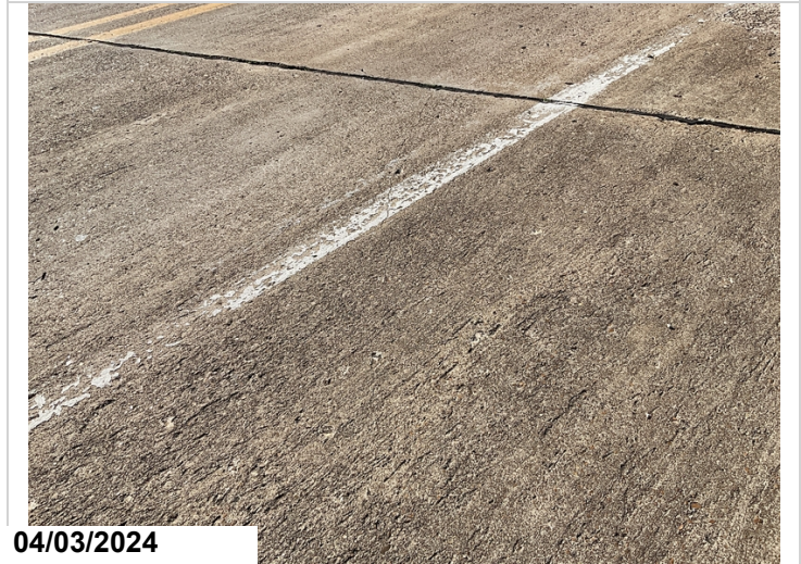
Span 2: Diagonal cracking to deck. CS3.
