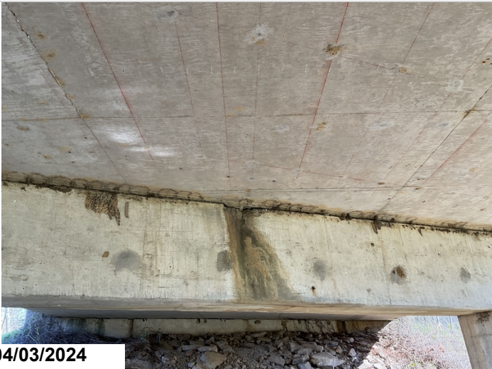
Bent 1, Ahead: Spalling to cap at key way. CS3Bent 1, adjacent to Column 1, Ahead: Delaminated area to cap.
