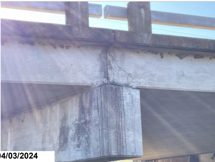
Span 3, Bent 2, Right & Left edges of slab: spalling.
