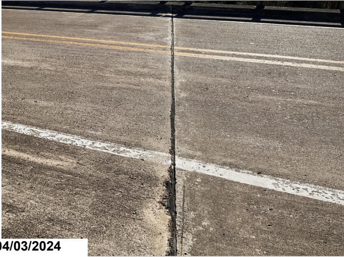
Joints at Bents 1 & 2: Seal adhesion failure.
