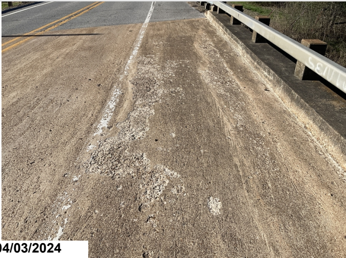
Span 3, Right & Left gutter line: Moderate to heavy abrasion to deck. CS3.
