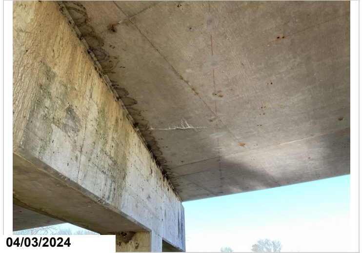
Span 2, Bent 2: Cracking with efflorescence to undersurface of deck. CS2.
