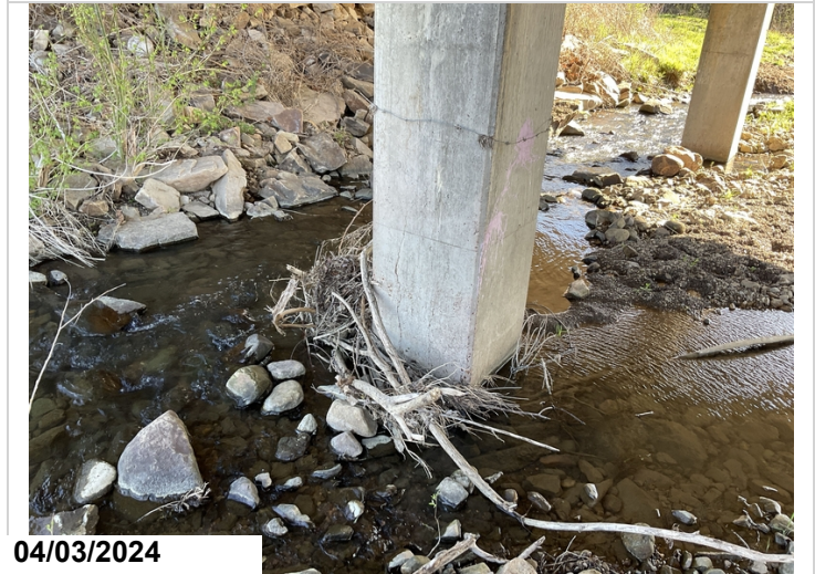
Bent 1, Column 2: vertical cracking.
