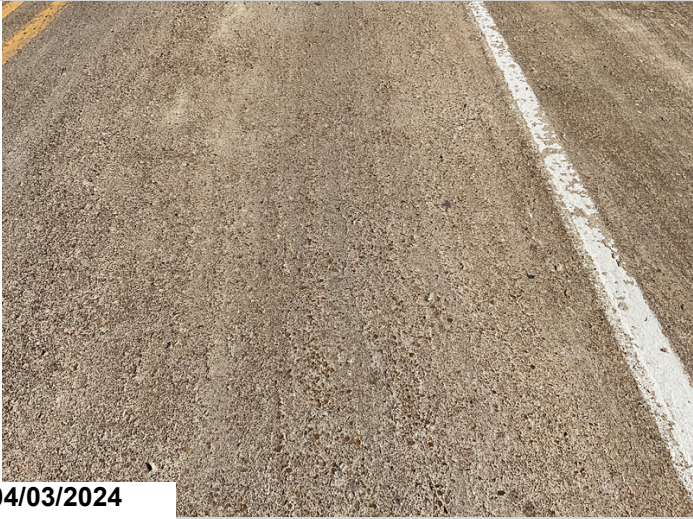
Span 1: Longitudinal cracking to deck. CS2.
