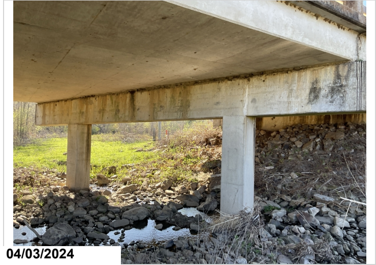
Bent 2, Back: cracking with efflorescence.
