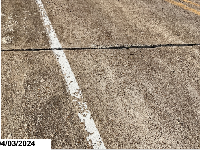
Spans 2 & 3: longitudinal cracking to deck. CS2
