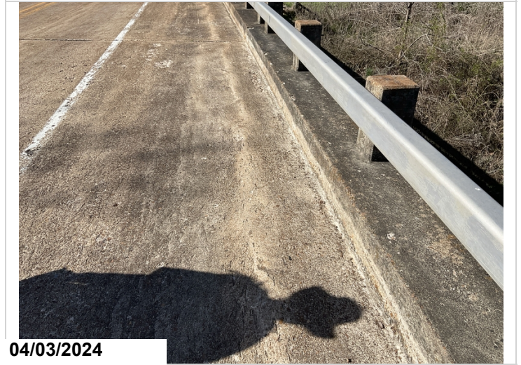
Spans 1 - 3, Right & Left gutter lines: Moderate abrasion to deck. CS3
