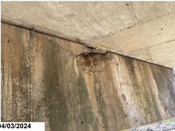
Bent 2, Ahead, adjacent to Column 1: Spalling to cap with exposed reinforcing steel. CS3.
