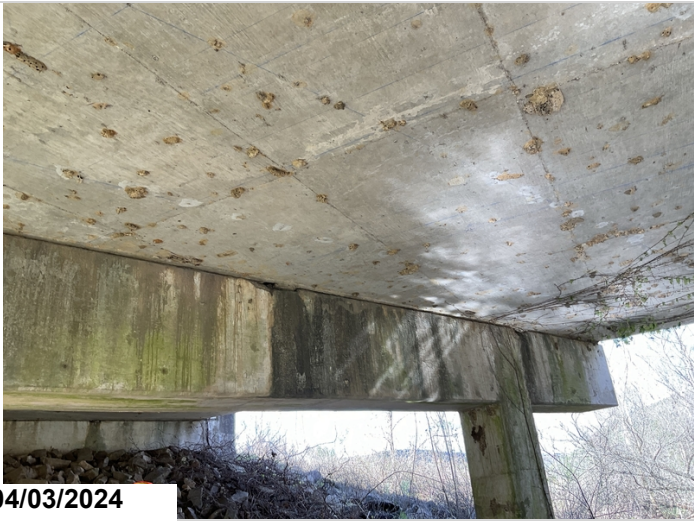
Bent 2, Back, Keyways: spalling.
