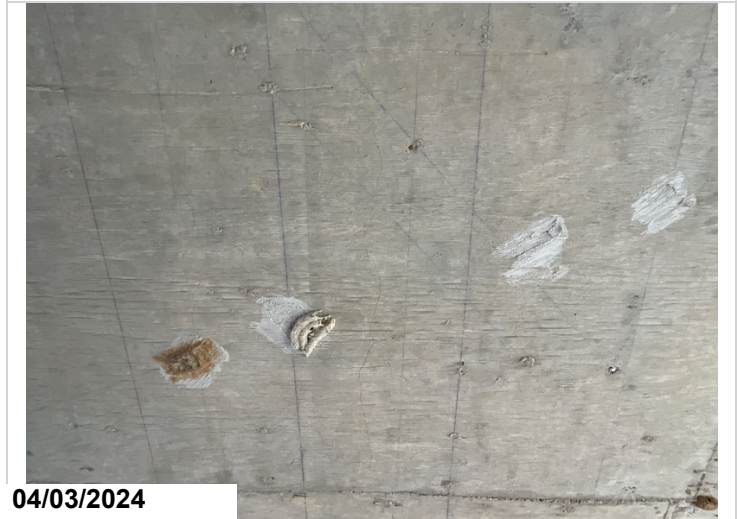
Spans 1 - 3: typical minor cracking to undersurface of deck. CS2
