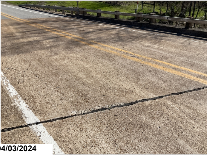
Spans 1 - 3: Minor abrasion to deck. CS2.
