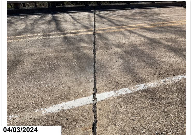
Joints at Bents 1 & 2: Seal adhesion failure. CS3.
