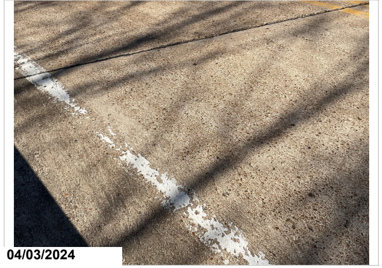
Span 1: diagonal cracking to deck. CS2.
