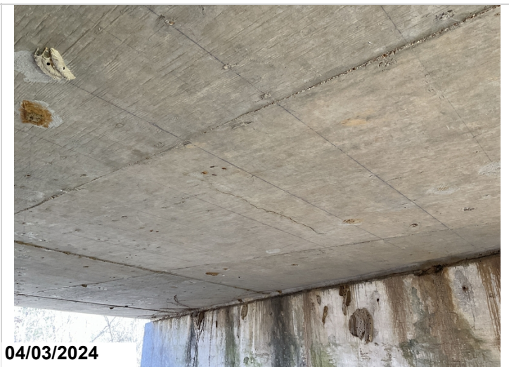
Span 3: longitudinal cracking with rust staining to undersurface of deck. CS3.
