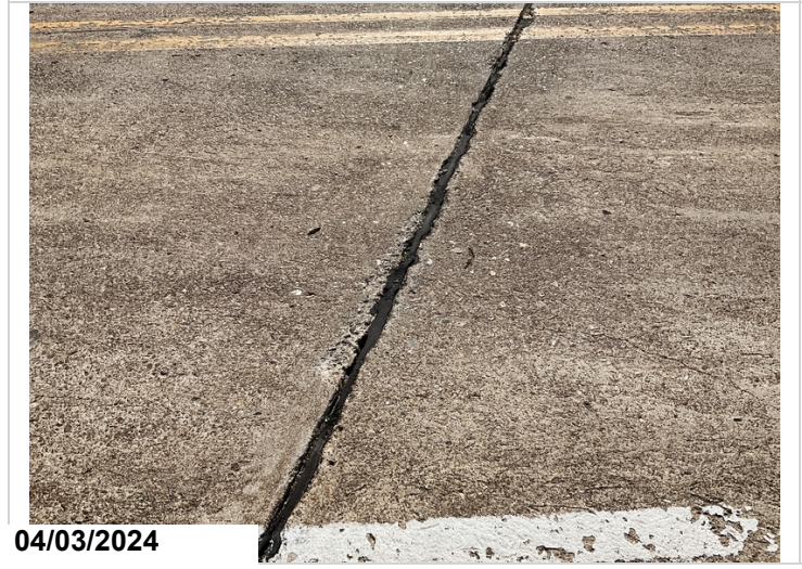
Span 2, Bent 2: spalling to deck. CS3.
