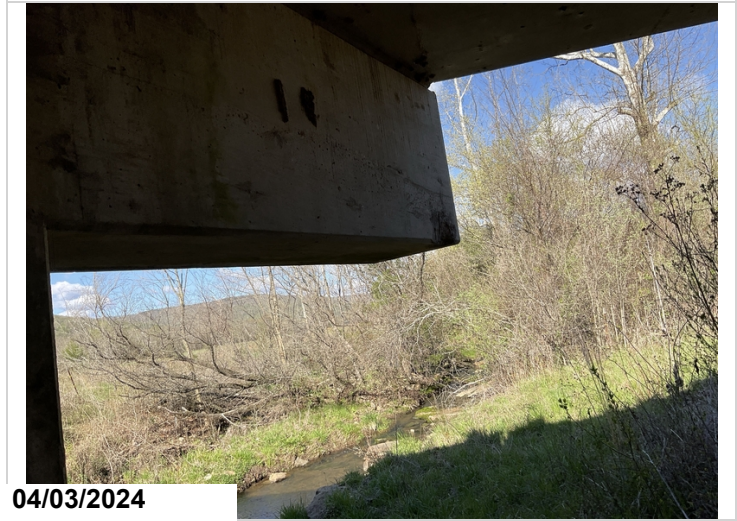
Bent 1, Back, Right: spalling. CS3.
