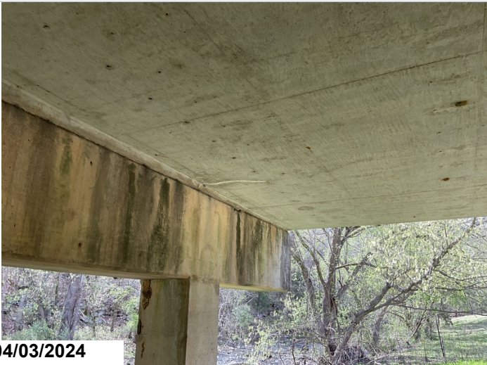
Span 1, Bent 1: cracking with efflorescence.
