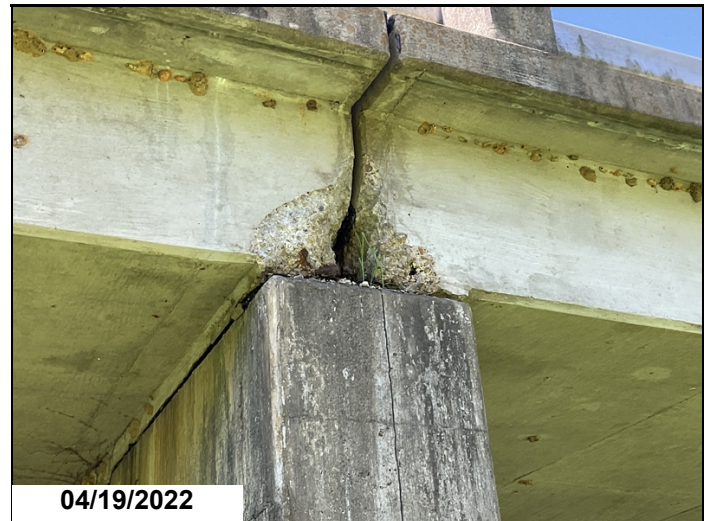
Spalls to Outside Edge of Deck @ Bents 2 & 4Lt side of bent 4.
