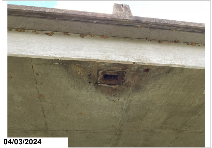
Span 4, Right drain: delaminated with minor efflorescence.
