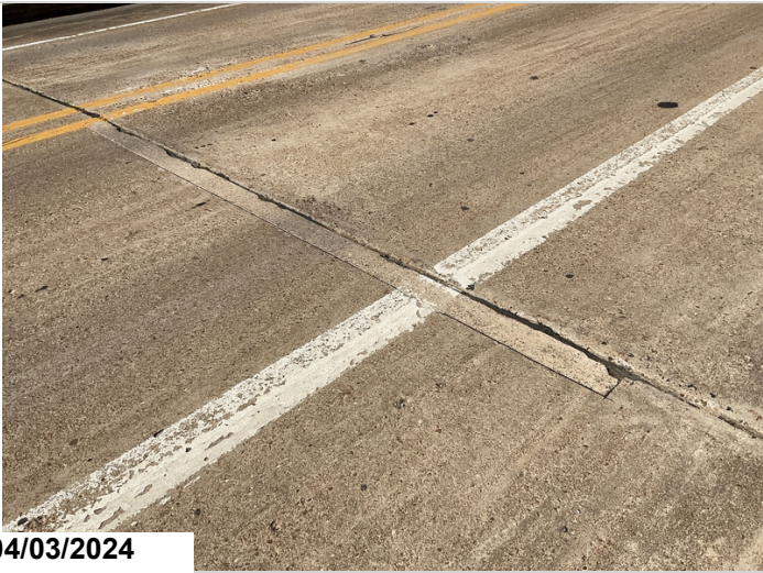
Span 2, Bent 1: 13' patched area in Left lane. CS2.
