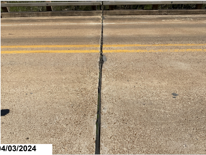
Joints at Bents 1 - 4: Typical seal adhesion failure. CS3.
