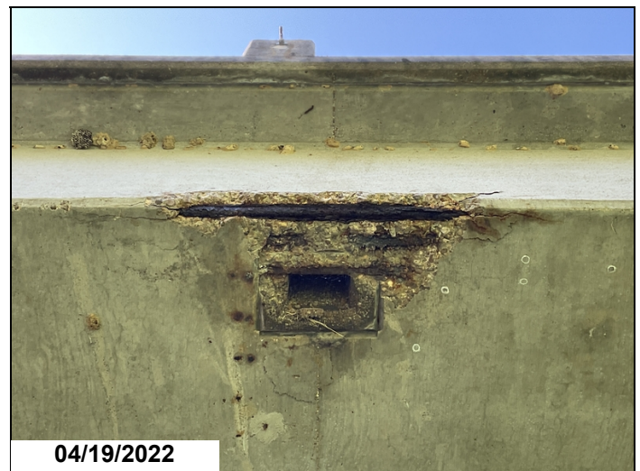
Span 5 Scaling to Left & Right Gutter Lines.
