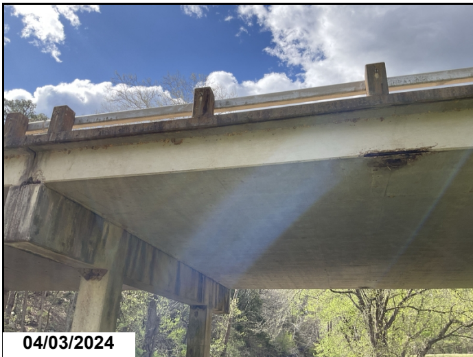
Span 2, Left edge of slab, Midspan & Bent 2: spalling with exposed reinforcing steel.
