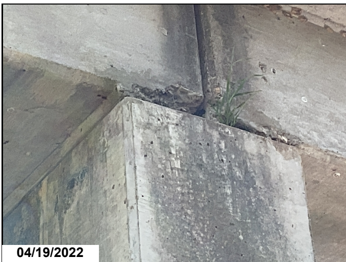
Spalls to Outside Edge of Deck @ Bents 2 & 4Rt side bent 2.
