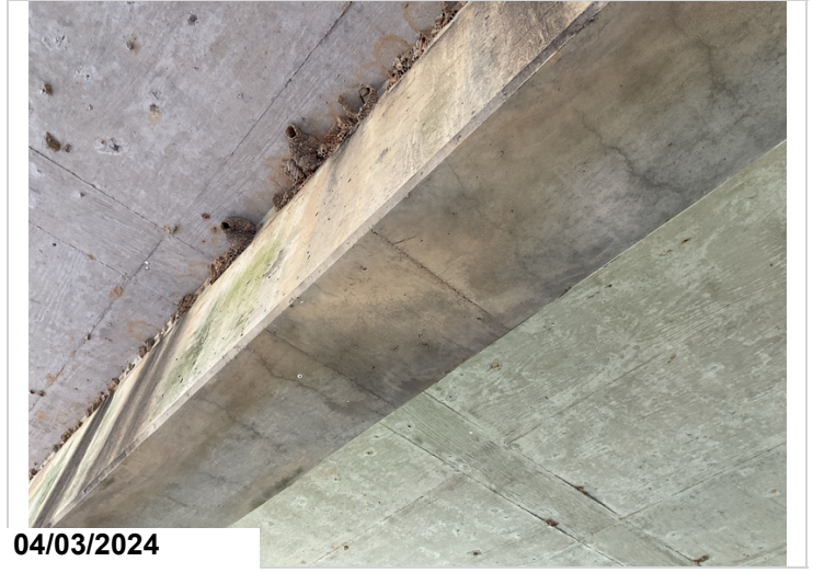
Bents 1, 2, 3, & 4, Bottom: cracking. CS2.
