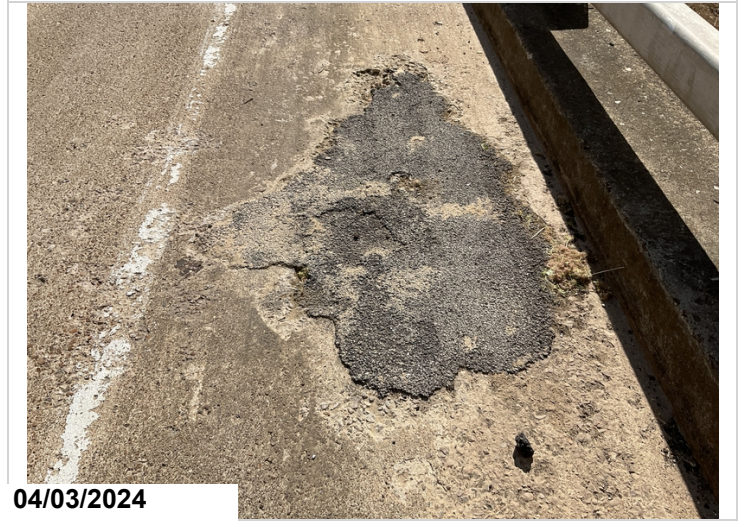
Span 5, Right gutter line: unsound patch.
