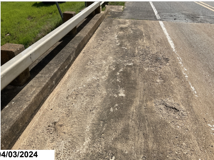
Span 5, Right & Left gutter lines: moderate abrasion. CS3.
