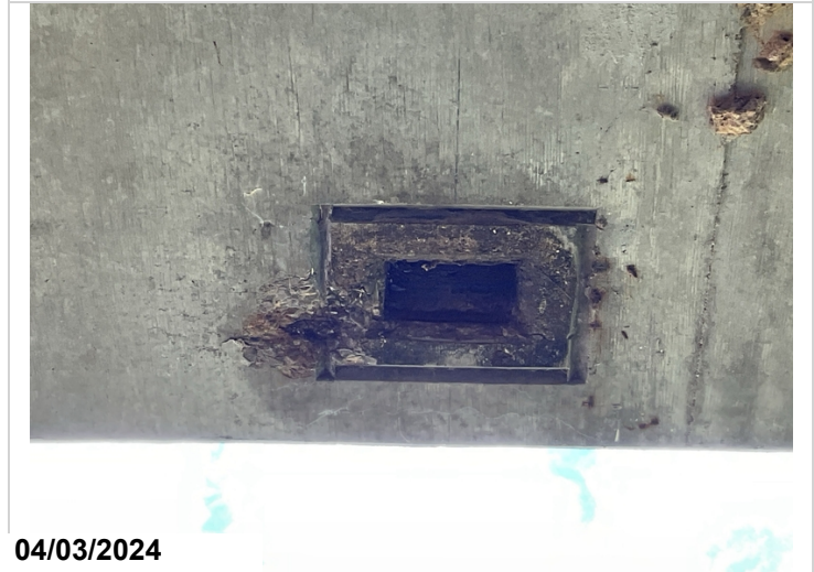
Span 4, Left & Right drains: spalling with exposed reinforcing steel. CS3.
