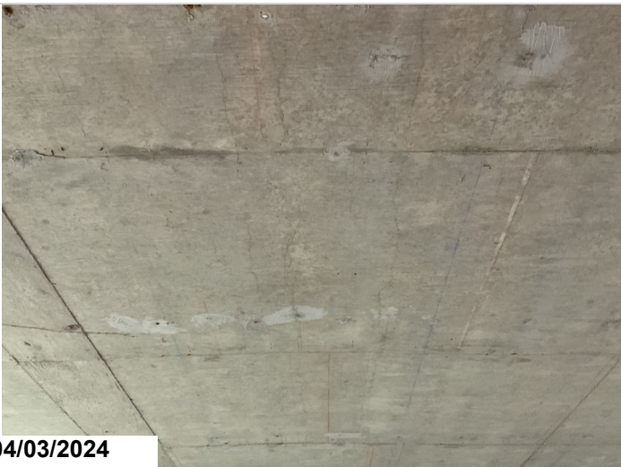
Span 5: minor hairline longitudinal cracking.
