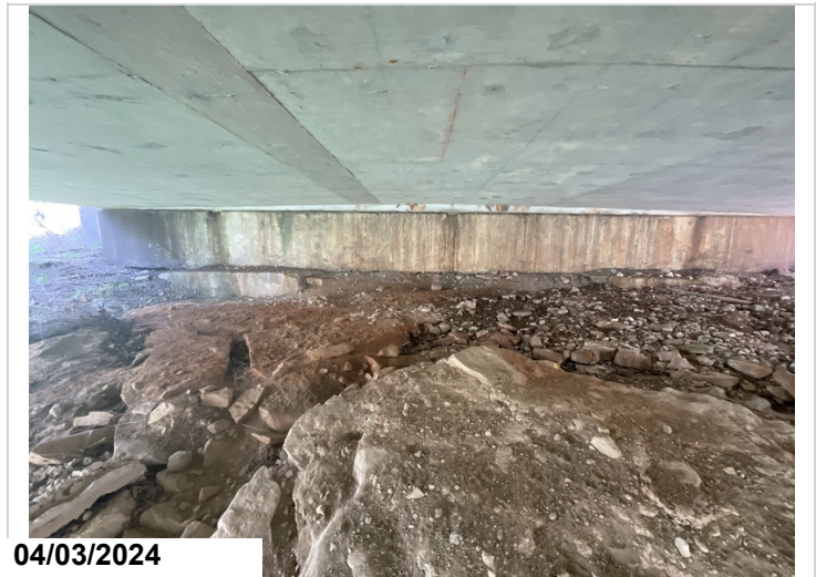
Abutment 2: minor embankment erosion.
