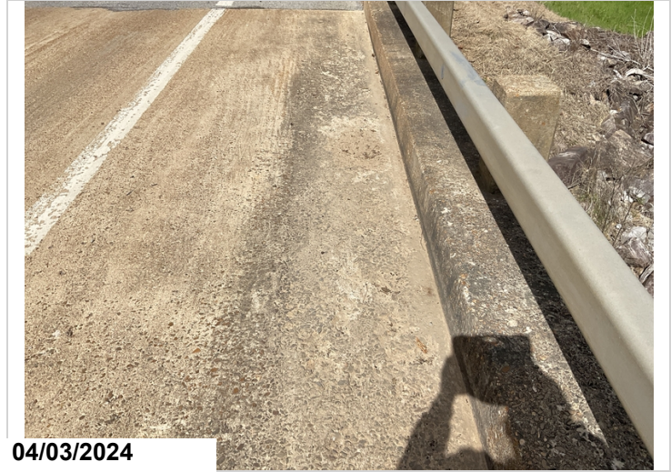
Span 1, Left gutter line: moderate abrasion. CS3.
