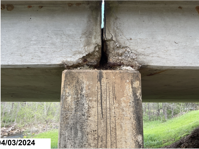
Spans 4 & 5, Bent 4, Right & Left edge of slab: spalling with exposed reinforcing steel. CS3.
