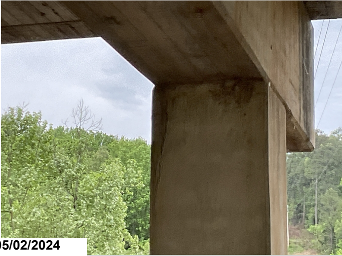
Bent 3, Column: Typical vertical cracking.
