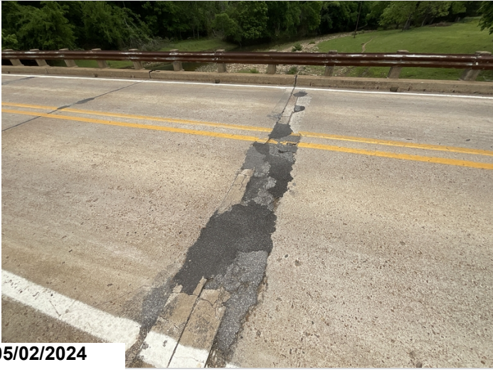
Joint at Bent 2: Unsound patched areas.
