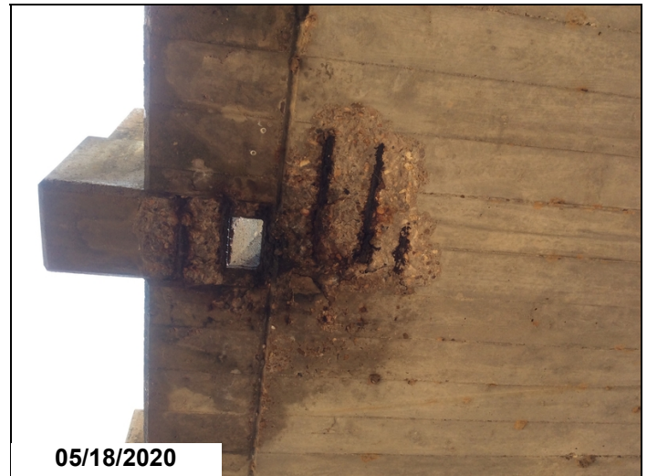
Spalls with corroded rebar exposed to soffit @ drain opening @ Left side of Span 4.
