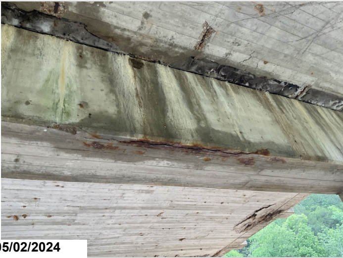
Bent 1, Bottom, Back: Wide cracking with rust staining. CS3.
