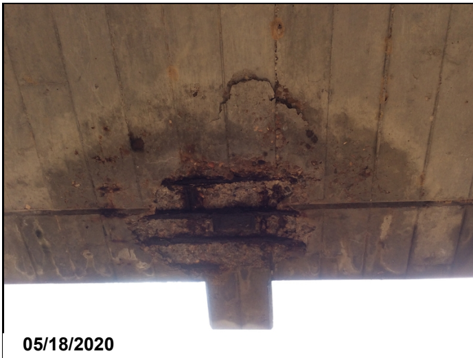
Spalls with corroded rebar exposed to soffit @ drain opening @ Right side of Span 4.
