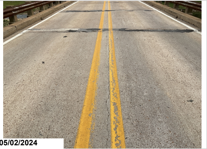
Spans 1 & 2: Longitudinal cracking. CS3.
