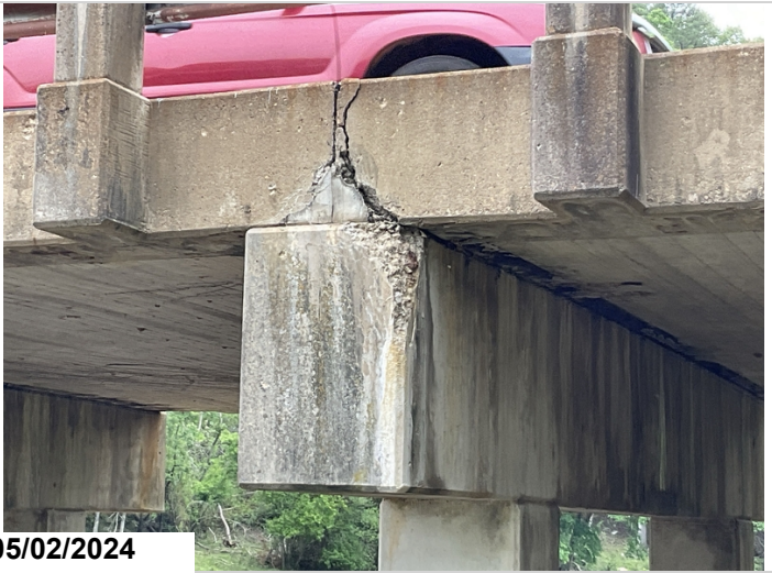
Bent 1, Left: Spalling with exposed reinforcing steel with section loss. CS3.
