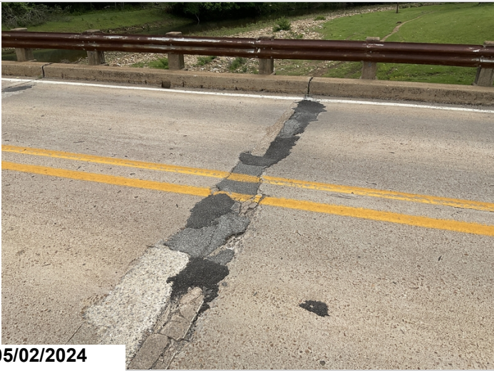
Joint at Bent 1: Unsound patched areas.
