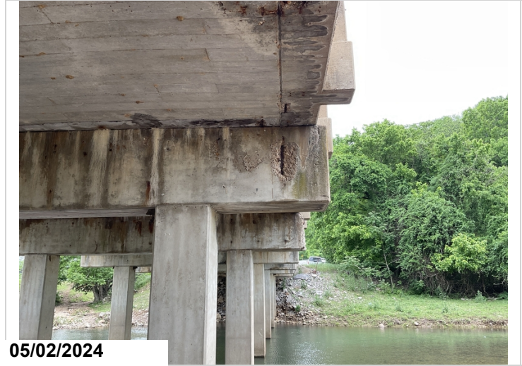
Bent 4, Back, Right: Spalling with exposed reinforcing steel. CS3.
