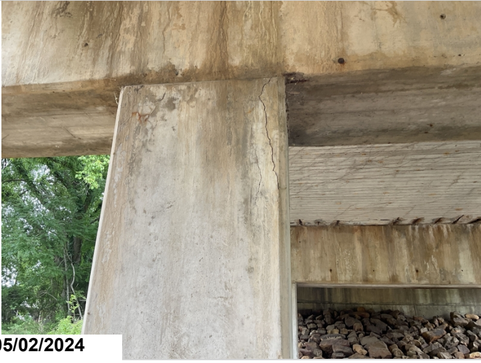
Bent 2, Columns: Typical vertical cracking. CS2.
