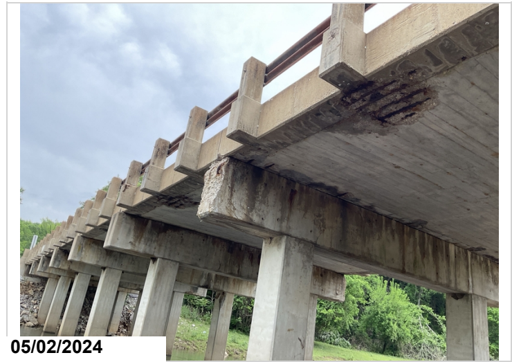
Bent 4, Left: Spalling with exposed reinforcing steel with section loss. CS3.
