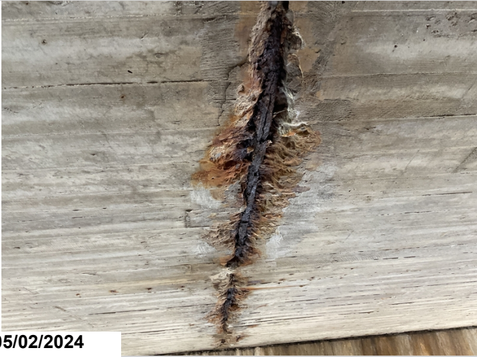
Span 10, Centerline: Spalling with exposed reinforcing steel with section loss. CS3.
