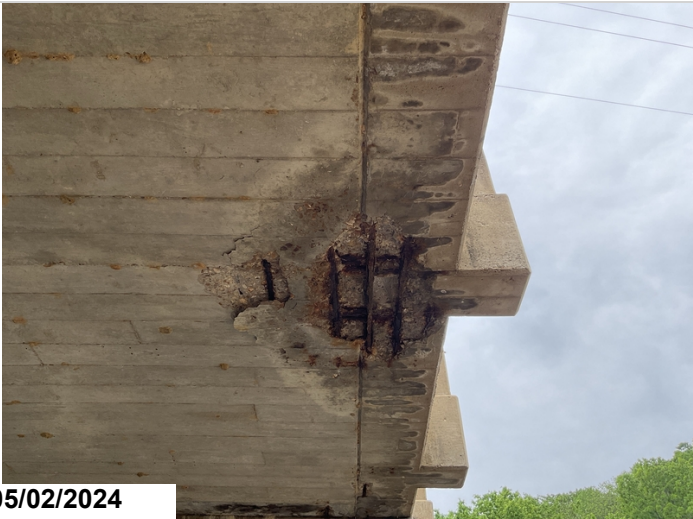
Span 4, Drains: Spalling with exposed reinforcing steel with section loss. CS3.
