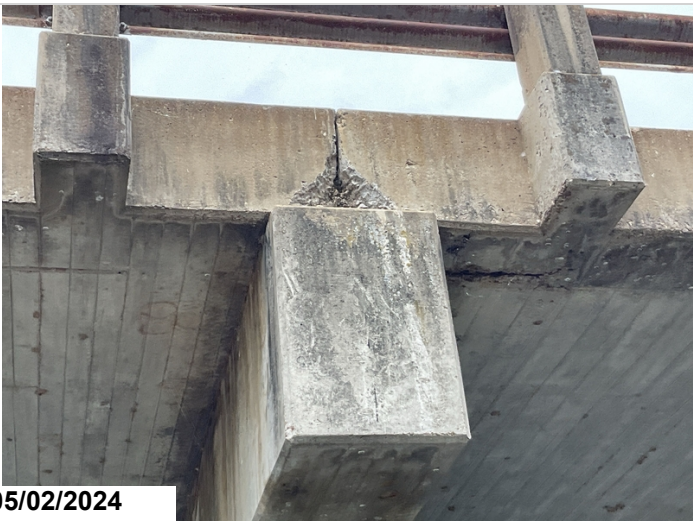
Spans 6 & 7, Bent 6: Typical spalling to edge of Slab.
