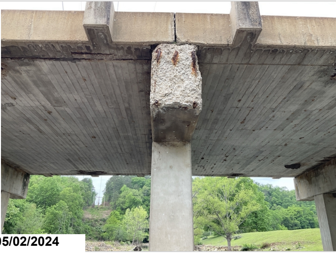
Bent 5, Right: Spalling with exposed reinforcing steel with section loss. CS3.
