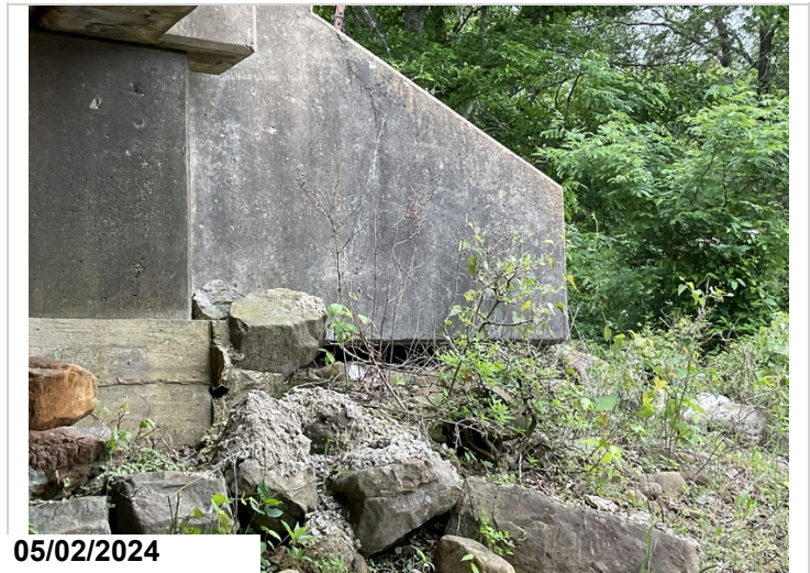
Abutment 1, Left Wing Wall: Undermining.
