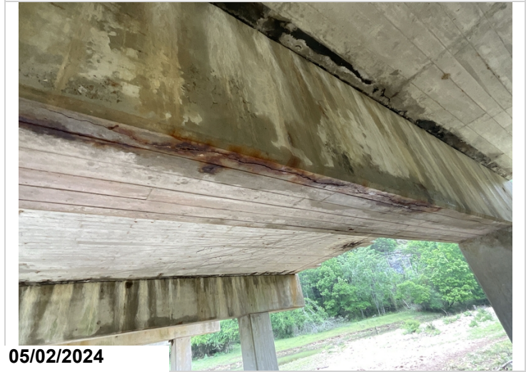
Bent 1, Bottom, Back: Delaminated area for 10'.
