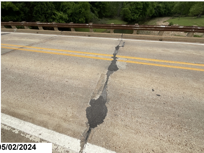
Joint at Bent 6: Unsound patched areas.
