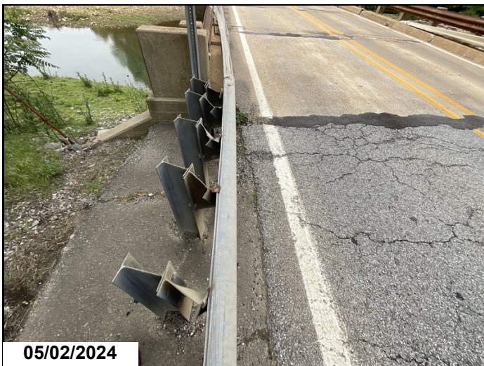
Abutment 2, Right, Transition: Damage.
