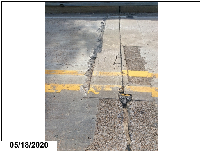
Span 10: Spalls to deck at joint.
