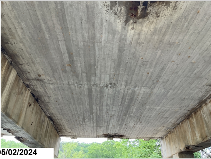
Span 9, Undersurface: Longitudinal cracking with efflorescence. CS2
