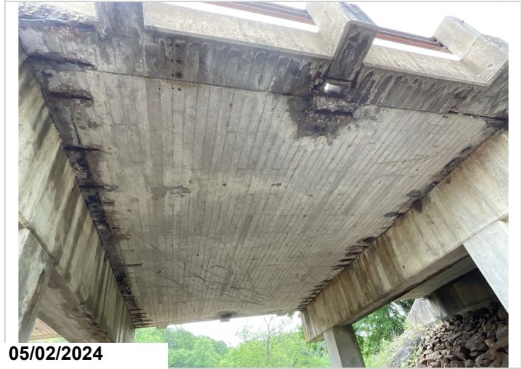
Span 2: Numerous spalls with exposed reinforcing steel section loss. CS3.
