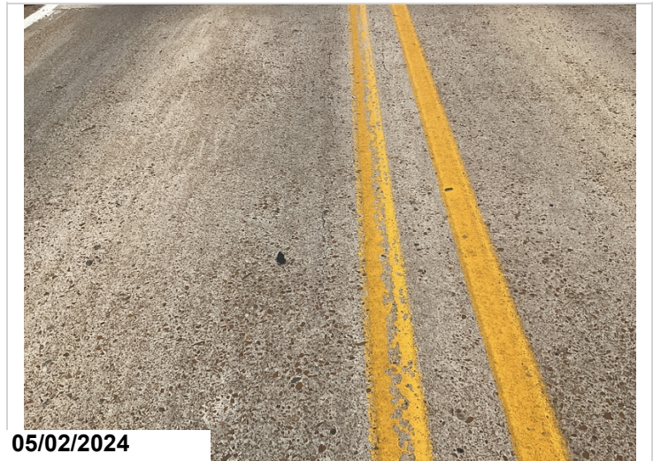
Span 3: Longitudinal cracking. CS3.
