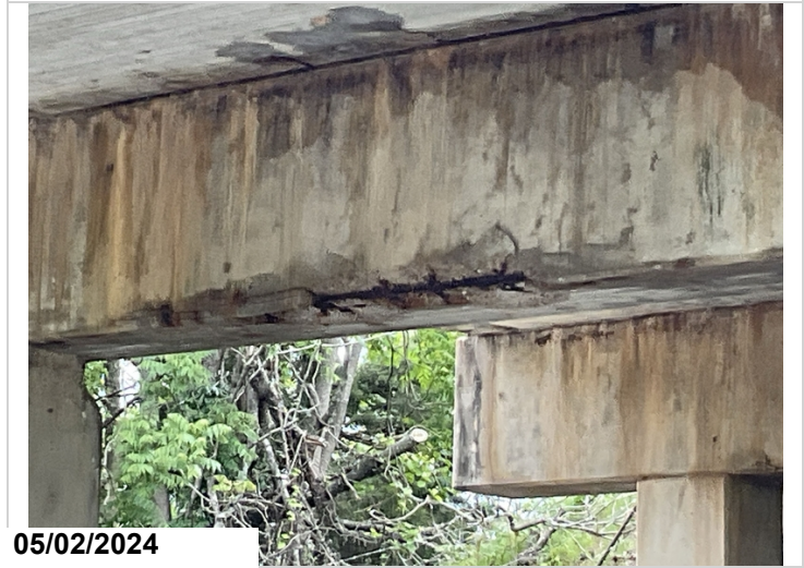
Bent 8, Back, Bottom: Spalling with exposed reinforcing steel with section loss. CS3..
