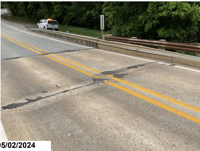
Joint at Bent 9: Patched & unsound patched areas.
