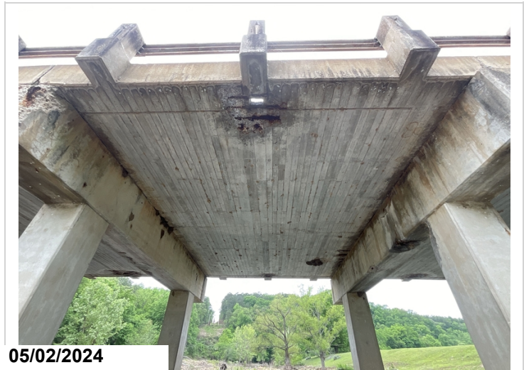
Span 6, Drains: Spalling with exposed reinforcing steel. CS3.
