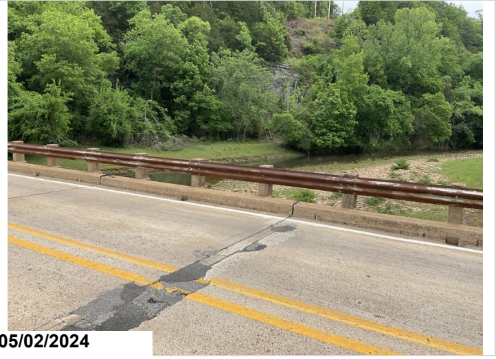
Bridge Railing: Surface corrosion typical throughout the Structure.
