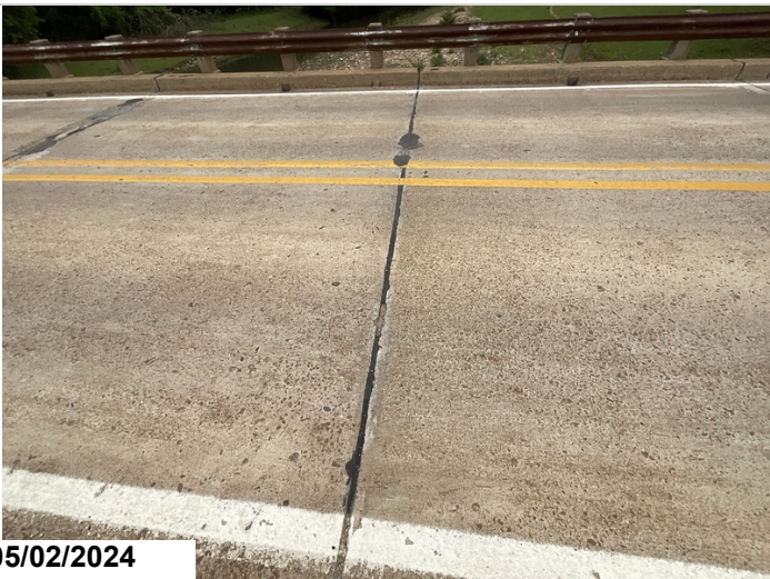
Joint at Bent 3: Seal adhesion failure.
