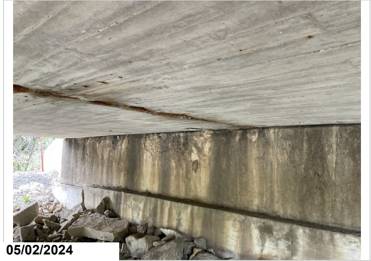
Abutment 2: Spalling.
