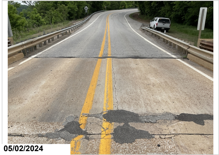
Span 10: Longitudinal cracking. CS3.
