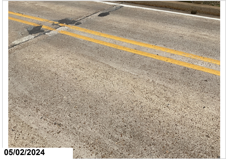
Span 5: Longitudinal & transverse cracking. CS3.
