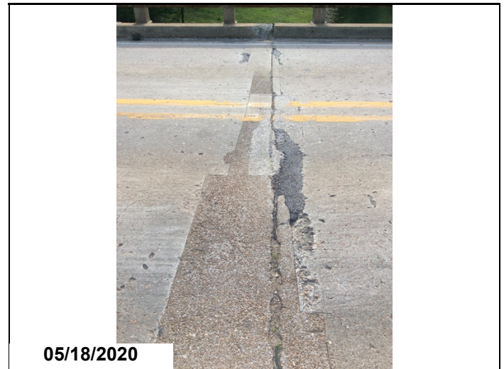
Spans 8 & 9 have spalls at joints.
