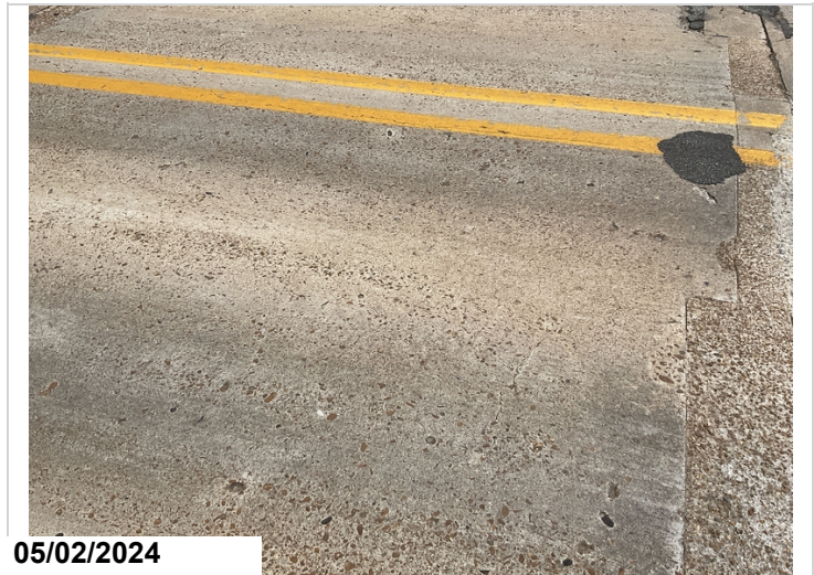
Span 9: Map cracking. CS3.
