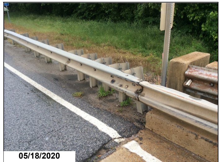
Right bridge rail @ Abutment 2. Collision damage.
