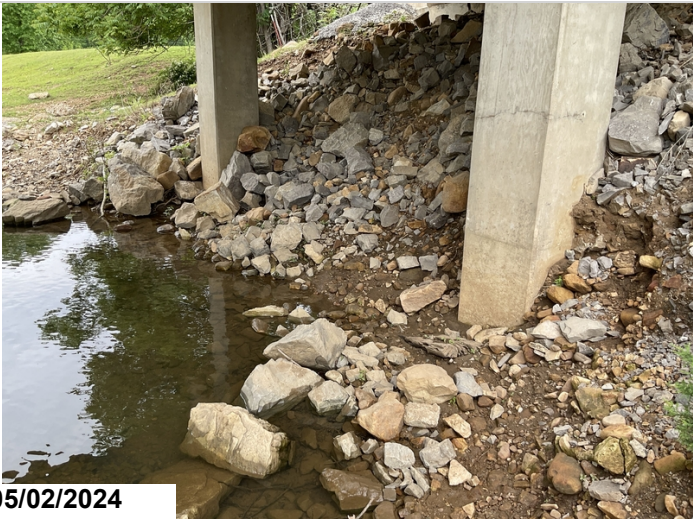
Bent 9, Columns: Embankment erosion.
