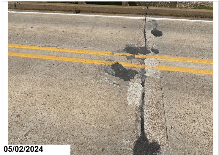
Span 6, Bent 5, near Centerline: Unsound patches & delaminated area.
