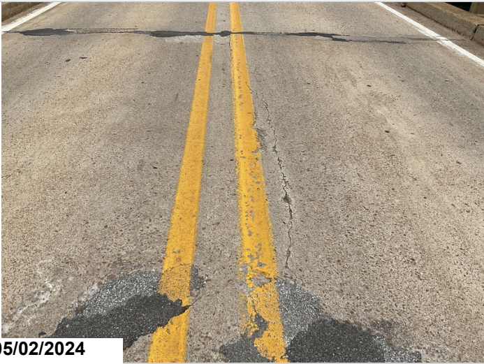
Span 6: Longitudinal cracking. CS3.
