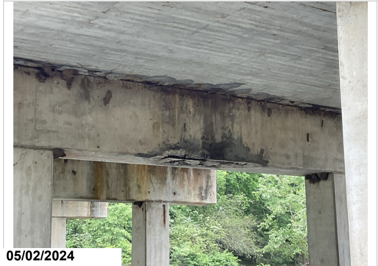
Bent 7, Ahead, Bottom: Spalling with exposed reinforcing steel with section loss. CS3.
