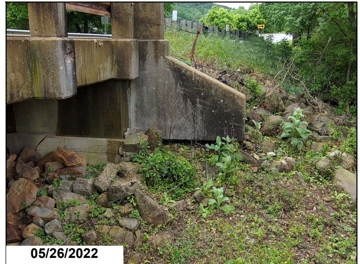
Abutment 1: Left wing is undermined 6" down and 1' back under.
