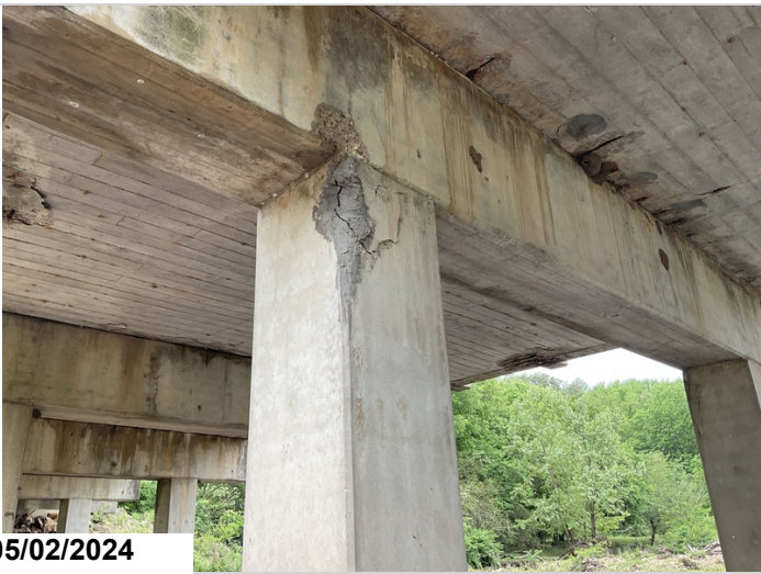
Bent 4, Column 2: Delaminated.
