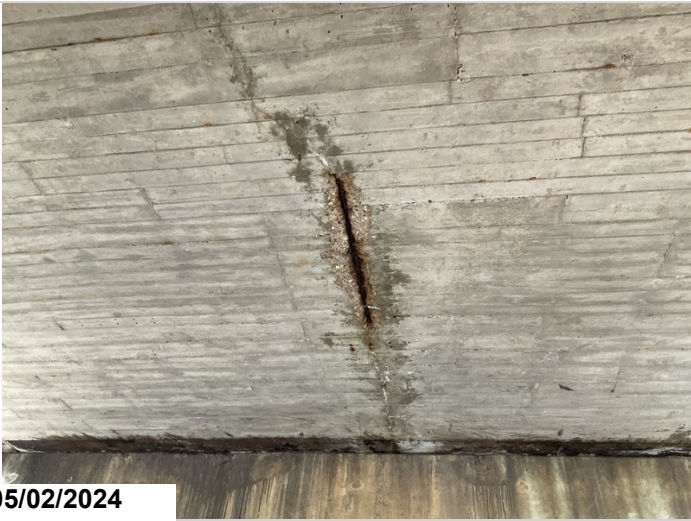
Span 1, Centerline: Spalling with exposed reinforcing steel with section loss. CS3.
