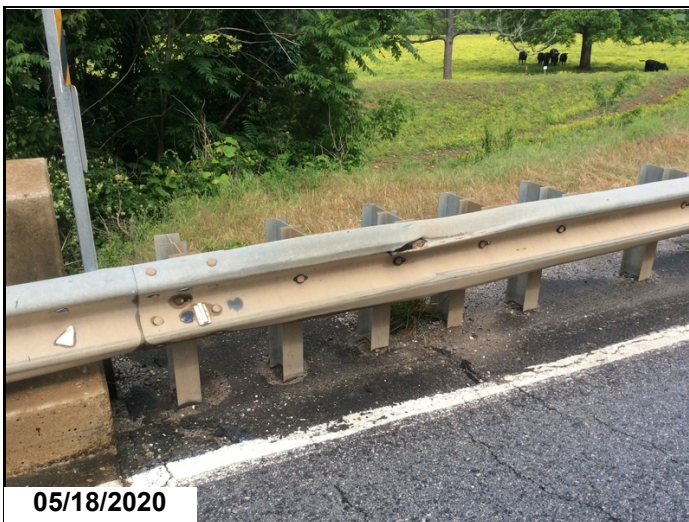
Left bridge rail @ Abutment 2. Collision damage.
