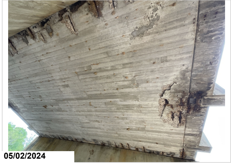
Span 3: Numerous spalls with exposed reinforcing steel section loss. CS3.
