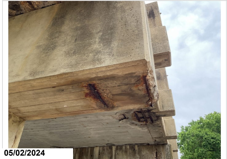
Bent 3, Bottom, Right: Spalling with exposed reinforcing steel with section loss. CS3.
