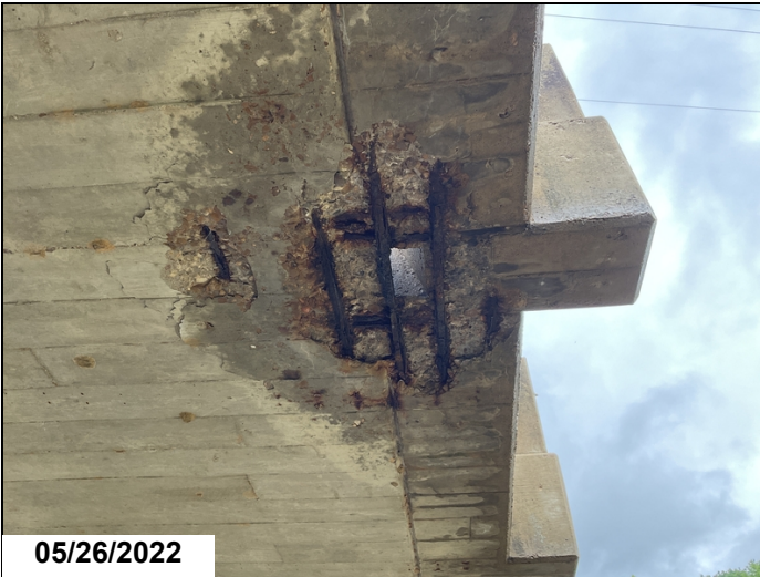
Spans 1 - 10 Spalls with corroded rebar exposed to soffit and at drain openings. Cracks / spalls to edges of deck over Bents 1 - 9
