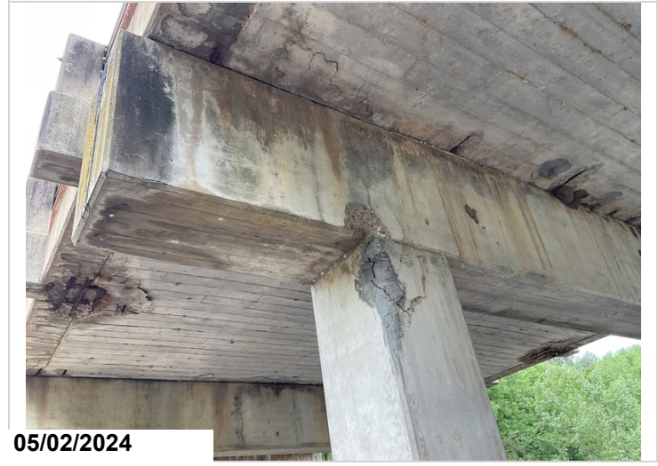
Bent 4, Ahead, adjacent to Column 2: Spalling. CS3.
