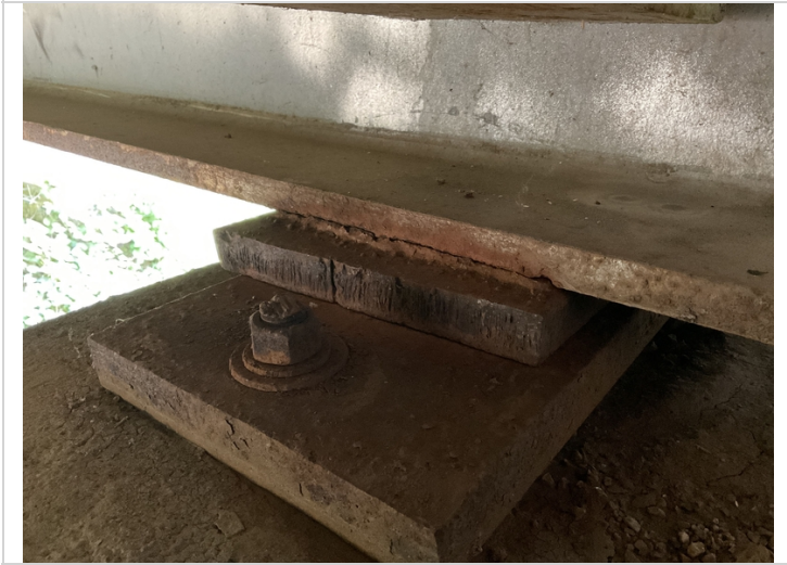
Broken weld to sole plate of bearing 2 @ end of span 1.
