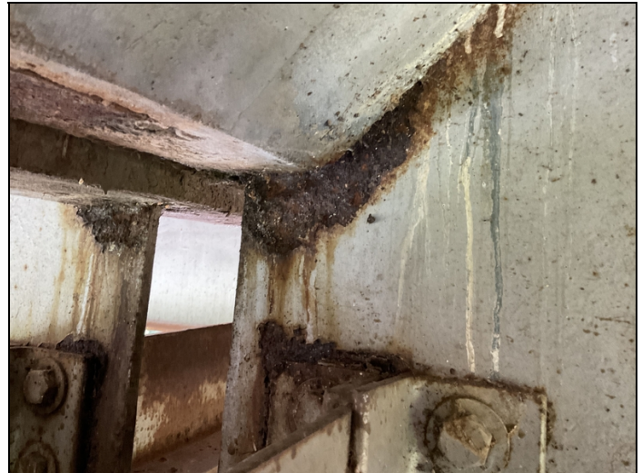
Rust and section loss, some with holes to ends of girders and bottom flange at all spans. Girder 2, end of span 2.
