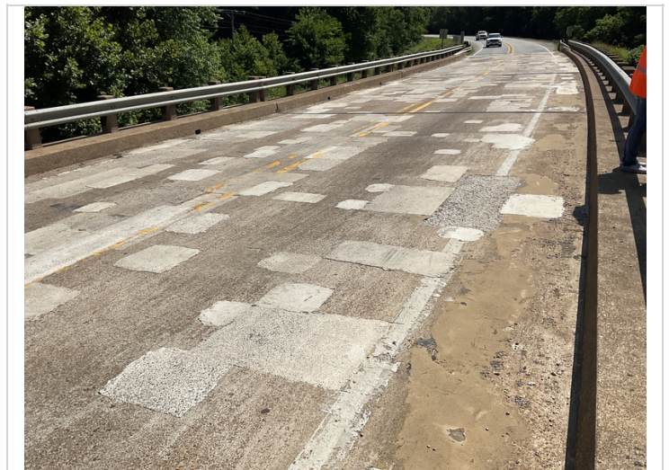
Typical patched areas to 90% of deck.
