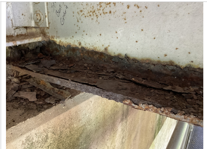
Heavy rust with section loss to bottom of web & flange to girder 2, end of span 3.
