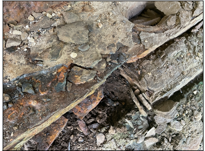
Heavy rust with section loss to girder 1 @ beginning of span 5. Holes to bottom flange on each side of web.
