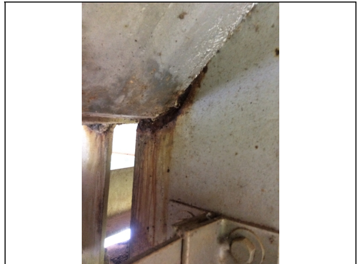
Rust and section loss, some with holes to ends of girders and bottom flange at all spans. Hole in web of Girder #4 at end of Span #2.
