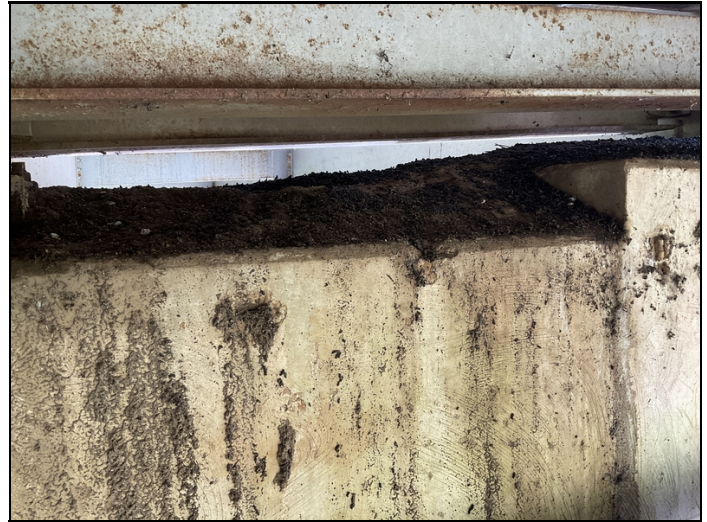
Debris on caps at all spans.
