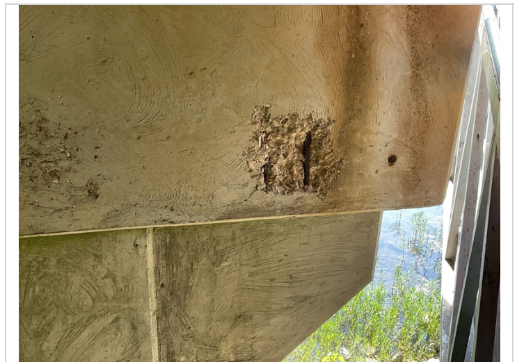
Spall with rebar exposed to rt end of cap with section loss @ backside of bent 1.
