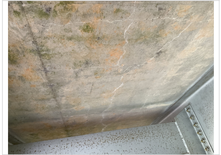
Typical efflor cracks to soffit @ all spans. Span 1
