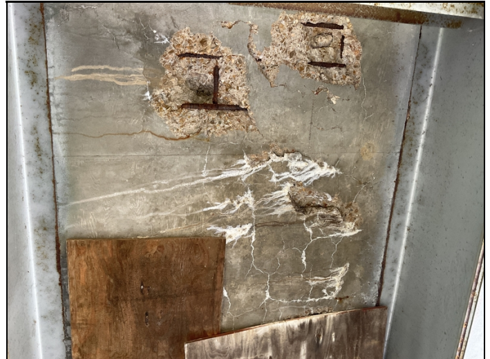
Spans #2 - #5 have spalls w/ rebar exposed, some with efflor. to soffit. Span 2, between girders 2 & 3.
