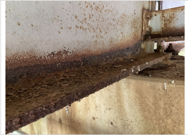
Typical rust to ends of girders @ all spans. Girder 3, end of span 2.
