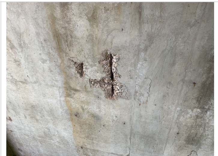
Spall with rebar exposed with section loss to pier wall @ ahead side of bent 1.
