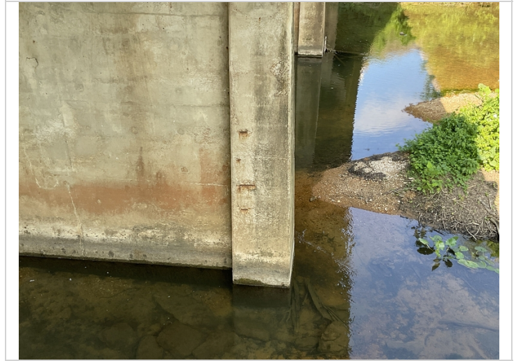
Spalls with rebar exposed to column 1 @ ahead side of bent 3.
