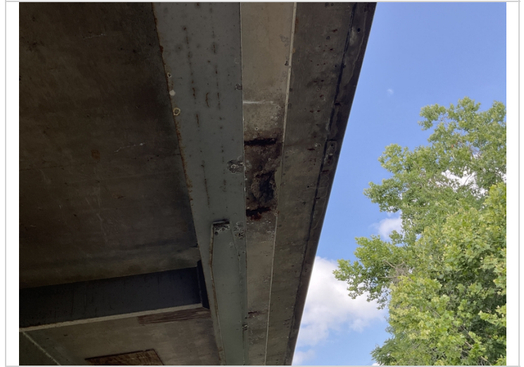
Spall with rebar exposed with section loss to Lt overhang @ span 2.
