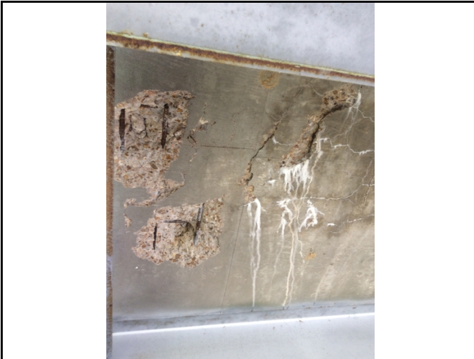
Spans #2 - #5 have spalls w/ rebar exposed, some with efflor. to soffit.
