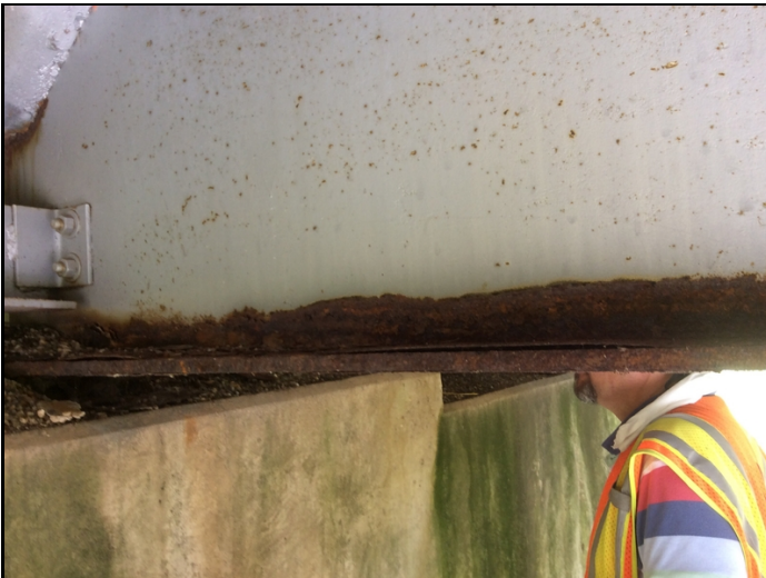
Rust and section loss to ends of girders and bottom flange at all spans.
