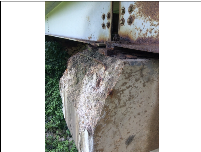
Efflor. map cracking, chemical deterioration, and spalls w/ rebar exposed to left end of cap at bent #4
