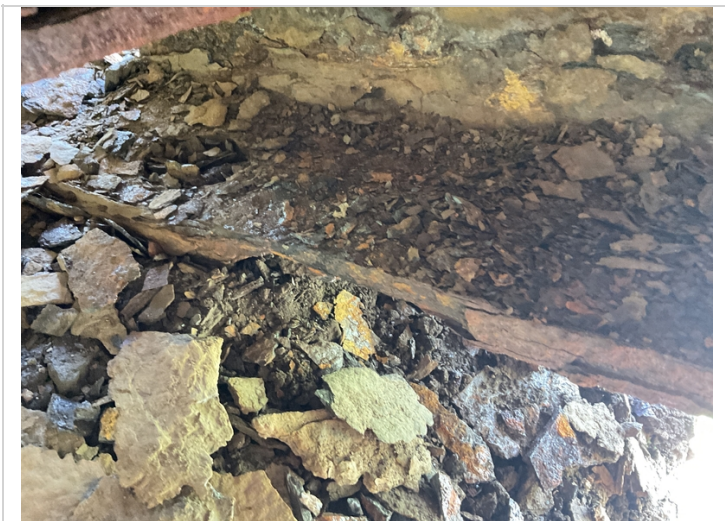
Heavy rust with section loss to girder 1 @ beginning of span 5. Holes to bottom flange on each side of web.
