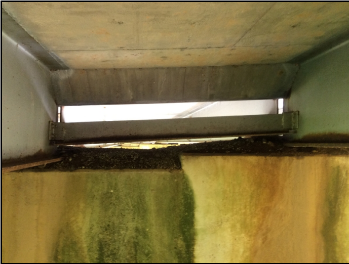
Typical debris on cap @ all spans.
