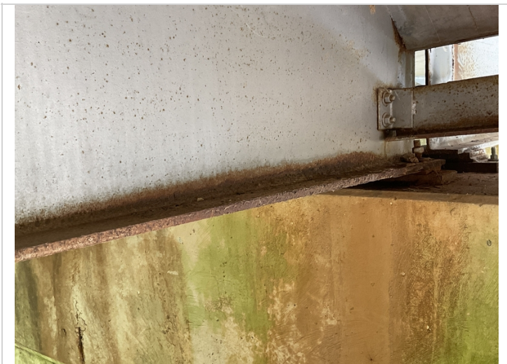
Typical rust to ends of girders @ all spans.
