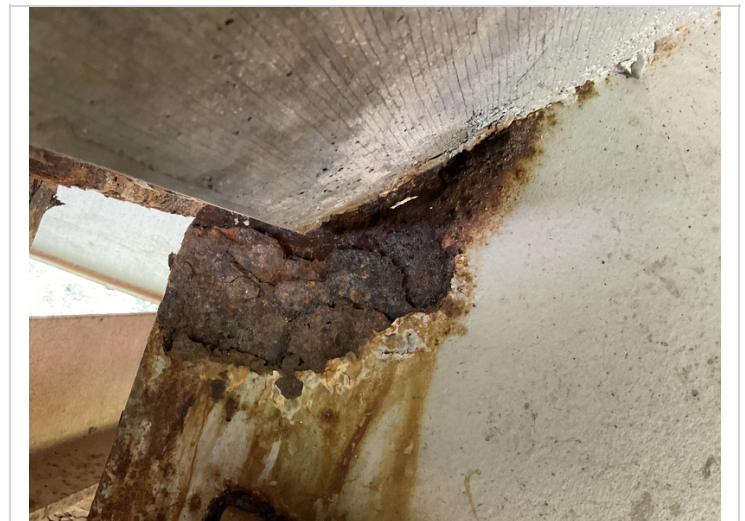
Hole in web below paving haunch @ girder 3, end of span 4.
