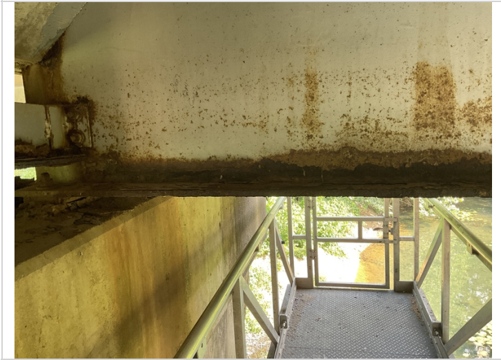
Heavy rust with section loss to girders 2 & 3 @ beginning of span 4.
