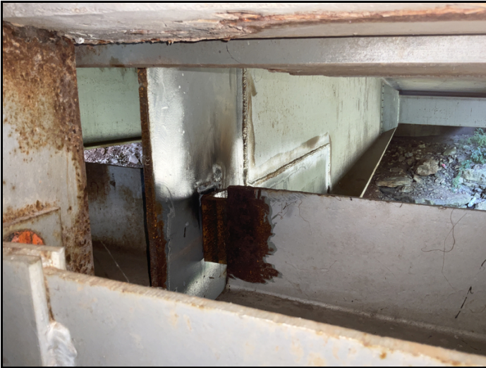
Diaphragm between Girders 1 & 2 @ end of Span 1 is not connected @ Girder 2.
