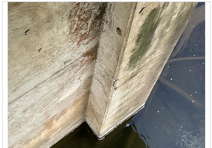
Cracking to column 1 @ ahead side of bent 2.
