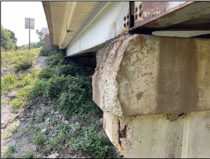
DEfflor. map cracking, chemical deterioration, and spalls w/ rebar exposed to left end of cap at bent #4
