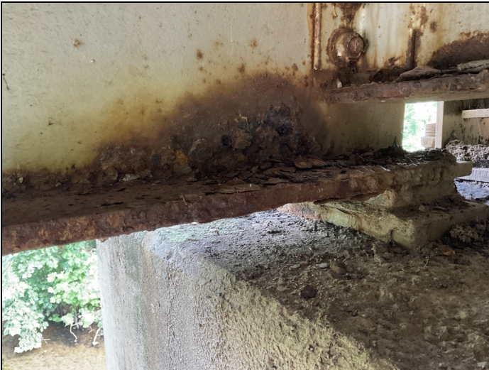
Rust and section loss, some with holes to ends of girders and bottom flange at all spans. Girder 1, end of span 2.
