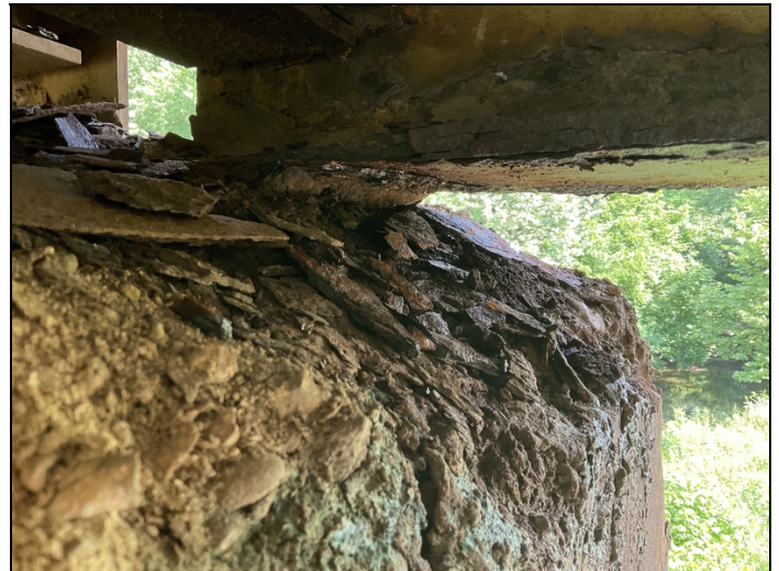
Efflor. map cracking, chemical deterioration, and spalls w/ rebar exposed & loss of bearing area to left end of cap at bent #4
