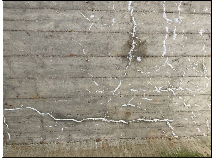
Transverse efflorescent cracks to soffit @ all Barrels. Barrel 4.
