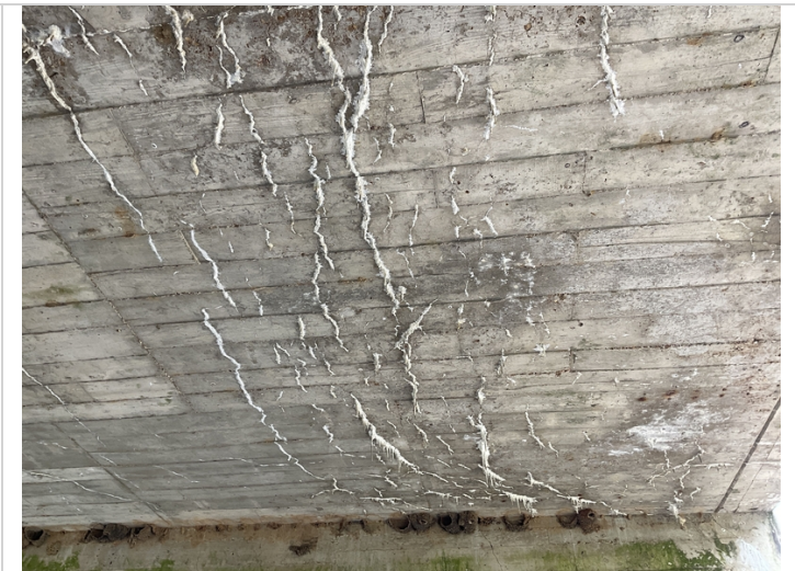
Efflor cracks to soffit @ barrel 2.
