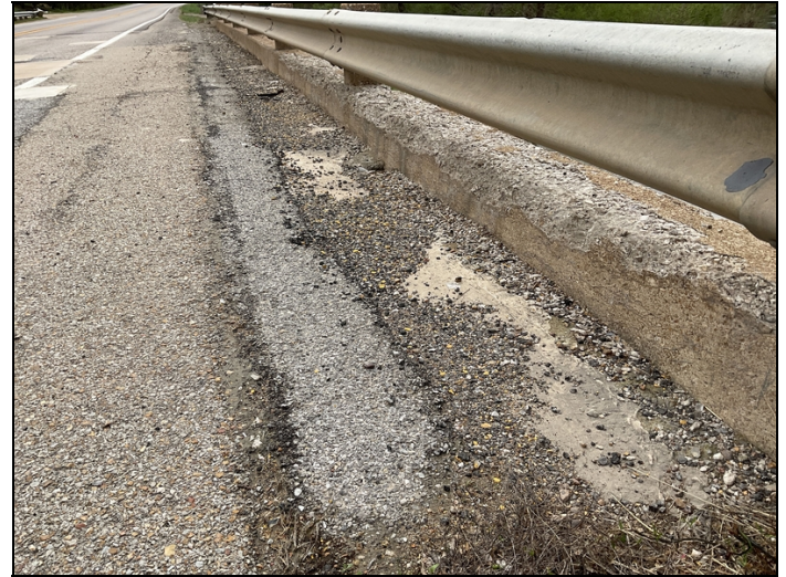
Heavy scaling, spalls & chemical deterioration to Left & Right curbs @ Barrels 1 - 4. Rt curb.
