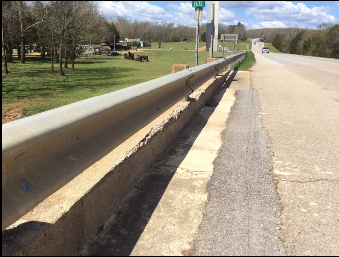
Heavy spalling to Right curb.
