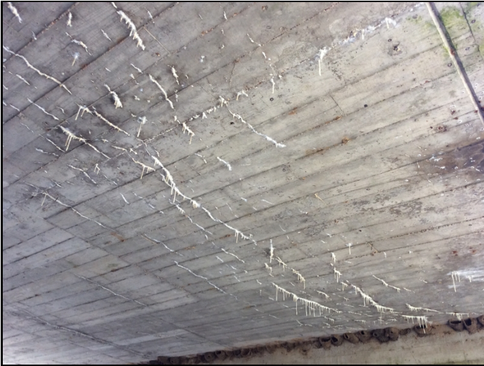
Efflorescent cracking to soffit in Barrel 3.
