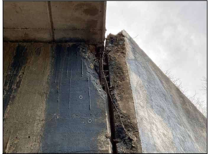
Spalls with some rebar exposed to Left & Right wings @ Abutments 1 & 2.
