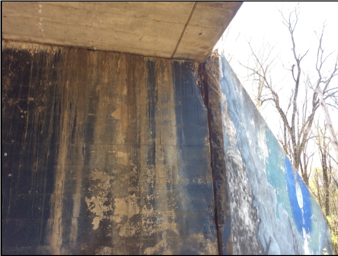
Spalls with rebar exposed to Right wing @ Abutment 2.
