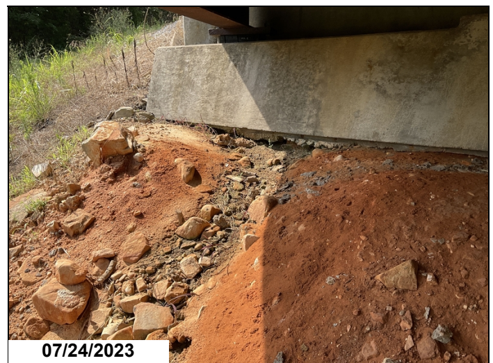
Minor scouring to Abutments 1 & 2 on Rt ends. Abutment 1.
