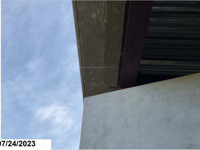
Efflor cracks to Lt & Rt overhangs.
