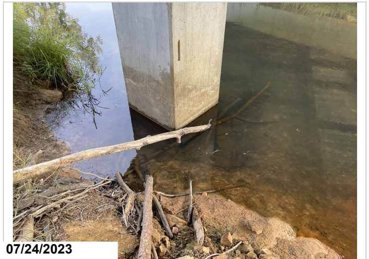
Local scour @ Columns 1 & 2 @ Bent 1.
