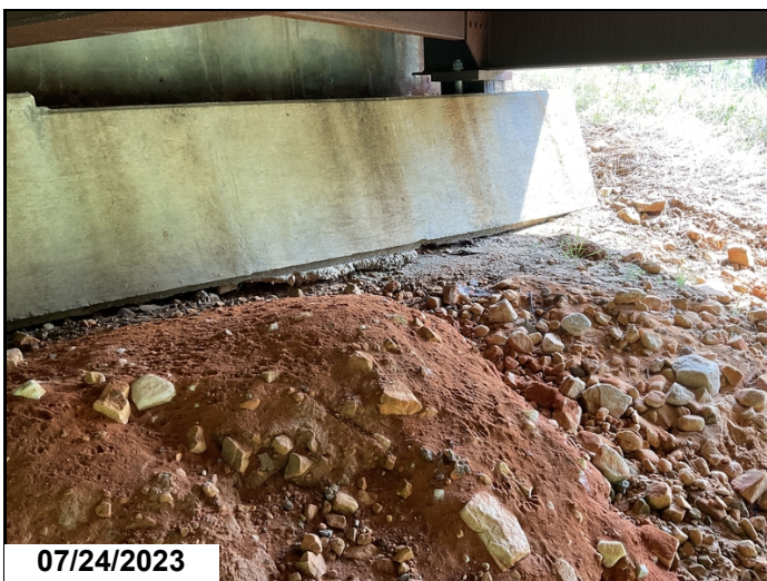
Minor scouring to Abutments 1 & 2 on Rt ends. Abutment 2.
