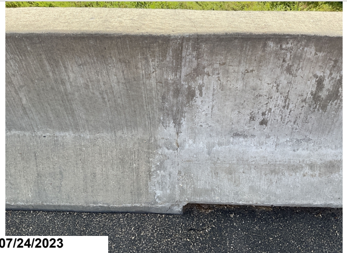
Typical cracks to Lt & Rt parapet wall.
