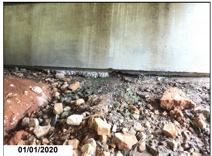
Minor erosion to Rt. end of Abutment 2
