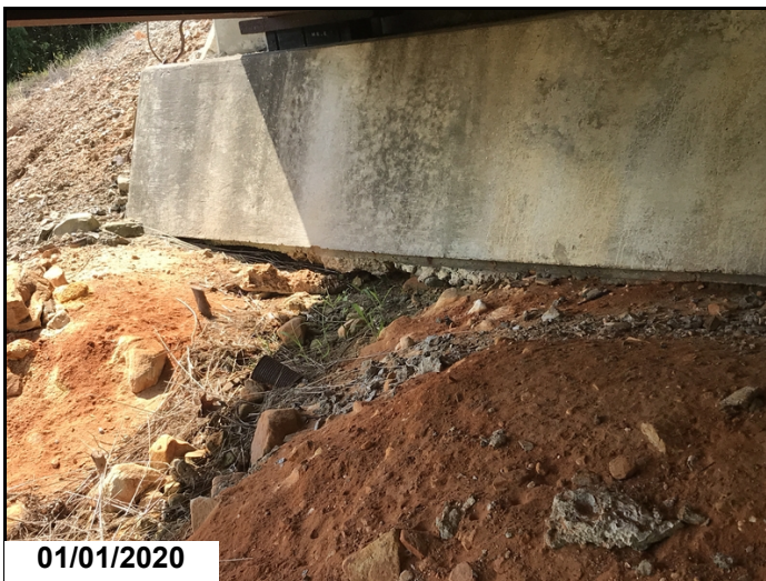
Minor erosion to Rt ends @ abutments 1.
