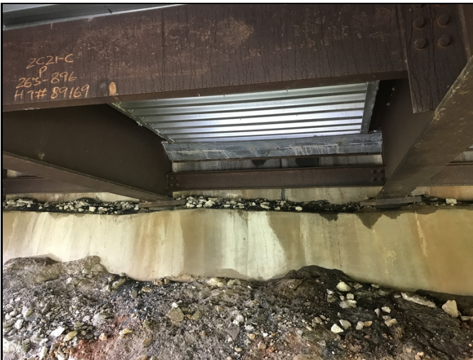
Heavy debris on cap @ Abutment 1.
