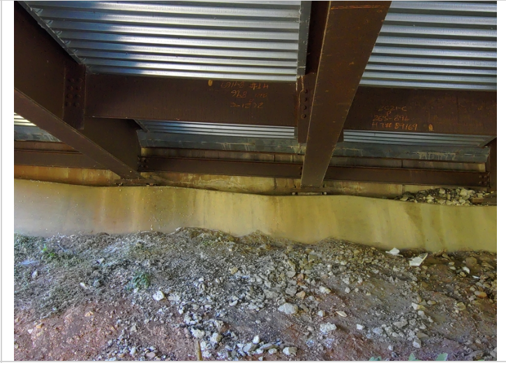
Efflor cracks @ abutment 1.
