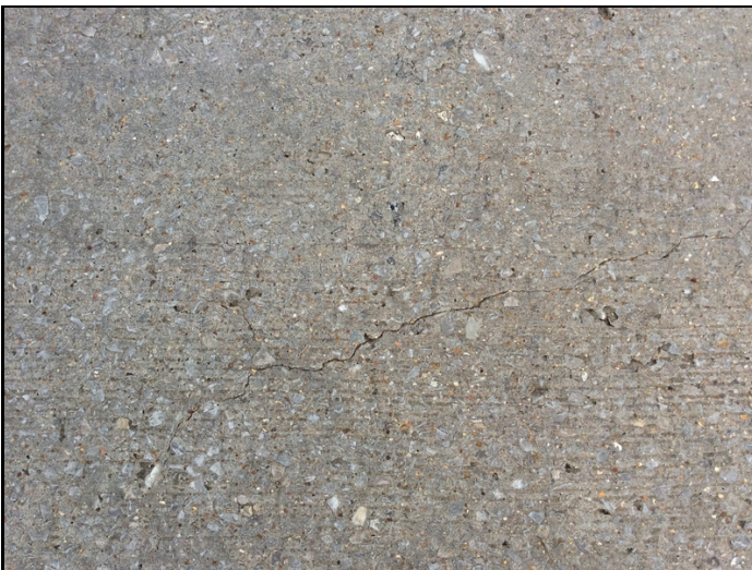
Transverse cracking to deck @ Span 1.
