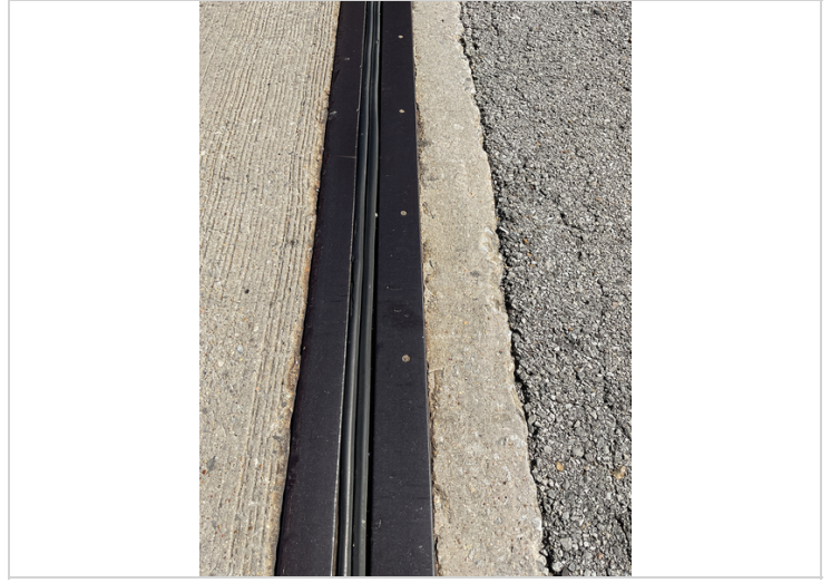
Cracking/tear to joint seal @ Abut. 2.
