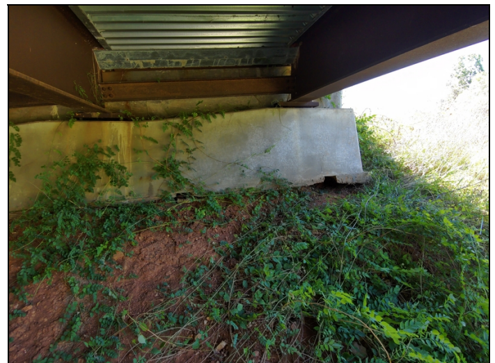
Abutment 2 has erosion to Left and Right ends. Right side.
