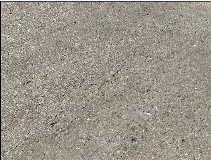
Deck at all spans Few longitudinal and transverse unsealed cracks.
