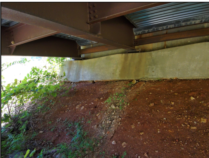
Abutment 2 has erosion to Left and Right ends. Left side.
