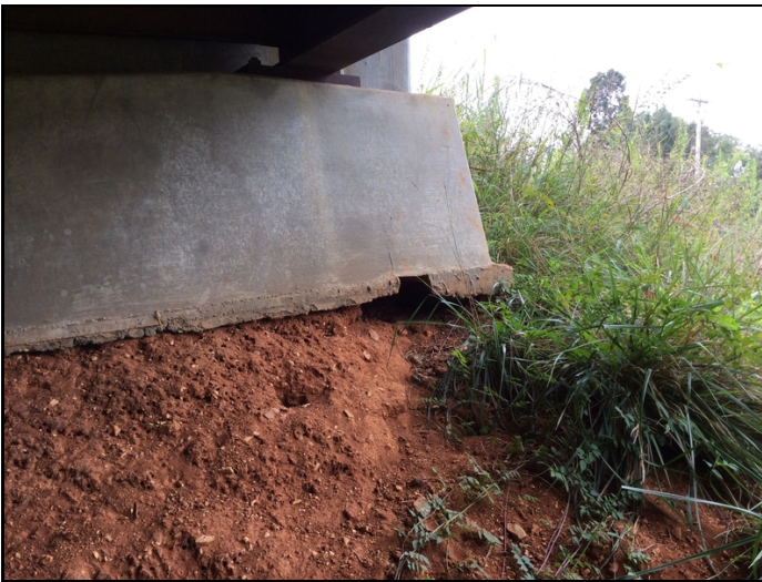
Scour to Right end of Abutment 2.
