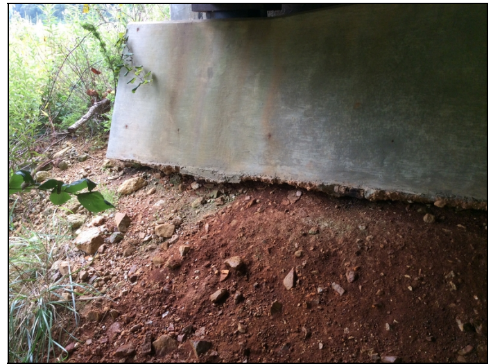
Scour to Left end of Abutment 2.
