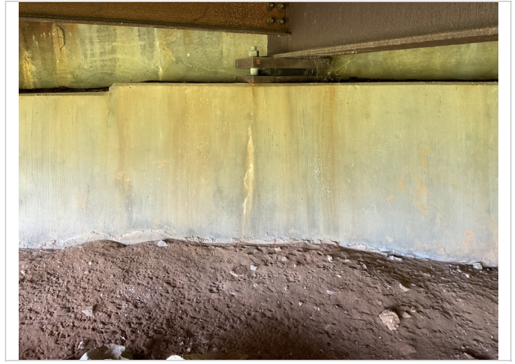
Typical efflor cracks to @ abutment 1 & 2.
