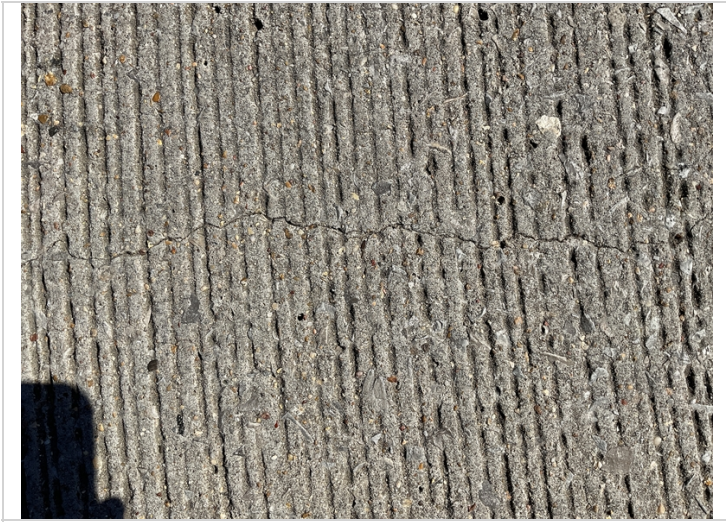
Typical cracks to deck @ all spans.
