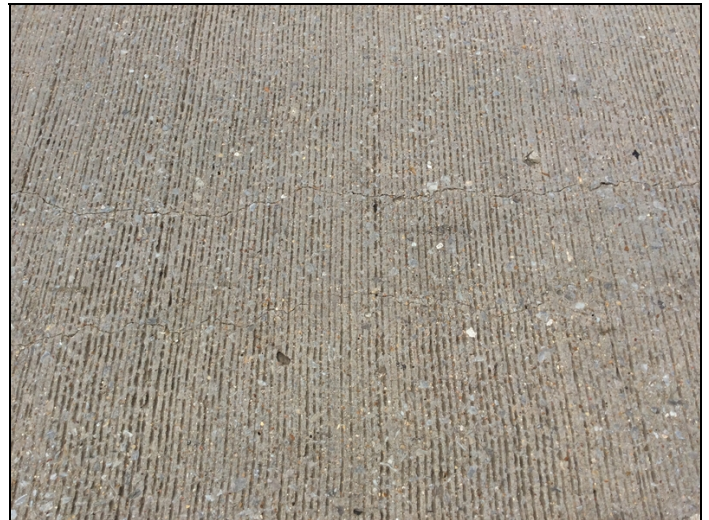
Longitudinal cracking to deck @ Span 1.
