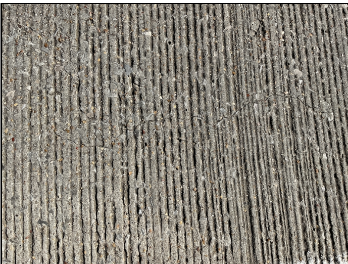
Deck at all Spans Several longitudinal and a few transverse unsealed cracks.
