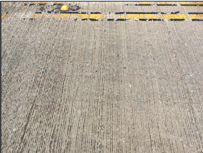
Transverse @ longitudinal cracking to deck @ Span 2.
