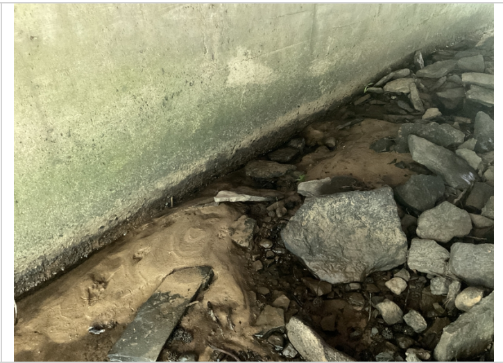
Typical abrasion to bottom of walls @ all barrels.
