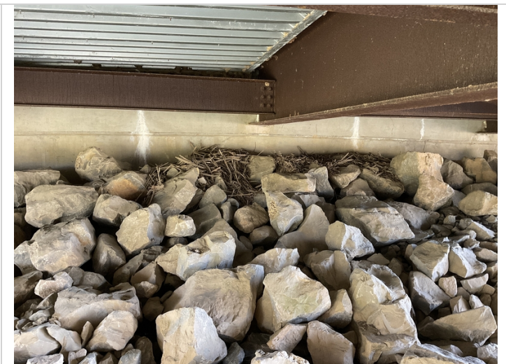
Typical efflor cracks to abutments 1 & 2.
