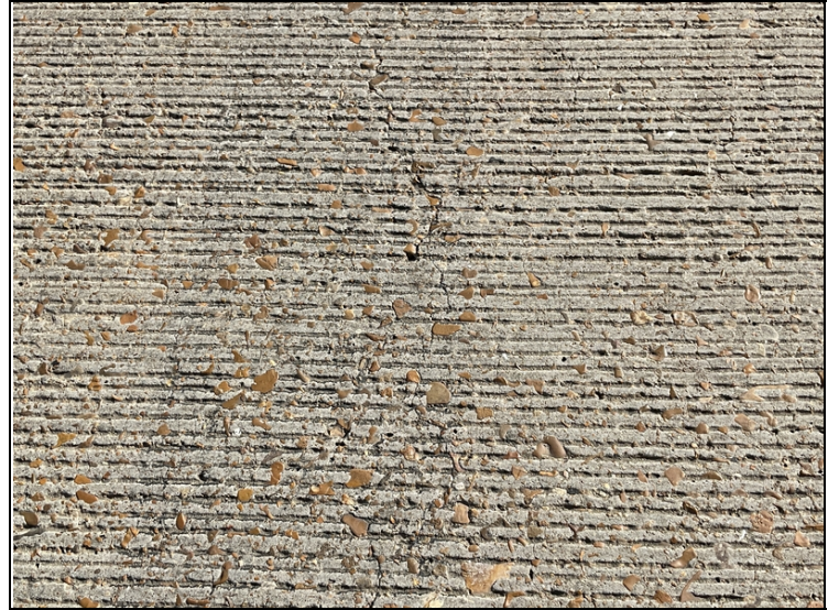
Unsealed cracks to deck @ Spans 1 - 3.
