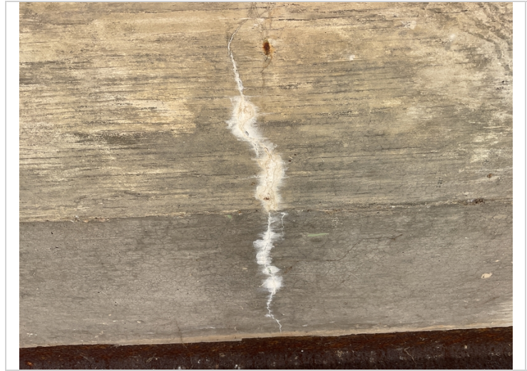
Typical efflor cracks to Lt & Rt overhangs.
