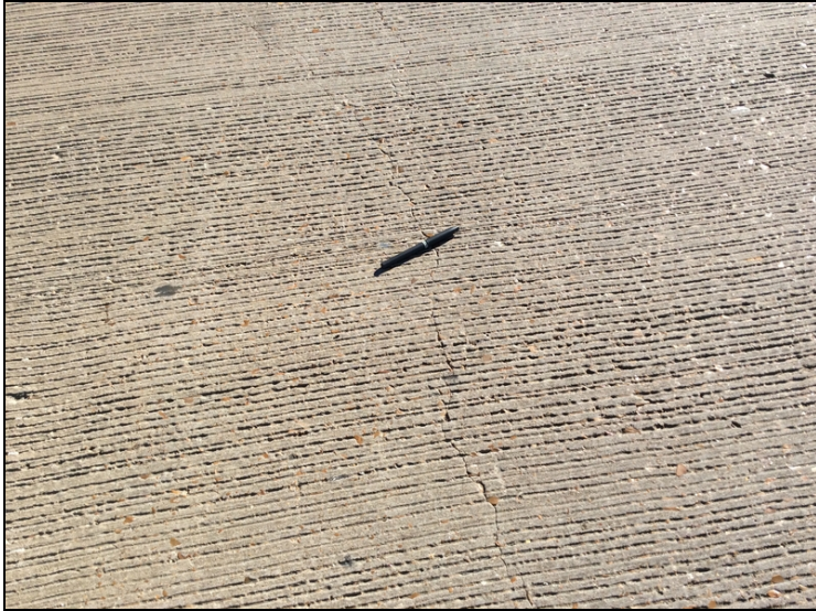
Typical deck cracking.
