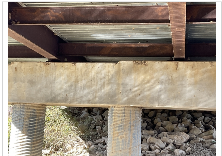
Minor spalls to ahead side of cap @ bent 1.
