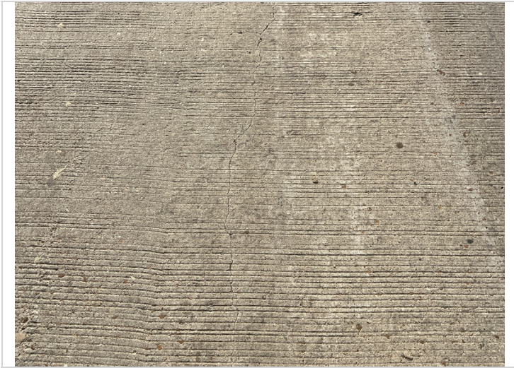
Typical cracks to deck @ all spans.
