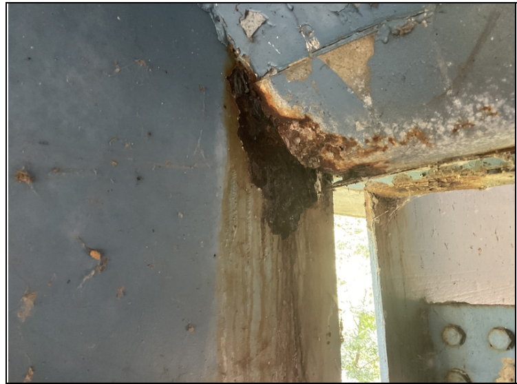
Rust with section loss to ends of girders at Spans 13, 17, 21 & 22. Girder 1, bent 13.
