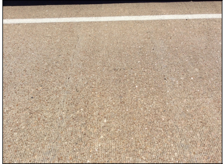
Unsealed transverse cracking to deck @ Span 8.
