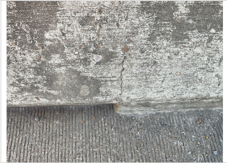
Typical vertical cracks to parapet wall.
