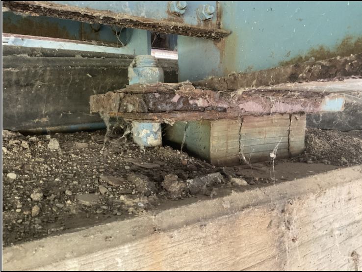
Rust to bearings and sole plates. Girder 3, bent 13.
