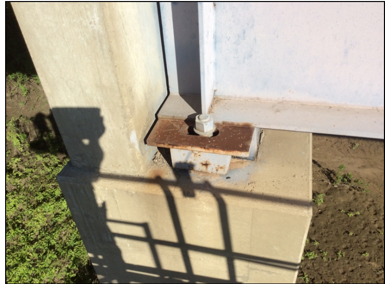
Rust to sole plate of Bearing 4 @ Bent 5 ahead.
