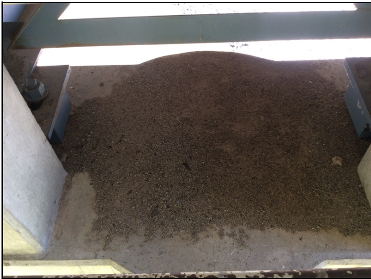
Debris on Cap @ Bent 5.
