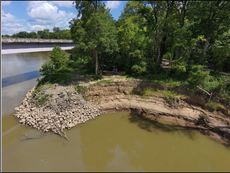
Erosion to rip rap repair.
