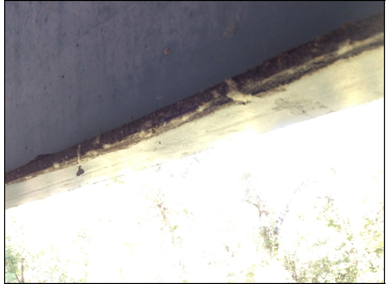
Rust with section loss to bottom flange of Girder 1 @ Span 13.
