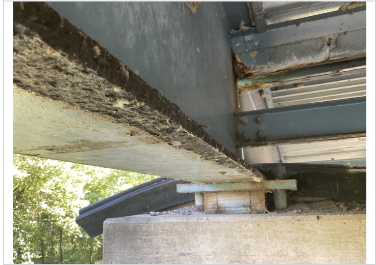
Areas of peeling paint to ends of girders 1 - 4 @ bent 13.
