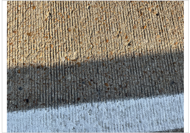
Typical cracks to deck.
