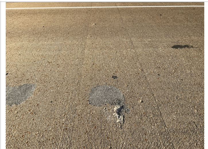
Few minor spalls with no rebar throughout deck.
