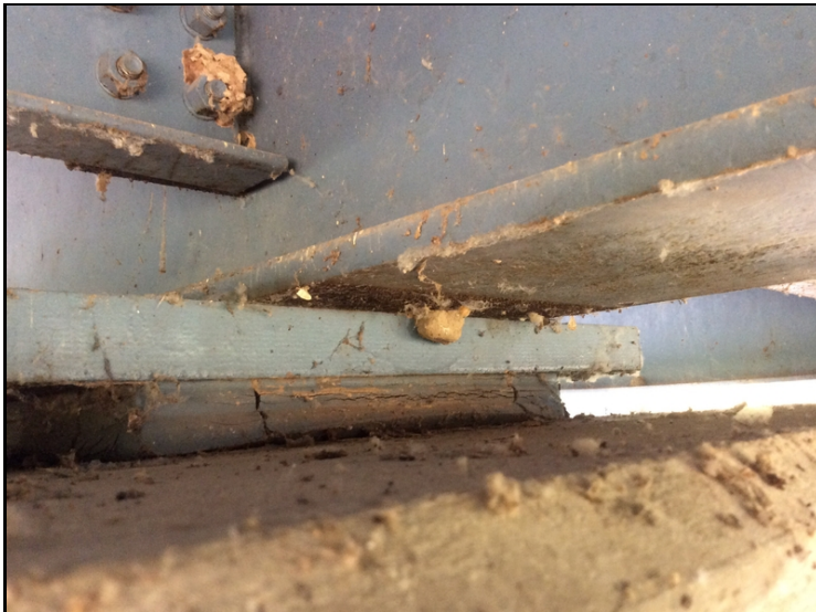
Surface rust to bottom of Girder 3 @ Bent 2.
