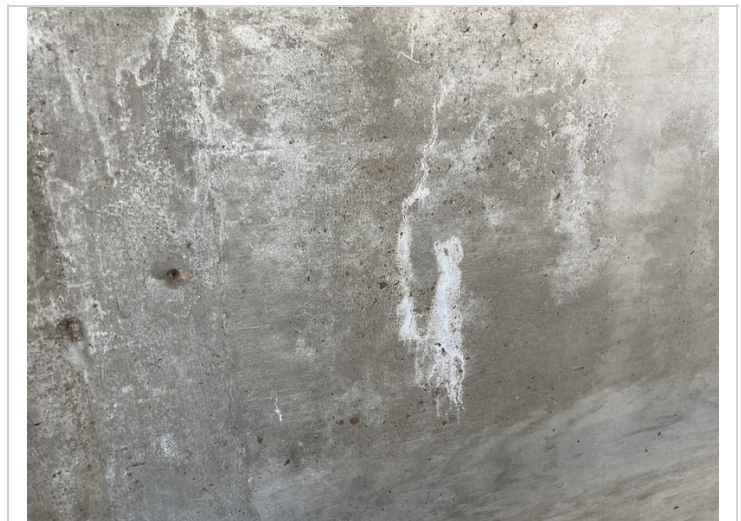
Efflor crack to back side of back @ bent 8.
