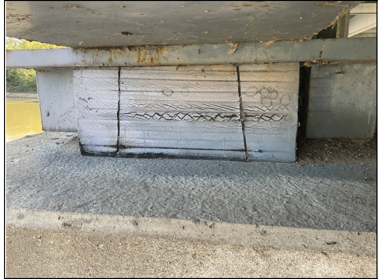
Cracks and deterioration to Elastomeric Bearings. Girder 1, bent 8.
