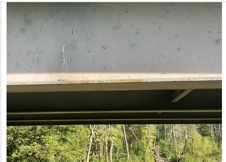
Typical Rust to bottom flange of girders.
