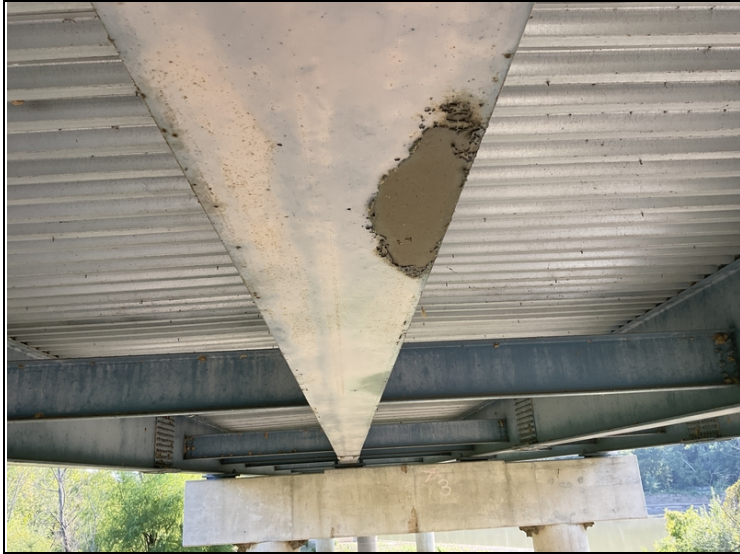
Paint is peeling with areas of surface rust on Girders at most spans.
