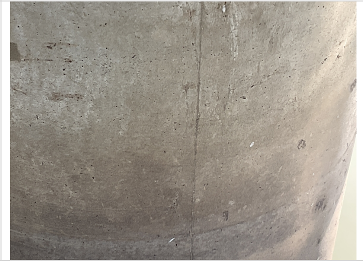
Cracking to column @ bent 7.
