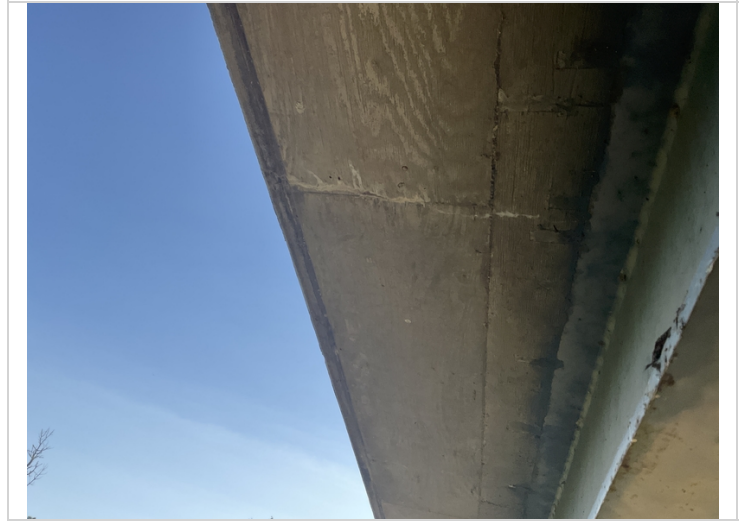
Typical cracks to Lt & Rt overhangs.
