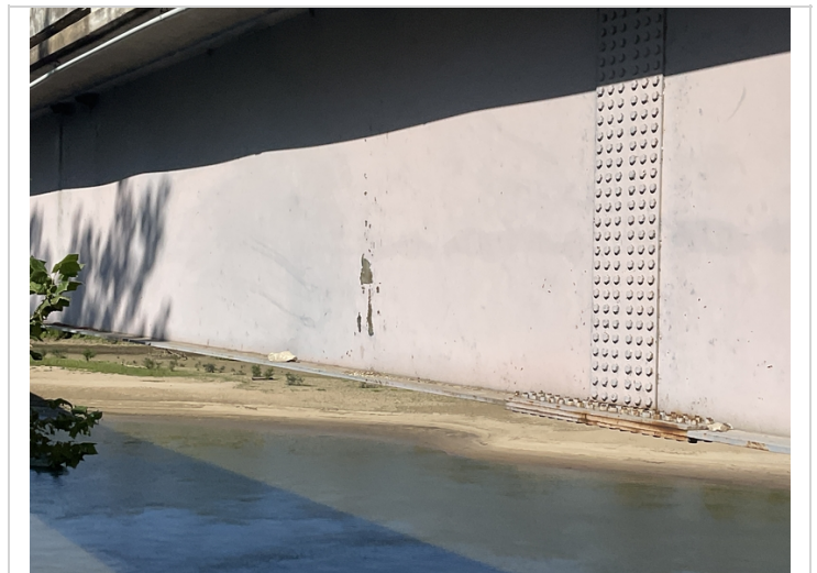
Peeling paint to outside of girder 4 @ span 8.
