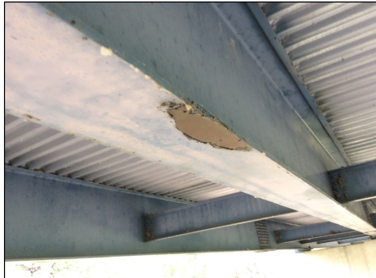
Peeling paint to bottom of Girder 2 @ Span 3.
