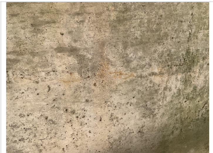
Rust stain crack to backside of cap @ bent 21.
