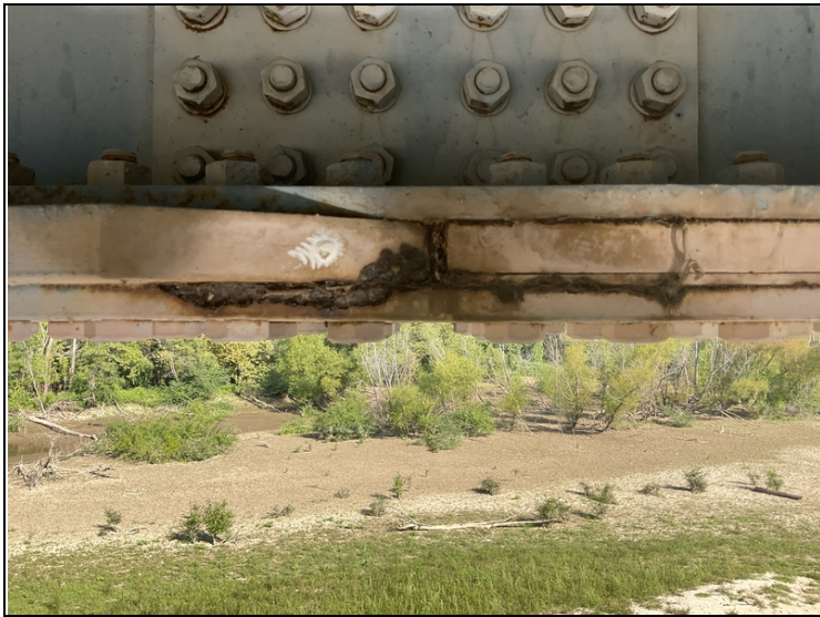
Pack Rust developing at bottom splice plates. Girder 1 & 4, first splice plate @ span 7.
