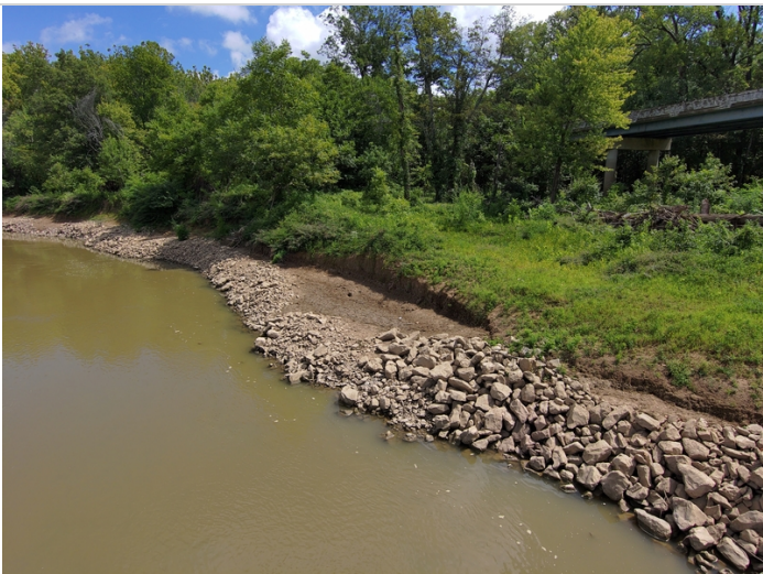
Typical Rip Rap repair made in the past. Up stream & down photos.
