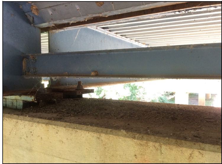
Debris on Cap @ Bent 17.
