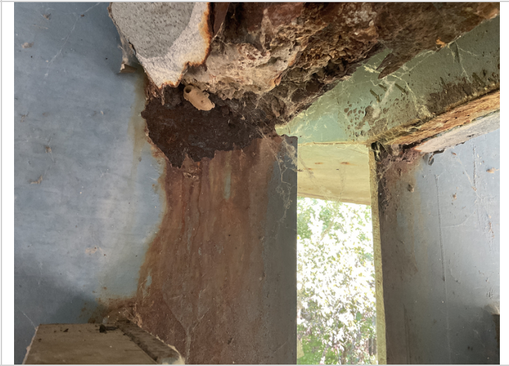
Hole to web, below paving haunch to girder 1 @ end of span 17.
