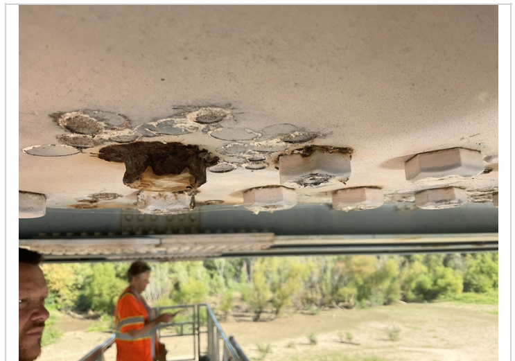
Rust to bolt @ first splice plate to girder 4, span 7.
