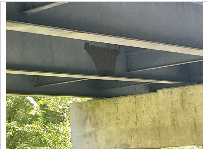
Peeling paint to end of girder 2 @ end of span 14.
