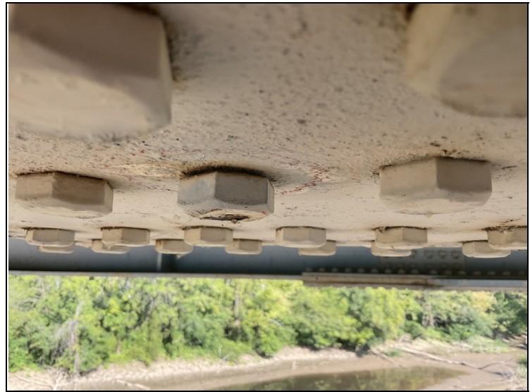
Loose bolt at field splice on Girder 2 at Span 6.
