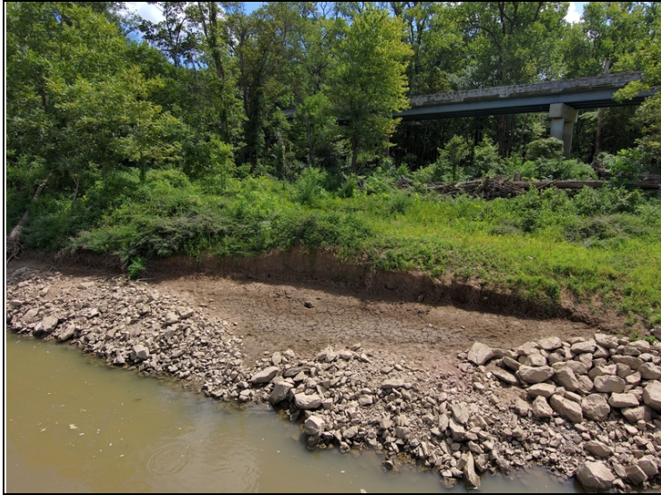
Erosion to rip rap repair.
