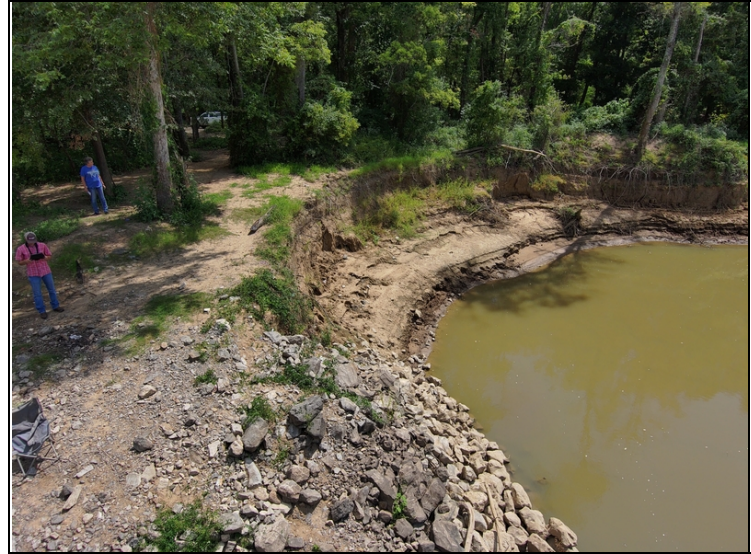
Erosion to rip rap repair.
