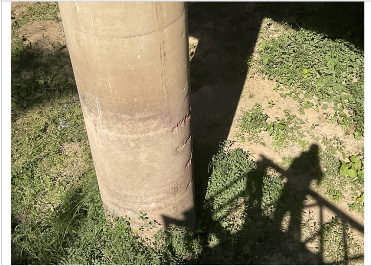
Spalls with rebar exposed to column 2 @ bent 17.
