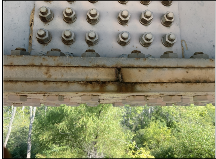
Pack Rust developing at bottom splice plates.
