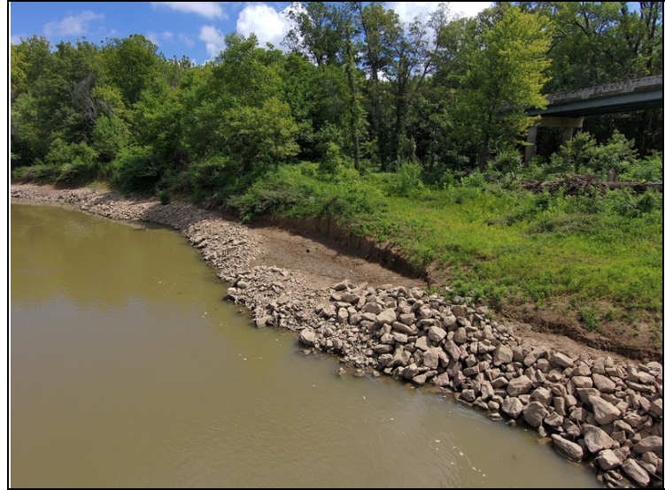
Erosion to rip rap repair.
