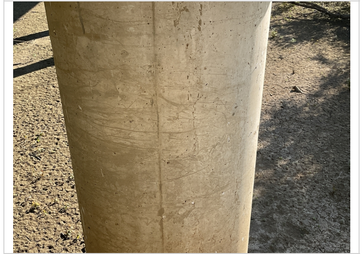
Vertical crack to column 2, backside of bent 2.
