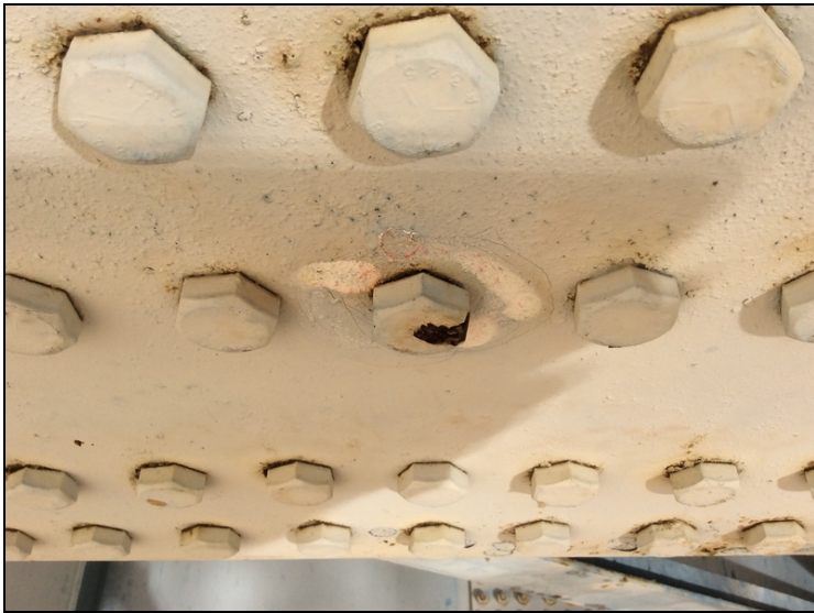
Loose bolt @ 2nd field splice @ Girder 2 Span 6.
