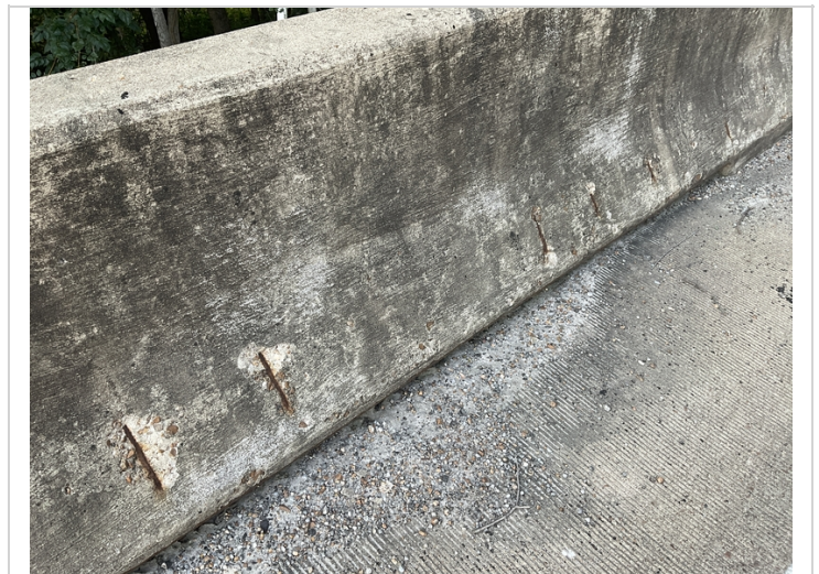
Typical spalls with rebar exposed to parapet wall.
