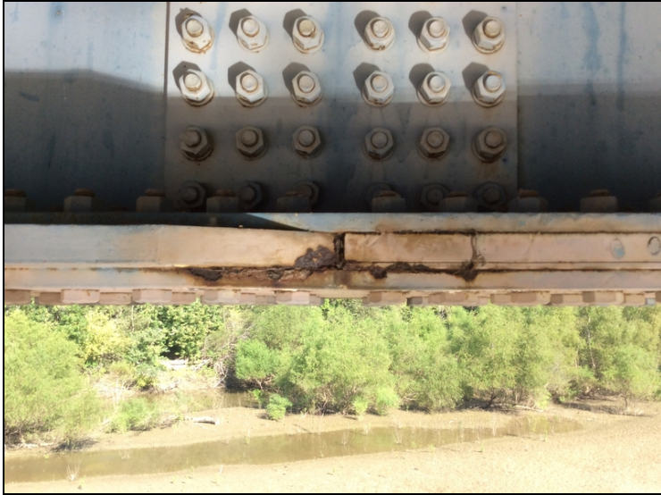
Pack rust to bottom of 1st splice plate @ Girder 1 Span 7.
