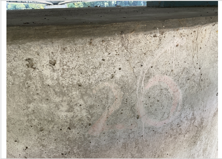
Cracking to backside of bent 6.
