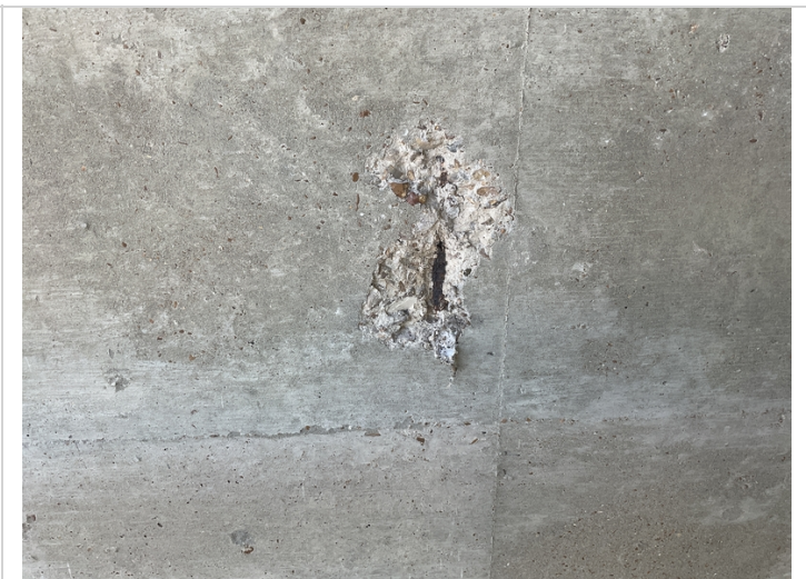
Spall with rebar exposed to back side of cap @ bent 8.
