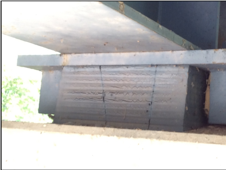
Cracking to Bearing 3 ahead @ Bent 5.
