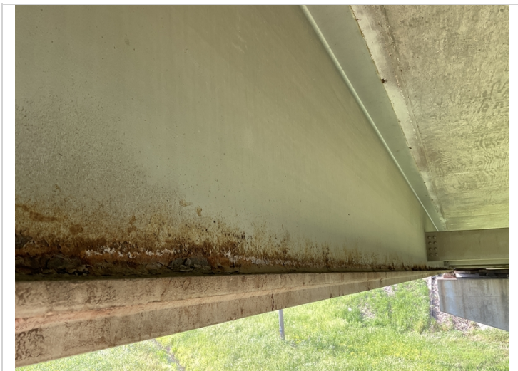
Typical Freckled to bottom flanges @ all girders.
