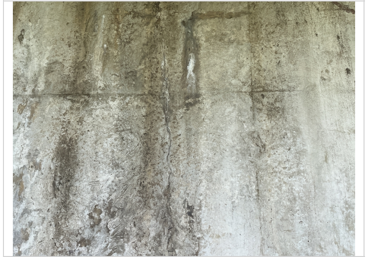
Vertical efflorescent cracking to ahead side of cap @ Bent 5.
