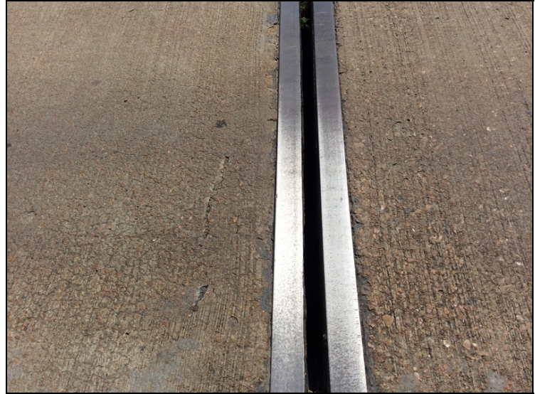
Compression joint seal is missing @ Bent 1.
