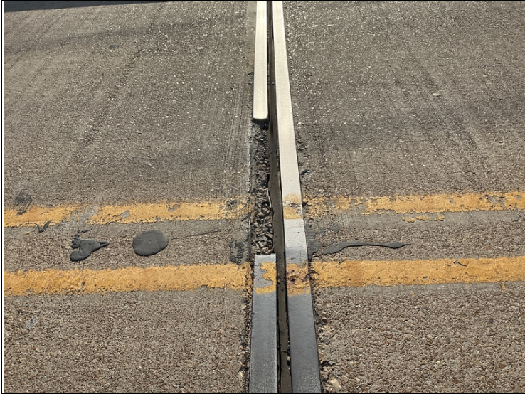
Bent 2 - Road iron on back side of joint is broke and pulled out of place at center line. Repaired.
