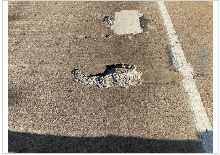
Spalls with no rebar exposed @ span 8.
