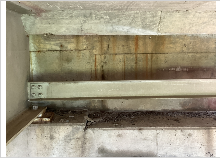
Efflor cracks to back wall @ abutment 1.
