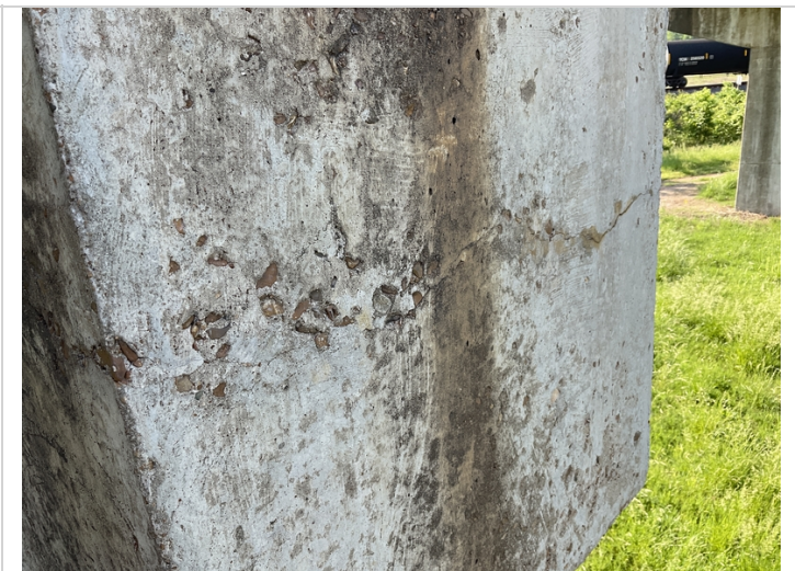
Horizontal crack to right side of cap @ bent 1.
