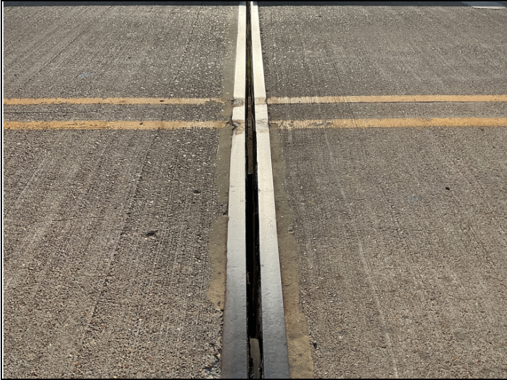
Joint seals are cracked, deteriorated, and leak. Joints have failed at Bents 1, 5 and 6. Bent 5.
