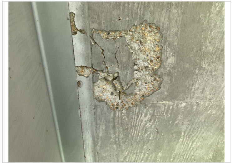
Spall to soffit between girders 2 & 3 @ span 6.
