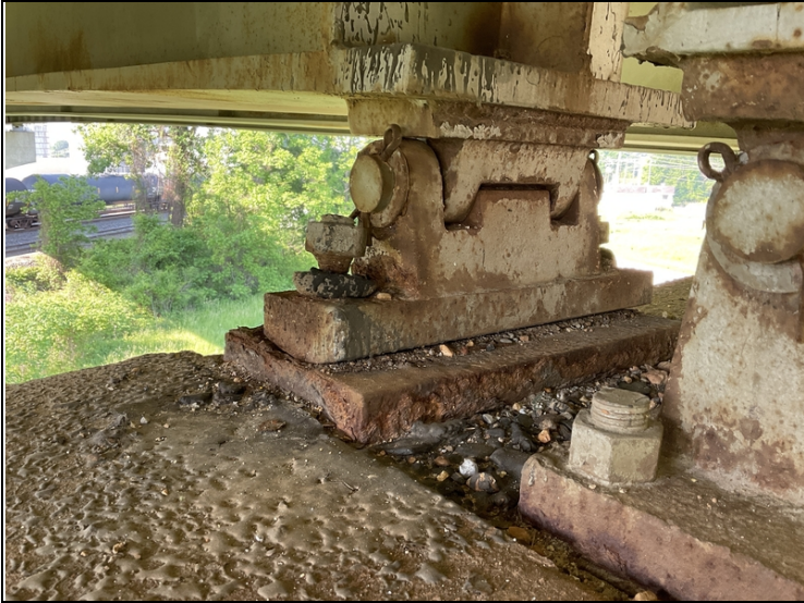
All bearings Rust and corrosion to all bearings
