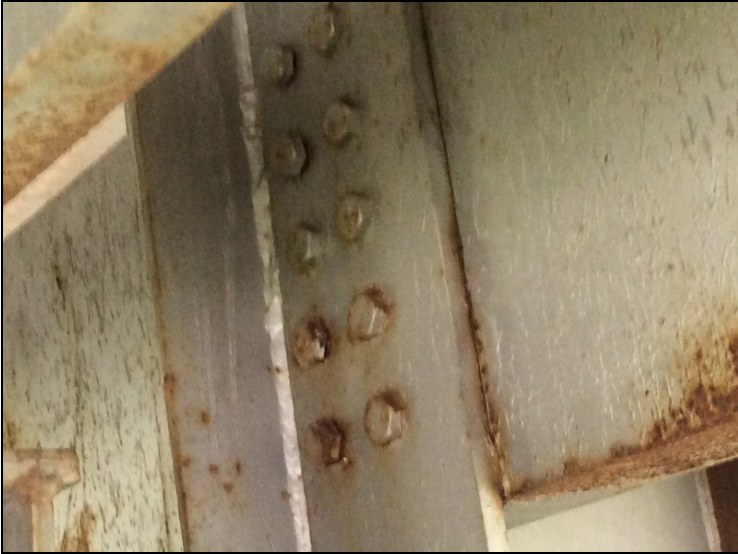
Loose bolts @ Diaphragm connection @ Girder 2 @ BOS 3.
