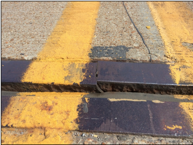
Road iron on back side of joint at Bent 2 broke and pulled out of place at center line.
