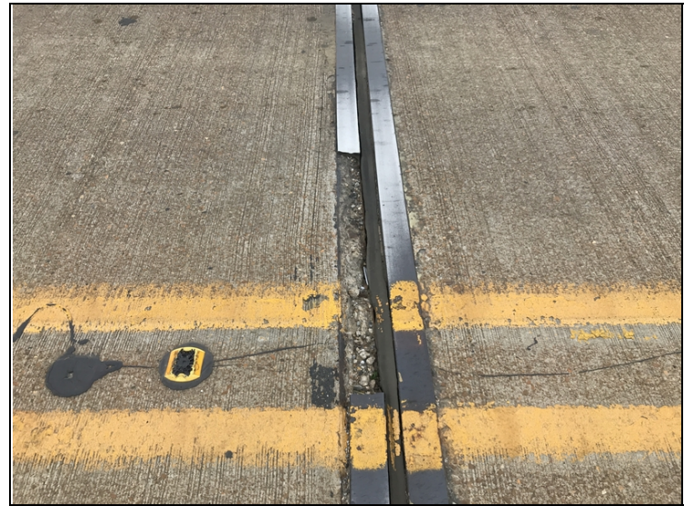
Bent road iron has been removed. (Remove maintenance need)
