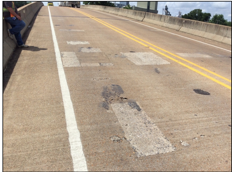
Spalls & delaminated areas to deck @ Span 1.
