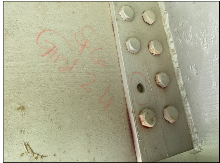
Span 6, 4th diaphragm connection between girders 1 & 2 has missing bolt.
