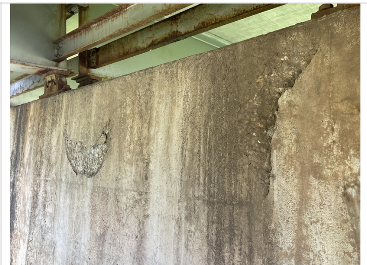
Large spalls to backside of cap @ bent 1.
