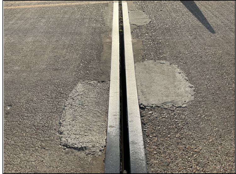
Joint seals are cracked, deteriorated, and leak. Joints have failed at Bents 1, 5 and 6. Bent 1.
