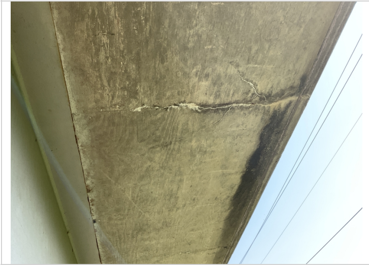
Typical efflor cracks to Lt & Rt overhangs.
