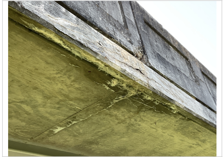
Efflor map cracking to rt overhang @ span 2.
