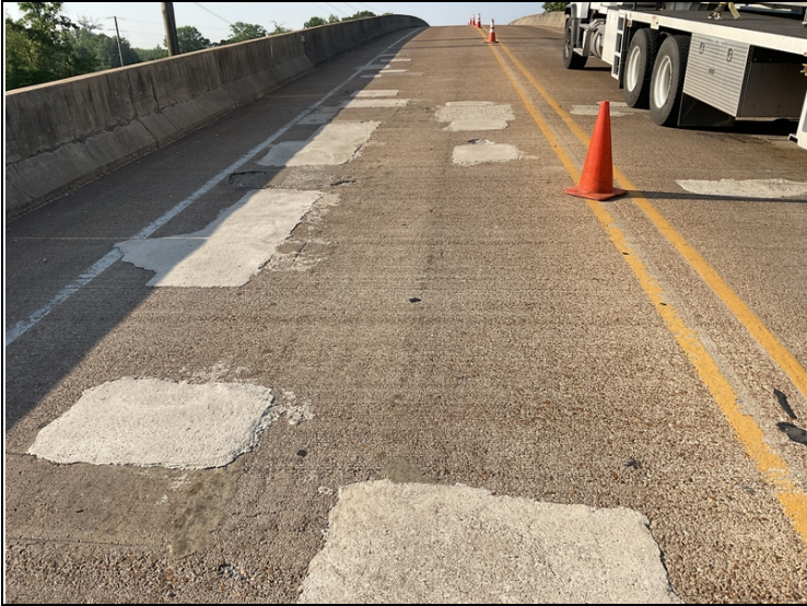
Spans 1 - 8 Spalls and delaminated areas to deck.
