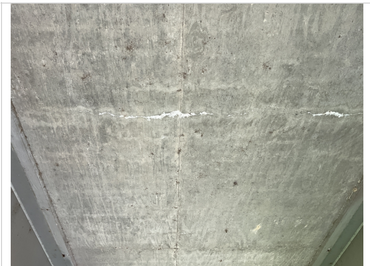
Typical efflor cracks to soffit @ all spans.
