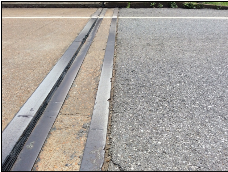
Minor Approach roadway settlement @ Abutment 2.
