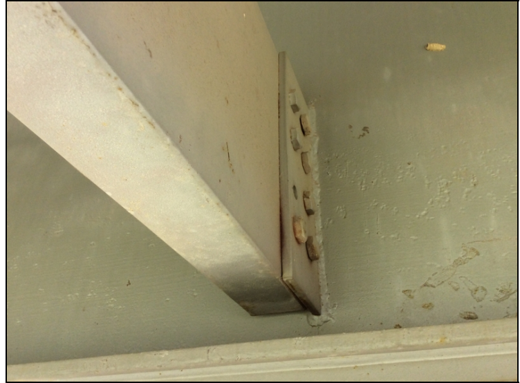
Loose bolts @ 3rd diaphragm connection between Girders 1 & 2 @ Span 6.
