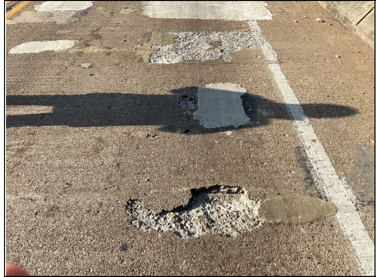
Spans 1 - 8 Spalls and delaminated areas to deck. Span 8.
