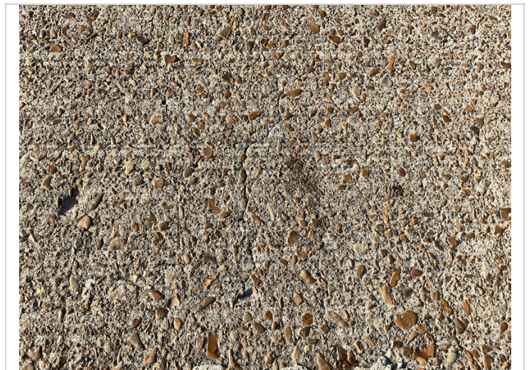
Typical cracks to deck @ all spans.
