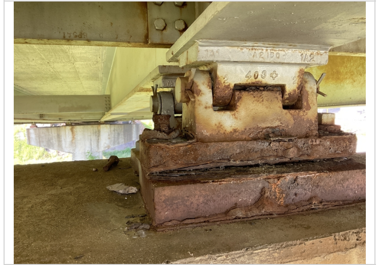
Missing bolt @ Moveable Bearing 3 @ Bent 6.
