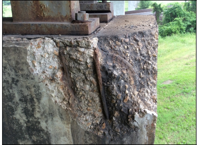
Deep spall with rebar exposed to top of Cap @ Bent 2. Right side.
