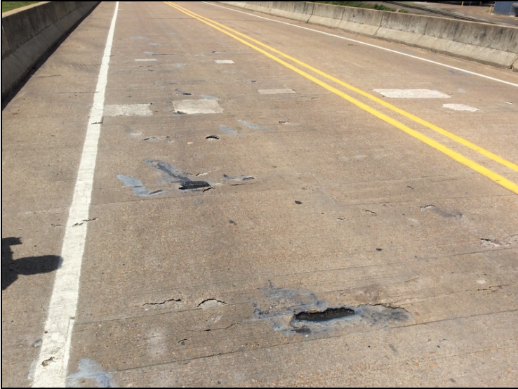
Spalls & delaminated areas to deck @ Span 6 Left lane.
