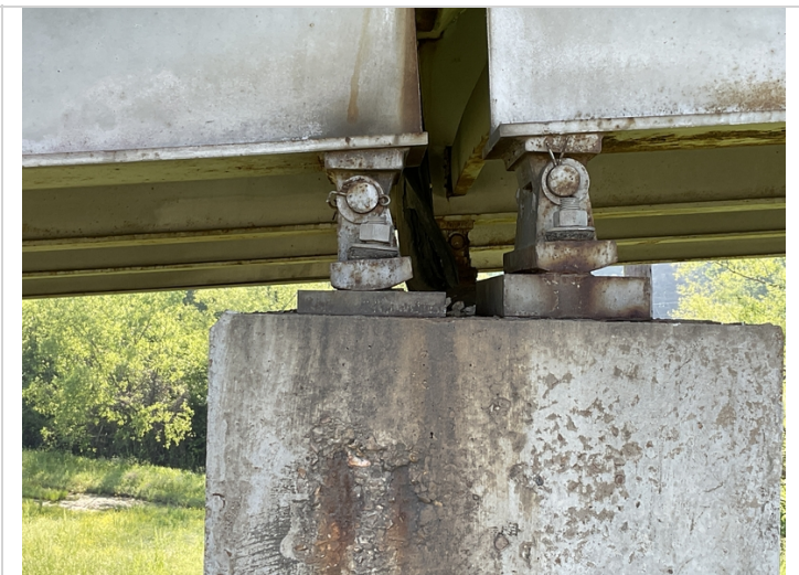
Moveable bearings have rotated back @ bent 1.
