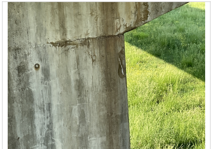
Efflor crack to column @ backside of bent 1.
