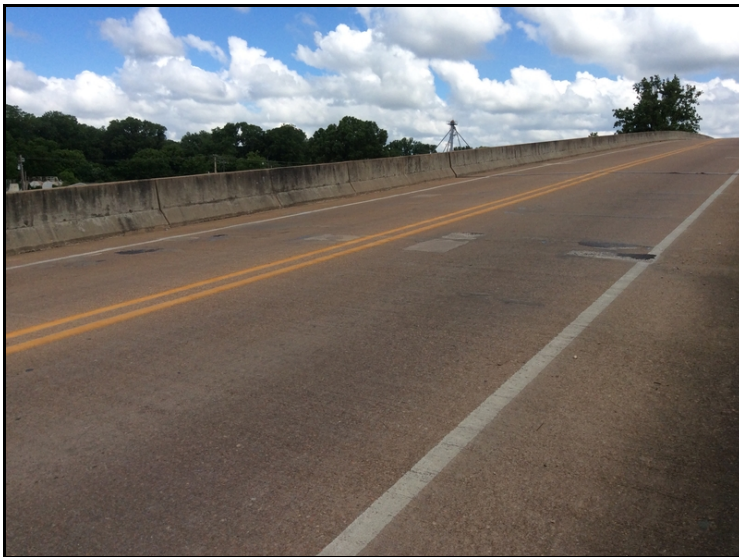
Span 8 - 10 ' of Spalls exposed to deck with no rebar exposed.
