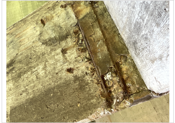
Spall with rebar exposed bottom rt side of cap @ bent 1.
