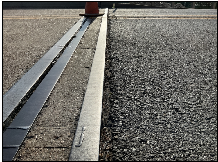
Approach roadways have minor settlement @ Abutments 1 and 2. Abutment 2.
