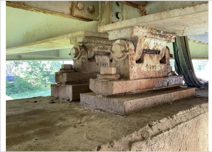
Typical rust with section loss to bearings @ all bents
