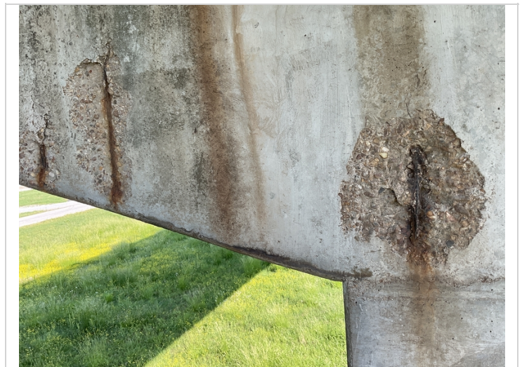
Spalls with rebar exposed to backside of cap @ bent 2.
