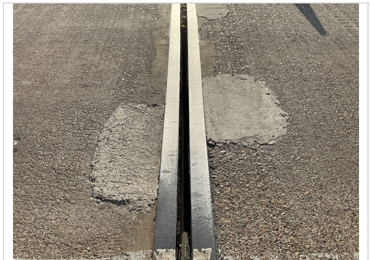
10' of compression joint seal missing @ bent 1.
