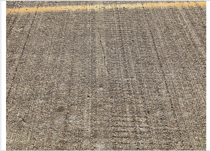
Typical cracks to deck @ all spans.
