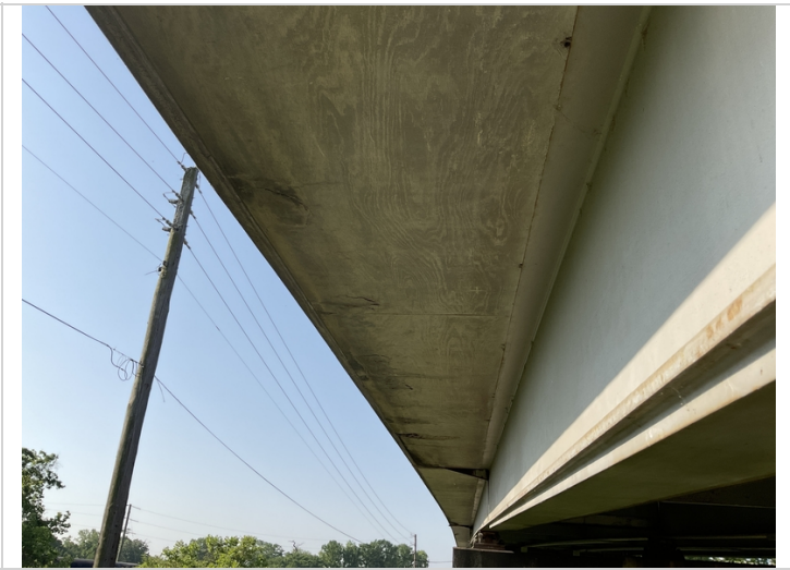
Few minor delays to rt overhang @ span 1.
