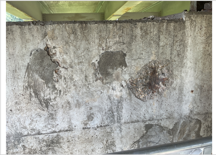
Spall to backside of cap with rebar exposed @ bent 4.
