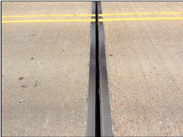
Pourable joint seal @ Bent 5.
