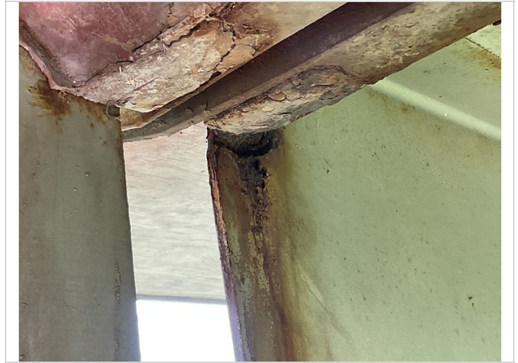
Corrosion to ends of girders @ all spans.
