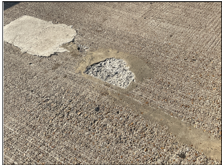
Spans 1, 2, 6 & 8 has spalls to deck with no rebar exposed. Span 2, Lt side.
