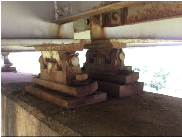
Bearing condition @ Bent 1.
