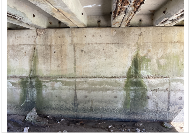
2 Full height vertical crack @ abutment 2.
