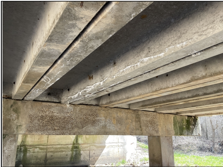
Span 1 - Longitudinal cracks with heavy efflorescence to Girders of Unit 3.
