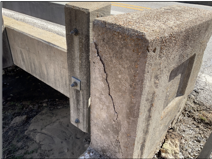
All concrete posts on Left side have collision damage.
