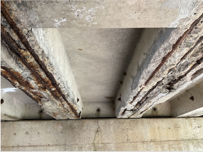
Span 2 - Large areas of delamination & cracks with rust stains to Units 1 - 7.
