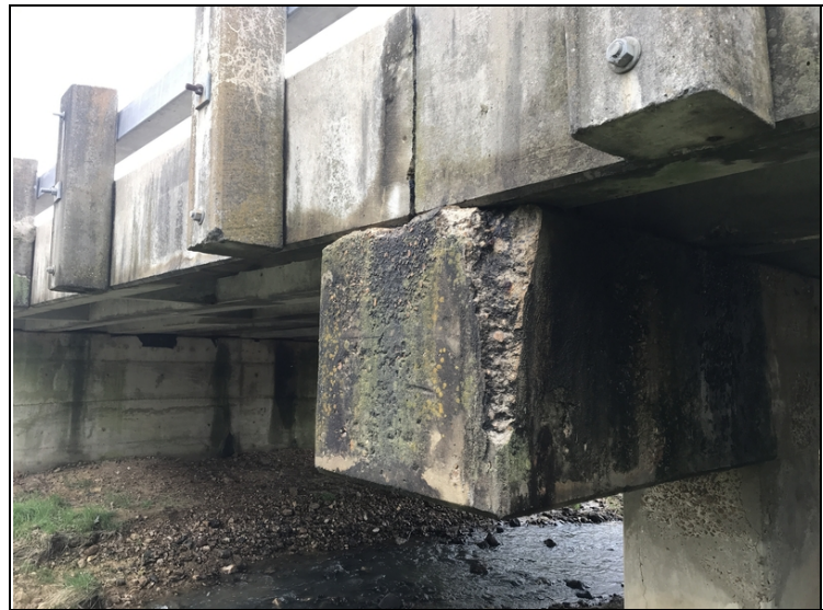
Cracking, Spalls and delaminated areas to Cap at Bent 1.
