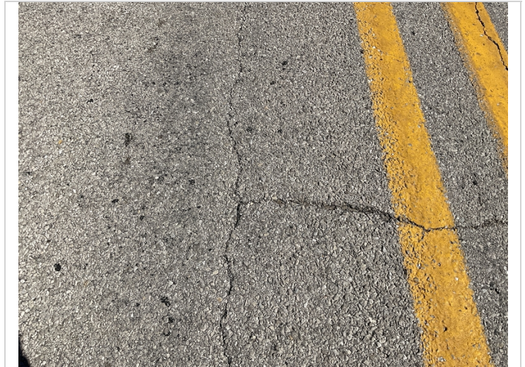
Typical cracks to wearing surface.
