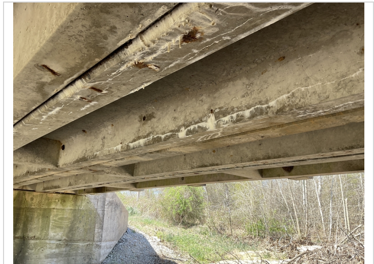
Efflorescent map cracking to girder @ Unit 3 @ Span 1.
