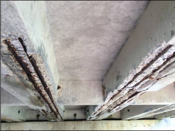
Unit 6 - Spall with 36' rebar exposed.
