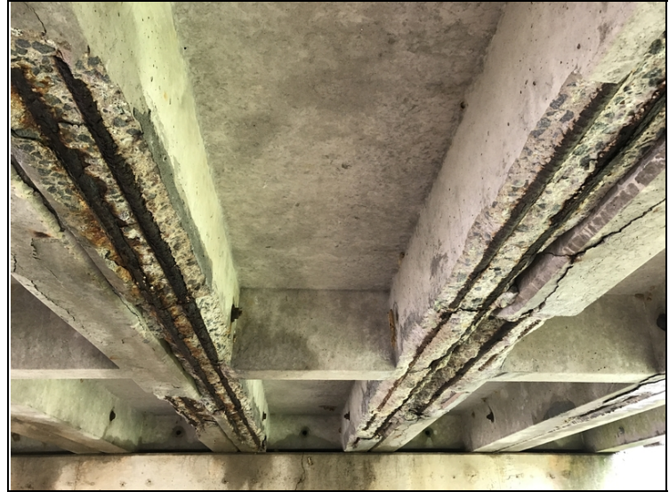
Span 2 - Large spalls with rebar exposed to Girders.
