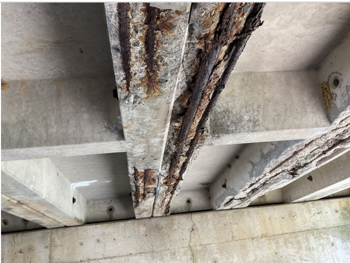
Spalls with rebar exposed to units 1 - 6.
