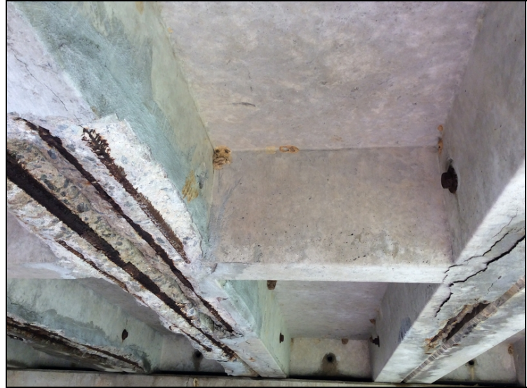
Unit 7 - Spall with 8' rebar exposed.
