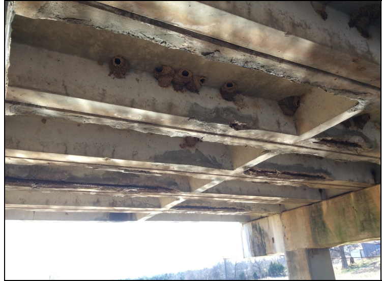
Typical of Spalls with rebar exposed to : Unit 4 at Span 1 Units 3, 4, 5, 6, & 7 at Span 2. Units 4, 5, 6, & 7 at Span 3. Units 2 thru 7 at Span 4 Units 2, 3, 4, 5, 6, & 7 at Span 5. (Span 4)
