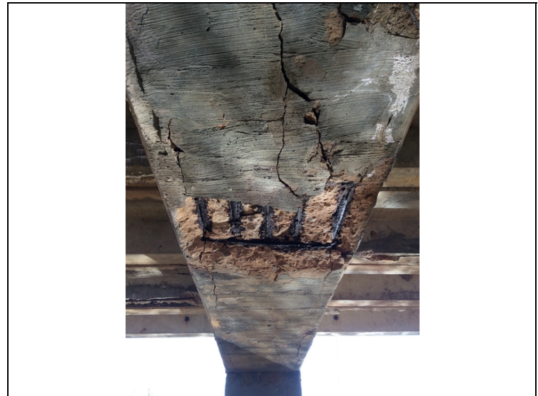
Areas of delaminating, cracking &/or spalls with rebar exposed to caps at Bents 1 - 4.
