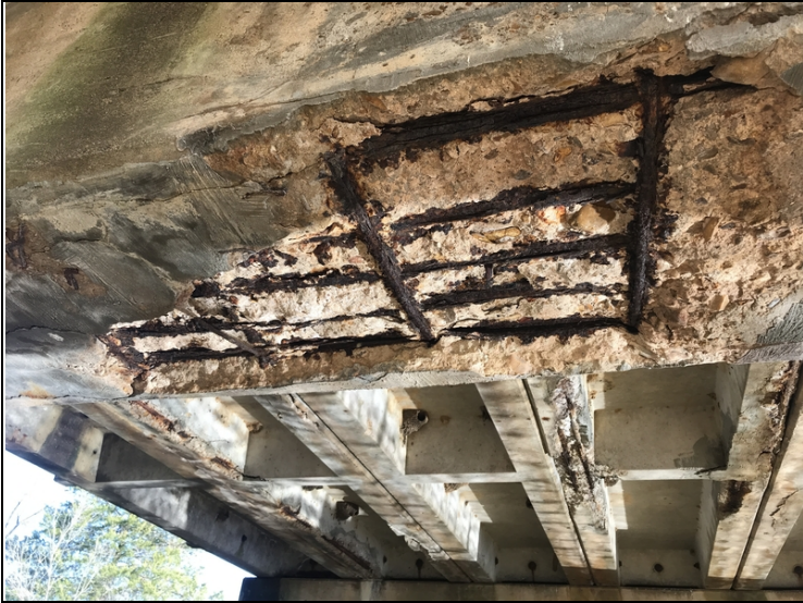
Areas of delaminating, cracking &/or spalls with rebar exposed to caps at Bents 1 - 4. Bent 1.
