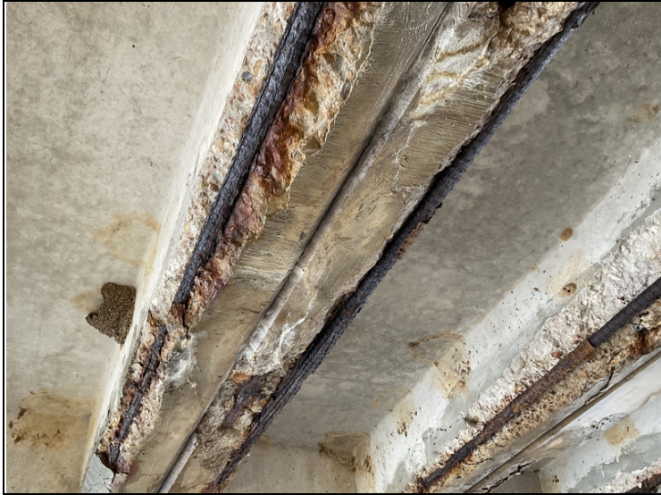
Spalls with rebar exposed with s/l & areas that are not adhered to concrete girders @ Unit 5 @ Span 4.
