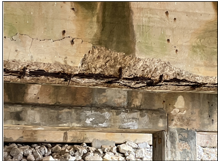
Spalls with rebar exposed with 100% s/l to bottom of cap @ Bent 3.
