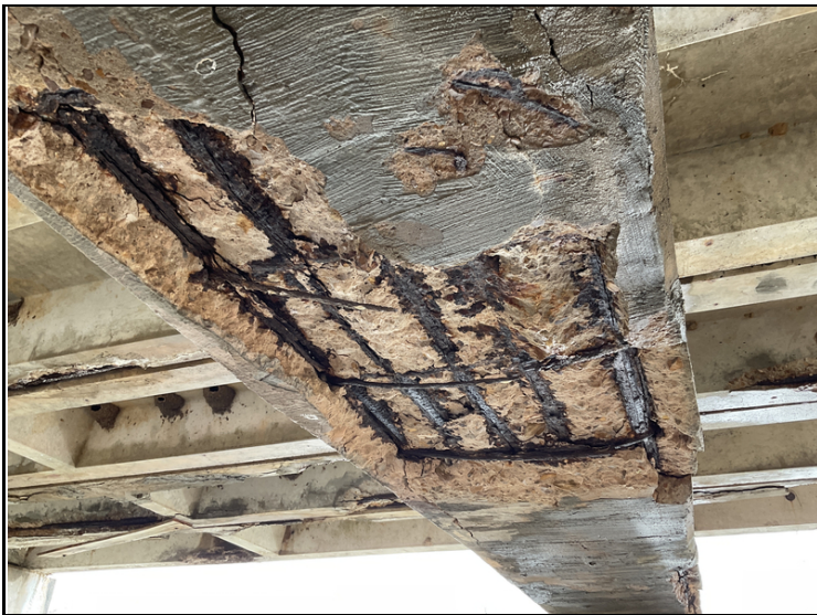
Spalls with rebar exposed with 100% s/l to bottom of cap @ Bent 2.
