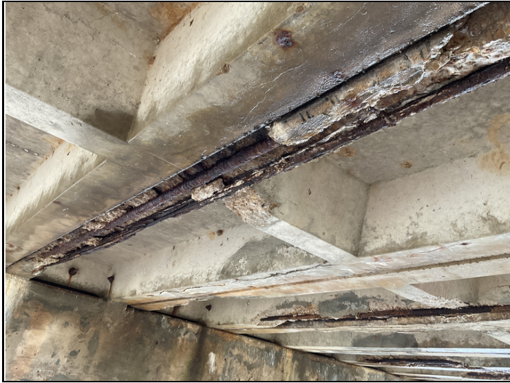
Spalls with rebar exposed with s/l & areas that are not adhered to concrete girders @ Unit 2 @ Span 2.
