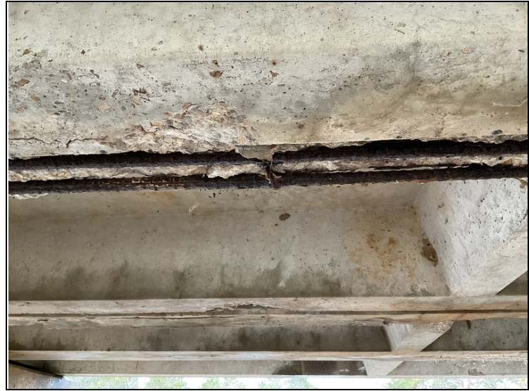
Spalls with rebar exposed with s/l & areas that are not adhered to concrete girders @ Unit 3 @ Span 5.
